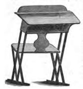
for the same, used in the high school for girls in Newburyport, Mass. The frame is cast iron, to which the seat and desk is attached by screws. The frame is strengthened by a brace extending from each side below the seat.
