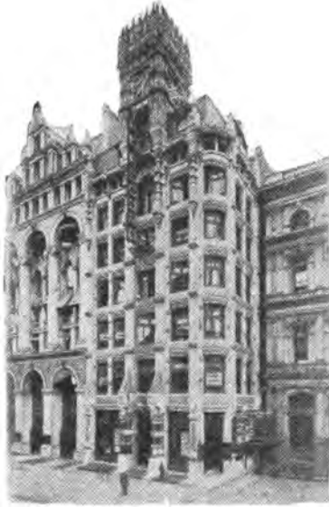
RECORD BUILDING Chestnut Street below Tenth. Courtesy of the Philadelphia Record.
