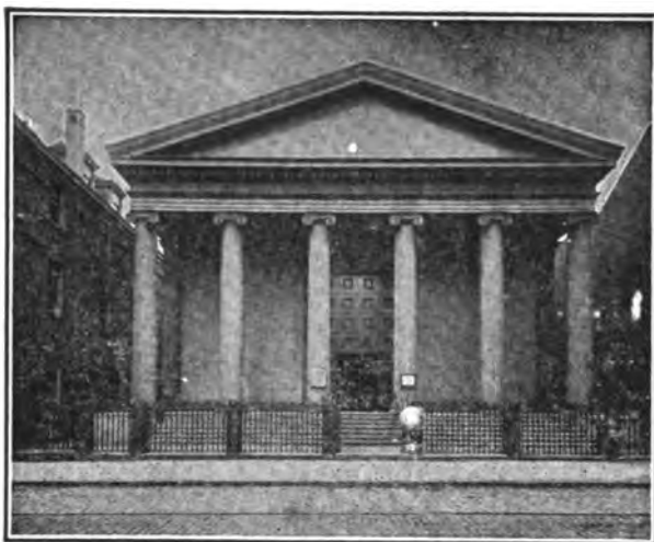
ST. ANDREW'S EPISCOPAL CHURCH Eighth Street above Spruce.
