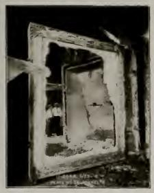
this construction might prevent the spread of a conflagration through a residential district. On the outer side of the studding, which would correspond to the inner side of the wall, No. 24 metal lath was fastened and plas-
