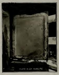
studs and outside of wall. What was left of the studding was charcoal, but the outside of the wall was intact and in a condition to resist more fire.
