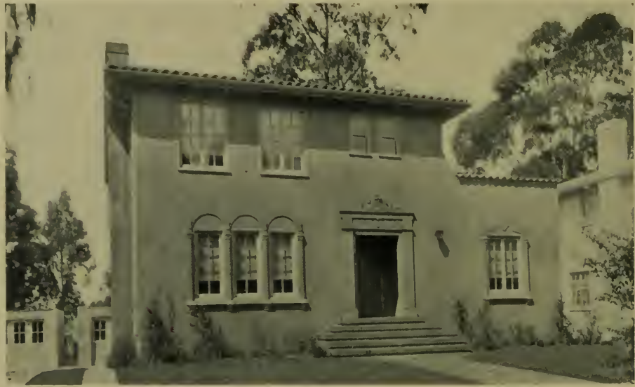
RESIDENCE OF MRS. L. SABINE, ST. FRANCIS WOOD, SAN FRANCISCO S. A. BORN BUILDING CO., DESIGNERS & BUILDERS, SAN FRANCISCO
