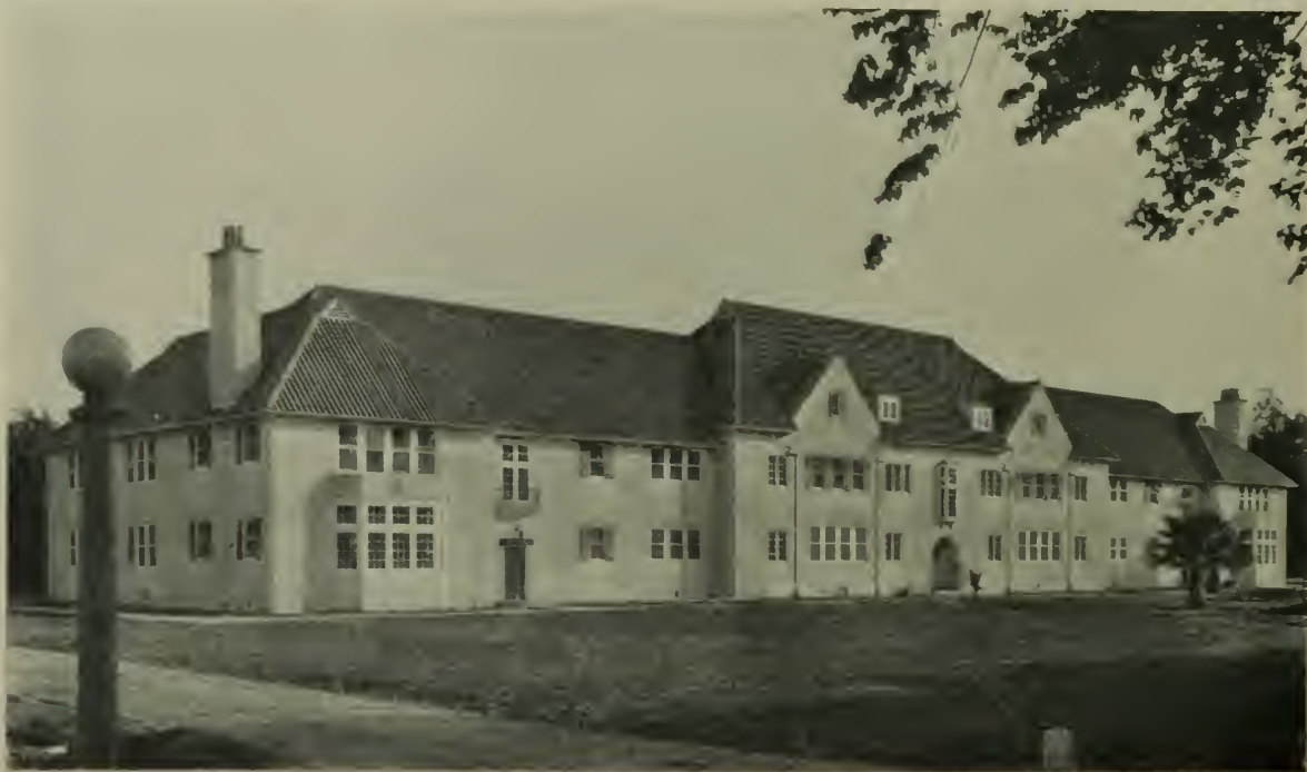
RECEIVING BUILDING, STATE HOSPITAL, STOCKTON, CALIFORNIA Division of Architecture, State of California, Designers
