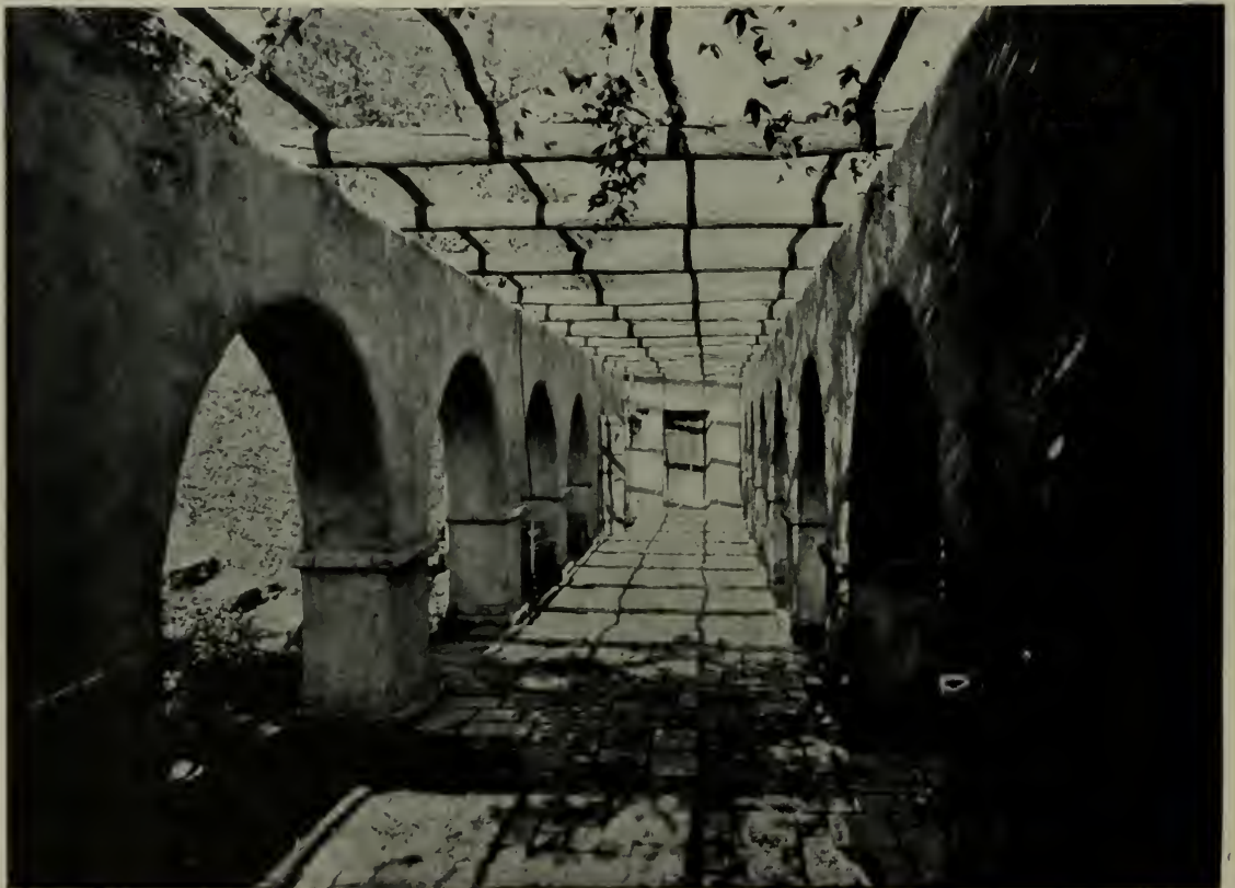
UPPER SERVANTS WING, ROOF TILE MADE BY HAND ON JOB, THOS. H. INCE RESIDENCE. ROY SELDON PRICE, ARCHITECT LOWER ARBOR FROM GARDNER'S COTTAGE TO CHAUFFEUR'S ROOMS, THOS. H. INCE RESIDENCE
