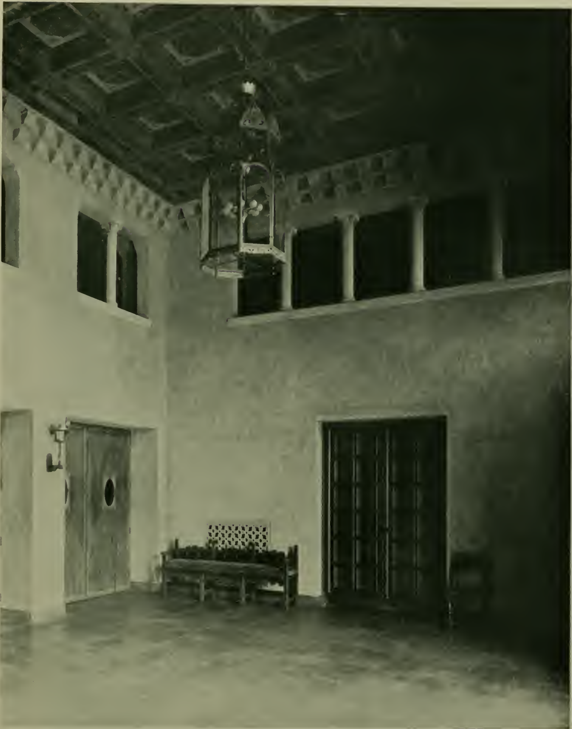
ENTRANCE LOBBY, THE FRIDAY MORNING CLUB, LOS ANGELES, CALIFORNIA. ALLISON & ALLISON, ARCHITECTS
