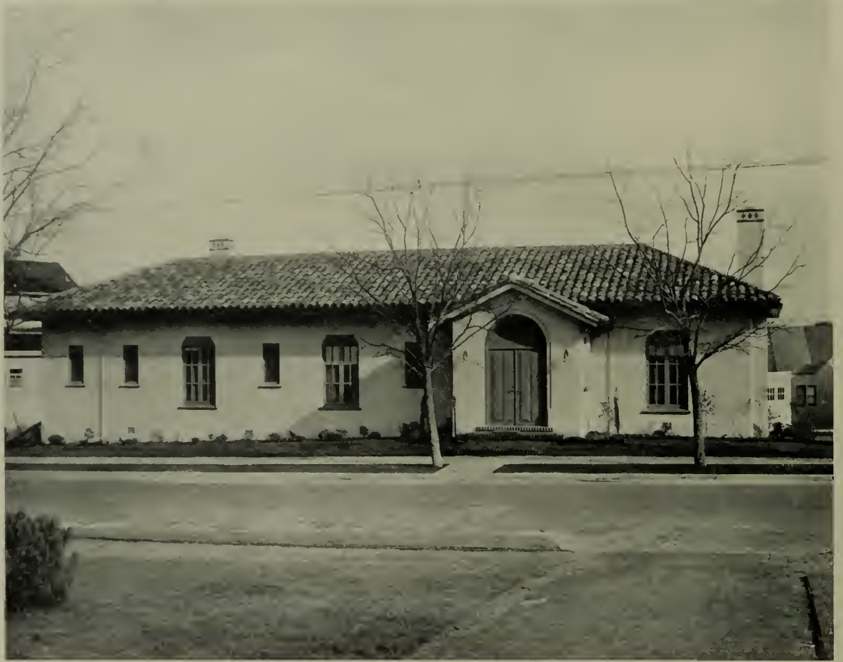
HOME OF MR. RUSSELL SELFRIDGE, SAN MATEO PARK, CALIFORNIA. JULIA MORGAN, ARCHITECT
