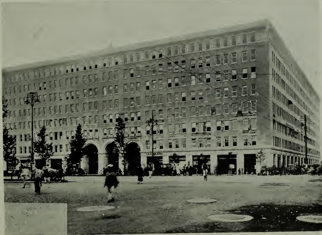
TOP: YUSEN BUILDING, TOKIO, STEEL FRAME STRUCTURE, FACED WITH TERRA COTTA, BACKED WITH COMMON BRICK. BOTTOM: MARUNOUCHI BUILDING, TOKIO, STEEL FRAME STRUCTURE, BRICK CURTAIN WALLS, TERRA COTTA TRIM.
