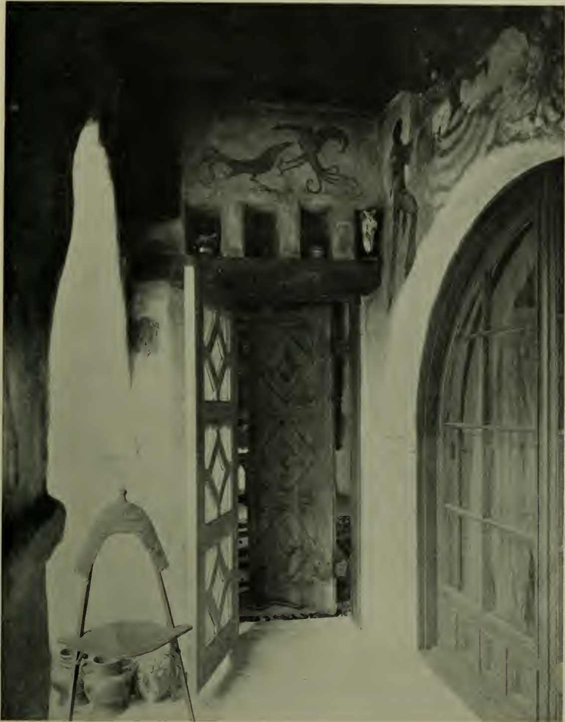
DOOR TO PATIO. POTTERY MADE ON JOB BY MEXICANS. THOS. H. INCE RESIDENCE. ROY SELDON PRICE, ARCHITECT
