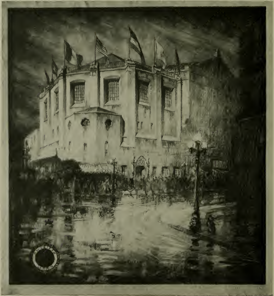
AMERICAN LEGION AUDITORIUM, SAN FRANCISCO, MORROW & GARREN, ARCHITECTS
