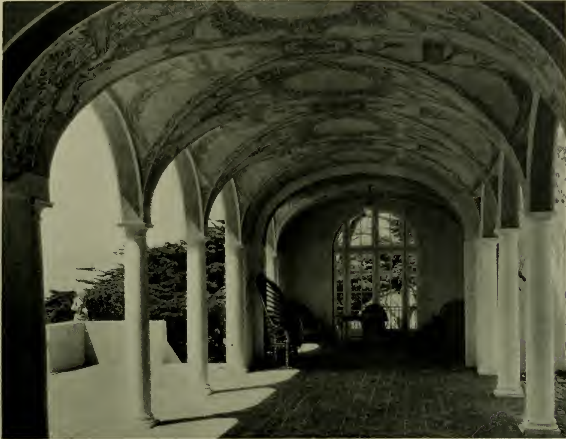
LOGGIA, C. W. CLARK RESIDENCE, PEBBLE BEACH, BAKEWELL &amp; BROWN, ARCHITECTS
