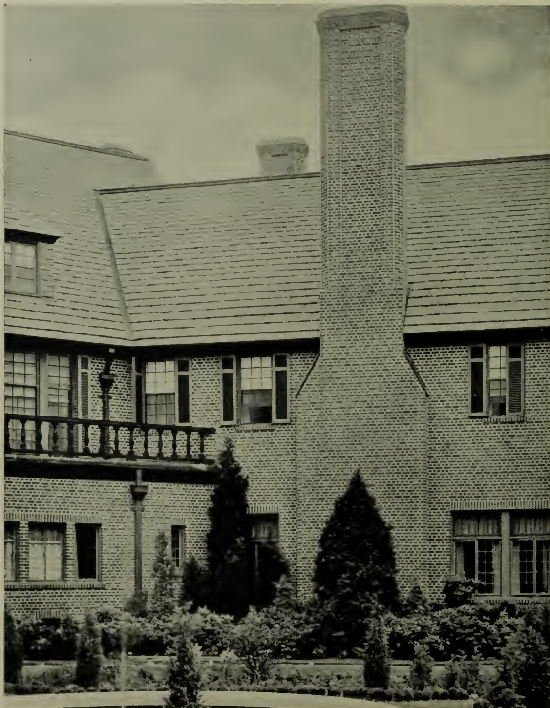
Detail of Residence, Locust Valley, Long Island. Kenneth Murchison, Architect
