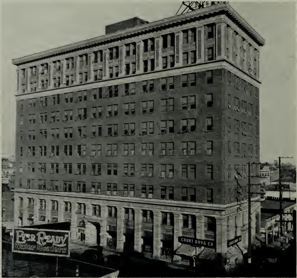
NOERENBERG & JOHNSON, ARCHITECTS, 401 L. A. RAILWAY BUILDING, LOS ANGELES. ARENZ-WARREN COMPANY, PAINTERS 2121 WEST PICO STREET, LOS ANGELES
