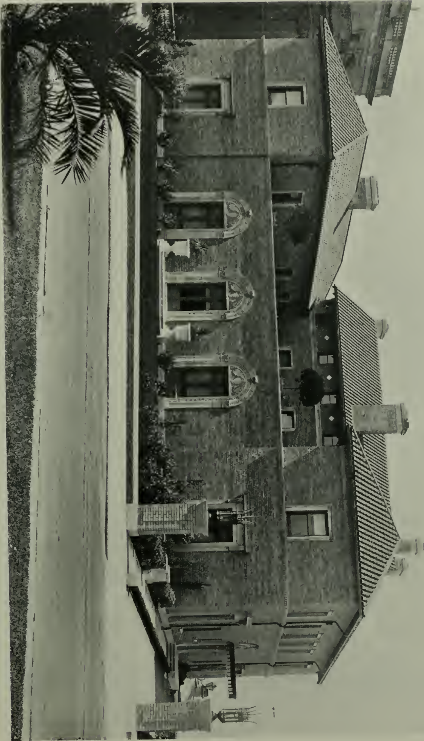
RESIDENCE OF MISS MARY L. PHELAN, SAN FRANCISCO, CHARLES PETER WEERS, ARCHITECT, SAN FRAN- CISCO, CALIFORNIA
