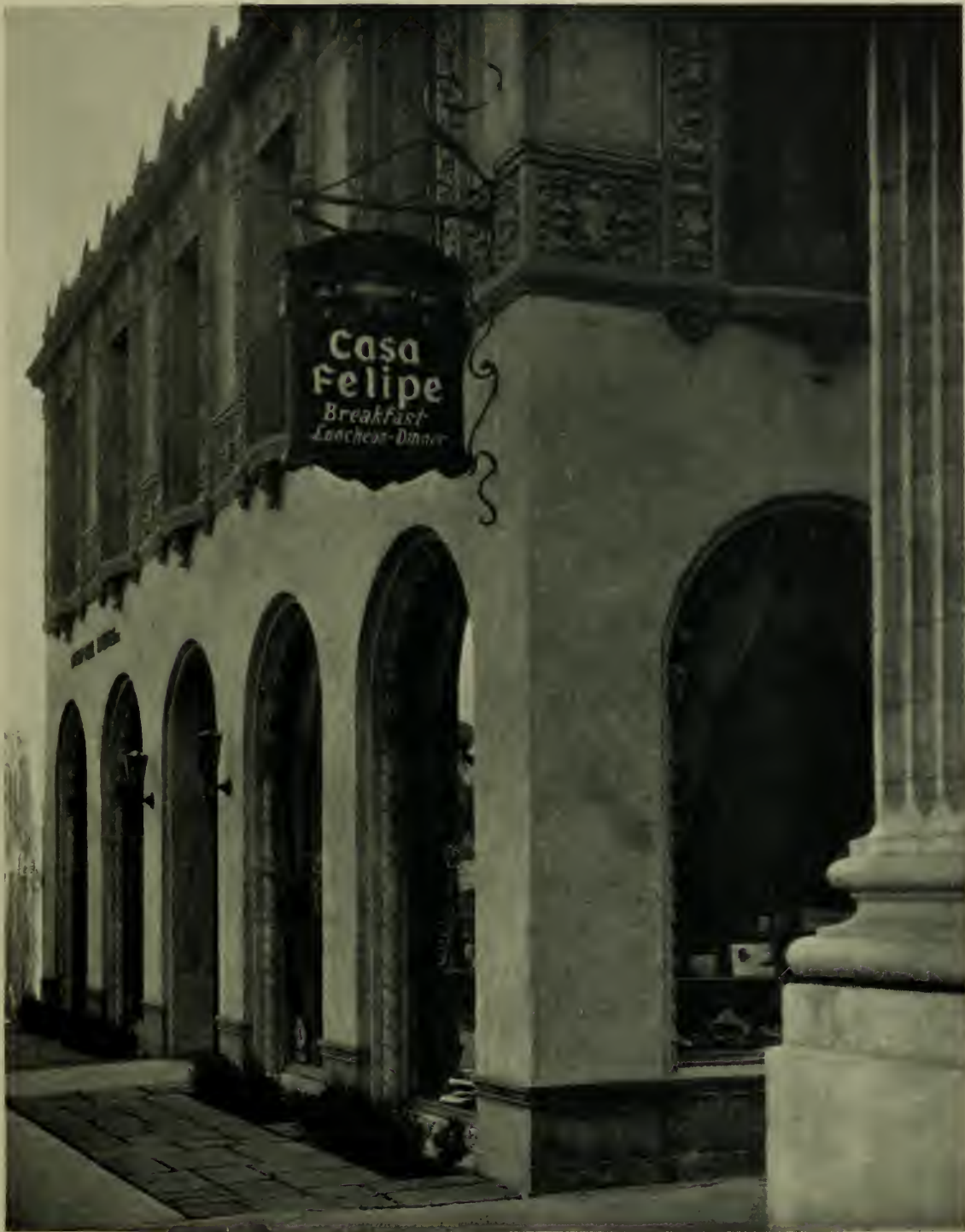
CORNER DETAIL. BUILDING FOR MRS. J. W. MCKINLEY, LOS ANGELES. MORGAN, WALLS & CLEMENTS, ARCHITECTS.
