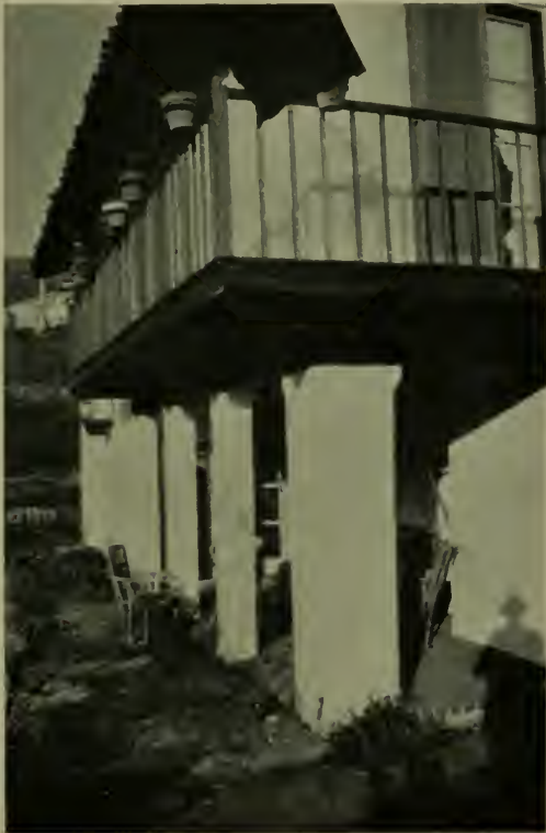
PORCH AND BALCONY, HOME OF HENRY SWIFT, BERKELEY, CALIFORNIA. ROLAND I. STRINGHAM, ARCHITECT
