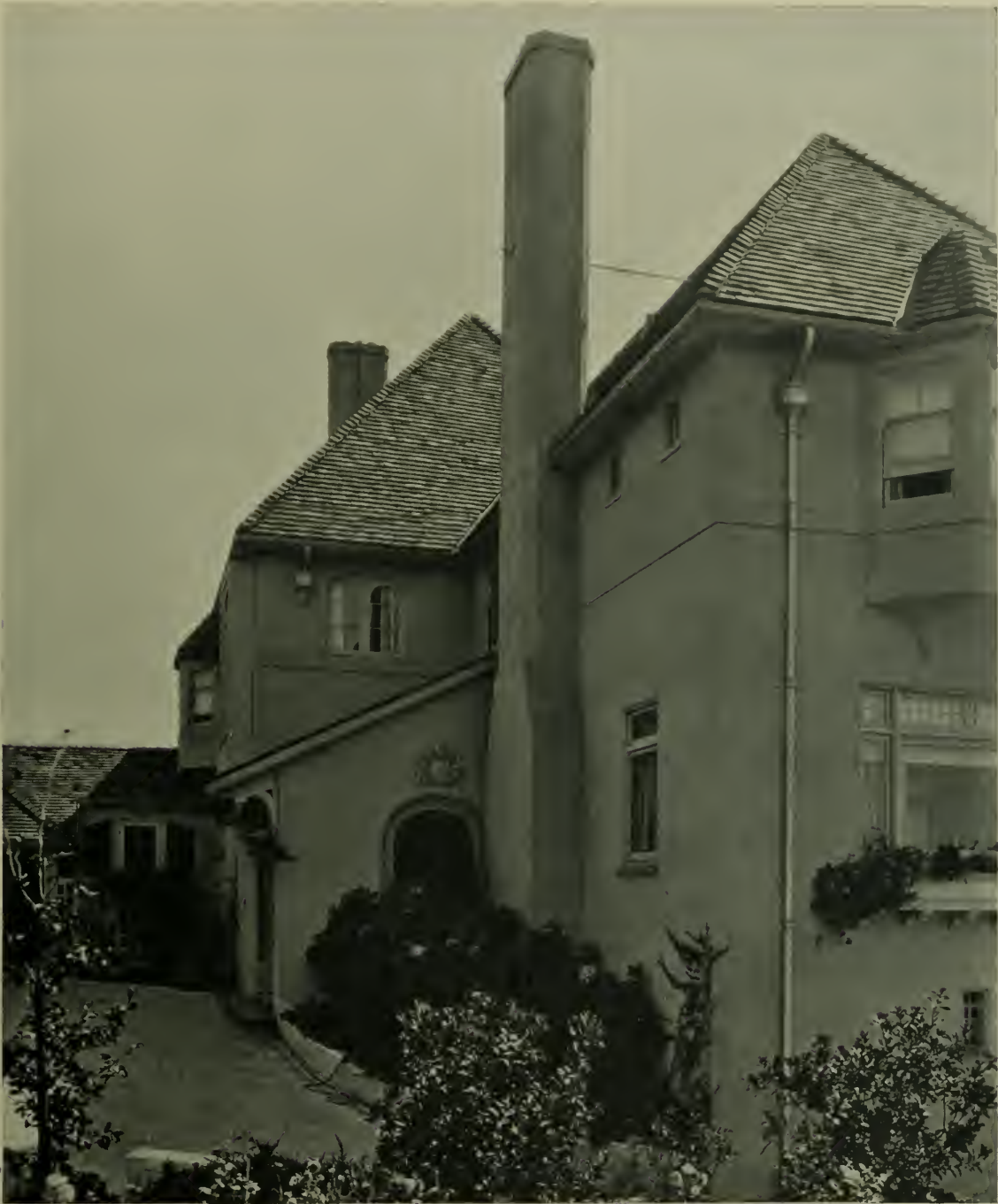
RESIDENCE OF G. A. MATTERN, CLAREMONT, CALIFORNIA, LOUIS M. UPTON, ARCHITECT
