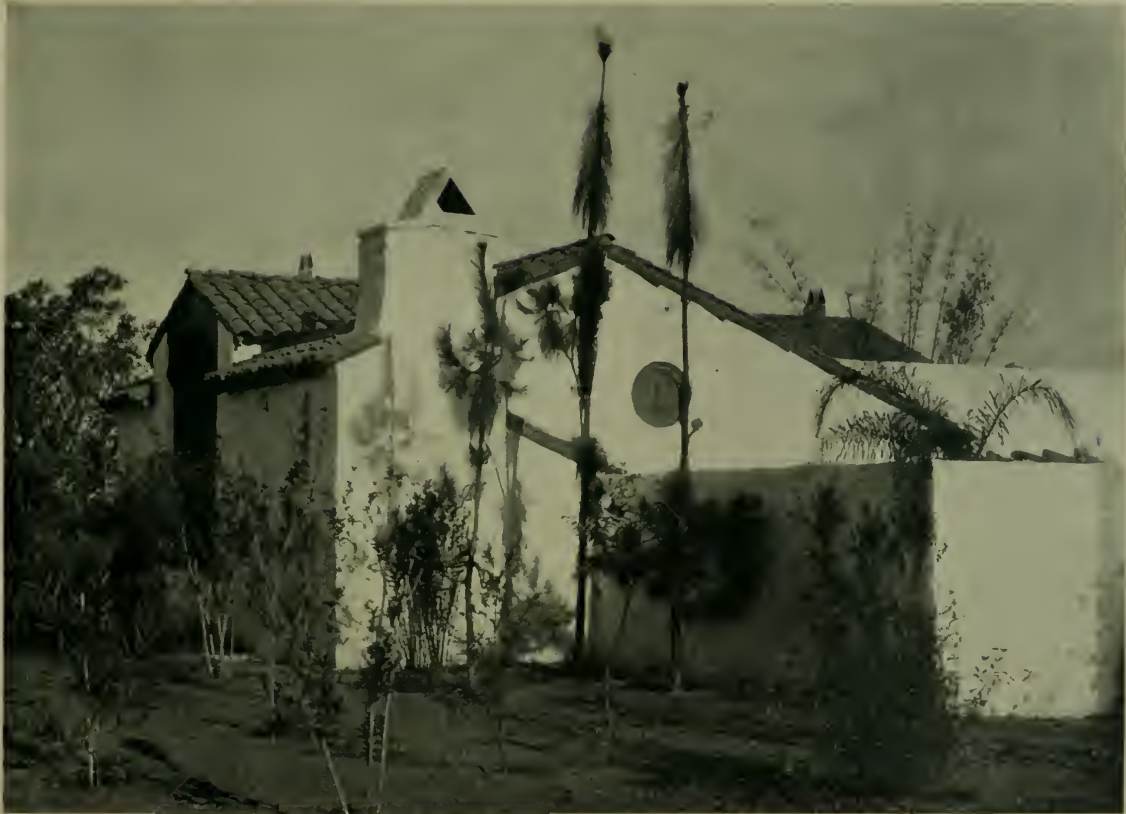
UPPER ENTRANCE GATEWAY, LOWER STUDIO OF JAS. SCRIPPS BOOTH, PASADENA MARSTON & VAN PELT, ARCHITECTS
