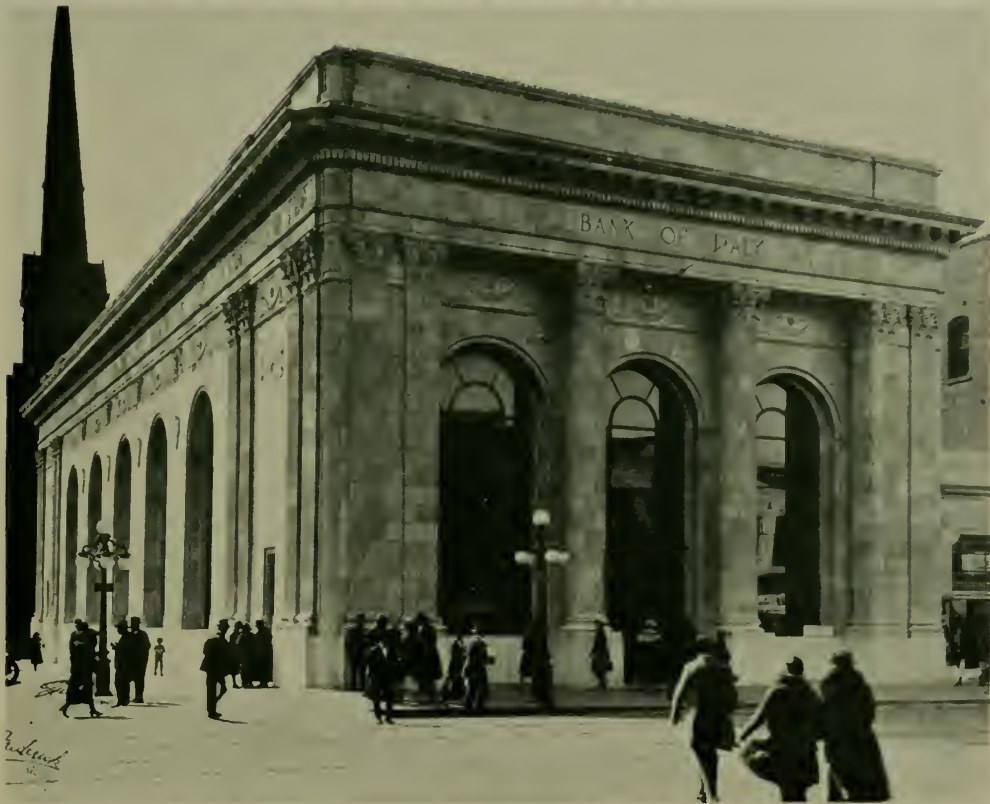
BANK OF ITALY, SACRAMENTO, CALIFORNIA. GEORGE C. SELLOM AND COMPANY, ARCHITECTS
