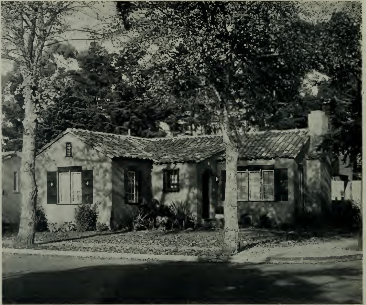
RESIDENCE OF ERNEST INGOLD, 1100 BALBOA AVENUE, BURLINGAME, CALIFORNIA H. C. BAUMAN, ARCHITECT
