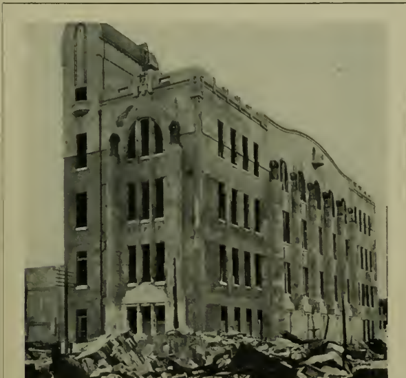
YOKOHAMA TELEPHONE BUILDING. TALLEST BUILDING IN YOKOHAMA. DAMAGED BY SKELETON CONSTRUCTION BUILDING LACKED STIFFNESS IN NARROW DIRECTION
