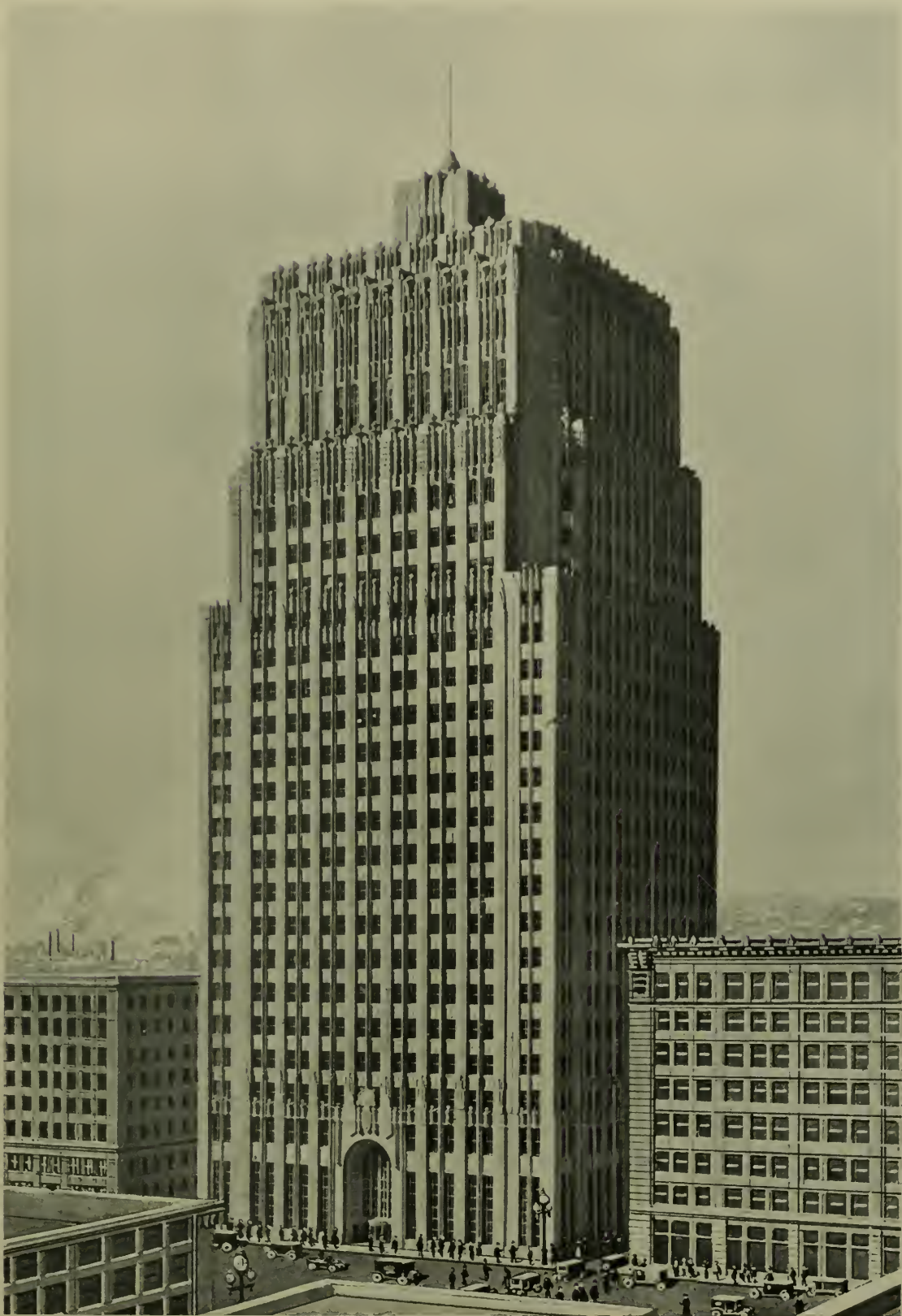
PACIFIC TELEPHONE AND TELEGRAPH COMPANY BUILDING, SAN FRANCISCO, CALIFORNIA J. R. MILLER AND T. L. PFLUEGER, ARCHITECTS. A. A. CANTIN, ASSOCIATE
