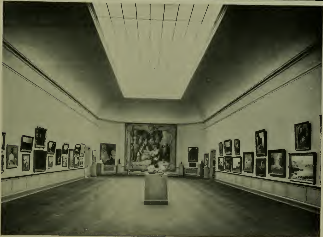
CALIFORNIA PALACE OF THE LEGION OF HONOR. GEORGE A. APPLGARH, ARCHITECT ABOVE—CENTRAL GALLERY. BELOW—TYPICAL GALLERY
