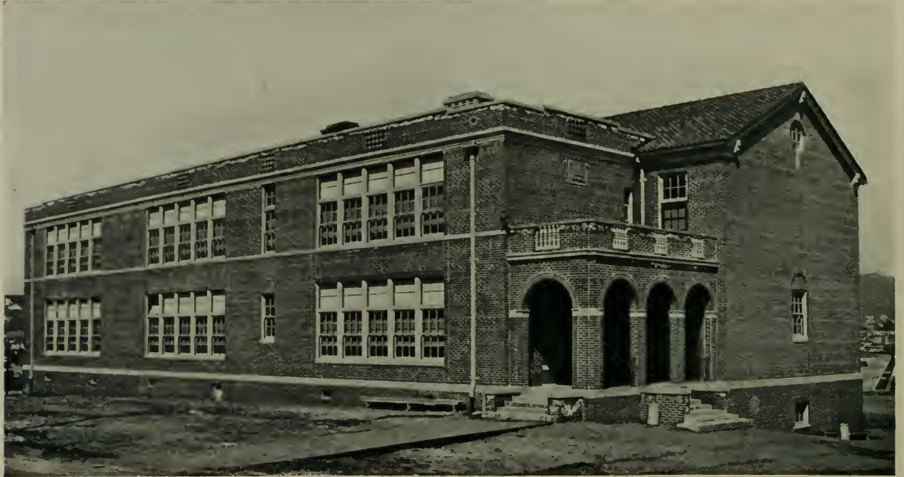
TOLAND WAY SCHOOL, LOS ANGELES, WILLIAM STACKO, CONTRACTOR
