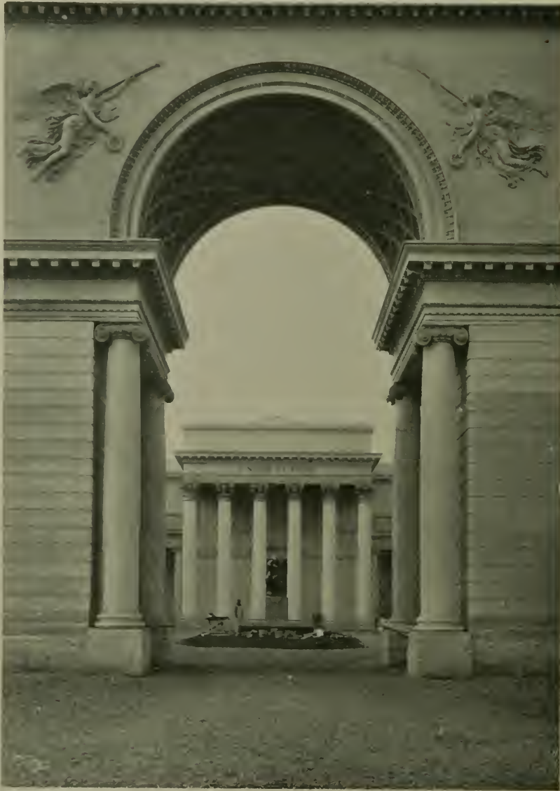
PORTALS OF CALIFORNIA PALACE OF THE LEGION OF HONOR George A. Applegarth, Architect. R. McLeran & Co., General Contractors
