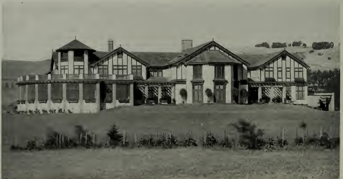
MAIN FACADE, BERESFORD COUNTRY CLUB; SYLVAIN SCHNAITTACHER AND G. ALBERT LANSBURGH, ASSOCIATE ARCHITECTS
