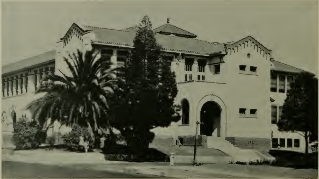
GRANT SCHOOL, WILTON PLACE AND HAROLD WAY, LOS ANGELES, CALIFORNIA Jeffery & Schaefer, Architects. R. G. Blessing, Roofing Contractor J. A. Hill Construction Co., General Contractors.
