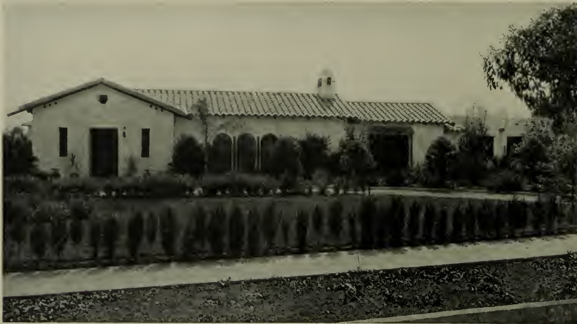
RESIDENCE OF ARTHUR ROSSON, BEVERLY HILLS, CALIFORNIA. BUILT OF ADOBE-GRANADA. TILED DETAILS OF CHIMNEY-GRILL, ETC., TAKEN FROM AUTHENTIC EXAMPLES OF OLD SPAIN
