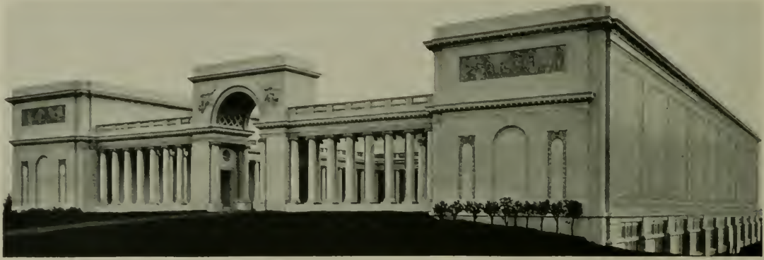
CALIFORNIA PALACE OF THE LEGION OF HONOR, LINCOLN PARK, SAN FRANCISCO George A. Applegarth, Architect. Ralph McLeran & Co., Builders. Walls of Dickey Mastertile
