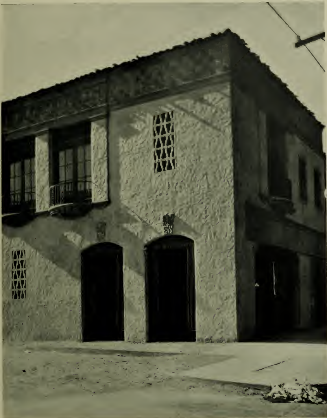
CORNER DETAIL. BILLOCKE ESTATE BUILDING, LOS ANGELES. MORGAN, WALLS & CLEMENTS, ARCHITECTS
