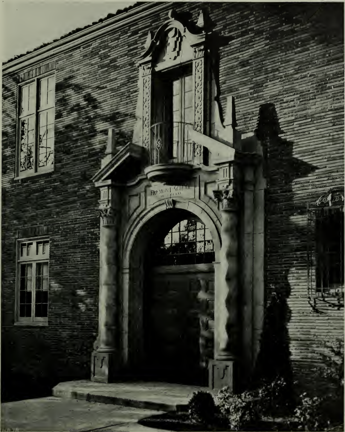
MAIN ENTRANCE, FREMONT SCHOOL, SACRAMENTO. HEMMINGS-PETERSEN-HUDNUTT, INC., ARCHITECTURAL AND ENGINEERING COMMISSION, DEAN AND DEAN, ARCHITECTS, DESIGNERS AND SUCCESSORS, SACRAMENTO, CALIFORNIA
