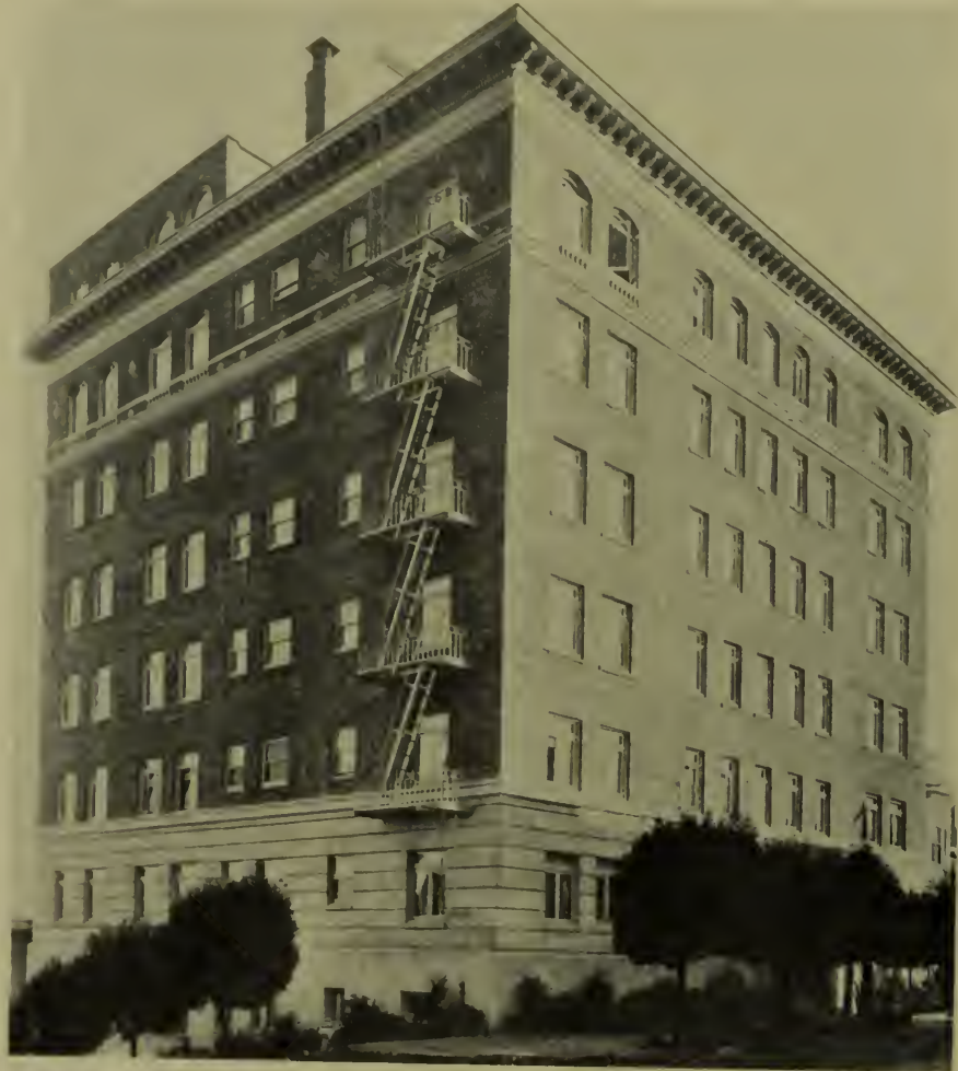
BRICE FAIR APARTMENTS, SAN FRANCISCO. E. E. YOUNG, ARCHITECT. M. A. LITTLE, CONTRACTOR. GEORGE BONNELL, PAINTER
