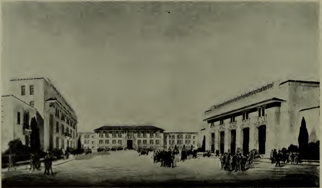
BERKELEY HIGH SCHOOL FROM NORTH, WILLIAM C. HAYS, ARCHITECT
