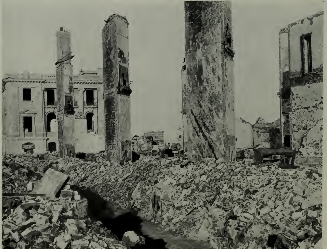
VIEW OF RUINS, SHOWING SALVAGEABLE MATERIAL
