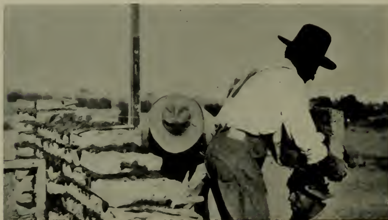
MEXICAN WORKMEN LAYING ADOBE BRICKS
