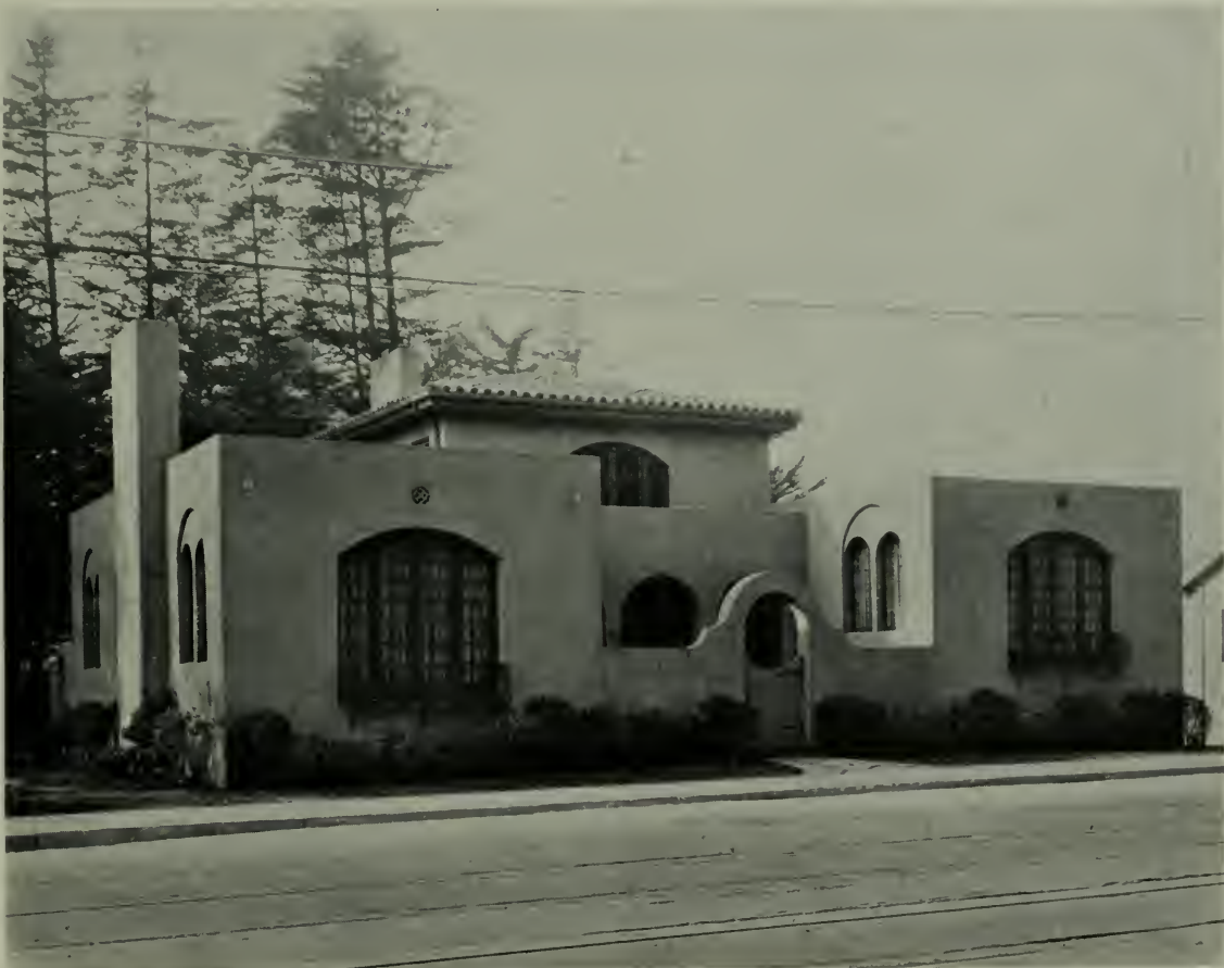
AN ADAPTATION OF MODERN SPANISH ARCHITECTURE IN HOLLOW TILE INGLESIDE TERRACE, SAN FRANCISCO, CALIFORNIA
