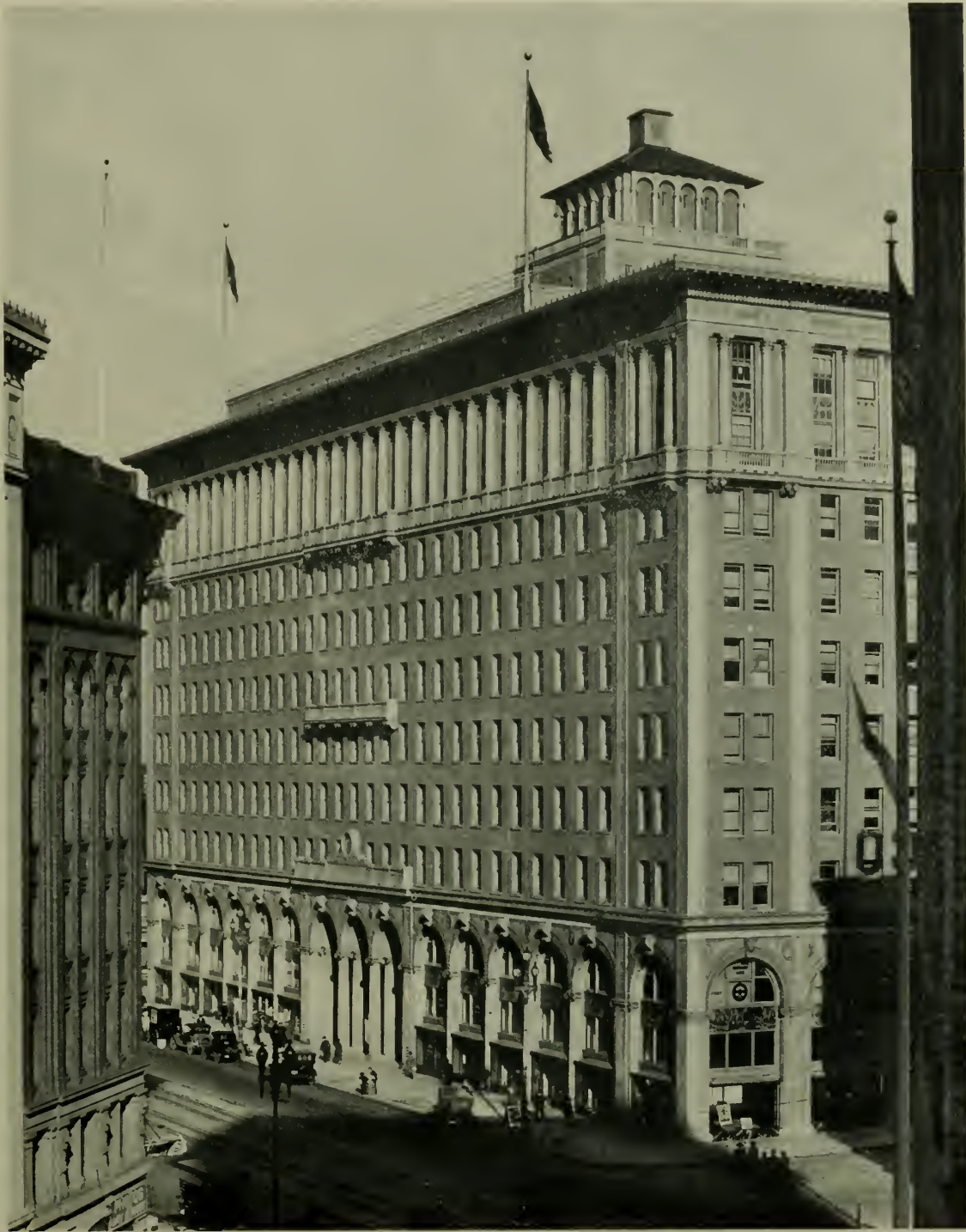
SOUTHERN PACIFIC BUILDING, SAN FRANCISCO, BLISS & FAVILLE, ARCHITECTS
