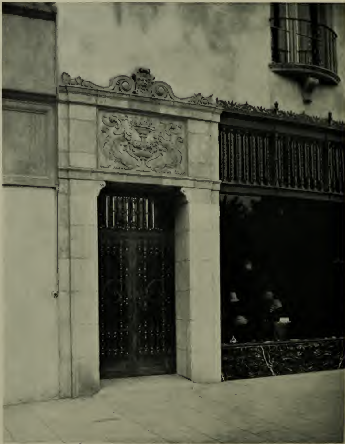
ENTRANCE DETAIL. BUILDING FOR MR. SPENCER THORPE, LOS ANGELES. MORGAN, WALLS & CLEMENTS, ARCHITECTS
