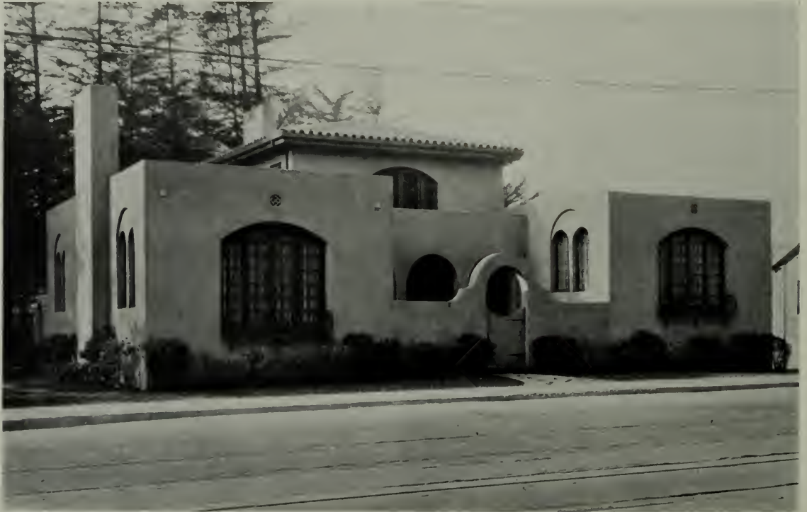
AN INGLESIDE TERRACE RESIDENCE OF STUCCO-DICKEY MASTER TILE
