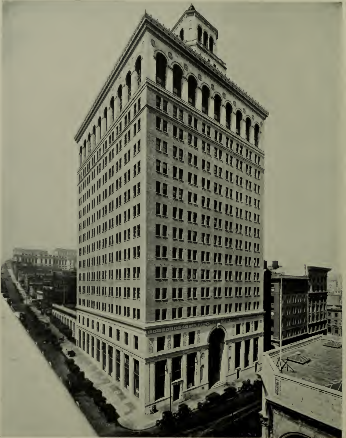
CALIFORNIA COMMERCIAL UNION BUILDING, SAN FRANCISCO, GEO. W. KELHAM, ARCHITECT
