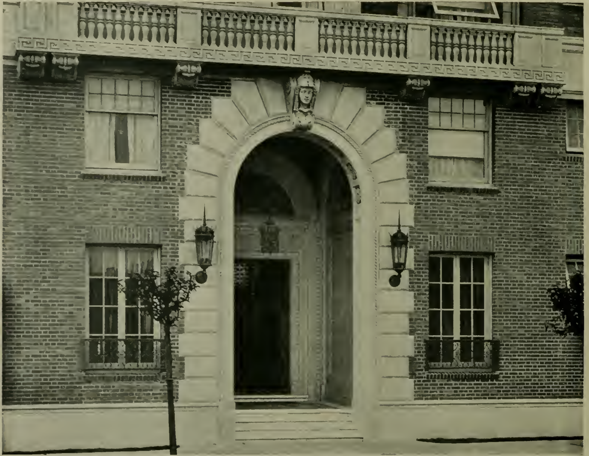
HUNTINGTON APARTMENTS, SAN FRANCISCO, CALIFORNIA. WEEKS & DAY, ARCHITECTS
