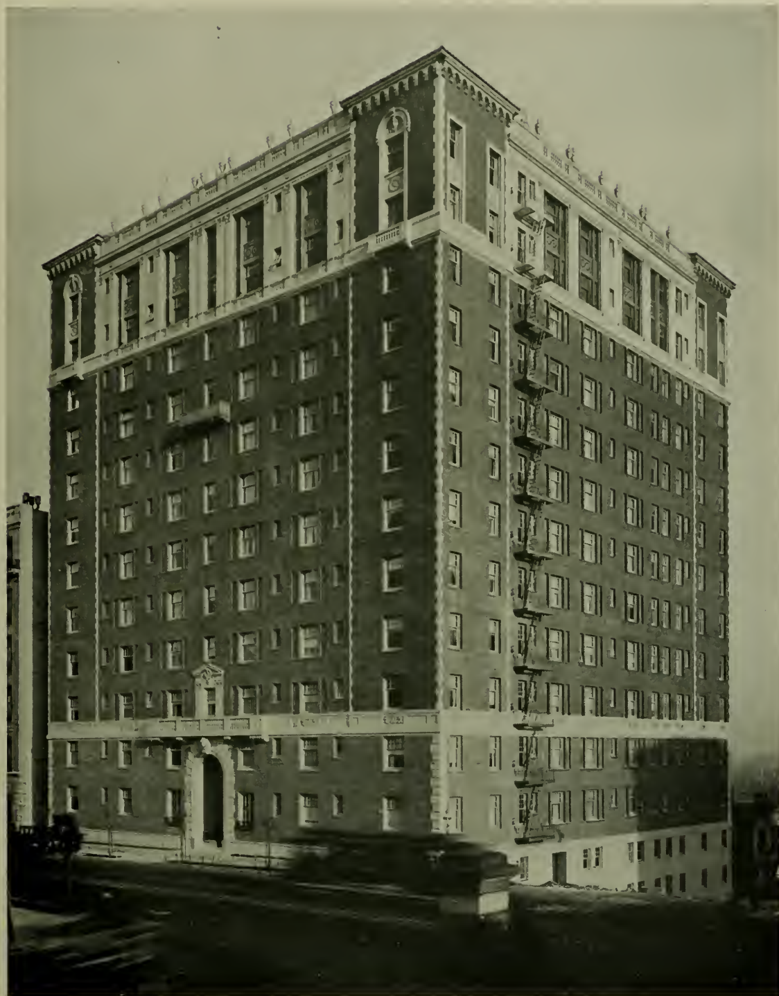
HUNTINGTON APARTMENTS, SAN FRANCISCO, WEEKS AND DAY, ARCHITECTS
