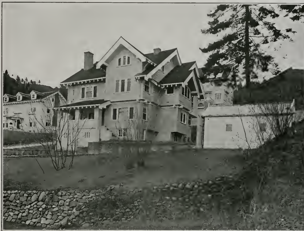
Side Elevation, Residence of Mr. Isaac L. White Mr. Edward T. Root, Architect, Portland
