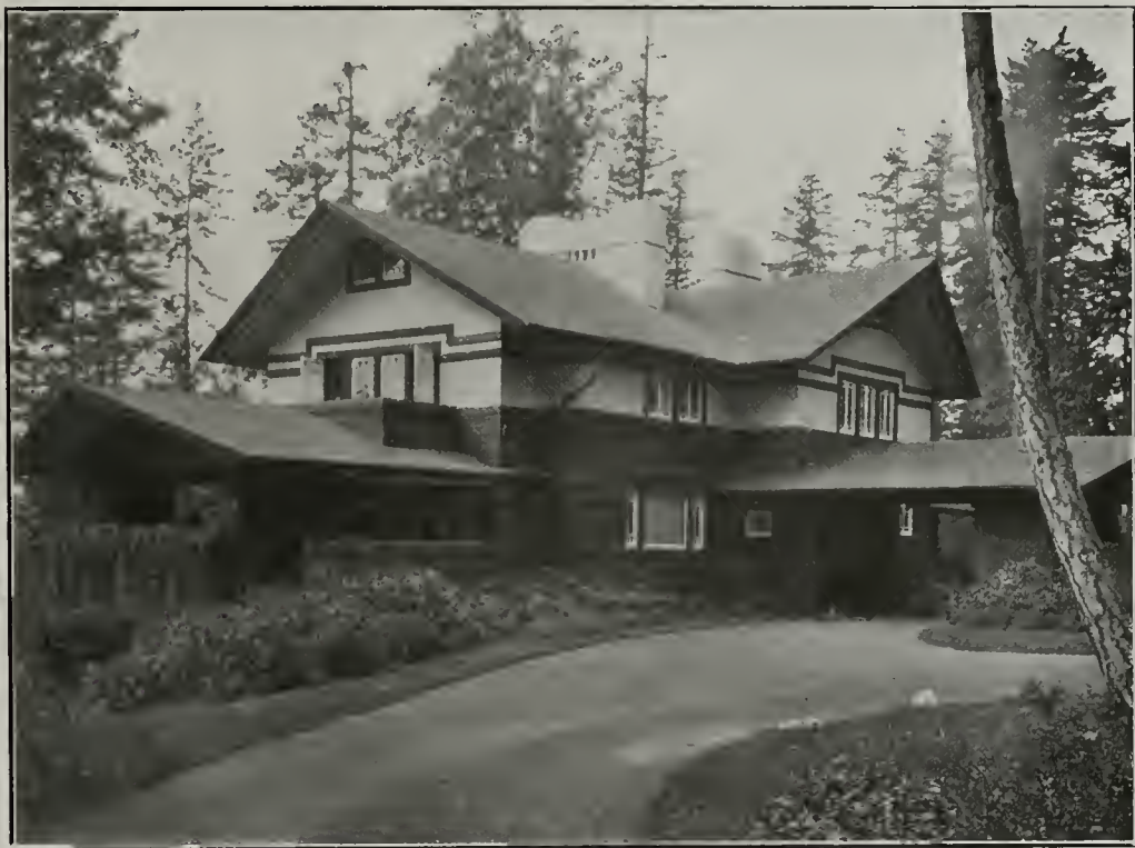
Side Elevation, Country Residence for Mr. C. H. Clarke Willatzen & Byrne, Architects, Seattle, Wash.
