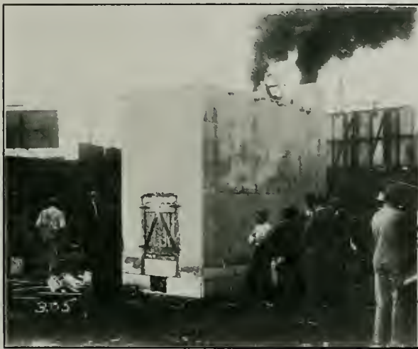
Showing building forty minutes after fire started
