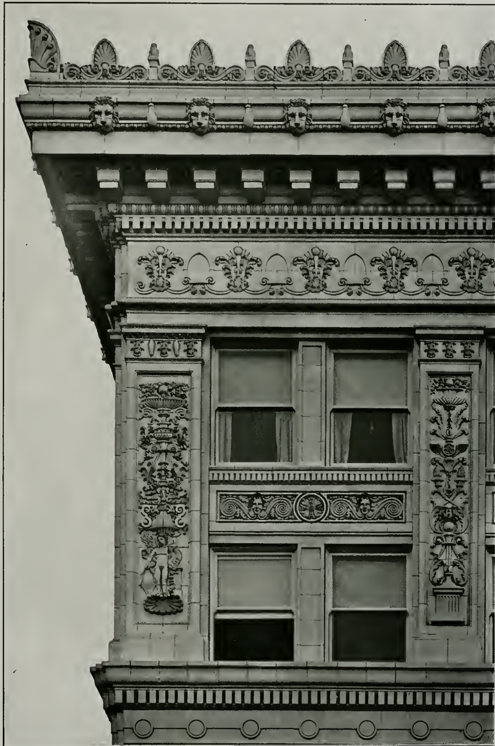
Terra Cotta Detail, Wilcox Building, Portland Whidden & Lewis, Architects
