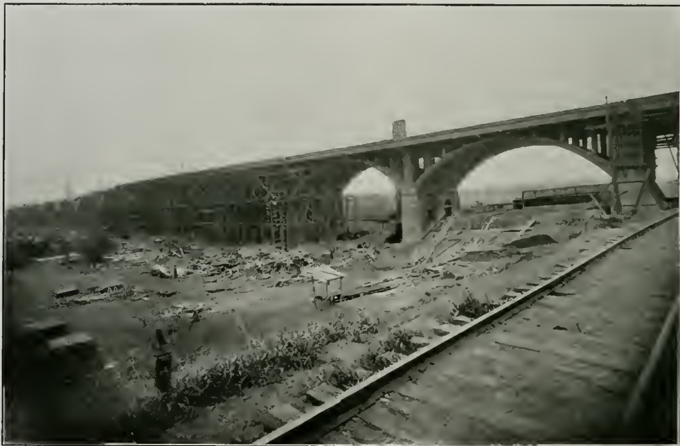
Dallas-Oak Cliff Viaduct, Dallas, Texas. Form Stripped from Archapons. Hedrick & Cochrane, Kansas City, Engineers
