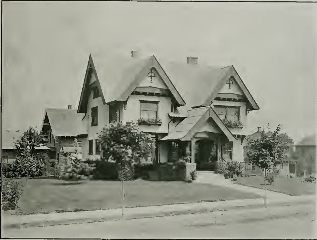
Front Elevation, Residence for Mr. J. D. Tresham Mr. D. L. Williams, Architect, Portland
