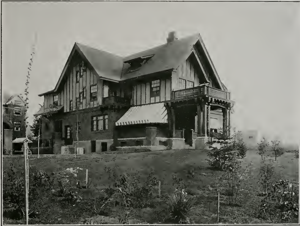
Side Elevation, Residence of Mr. Blaine R. Smith MacNaughton & Raymond, Architects, Portland
