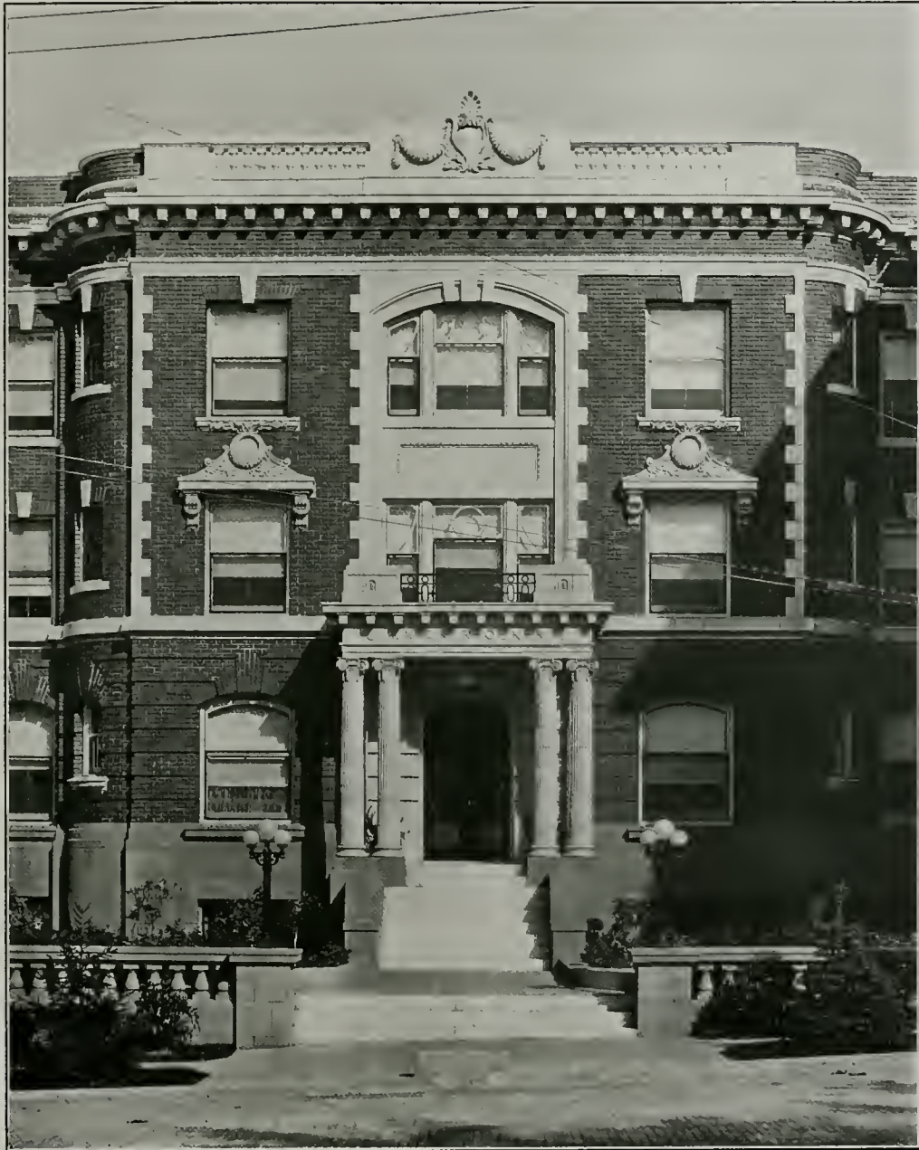
Knickerbocker Apartments, Spokane, Wash. Mr. Albert Held, Architect
