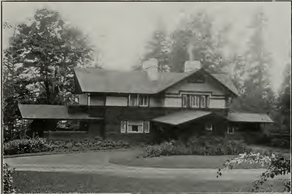
Front Elevation, Country Residence for Mr. C. H. Clarke Willatzen & Byrne, Architects, Seattle, Wash.
