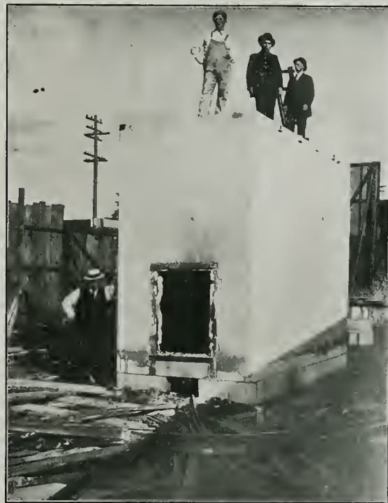
After the fire and water test. Demonstrating unimpaired strength of roof and walls and showing in foreground steel grate rails warped and twisted by heat
