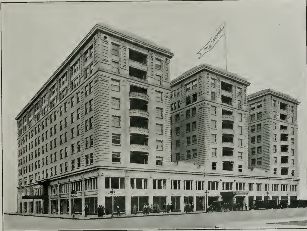
Hotel Multnomah, Portland H. Hanselmann, Architect
