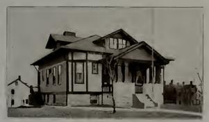
Road and side covered with Asbestos "Century" Shingles Bungalow owned by W. F. Crawford, Cincinnati, Ohio.
