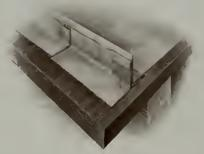
FIG. F.—STANDING-SEAM TIN ROOFING
