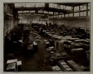
General view of new tinning department, showing the excellent lighting facilities. All handling of material done by overhead traveling scane. The tinning stacks are located in the recesses along either side of the finishing
