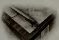
FIG. H.—STANDING-SEAM TIN ROOFING Third operation. Entire seam turned partly over.
