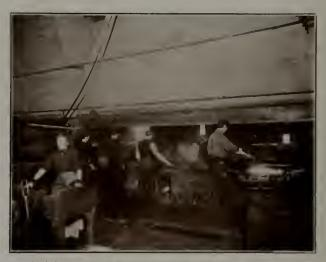
The full "seven open pat, palm oil, hand dipping stack," an exclusive process employed only by the N. A. G. Taylor Co. Used oilly in making the Target and Arrow brand of rooting tim. This is the old time process formerly employed in the company's works in Wales. All work done by hand, four skilled workmen being required. By this process the conting is slowly and thoroughly applied in successive layers on the sheet, resulting in an exceptionally durable rooting plate.
