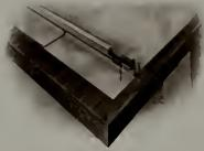
FIG. J.—STANDING-SEAM TIN ROOFING
