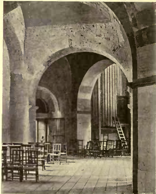
Fig. 719.—Aachen. Palace Chapel. Vaulting in the gallery (796-804).
