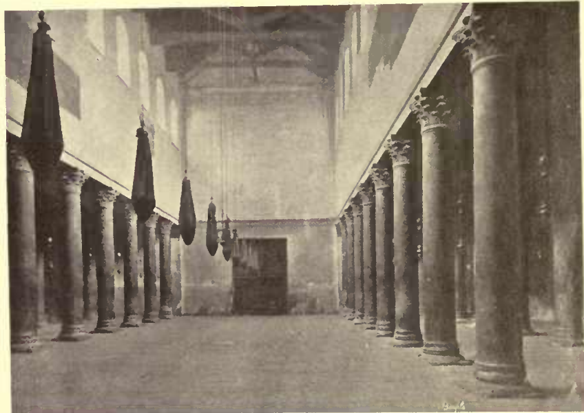
Fig. 385.—Bethlehem. Nave of the Church of the Nativity (327).
