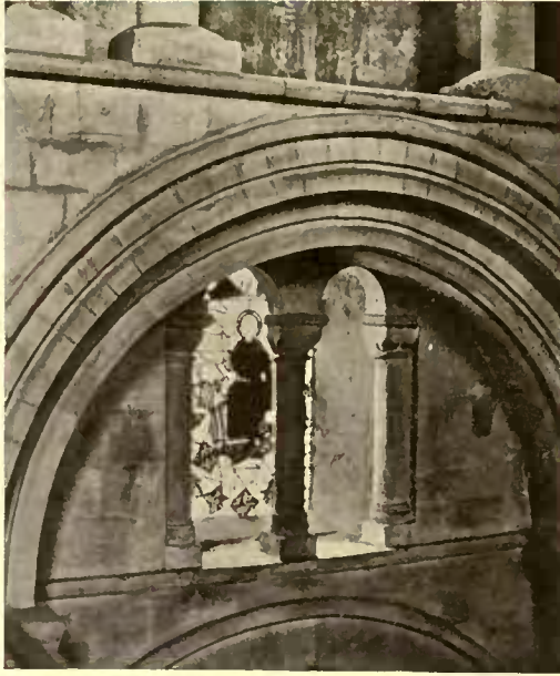
Fig. 670.—Oxford Cathedral. Opening in quasi-triforium (XIIth Century).
