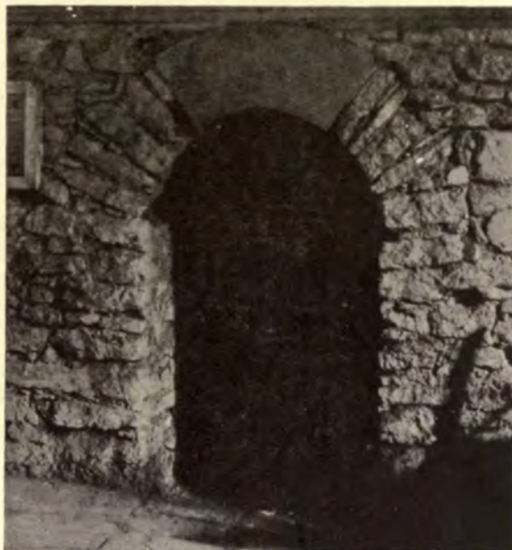
Fig. 567.—Oxford. Cathedral. Frontal arch of lateral apse of old church of St. Frideswide (XIth Century).
