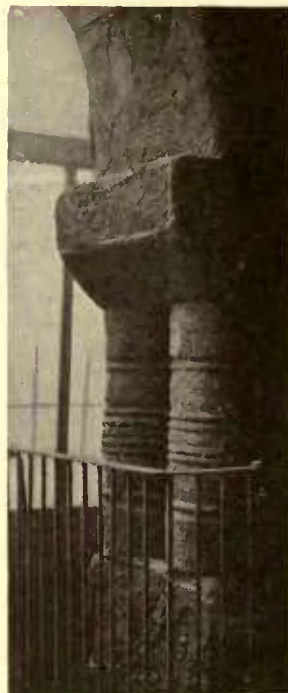
Fig. 526.—Monkwearmouth church. Baluster shafts in outer west door (VIIIth Century).
