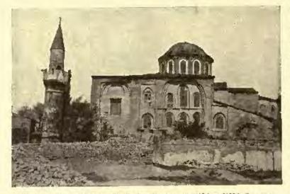
earthquake of 1117 which brought down a considerable portion of the church. The simplicity of the massive restored piers of the present dome. compared with those of the nave, and also the presence of single instead of compound Lombardic pendentives, lead me to think that the dome is original up to the low drum,
