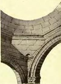
Fig. 275.—Lattakia. Augle raccord in four-faced arch (Hird Century).
