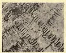
Fig. 363.-Rome. Villa called "Serte Bassi." Detail of ribbed vaulting (Hnd Century).
