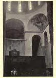
in San Vitale. In the nave they give strength to the barrel vaulting. Substantial buttresses project from the corresponding points of the exterior (Fig. 285). The transverse arches over the aisles carry arched ramping walls which bind the two sets of buttresses together.
