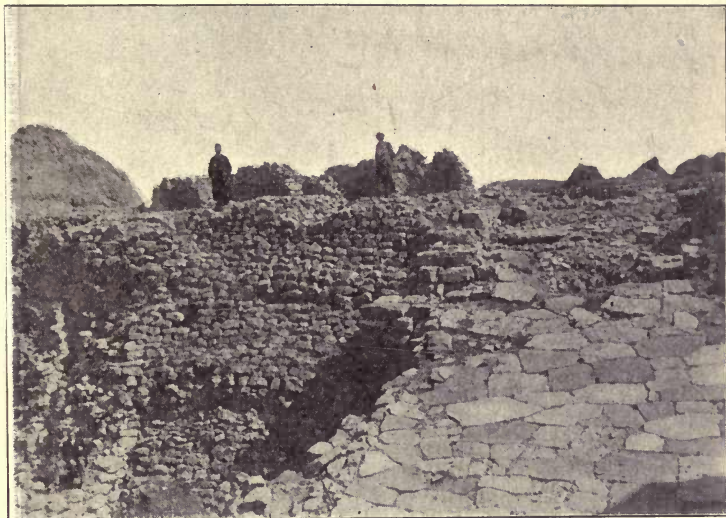
FIG. 337. — Paved road at Troy.
