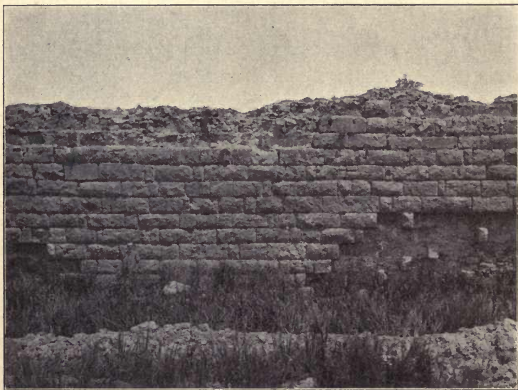
FIG. 13. — Equal coursed masonry at Magnesia.
