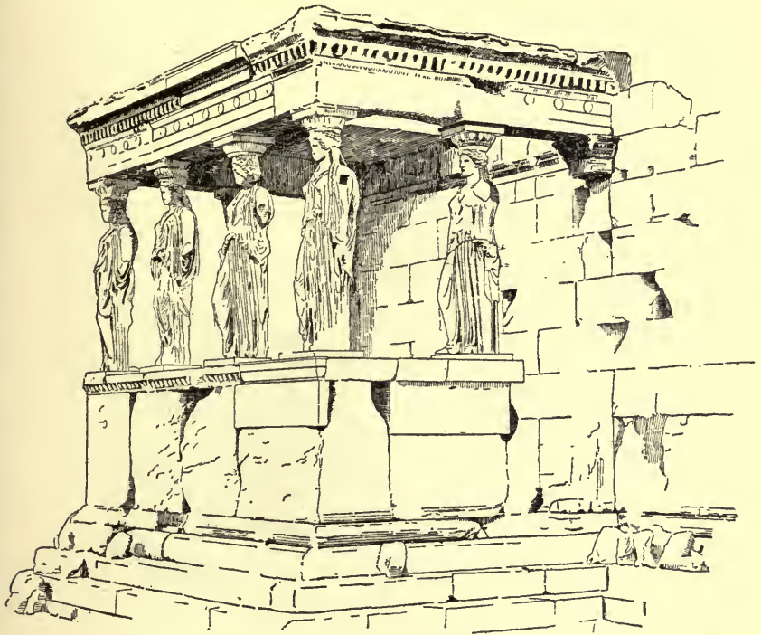
FIG. 25. Athens: Erechtheion, the southern portico.
