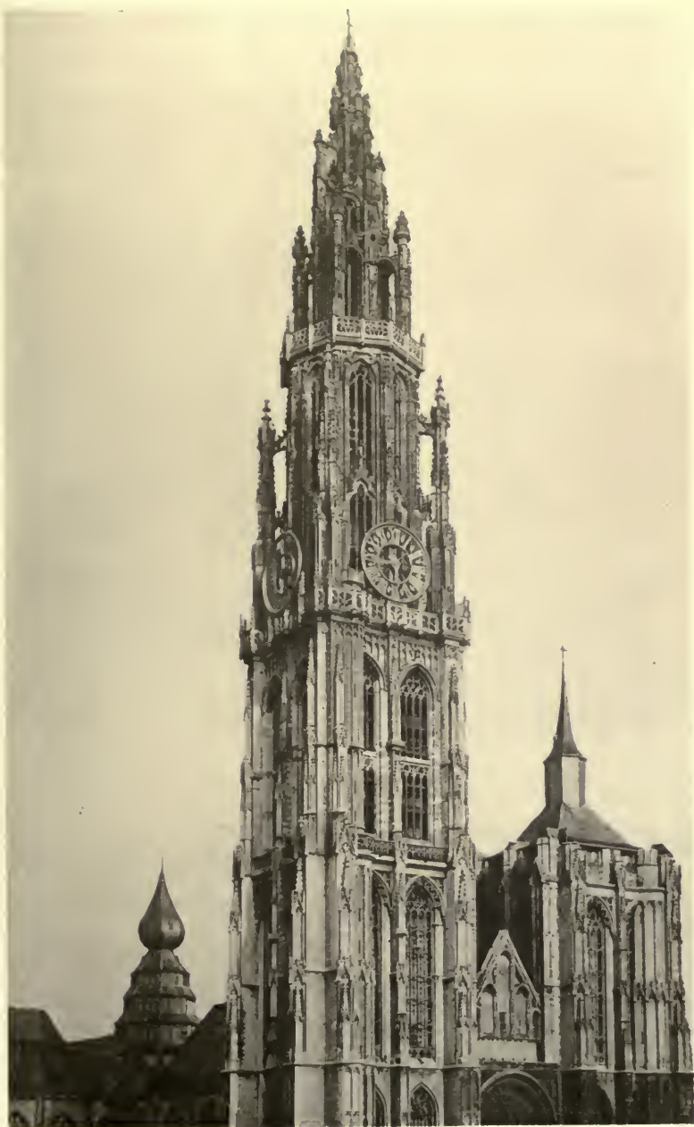
PLATE V. PART OF WEST FRONT OF CATHEDRAL OF ANTWERP, BELGIUM
