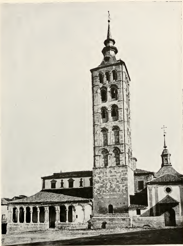
SOUTH PORCH AND TOWER San Estéban, Segovia
