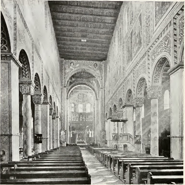
INTERIOR, LOOKING EAST St. Godehard, Hildesheim
