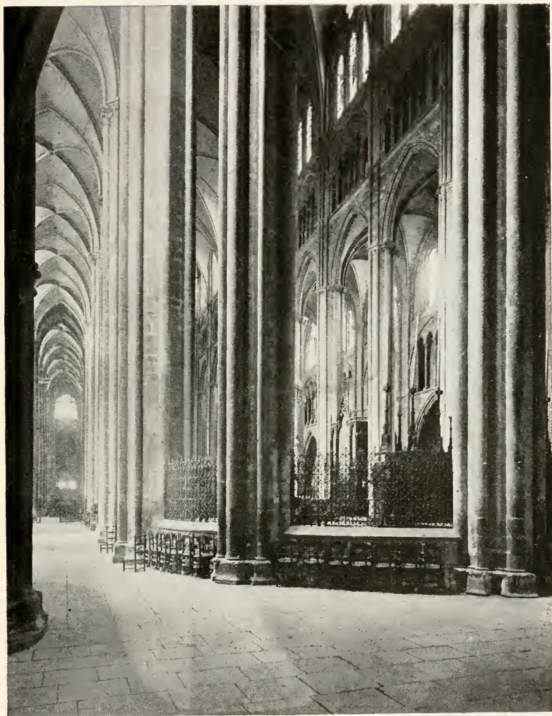
INTERIOR FROM AMBULATORY Cathedral, Bourges
