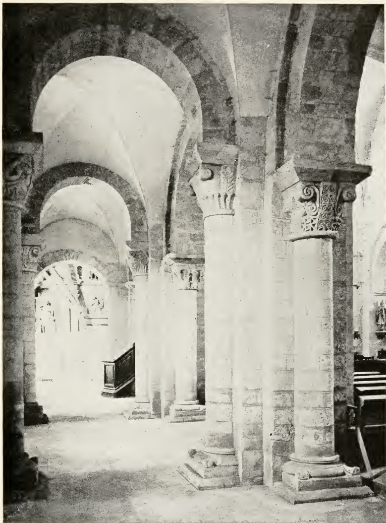
NORTH AISLE OF NAVE Church, Morienvall
