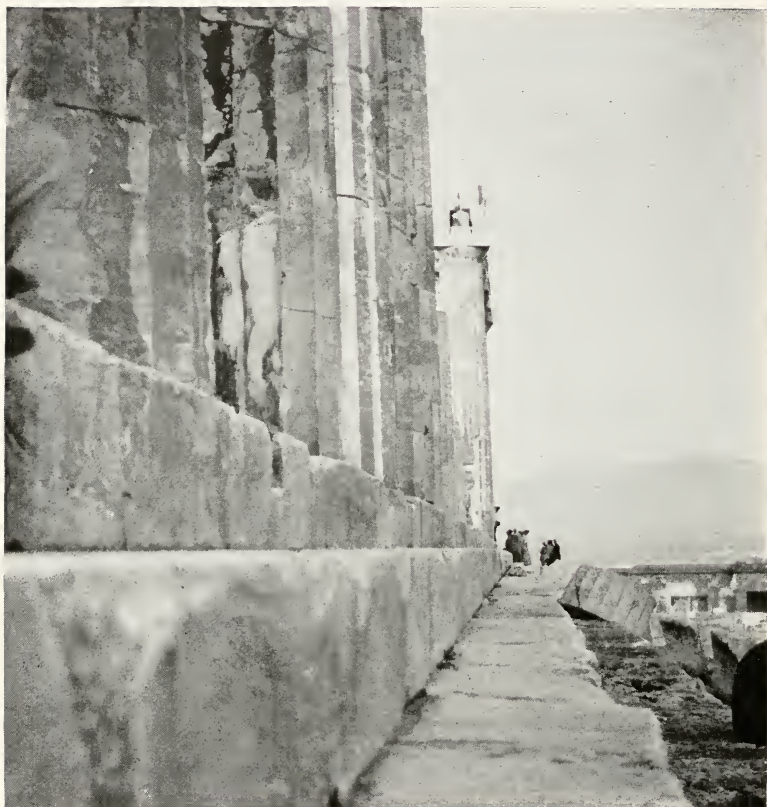
THE PARTHENON, STYLOBATE SHOWING CURVATURE
