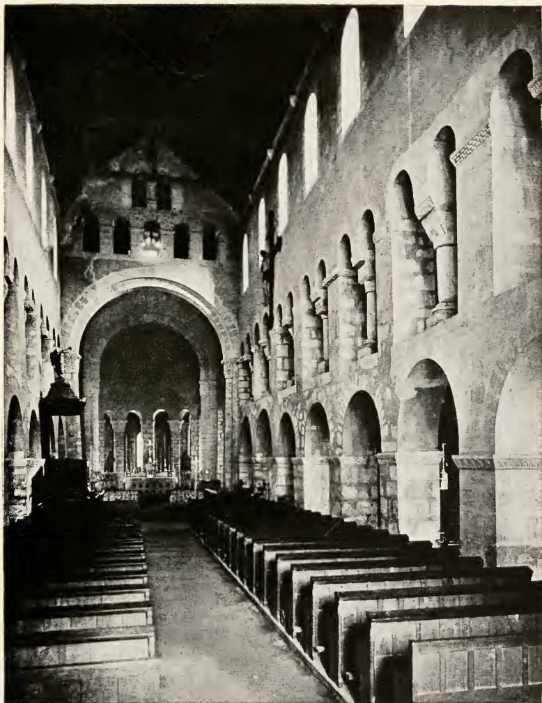
NAVE, LOOKING EAST Church, Vignory
