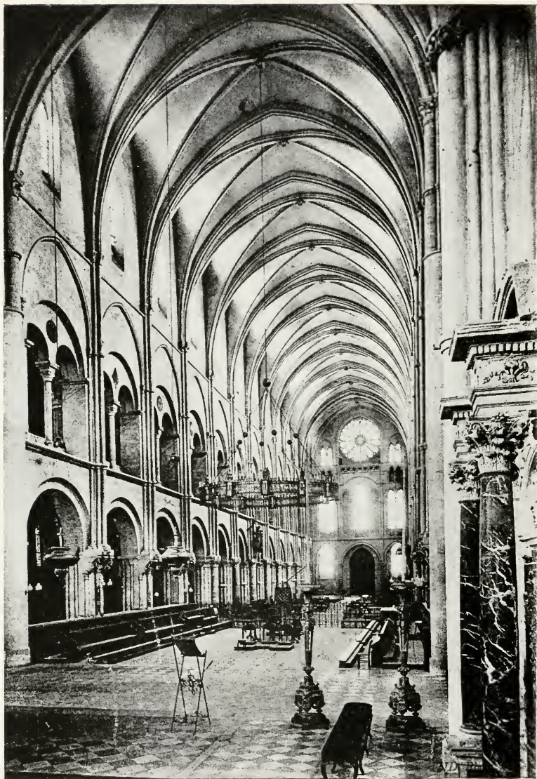
NAVE, LOOKING WEST St. Remi, Reims
