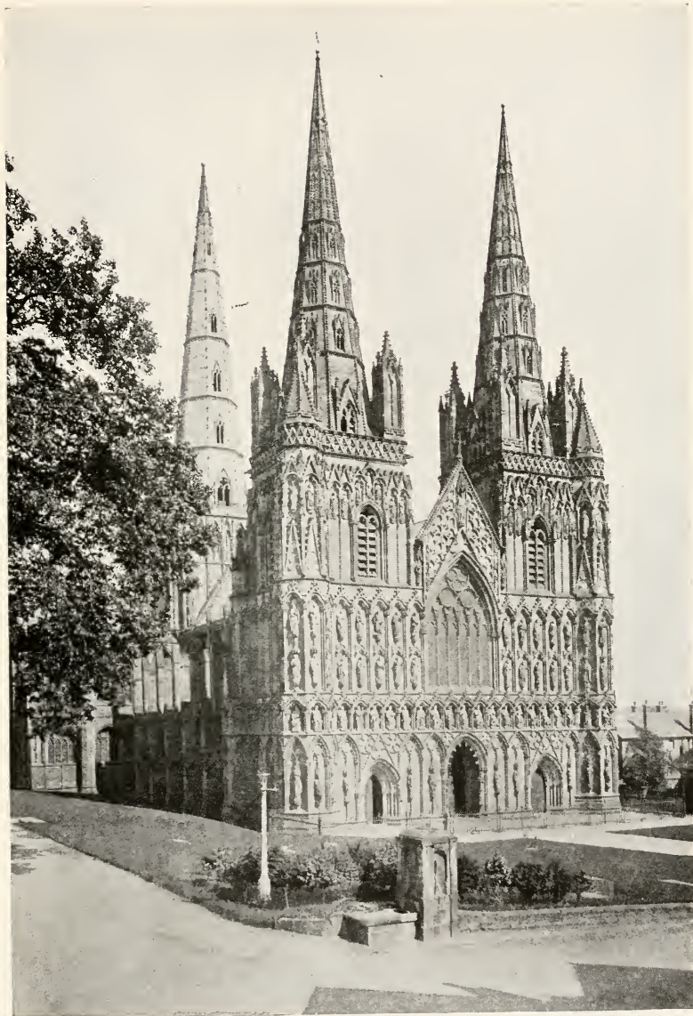
VIEW FROM NORTHWEST Cathedral, Lichfield
