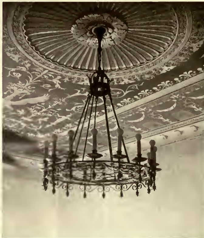
Wrought-iron lighting fixture in entrance lobby.
