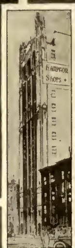
The Hampton Exhibits occupy this entire building. No branches or associated companies.
