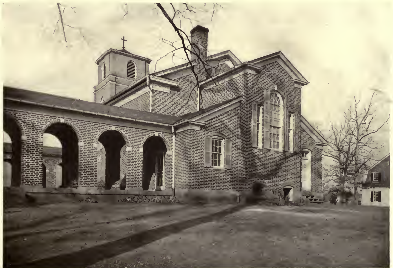
EMANUEL EPISCOPAL CHURCH, GREENWOOD, VA.
