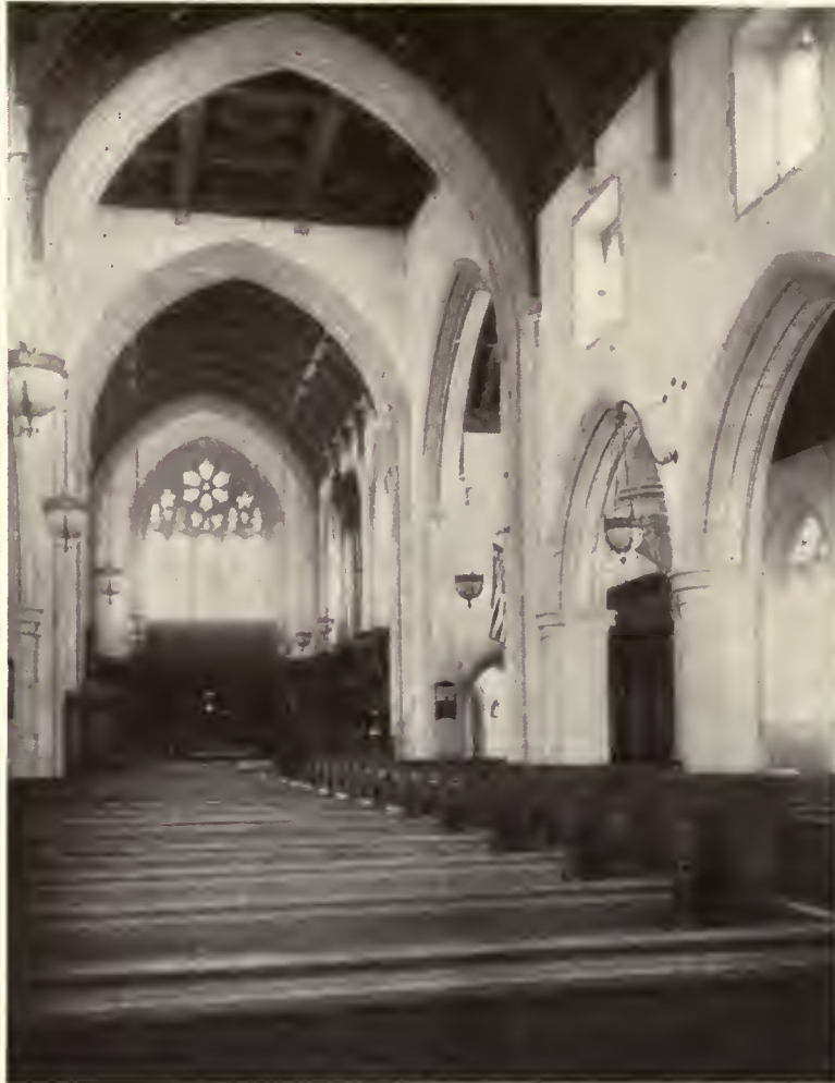
Interior, St. Michael's Church, Litchfield, Conn.
