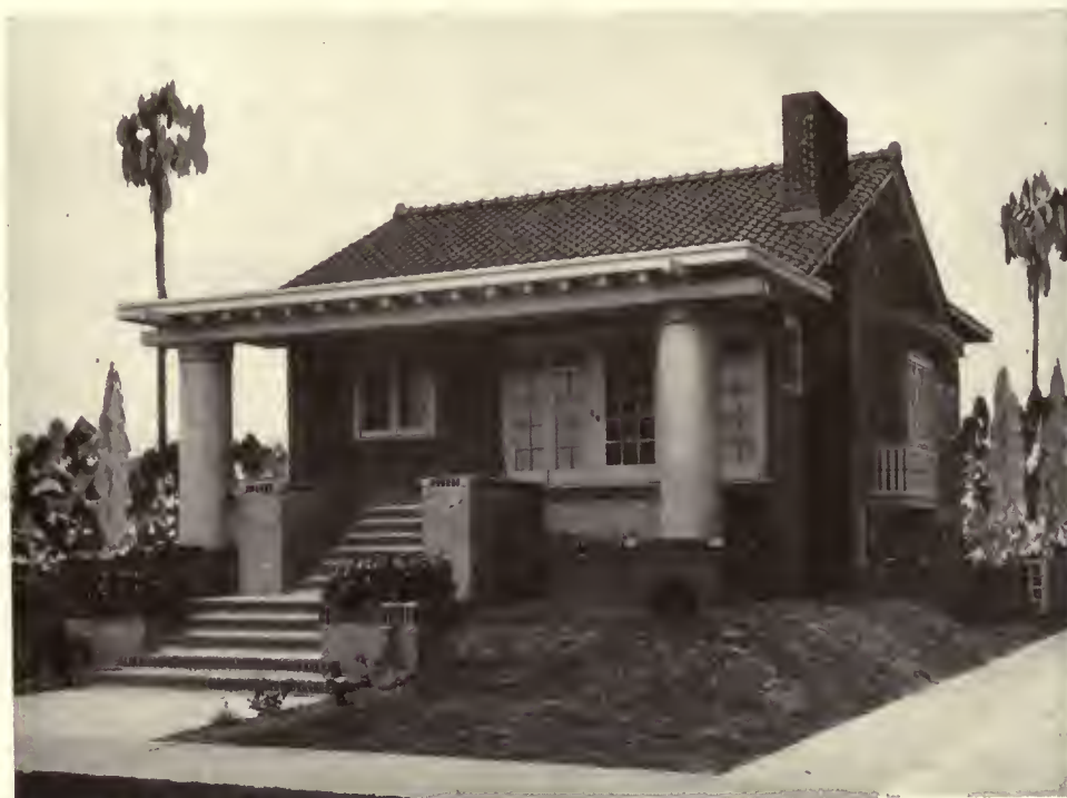
House, John L. Cahill, New Orleans, La. Morgan D. E. Hite, Architect.
