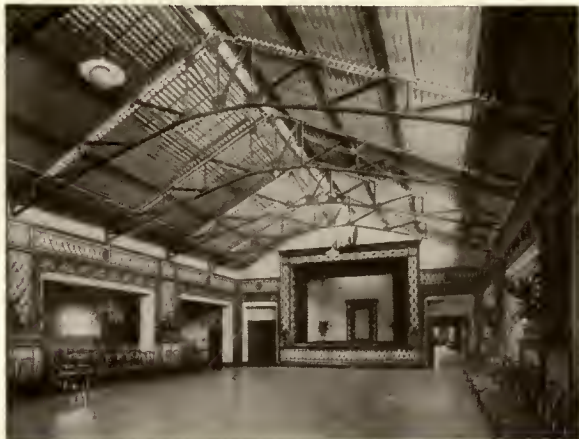
Ventilighters are installed in the Auditorium and Recreation Rooms of the Globe Indemnity Building, Newark, N. J. Frank Goodwillie, Architect
