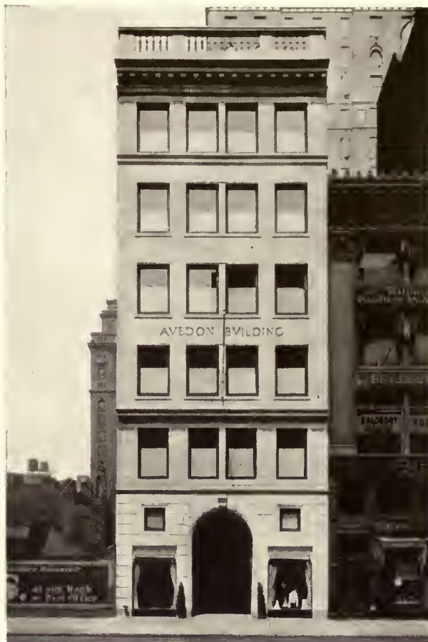
AVEDON BUILDING (RETAIL SHOP), FIFTH AVENUE, NEW YORK. Harry Allan Jacobs, Architect.
