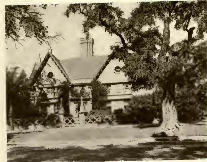
Pickering House, Salem. (Present condition.)
