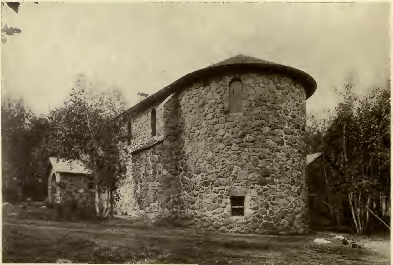
DETAIL OF EXTERIOR.
