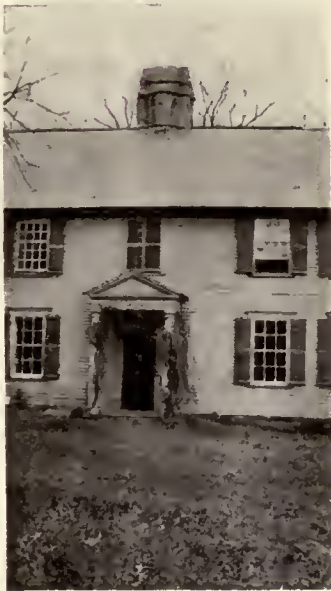
Governor Bradstreet House. The chimney alone is of the seventeenth century; the rest was altered in Georgian period, when pitch of roof was lowered, as may be seen by examining chimney.
