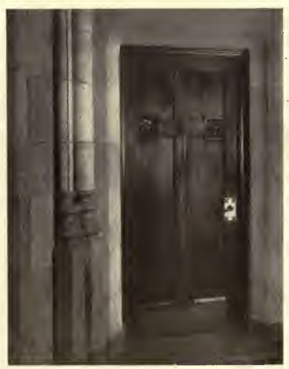
Door detail, main church auditorium.
