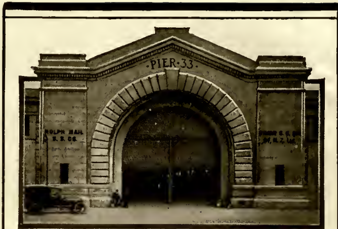
Main Entrance Doors, Pier 33, San Francisco
