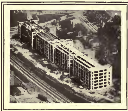
Barrett Specification 10-year Bonded Roof on addition to Endicott-Johnson Corp. plant, Johnson City, N. Y. Eng. & Gen'l. Cont.: Thompson & Binger, New York; Roofer: Central City Roofing Co., Syracuse, N. Y.
