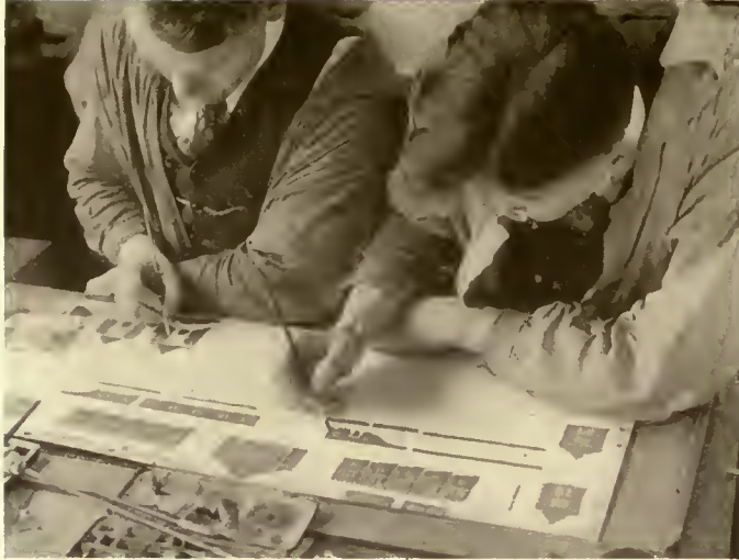
No. 1. Painting the elevations of the various sides of the model upon mounted Whatman paper.
