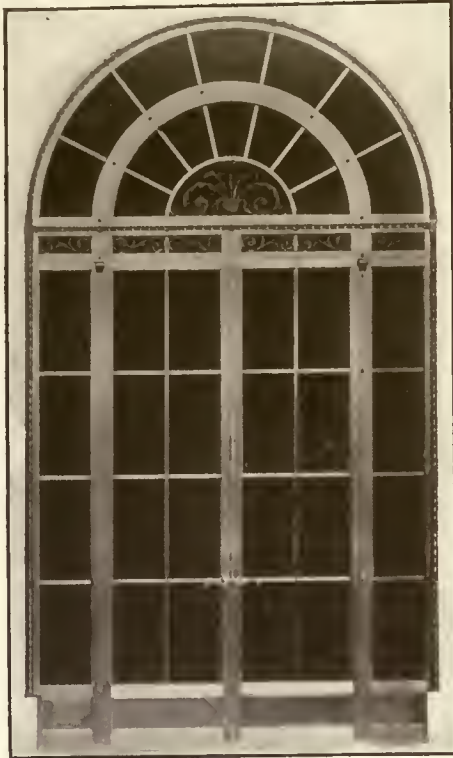
BRONZE SCREEN FOR FREER COLLECTION BUILDING SMITHSONIAN INSTITUTE, WASHINGTON, D.C. CHARLES A. PLATT, ARCHITECT, NEW YORK. EXECUTED BY THE GORHAM CO., ARCHITECTURAL BRONZE DEPT. EXTRUDED BARS AND SHAPES SUPPLIED BY THE AMERICAN BRASS COMPANY
