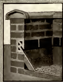
Corner of Roof Showing Brick Wall with Flashing Block and Flashing Installed
