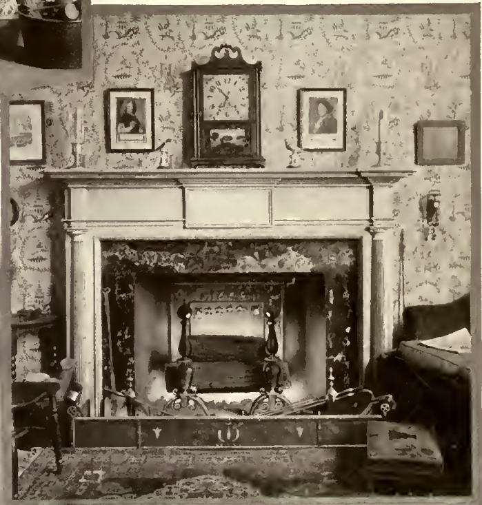
2094. Replica of an old mantel in Baltimore. Elaborately moulded with engaged elliptical fluted columns. Appropriate for a large dining-room.
