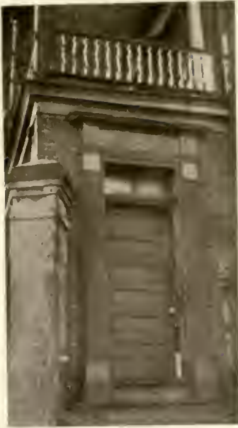
Doorway, 301 East Bay Street South, Charleston, S. C.
