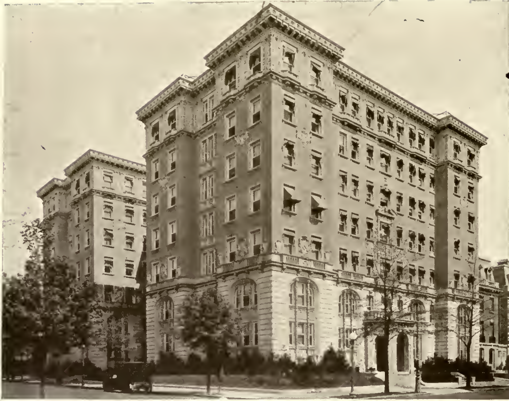
Connecticut Avenue Apartment House, Washington, D. C. Hunter & Bell, Architects; Bates Warren, Builder Atlantic Terra Cotta in light ivory matt glaze for two-story base, entrances, decorative details of shaft and entablature
