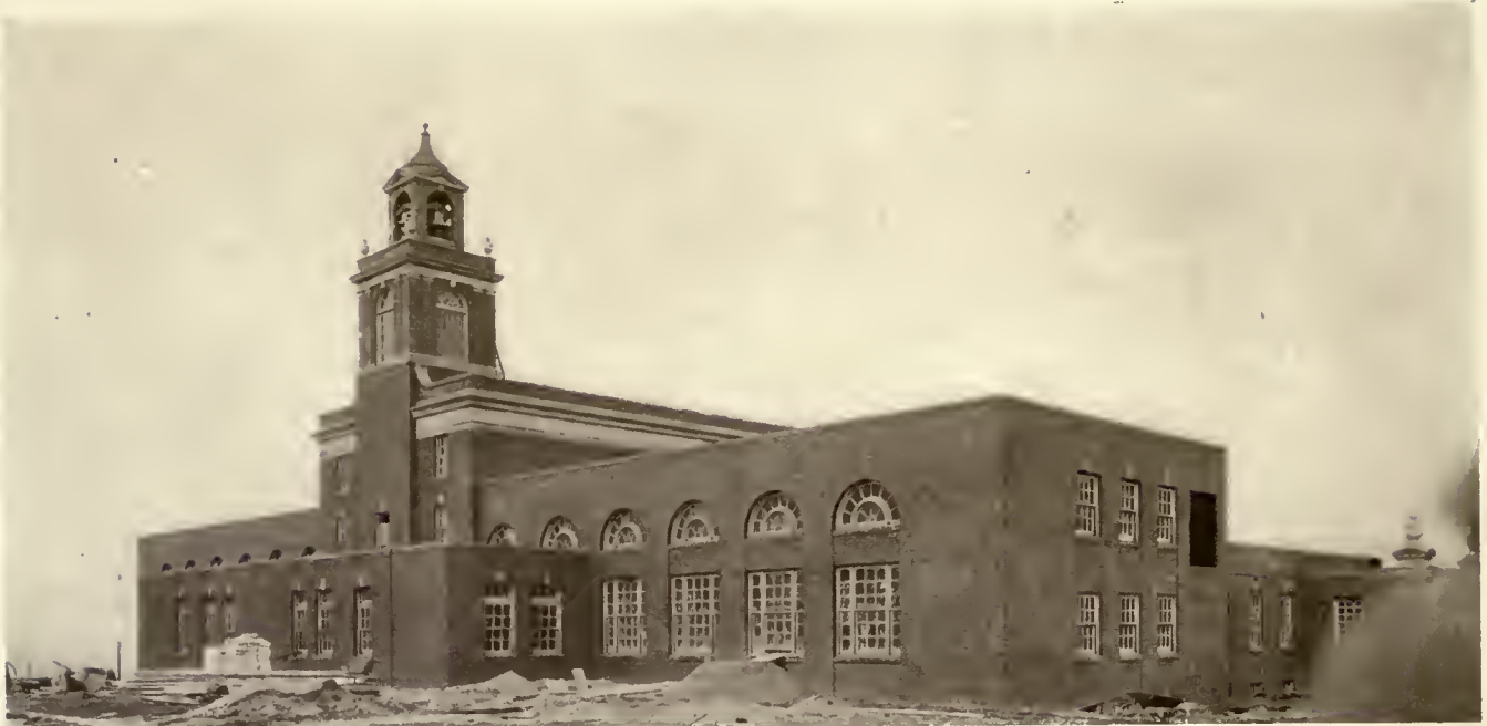
South elevation, bell-tower, Nela Park, Cleveland, Ohio (showing cafeteria.)
