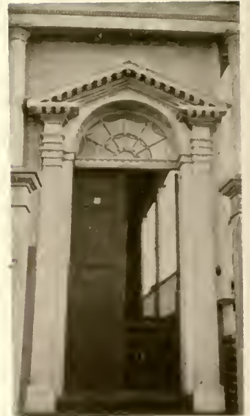
Doorway, 39 Bay Street South, Charleston, S. C.
