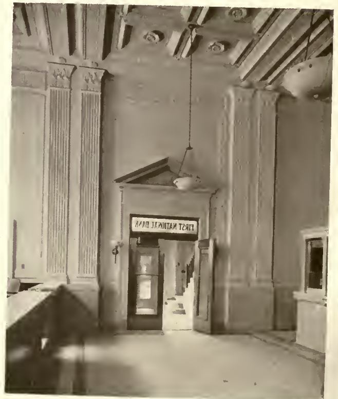
DETAIL, BANKING-ROOM. Childs & Smith, Architects.
