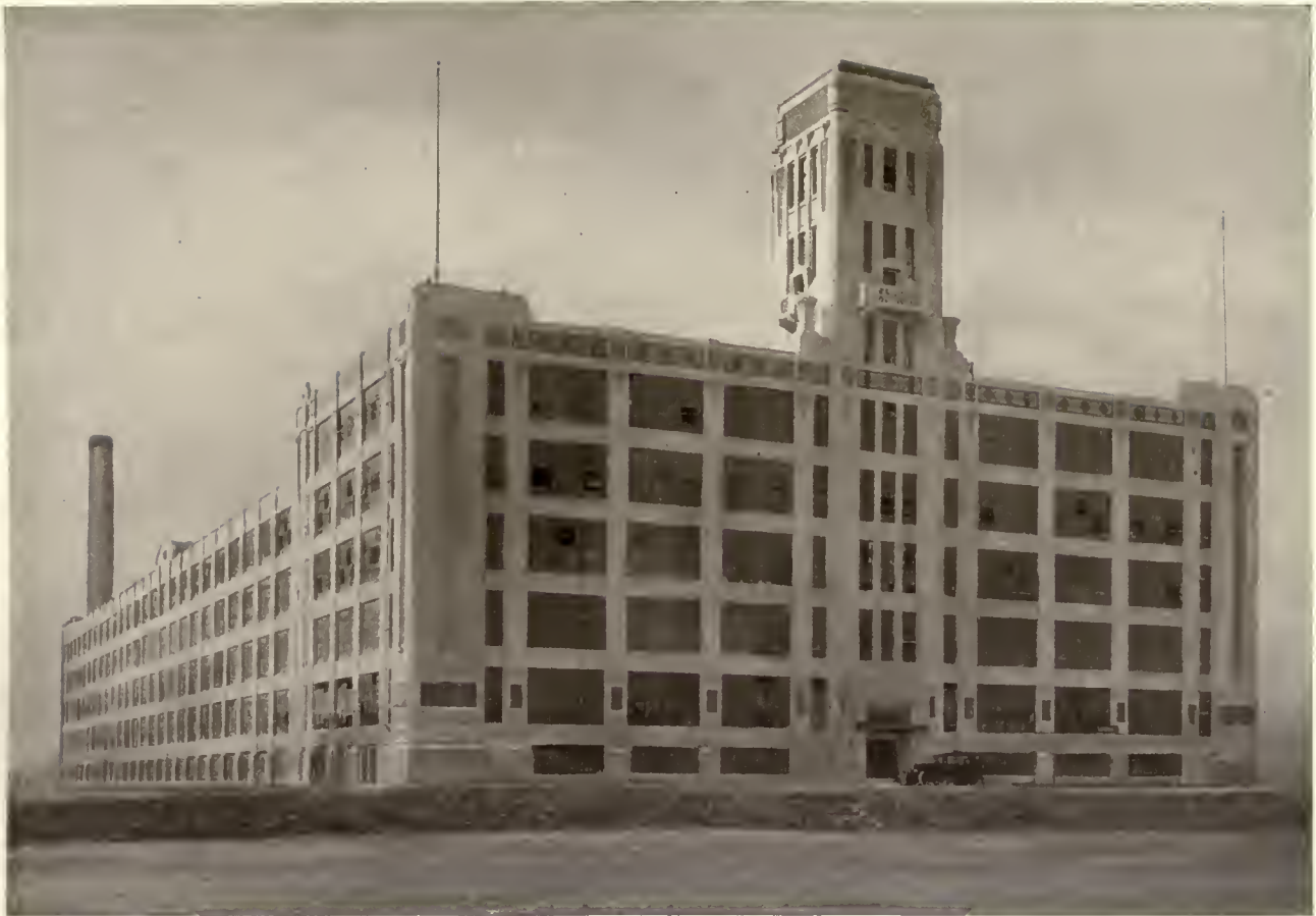
THE AMERICAN CHICLE CO. BUILDING, LONG ISLAND CITY, N. Y.
