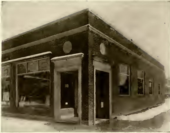
Fillmore Avenue Branch, Marine Trust Co., Buffalo, N. Y. Harold Jewett Cook, Architect.
