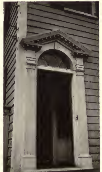
Doorway, 55 Church St., Charleston, S. C.
