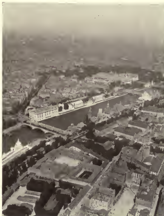
Fig. 5 An airplane view of the Paris Fair, showing the effect of utilizing the natural beauty of a river's banks.
