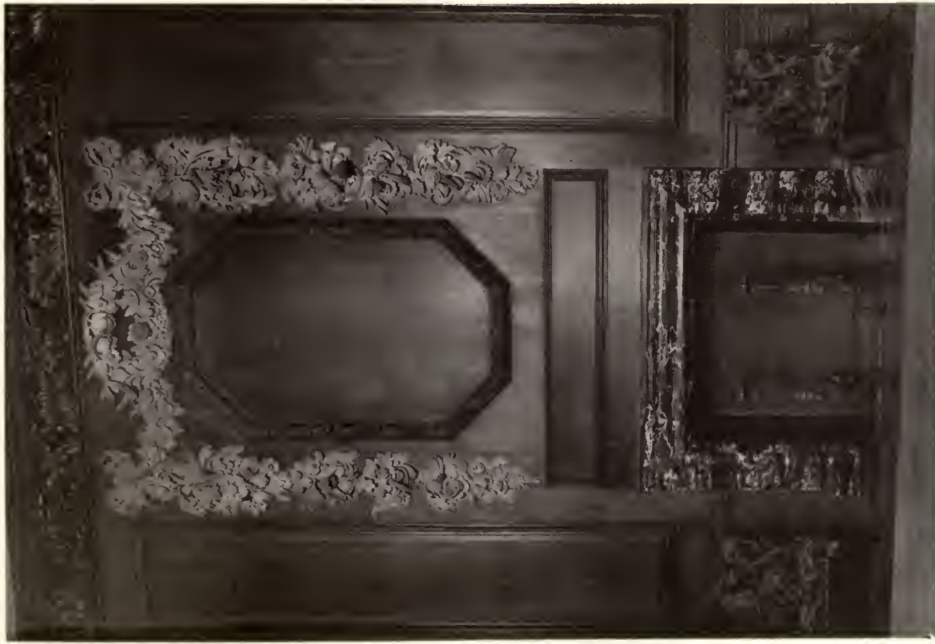
MANTELS IN SALESROOMS, CAMMEYER BUILDING, 677 FIFTH AVENUE, NEW YORK.
