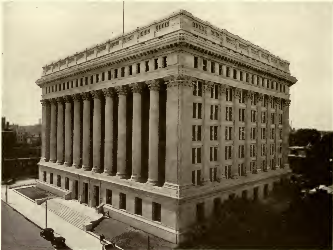
Northwestern Mutual Life Insurance Building, Milwaukee, Wis.
