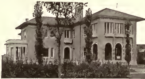
Equipped with Kernerator Residence of W. J. Fleming, Chicago, Ill. Tullmudge & Watson, Architects
