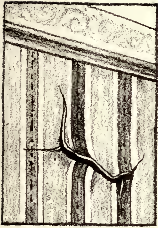
THE DEFECTIVE PLASTER
