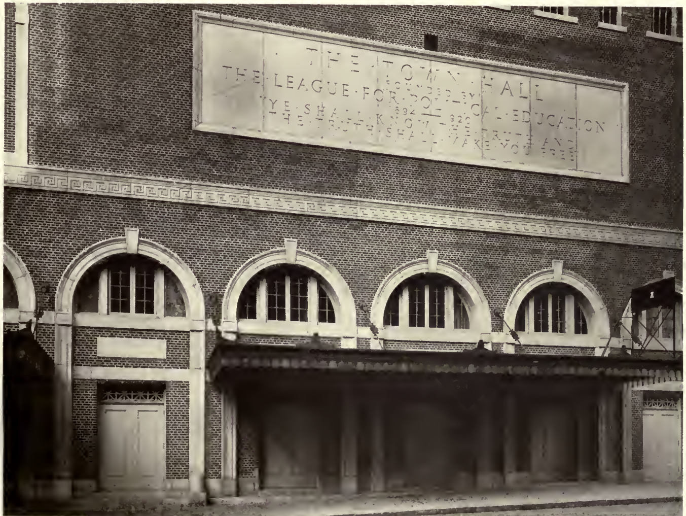
ENTRANCE DETAIL, THE TOWN HALL, NEW YORK CITY.
