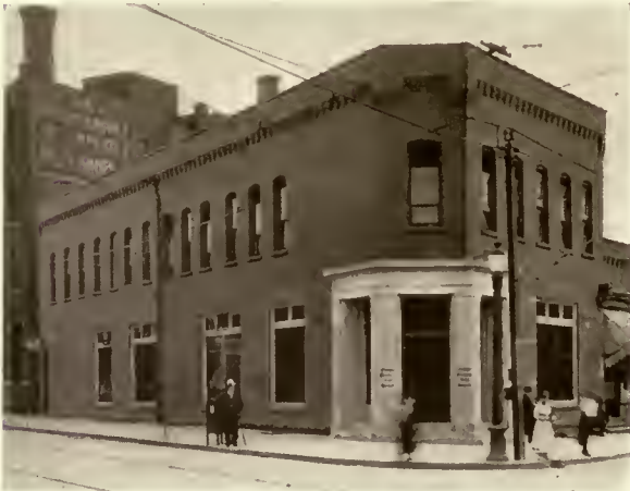
Genesee Street Branch, Citizens Commercial Trust Co., Buffalo, N. Y. Harold Jewett Cook, Architect.
