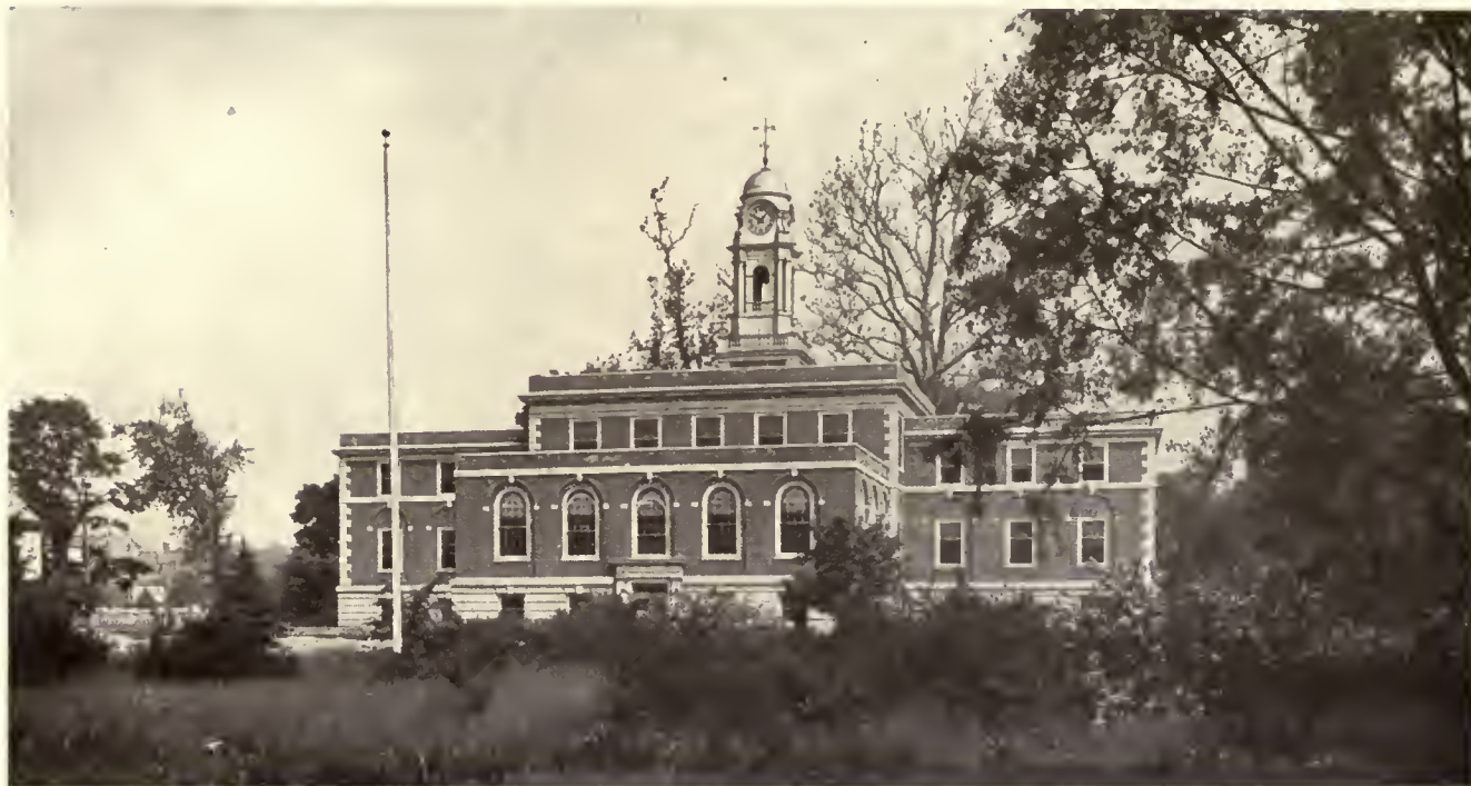
Rear view, Town House, Hempstead, Long Island, N. Y.
