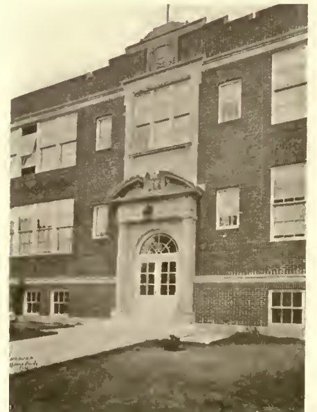
Entrance detail, school, Glens Falls, N. Y. Tooker & Marsh, Architects. Arthur W. Coote, Associate.
