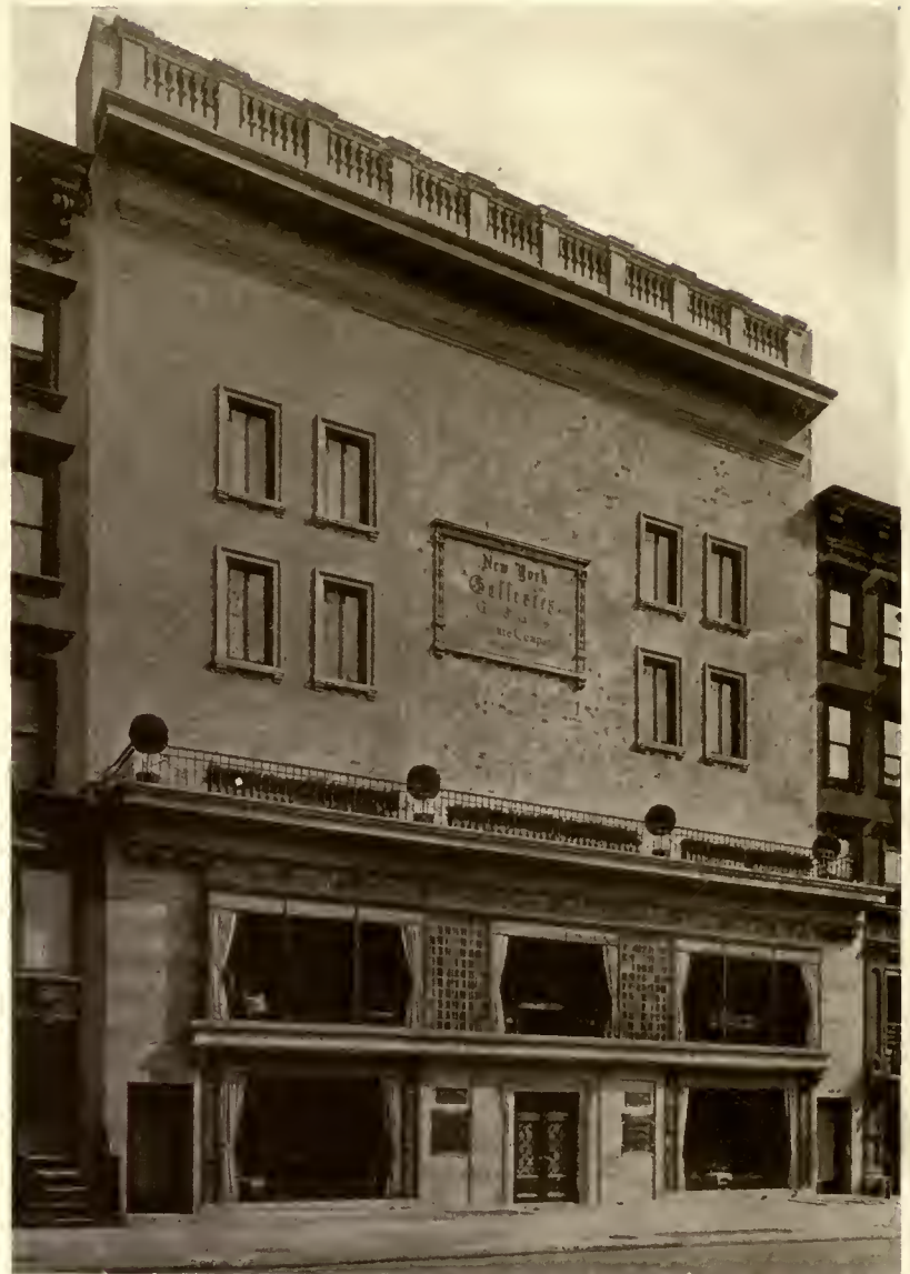
New York Galleries, 419 Madison Avenue, New York City. (Alteration.) Geo. Mort Pollard, Architect.
