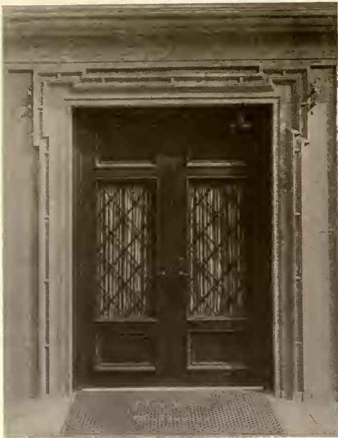
Doorway, New York Galleries, 419 Madison Avenue, New York City.
