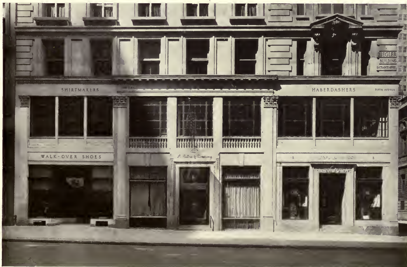
Three shops (offices above), 512 Fifth Avenue, New York (alteration).
