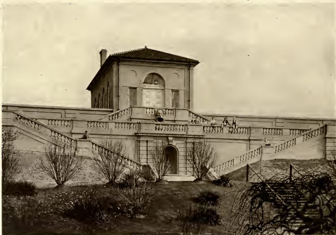
BUILDING AT RESERVOIR.
