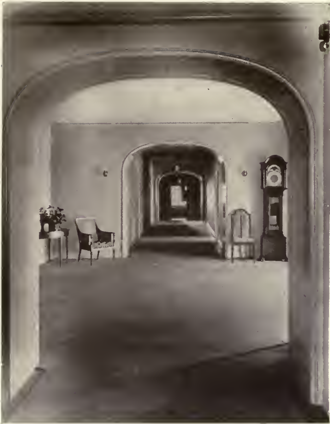
Entrance-hall and corridor.
