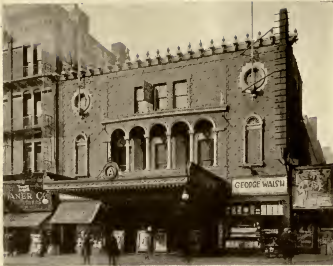
Arena Theatre, New York. S. B. Eisendrath, Architect. B. Horwitz, Associate.
