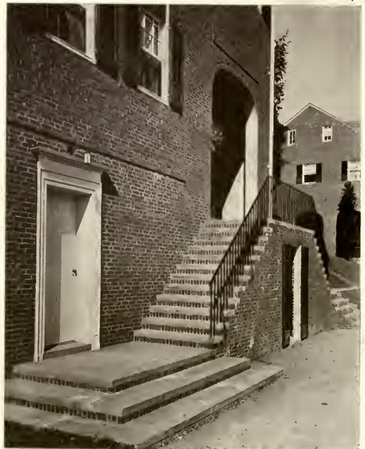
THE CLOISTER STAIRS.
