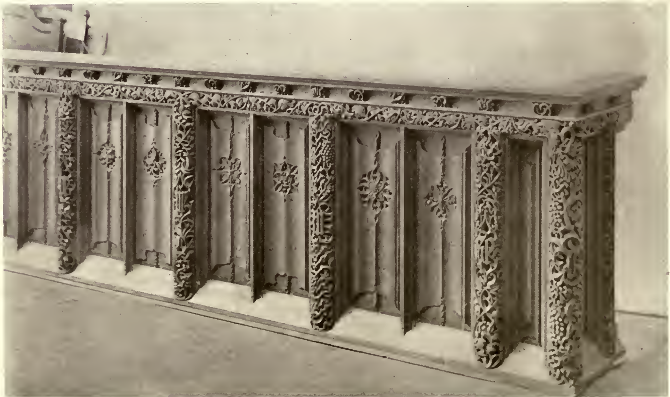
Parapet over Choir.
