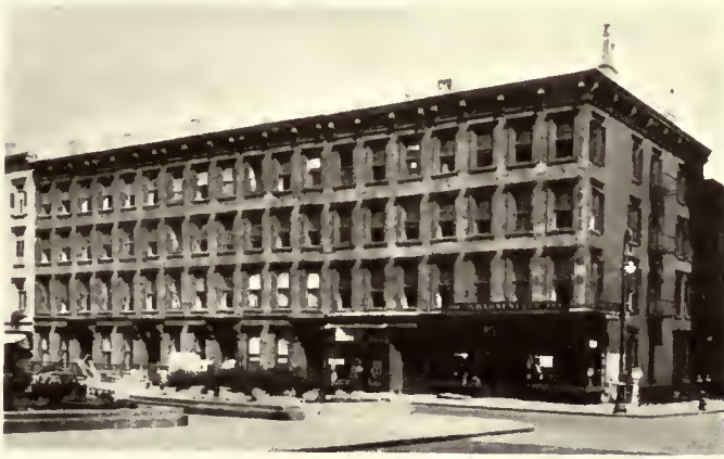
421-431 Park Avenue (before alteration).
