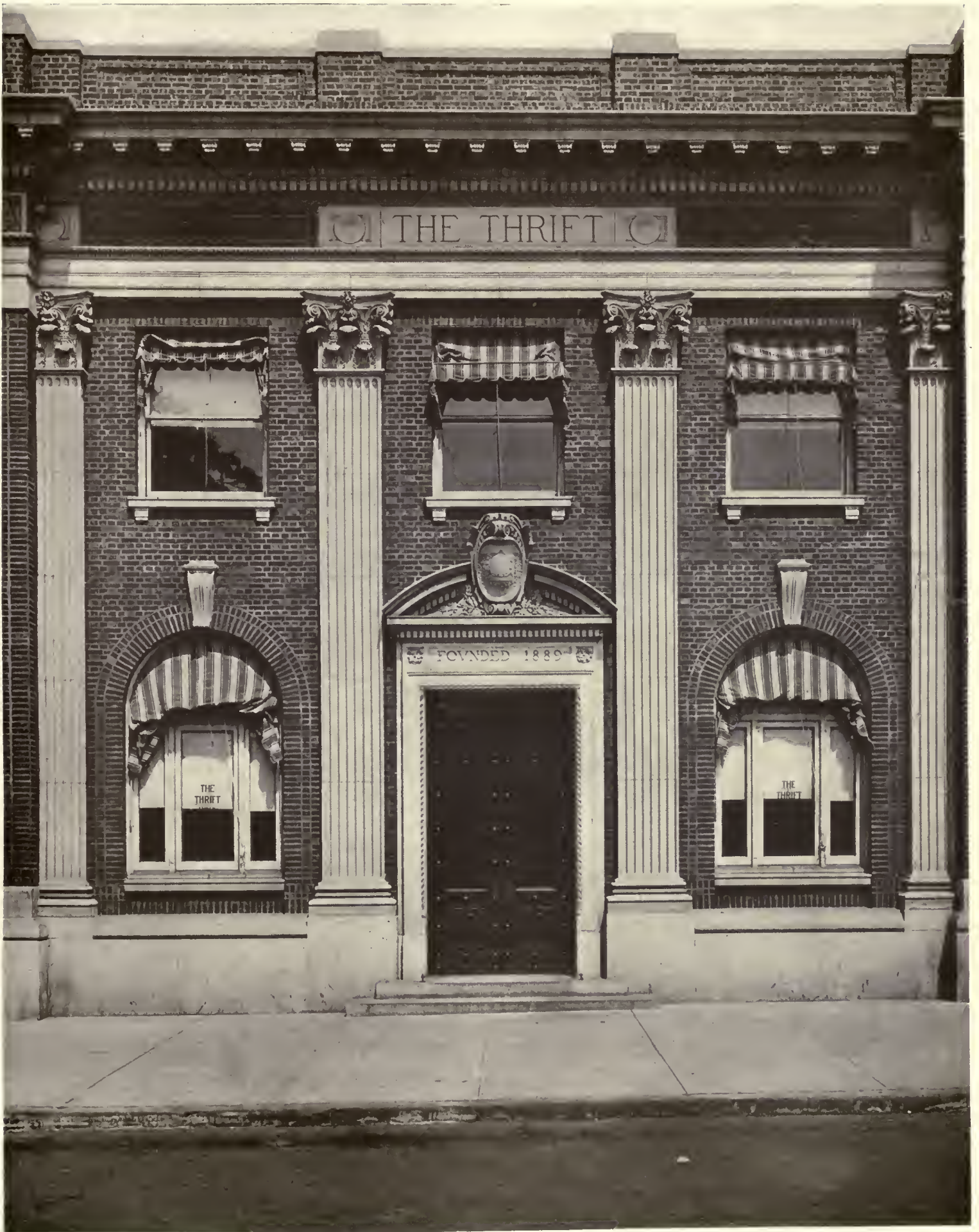
ENTRANCE DETAIL, THE THRIFT BANK, DE KALB AVENUE CORNER RYERSON STREET, BROOKLYN, N. Y. Shampan & Shampan, Architects.
