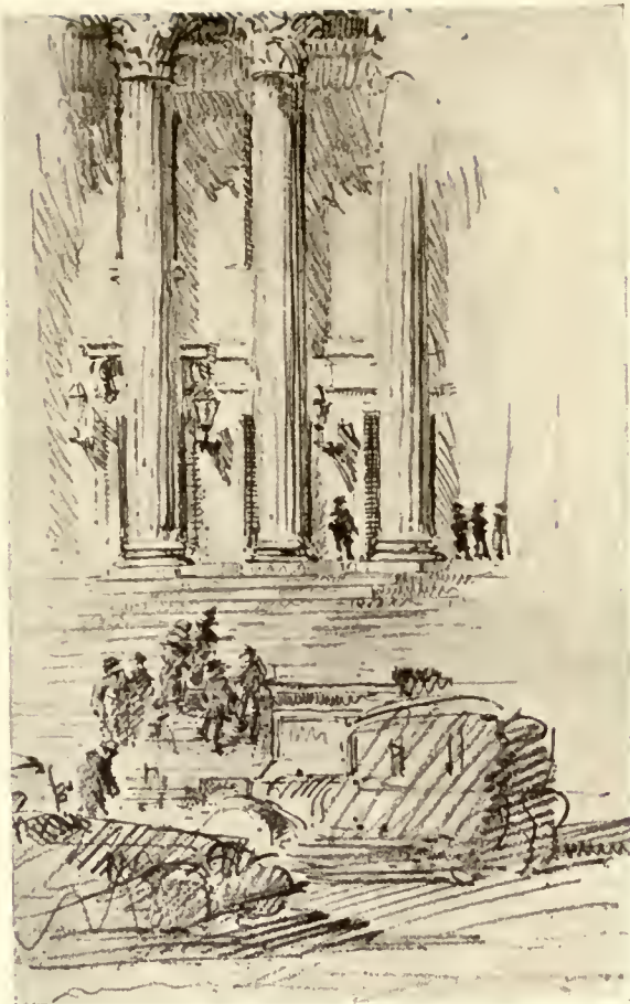
Detail of columns.
