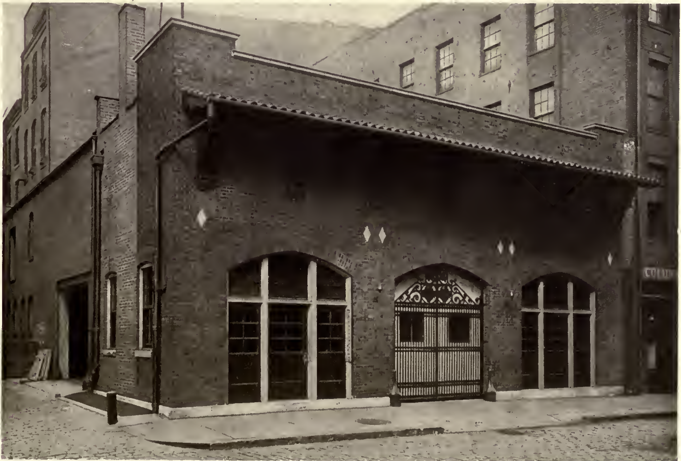
DISTRIBUTION STATION, CHESTNUT STREET.
