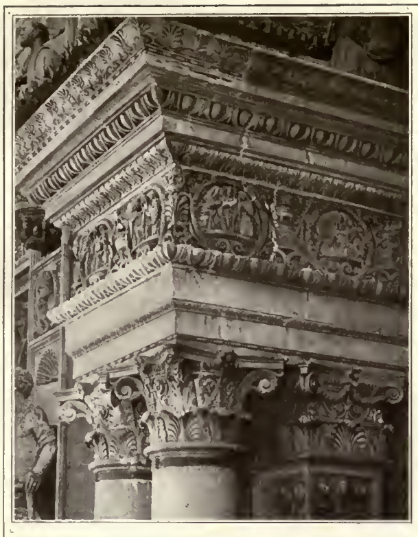
The façade—capitals with entablature and cornice.
