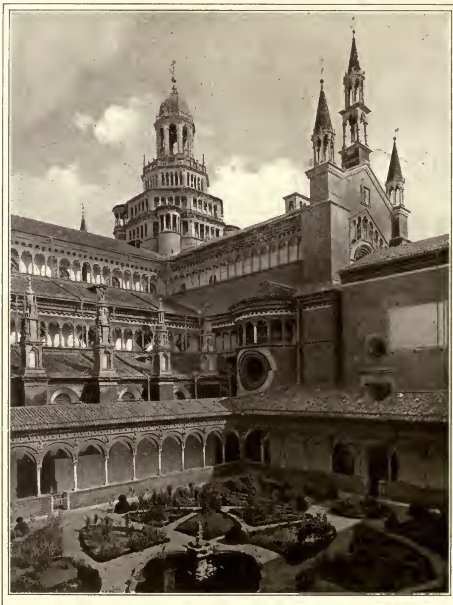
The church from the little cloister.
