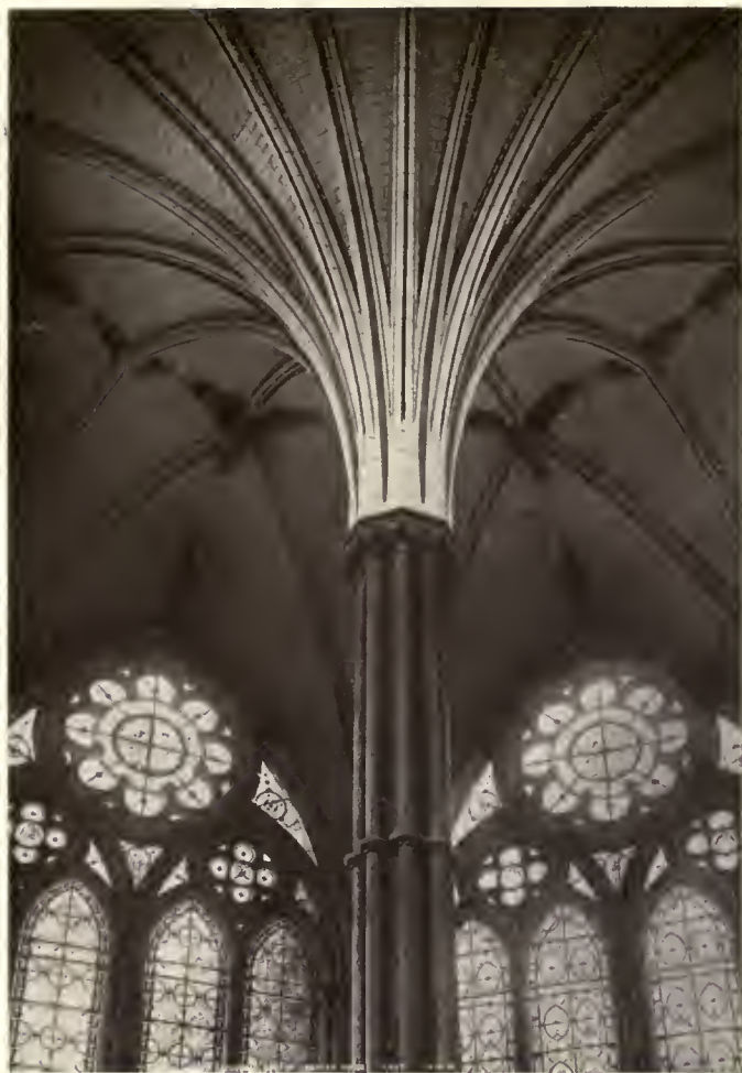
Salisbury Cathedral roof of chapter-house.
