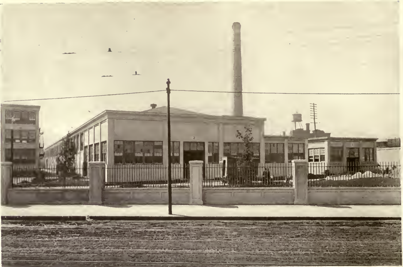
SERVICE BUILDINGS NO. 1 AND NO. 2.
