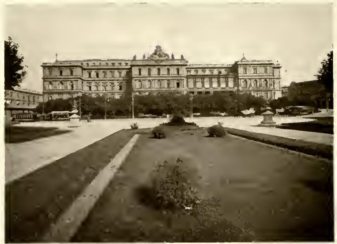
GOVERNMENT PALACE. (The building is constructed with bricks on a piece of ground that forms a parallelogram. The façades cut at right angles and measure 125 metres by 81 metres. The building has on its highest part a group of gigantic statues, made by the sculptor Bianchi.)
