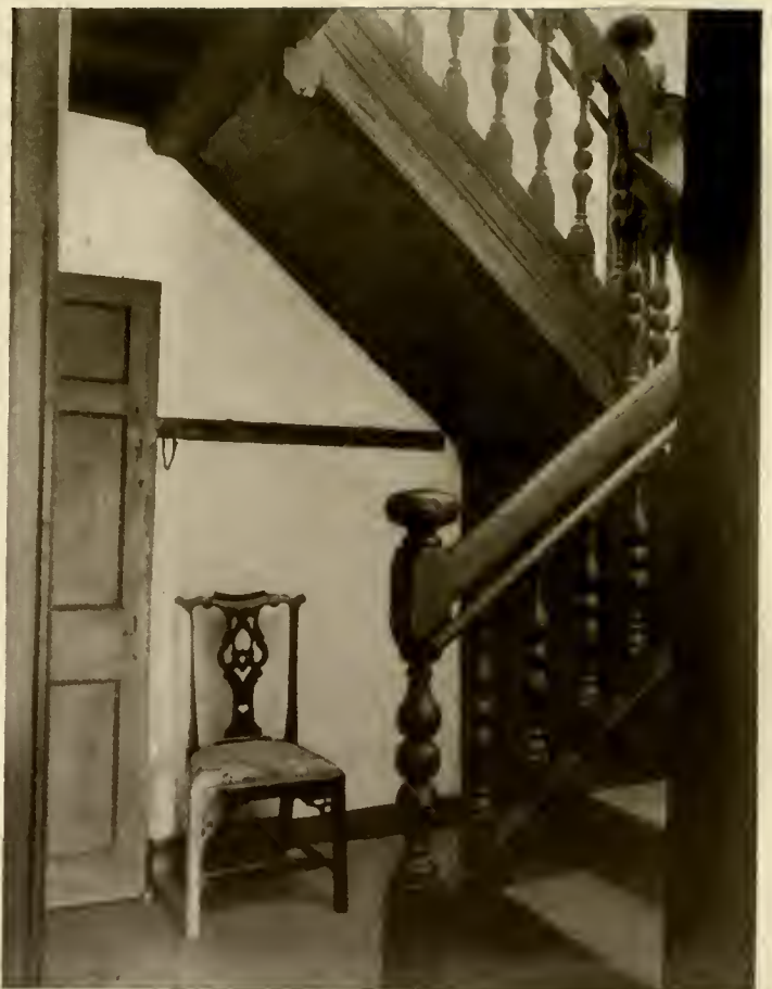
"NORWOOD," PEMBROKE; BUILT C. 1680. SEVENTEENTH CENTURY STAIRCASE DETAIL.
