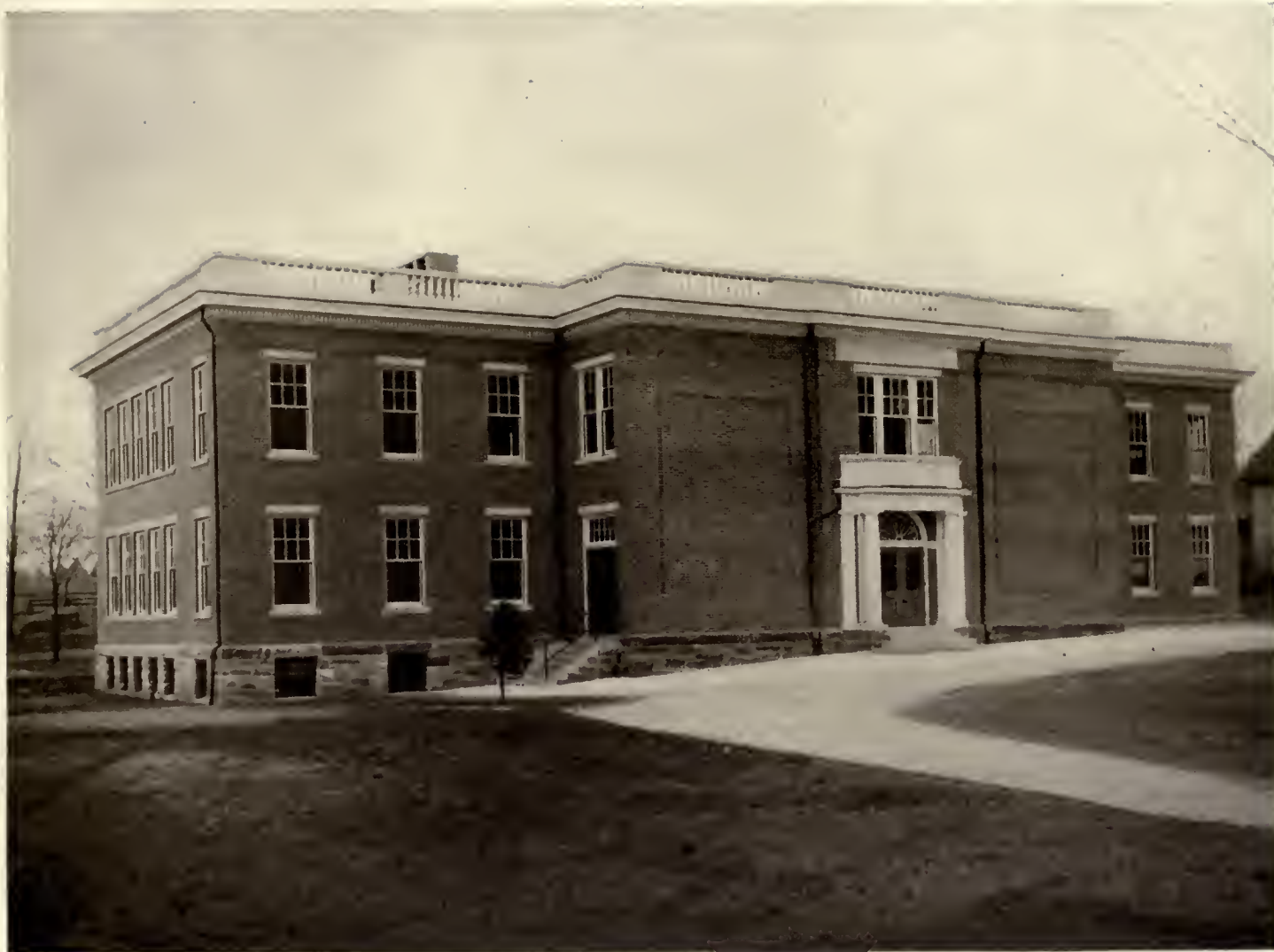
New Jordan School, Waterford, Conn. Louis H. Goddard, Architect.
