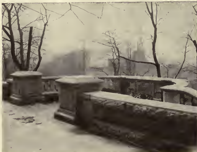
Section of Terrace Wall with tablet to John Mervin Carrère.
