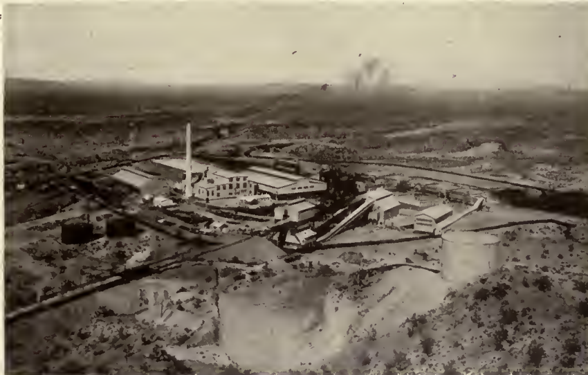
Ajo plant of New Cornelia Copper Company.
