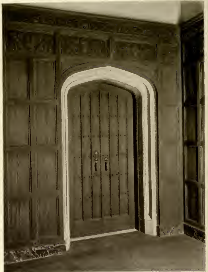
Detail, third floor.
