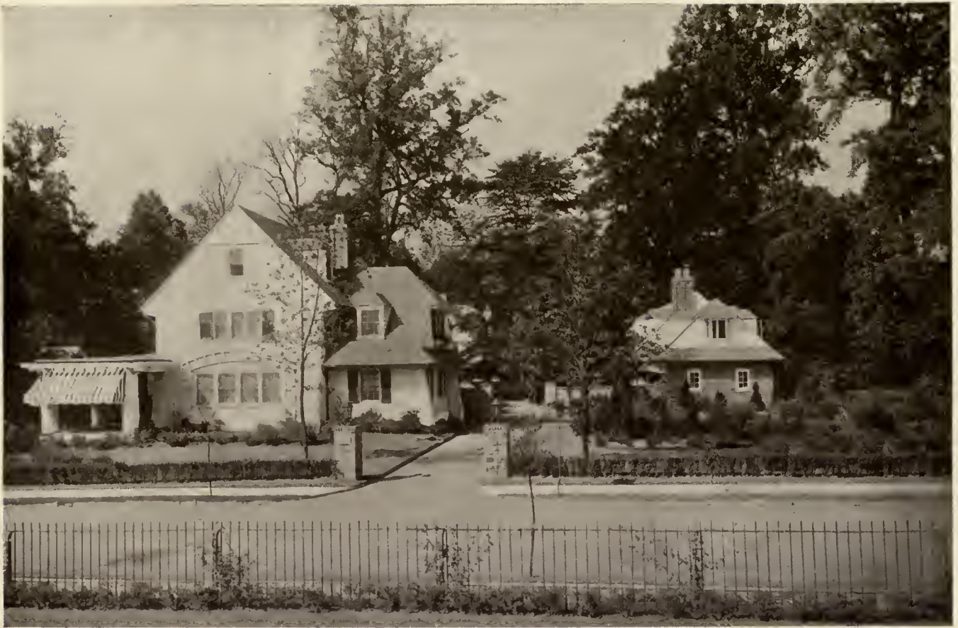
HOUSE AND GARAGE.
