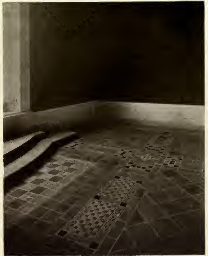
FLOOR IN CLEVELAND ART GALLERY. Touraine Quarry field in Travertine color. The ornamental part in Tuscan glazes and Tuscan inlay decoration. Arthur Loomis Harmon, Architect.
