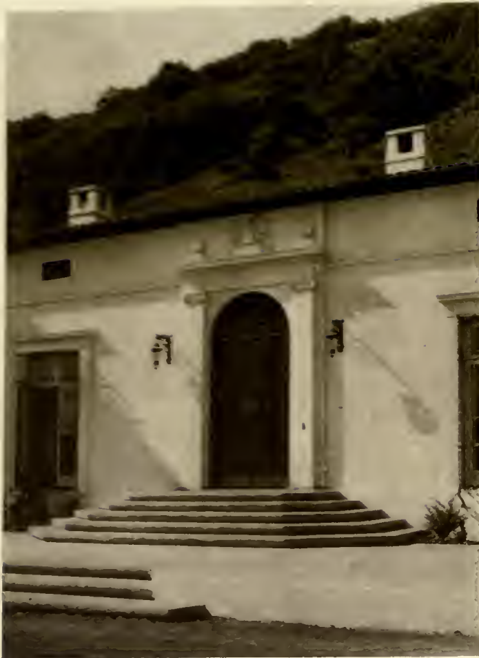
Main entrance, residence, J. H. Pershine, Santa Barbara, Cal. Myron Hunt, Architect. The crest over the door is taken from the authentic coat of arms of the owner, granted by the King of Spain.
