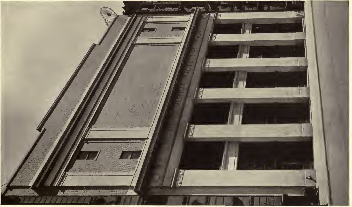
EAST 85TH STREET ADDITION.
