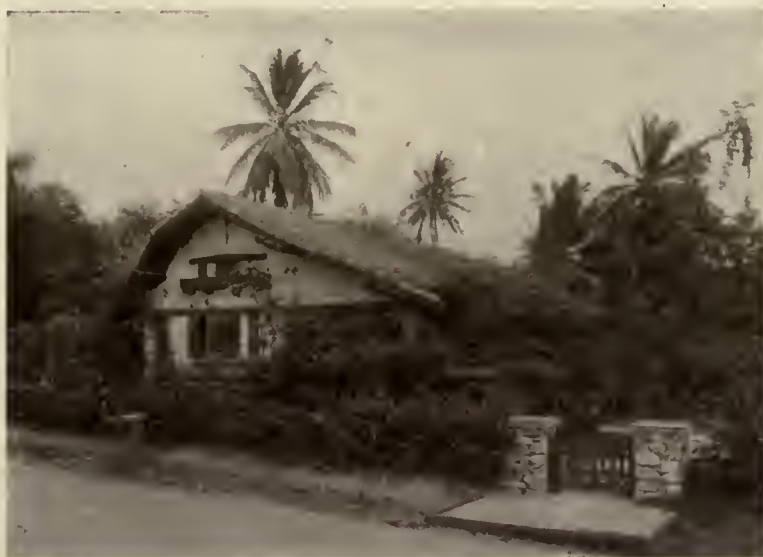
Architect's residence, Monte Flores, P. R. Reinforced concrete, old Spanish tile roof, mosaic floors, solid mahogany interior finish. Antonio Nichodemá, Architect.
