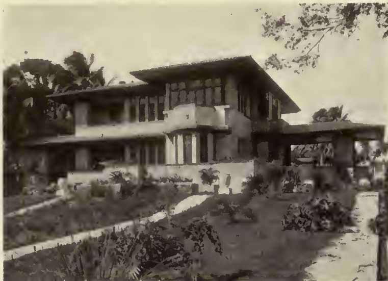
Residence of Mrs. C. McCormick, Santurce, San Juan, P. R. Concrete and terra-cotta, sills of faience tiles, parquet floors, beam ceilings. Antonio Nichodema, Architect.
