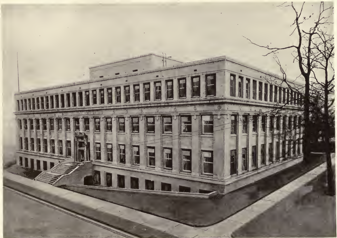
OFFICE BUILDING, YOUNGSTOWN SHEET & TUBE CO., YOUNGSTOWN, O.
