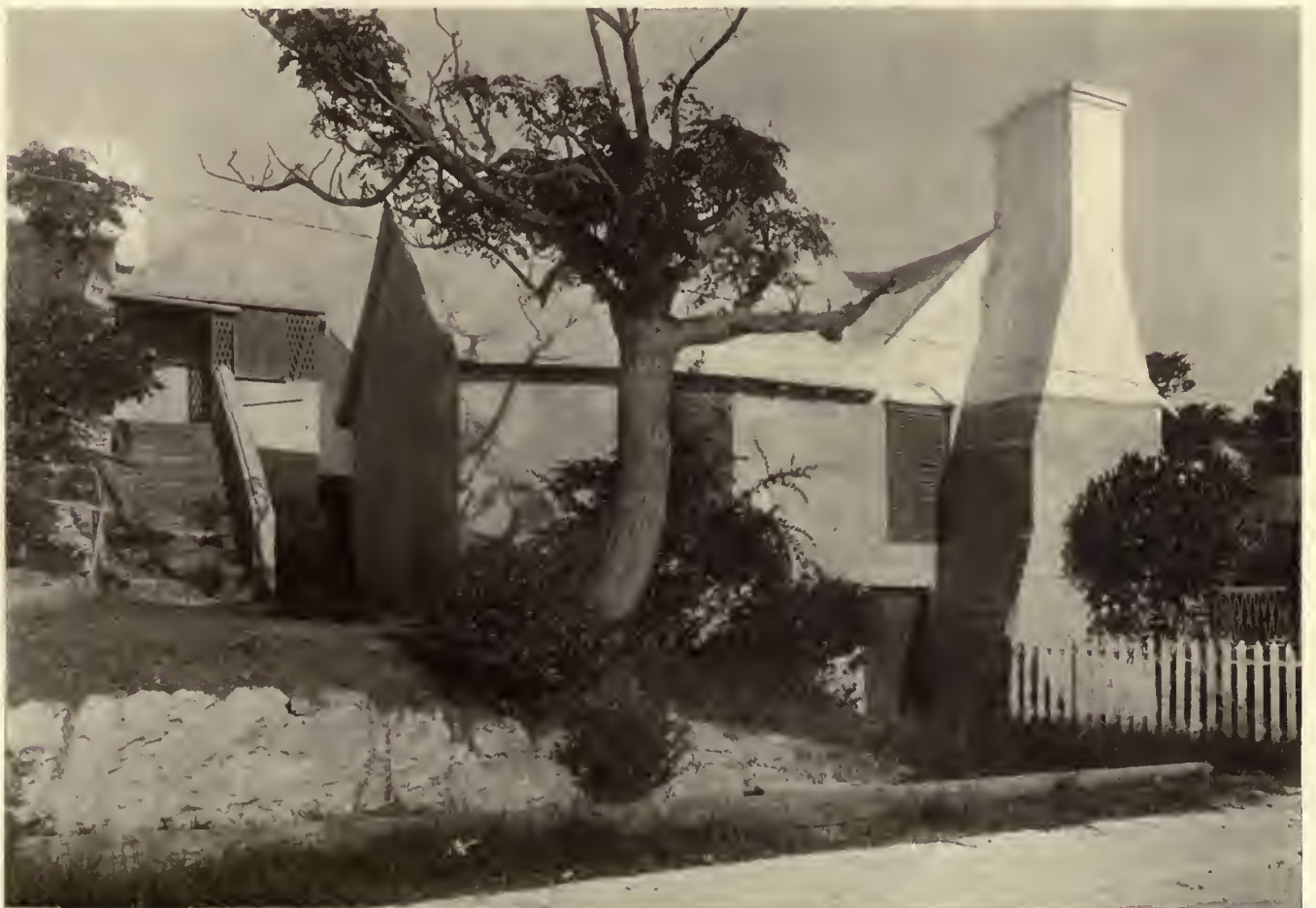
Late seventeenth century house, showing exterior chimney base with battered and stepped weatherings and moulded cap. Also drip-stone and cruciform plan.
