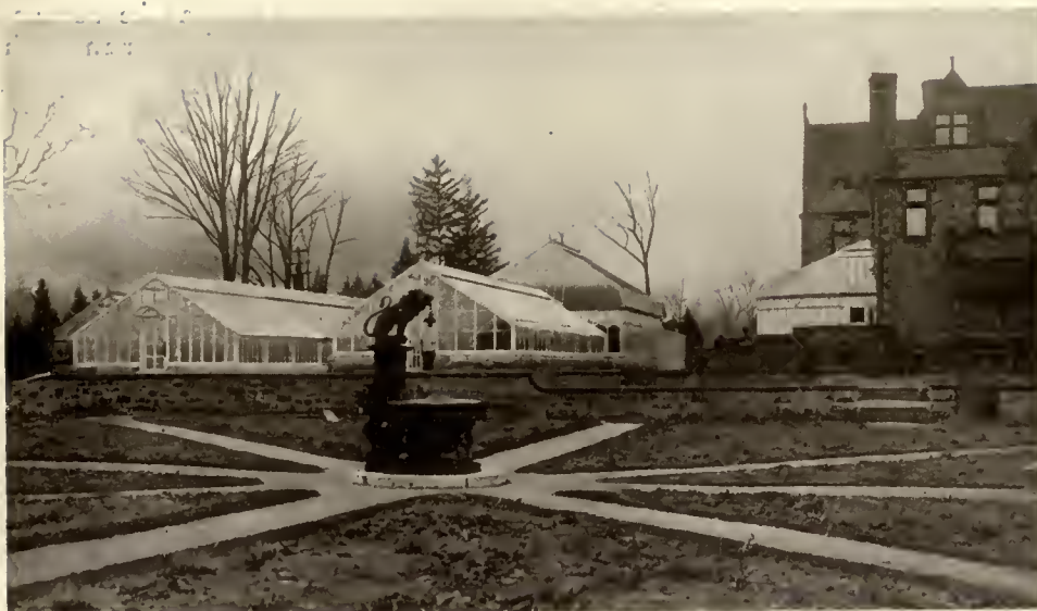
Greenhouse and conservatory in relation to residence, Daniel J. Reid, Irvington, N. Y.
