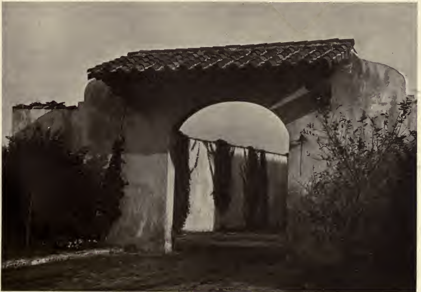
ENTRANCE TO SERVICE COURT.
