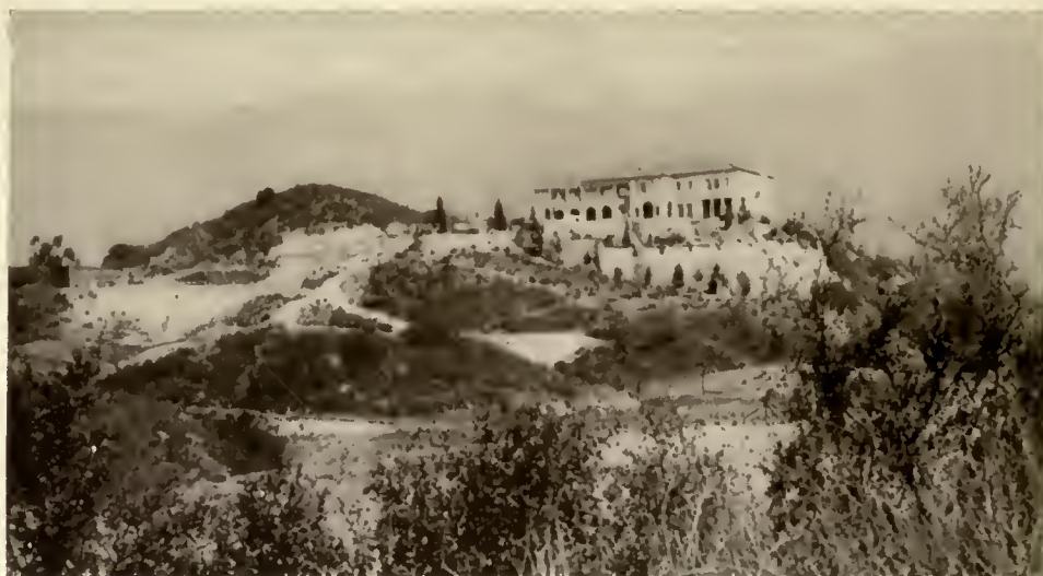
The Malcolm McNaughton residence, La Canada. Reginald Johnson, Architect.
