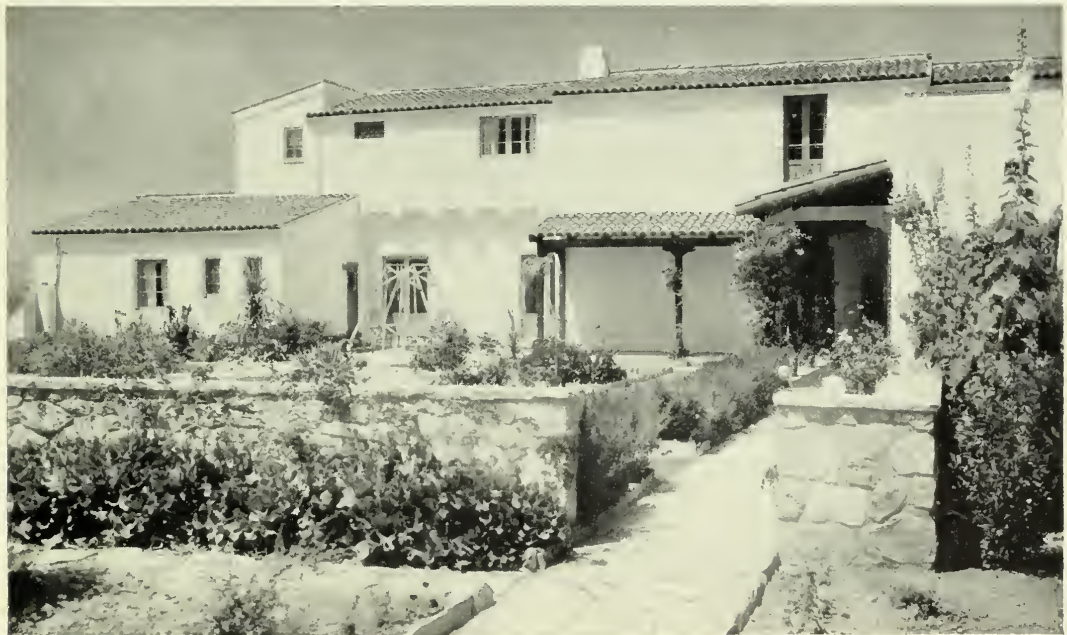
RESIDENCE OF D. K. LAWYER, PALOS VERDES ESTATES John Byers, Architect
