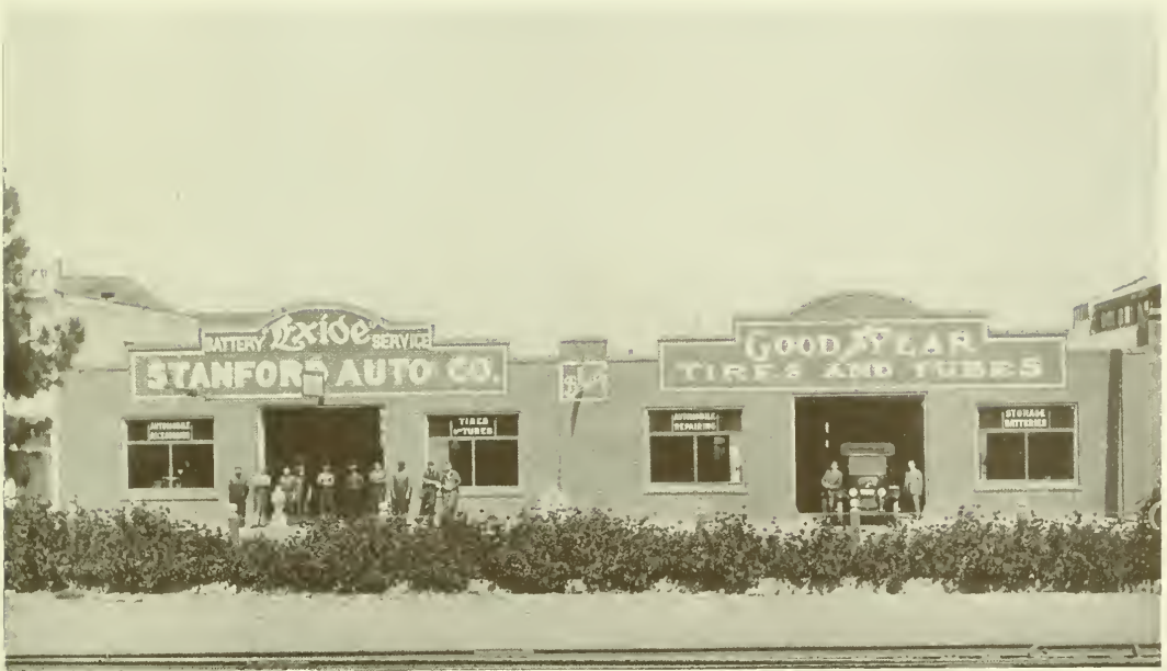
BUILDING FOR STANFORD AUTO COMPANY, PALO ALTO Photo Taken Before Alterations
