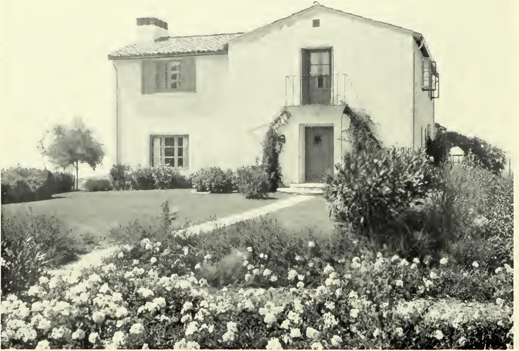
EAST FRONT, RESIDENCE ON GRANVIA LA COSTA, PALOS VERDES ESTATES Winchton L. Risley, Architect
