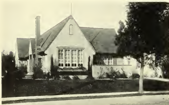
A G. W. Williams Co. Built Home, Burlingame, California
