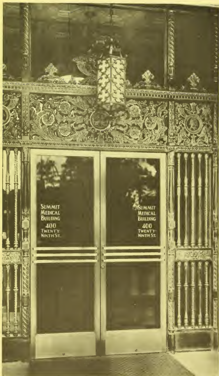
A METAL SCREEN AND DOORWAY POSSESSING DIGNITY, BEAUTY OF DETAIL AND SURFACE. LEAFAGE AND ORNAMENTS REFLECT A FINE APPRECIATION OF DESIGN AND SKILL IN CRAFTSMANSHIP. SUMMIT MEDICAL BUILDING, OAKLAND. ASHLEY, EVERS & HAYES, ARCHITECTS.
