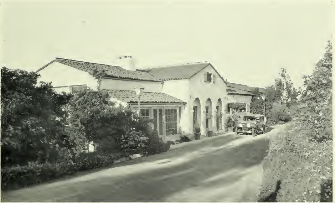
SOUTH FRONT, GOLF CLUB HOUSE, PALOS VERDES ESTATES Clarence E. Howard, Architect
