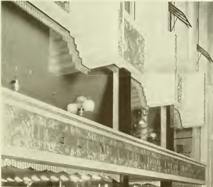
CLOSE-UP VIEW OF REMODELED ARCADE BUILDING, SAN DIEGO
