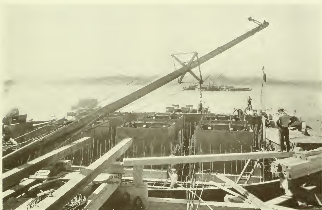
FORMS FOR CAISSON, SUISUN BAY BRIDGE, NEAR BENICIA, CALIFORNIA
