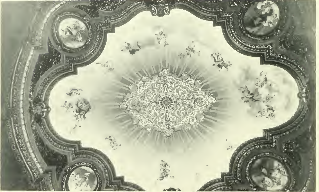
CEILING IN MAIN AUDITORIUM, FOX THEATER, SAN FRANCISCO Thos. W. Lamb, Architect; H. A. Minton, Associate
