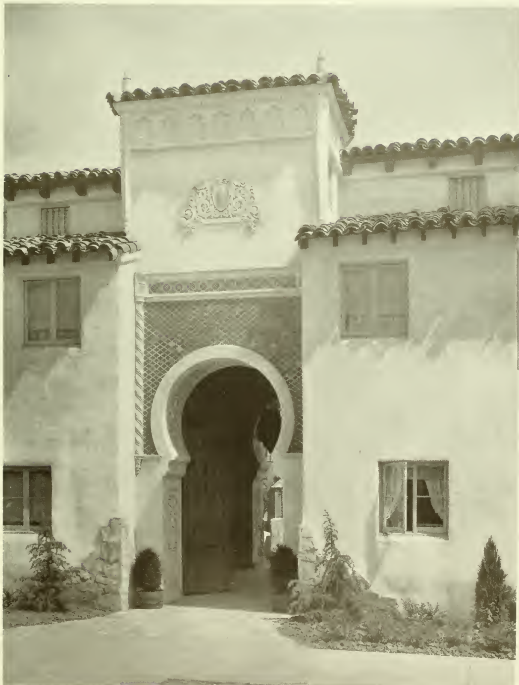
ENTRANCE, CIELITO LINDO APARTMENTS, OAKLAND, CALIFORNIA CASEBOLT DAKIN, ARCHITECT
