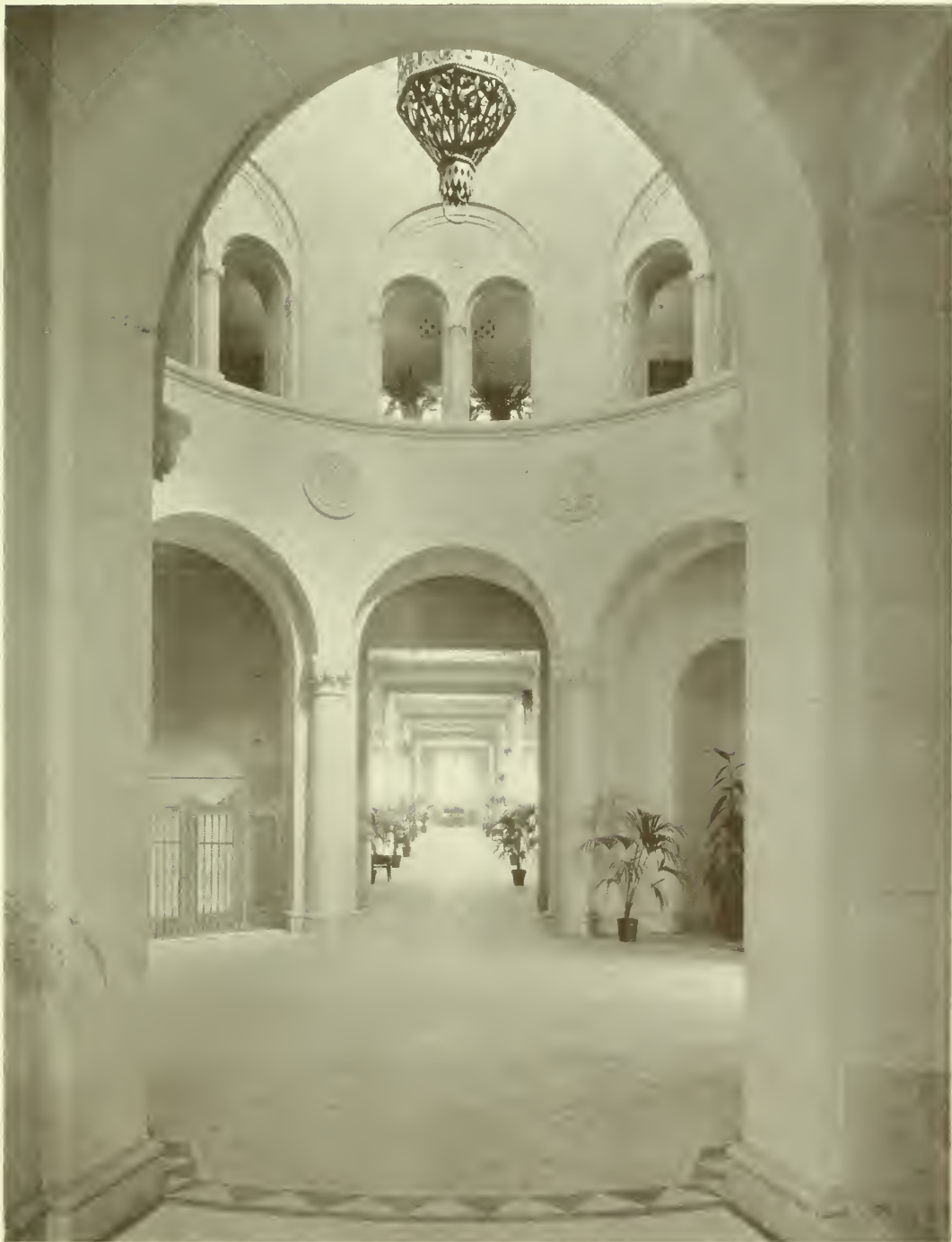
ROTUNDA, OAK HILL MAUSOLEUM, SAN JOSE, CALIFORNIA ALBERT F. ROLLER, ARCHITECT
