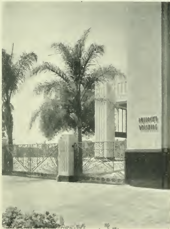
ENTRANCE GATES TO PARKING SPACE, BULLOCK'S WILSHIRE STORE, LOS ANGELES
