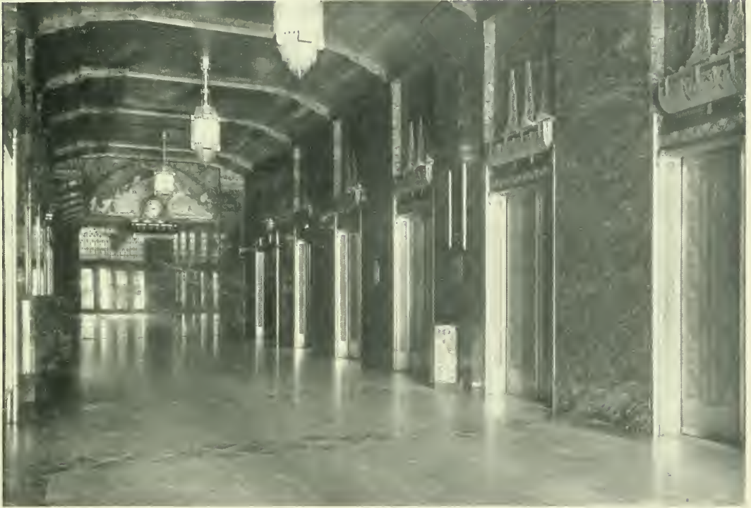
MAIN LOBBY, NORTHERN LIFE TOWER, SEATTLE, WASHINGTON
