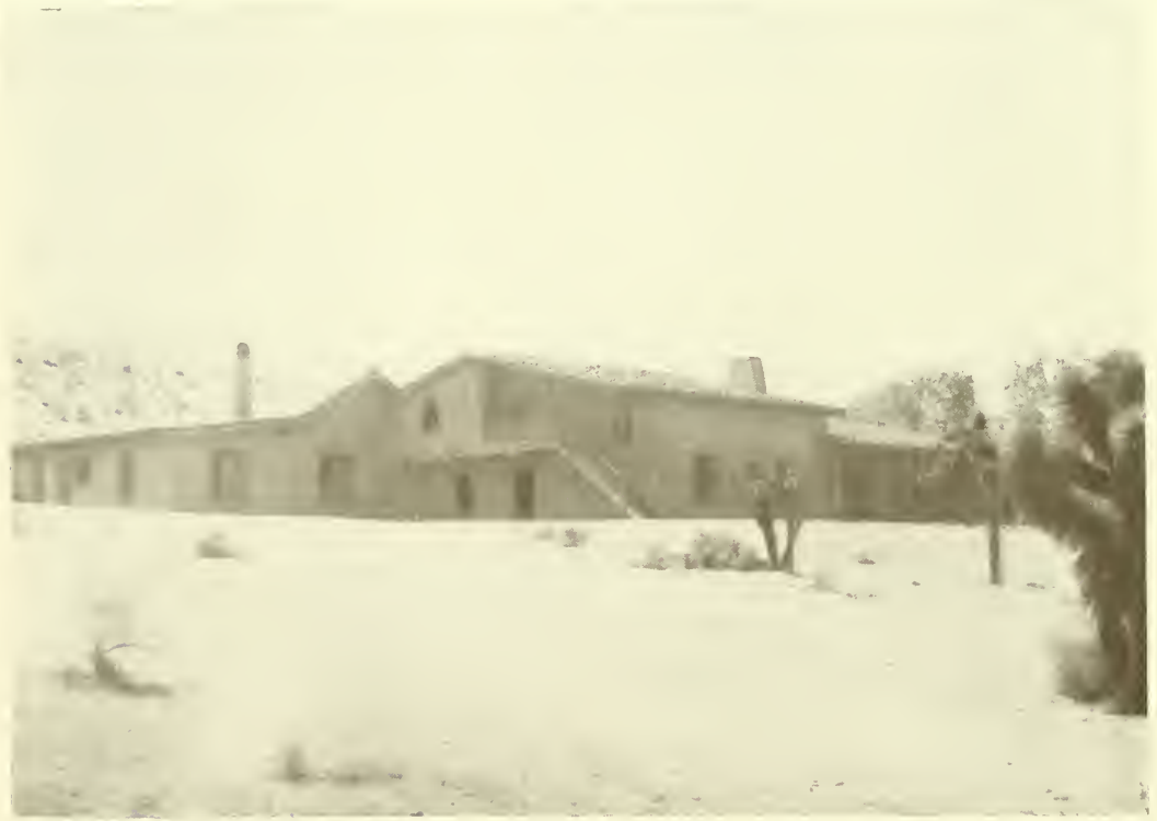
RANCH HOUSE FOR KEMPER CAMPBELL, VICTORVILLE, CALIFORNIA
