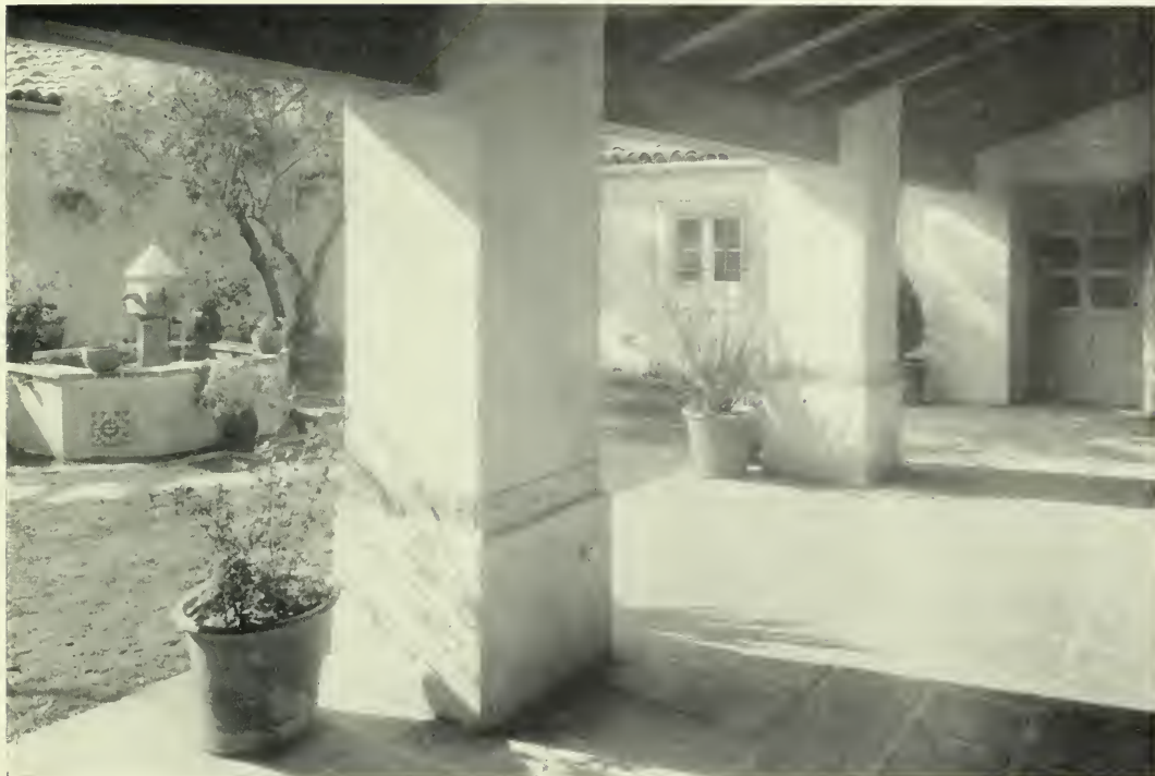
PATIO, RESIDENCE OF H. LEMONT SCHMIDT, PALOS VERDES ESTATES
