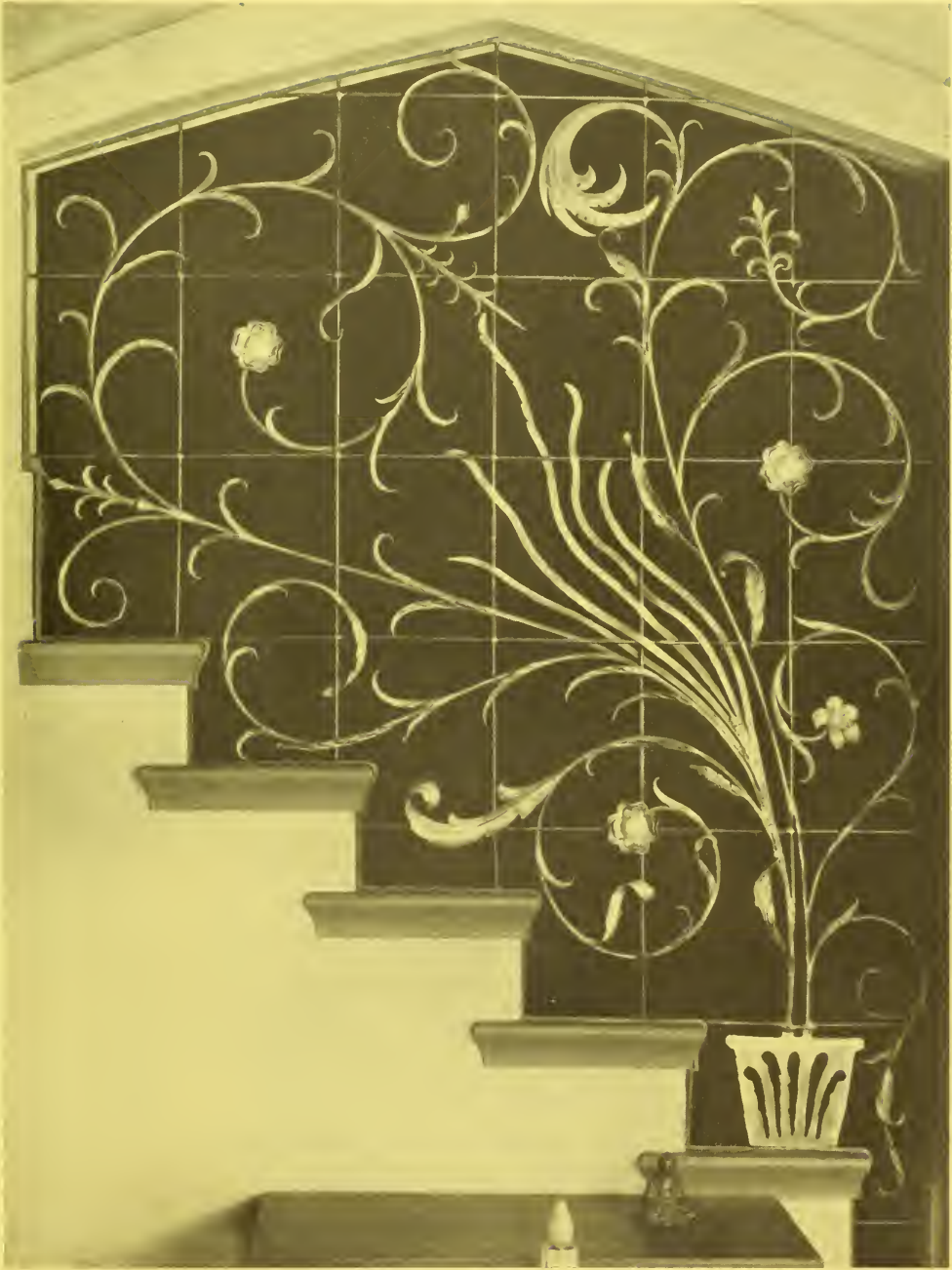
THIS RAIL IN IRON CLIMBS IN WELL ORDERED LINES AND FORM UP THE STAIR, FUNCTIONING AS A GUARD AND GUIDE AND FORGED WITH SKILL AND BEAUTY. RESIDENCE IN OAKLAND, CHARLES W. McCALL, ARCHITECT
