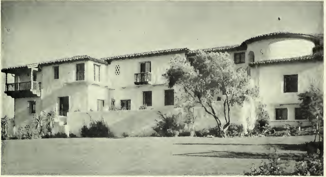
NORTH FACADE, RESIDENCE OF EARLE W. GARD, PALOS VERDES ESTATES Kirtland Cutter, Architect
