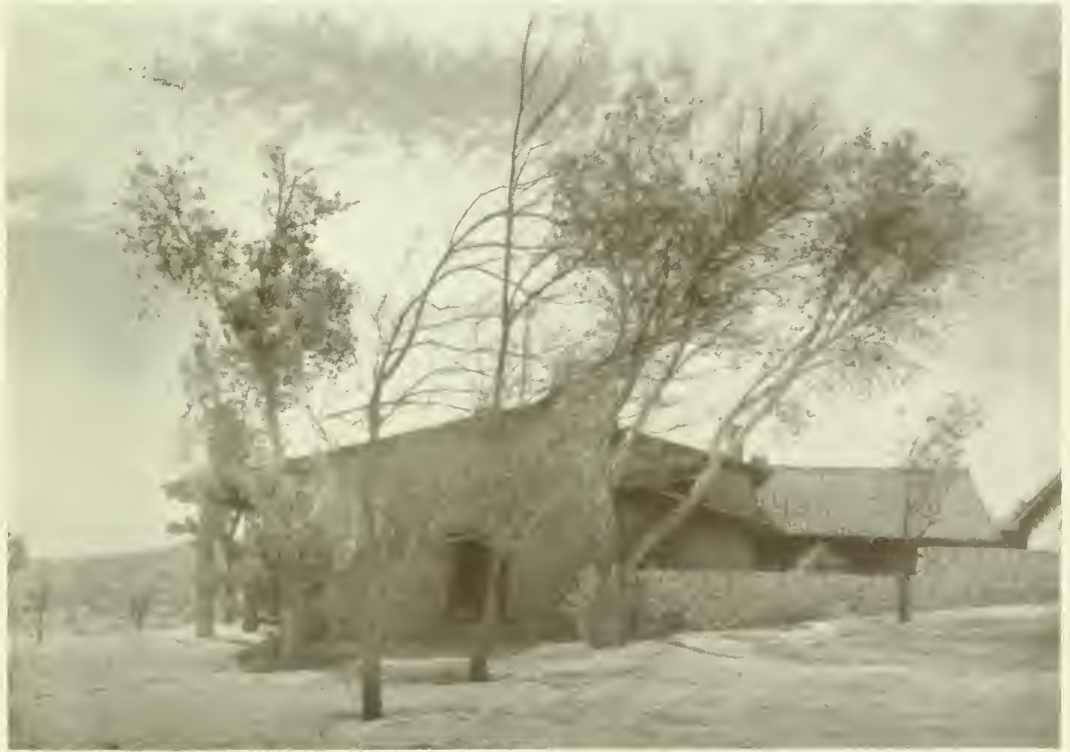
RANCH HOUSE FOR KEMPER CAMPBELL, VICTORVILLE, CALIFORNIA
