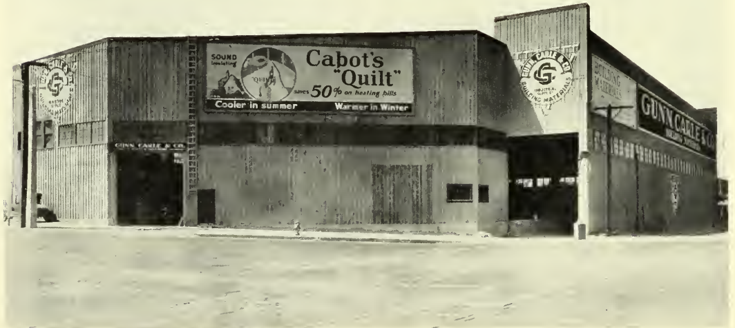
NEW WAREHOUSE OF GUNN, CARLE & CO., SAN FRANCISCO
