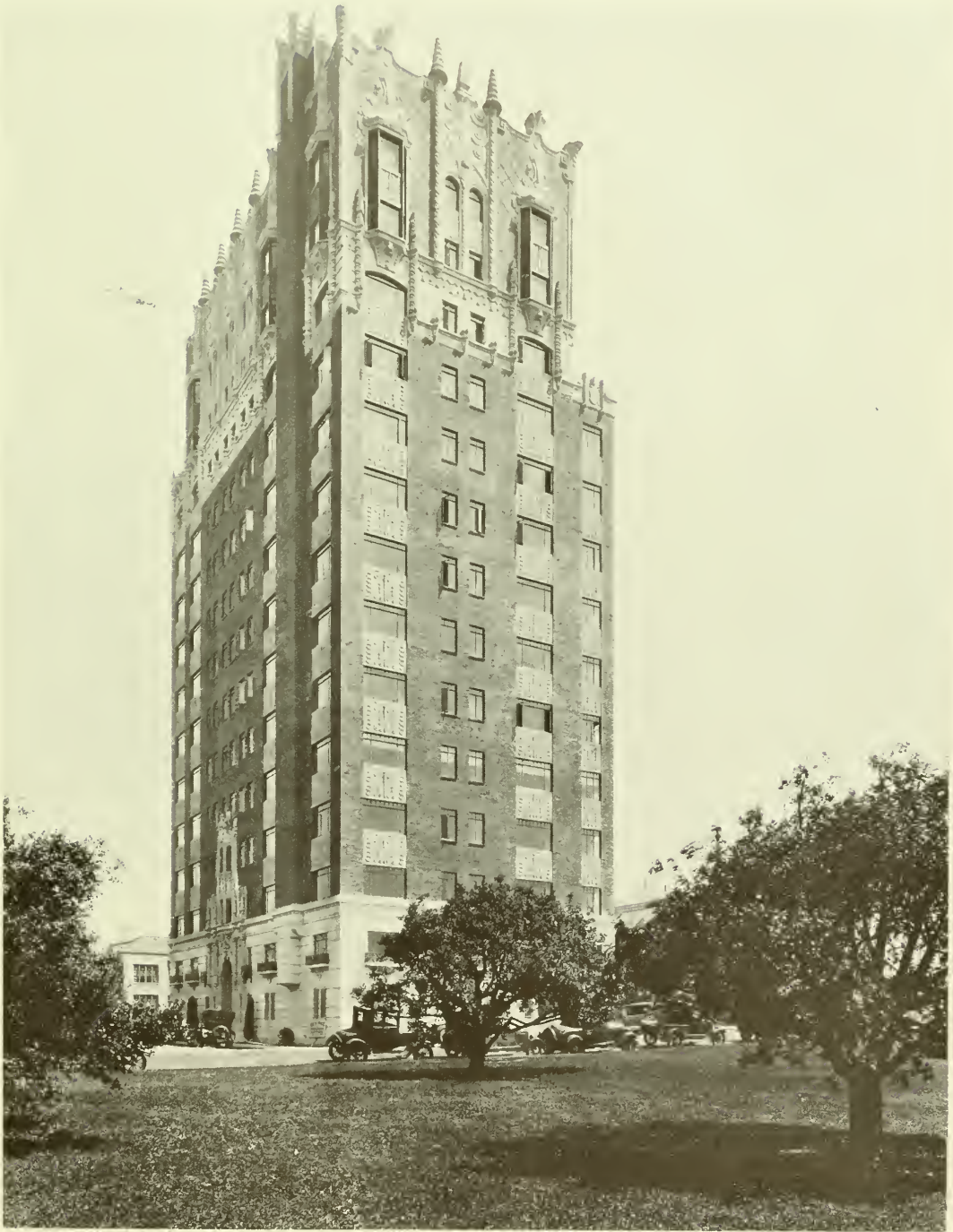
BELLEVUE STATEN APARTMENTS, OAKLAND, CALIFORNIA H. C. BAUMANN, ARCHITECT
