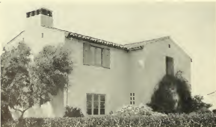
SIDE VIEW, RESIDENCE ON GRANVIA LA COSTA Winchton L. Risley, Architect
