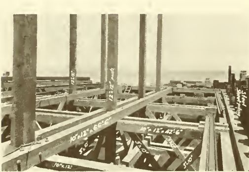
FIG. 3—INTERIOR BRACING AND STRUTTING
