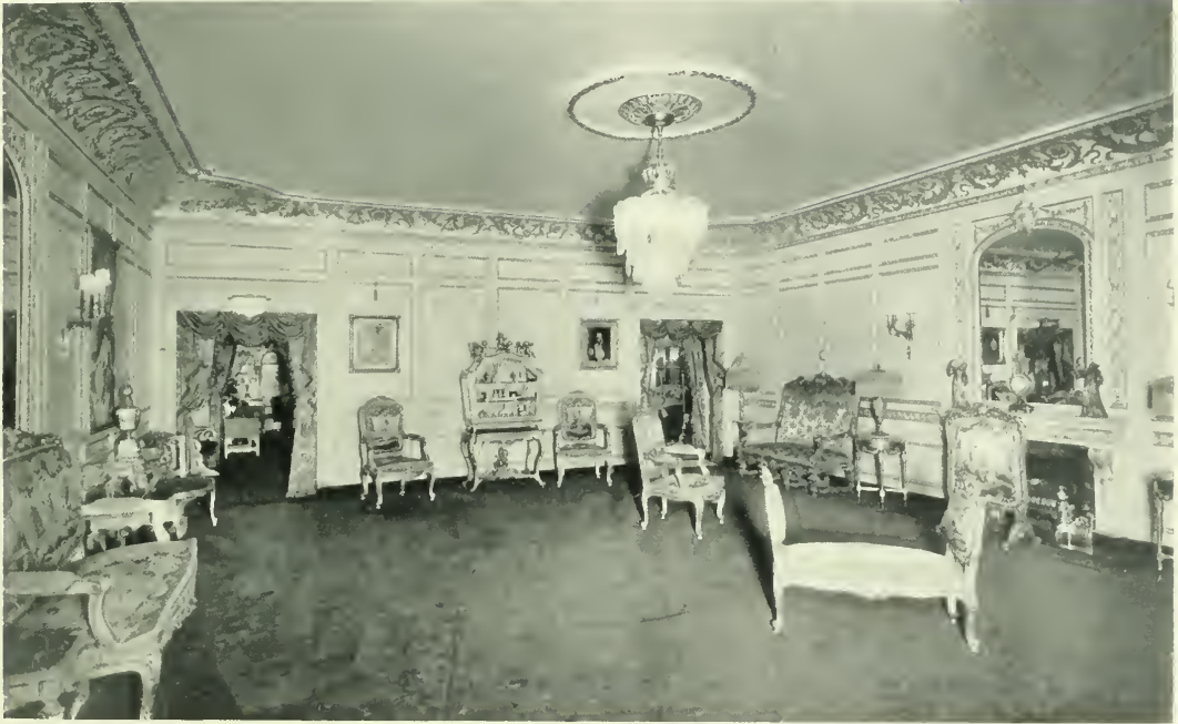
WOMEN'S LOUNGE, FOX THEATER, SAN FRANCISCO Thos. W. Lamb, Architect; H. A. Minton, Associate
