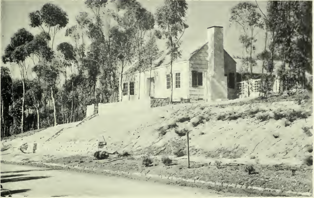
RESIDENCE OF MISS STELLA SMITH, PALOS VERDES ESTATES Winchton L. Risley, Architect
