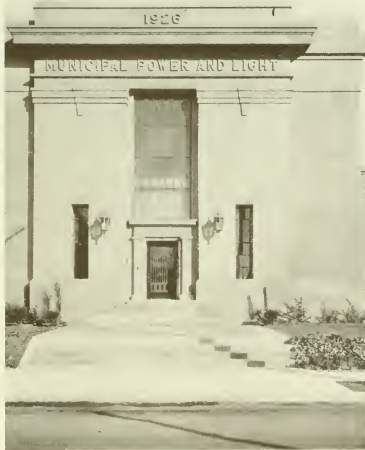
TRINITY STREET DISTRIBUTING STATION
