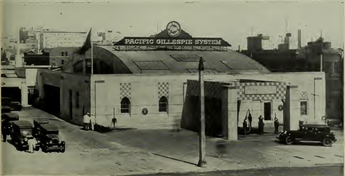
PACIFIC GILLESPIE SYSTEM BUILDING, SAN FRANCISCO Villadsen Bros., Inc., Constructors
