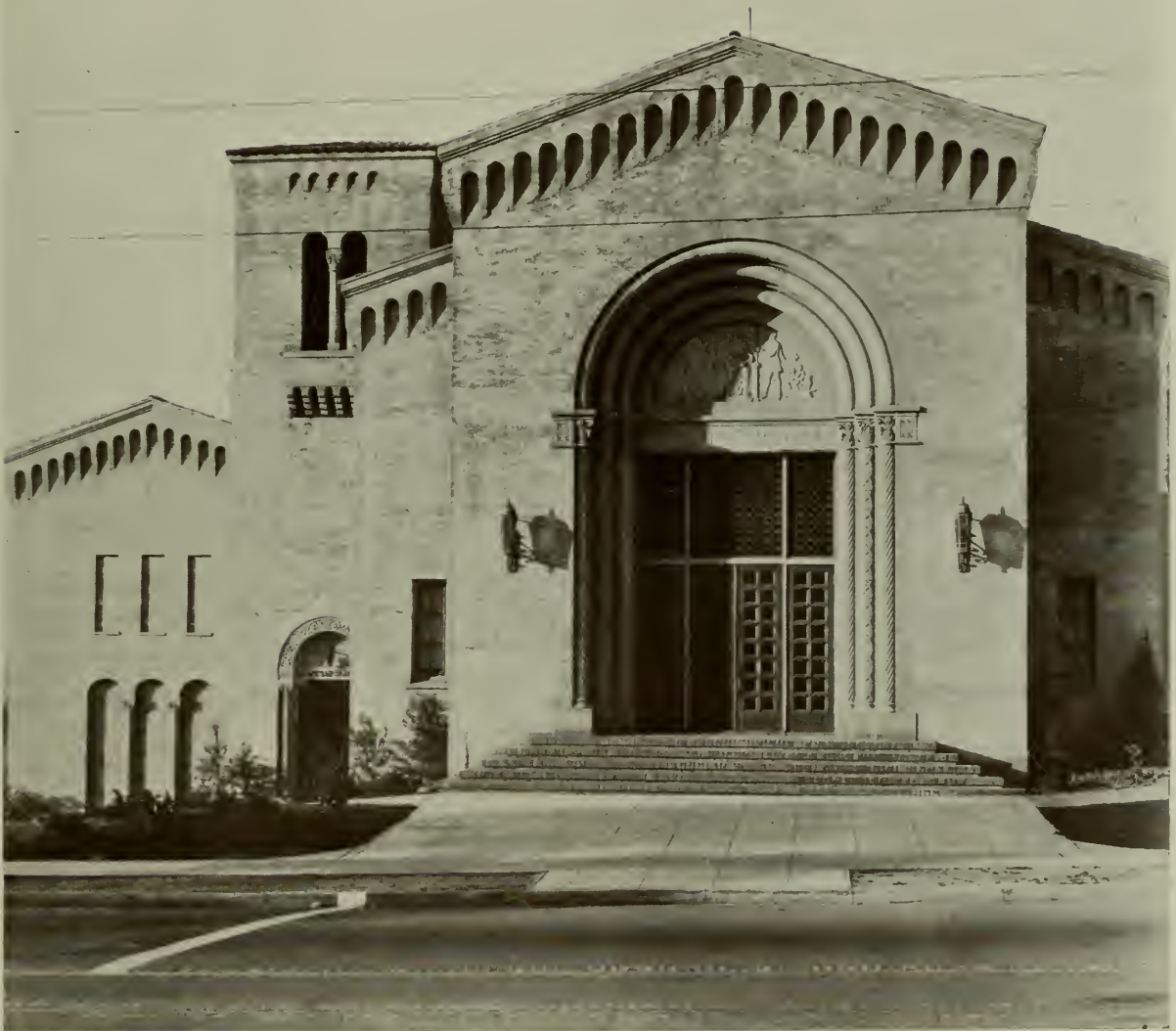
GRAND AVENUE SCHOOL, SOUTH SAN FRANCISCO, CALIFORNIA E. L. NORBERG AND JOHN E. NORBERG, ARCHITECTS
