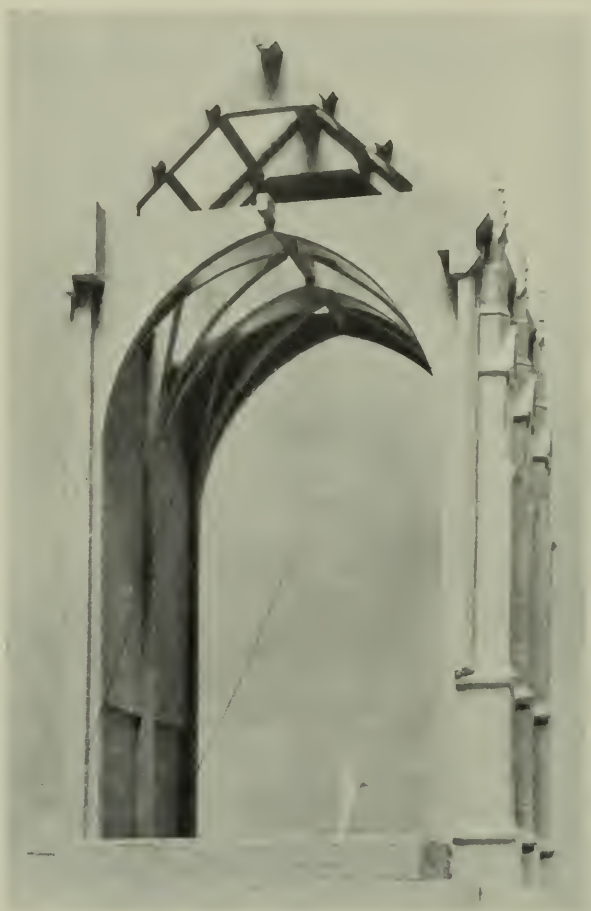
MODEL OF CONCRETE CONSTRUCTION OF GRACE CATHEDRAL CHAPEL, SHOWING RIBS AND VAULTING
