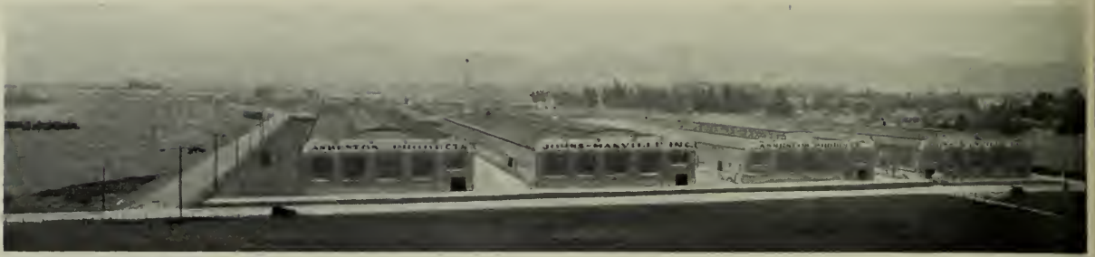
JOHNS-MANVILLE PLANT, PITTSBURGH, CALIFORNIA; THE TWO WINGS ON THE LEFT ARE BEING ADDED H. J. Brunner, Structural Engineer
