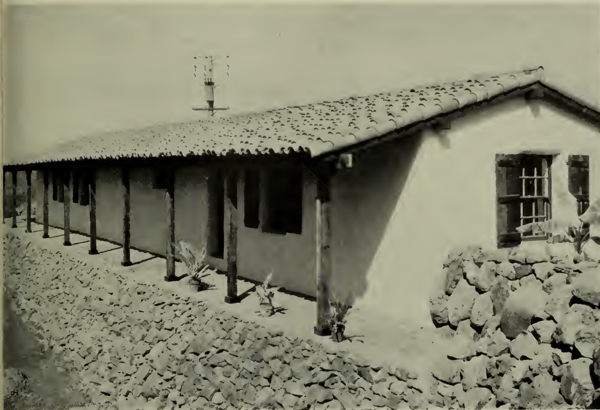
PUMPHOUSE, ESTATE OF DOUGLAS FAIRBANKS AND MARY PICKFORD, RANCHO SANTA FE L. J. Rice, Architectural Supervisor
