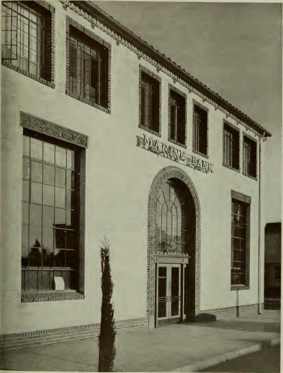
MARINE BANK BUILDING, SANTA MONICA, CALIFORNIA HENRY F. WITHEY, ARCHITECT
