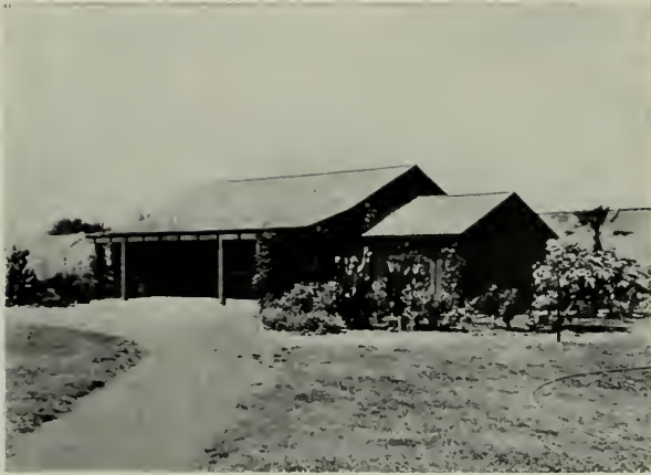
SUPERINTENDENT'S HOME, AUTOMOBILE PARK, MARYSVILLE
