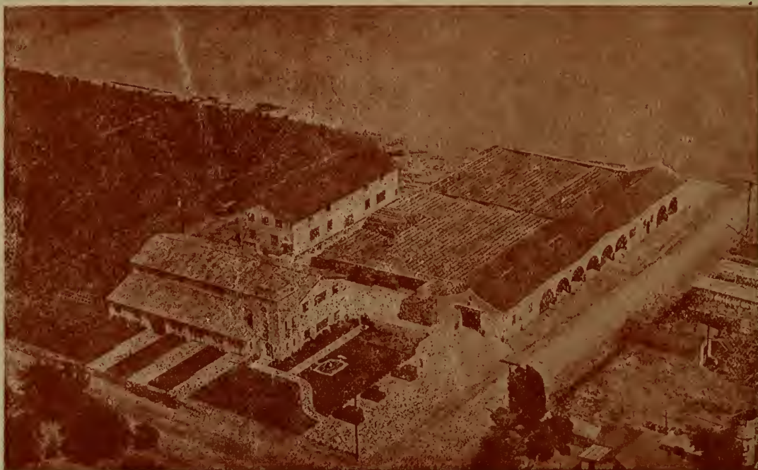
New home of John Bodger & Sons Company at El Monte, the largest and most modern seed plant in the world. It was constructed with Monolith Plastic Waterproof Portland Cement.
