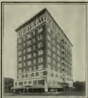
Oakland — Medical Arts Building
