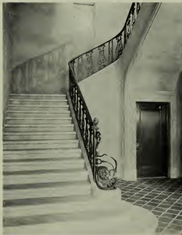
INTERIOR STAIRWAY, PASADENA CITY HALL Bakewell and Brown, Architects
