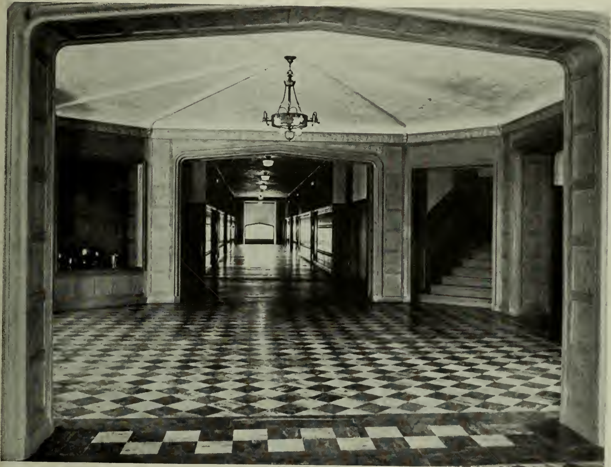
LOBBY, ACADEMIC BUILDING, UNION HIGH SCHOOL, SAN MATEO
