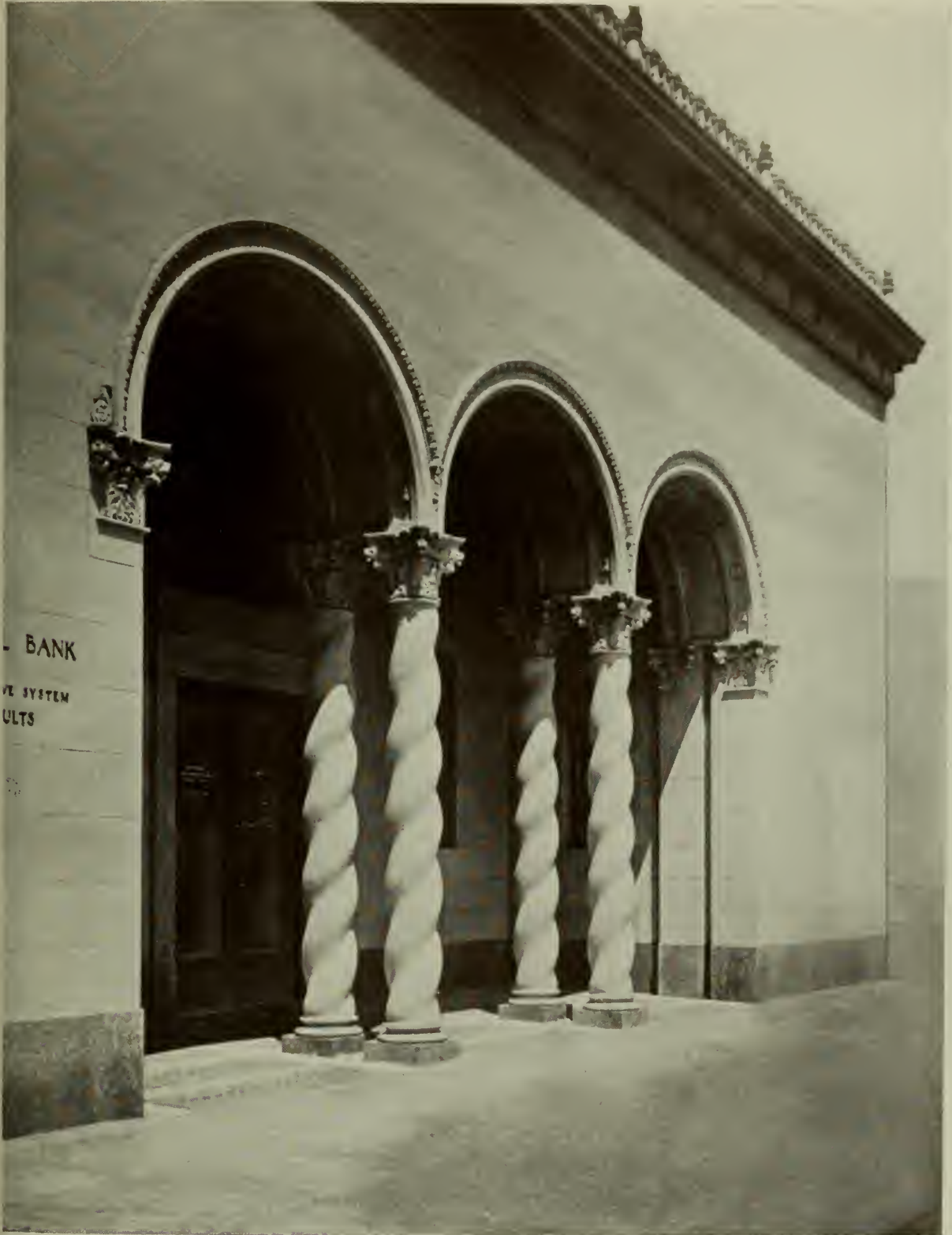
ENTRANCE DETAIL, FIRST NATIONAL BANK, ARTESIA, CALIFORNIA HENRY F. WITHEY, ARCHITECT
