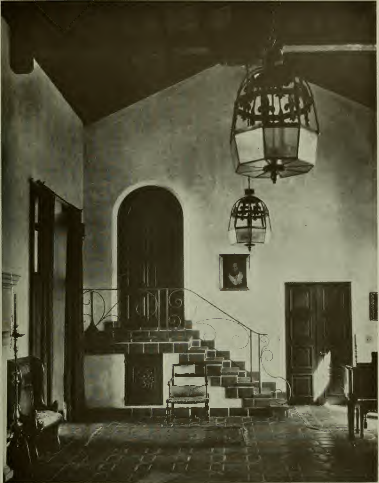
HOUSE OF CHARLES LUX LEWIS, LOS ANGELES, CALIFORNIA JOHN K. BRANNER, ARCHITECT
