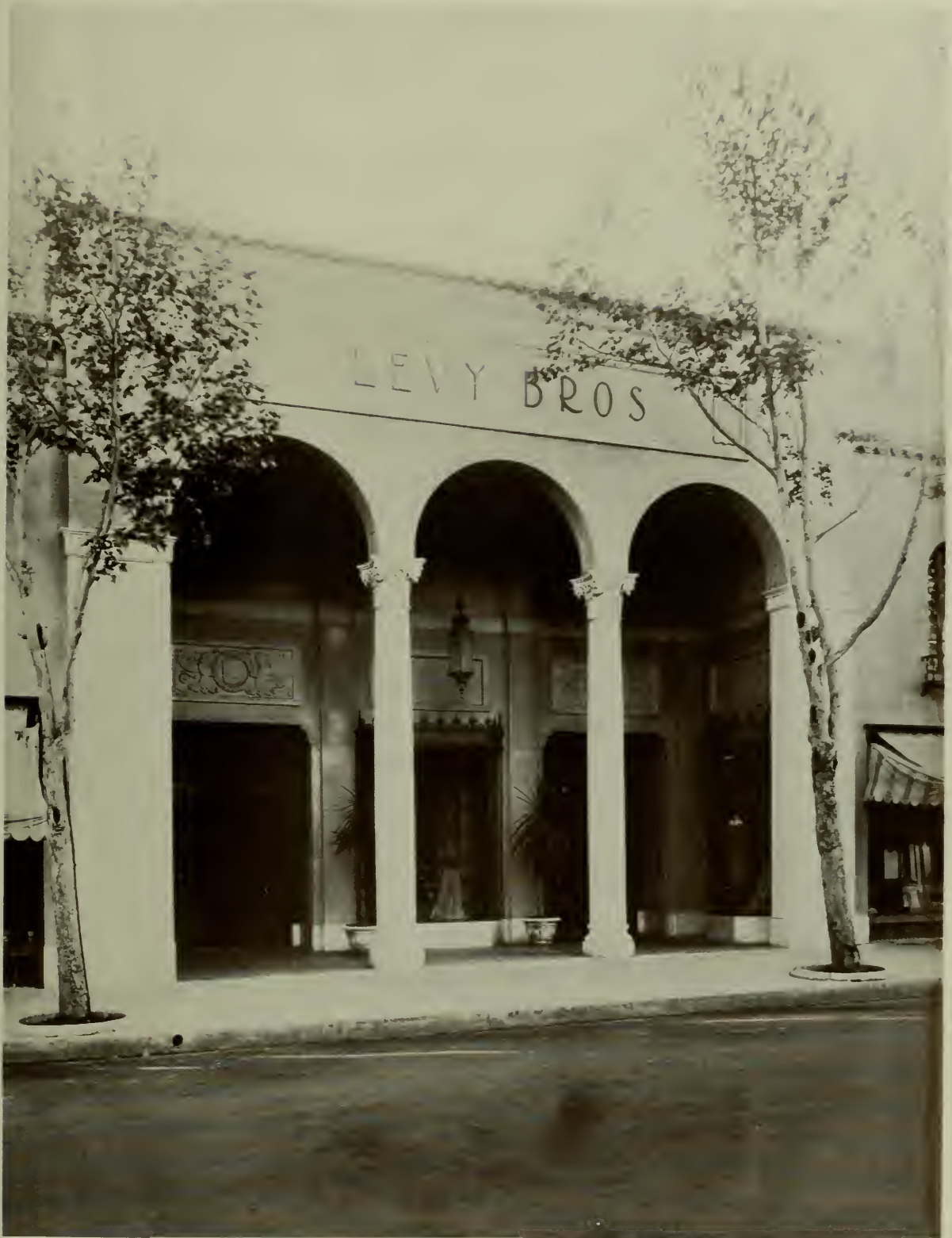
ENTRANCE DETAIL, STORE BUILDING FOR LEVY BROS., BURLINGAME E. L. NORBERG AND JOHN E. NORBERG, ARCHITECTS
