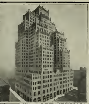
St. Louis — Bell Telephone Building
