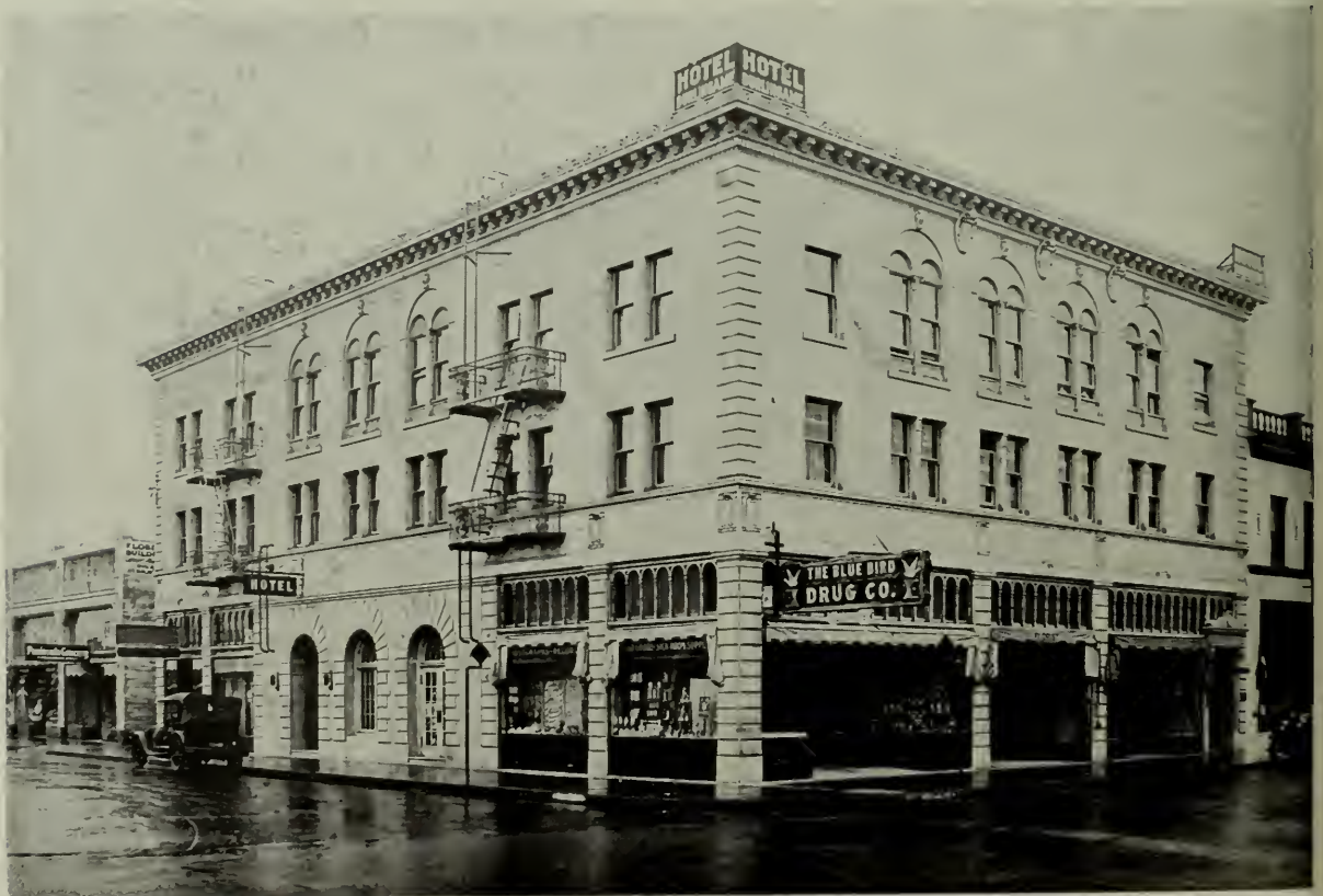
HOTEL BURLINGAME, BURLINGAME, CALIFORNIA E. L. Norberg and John E. Norberg, Architects
