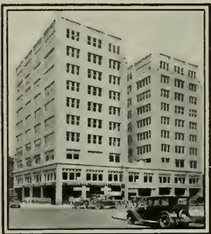
Detroit — Stephenson Building
