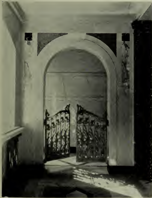
CORRIDOR, THE CATACOMBS, CYPRESS LAWN B. J. S. Cahill, Architect
