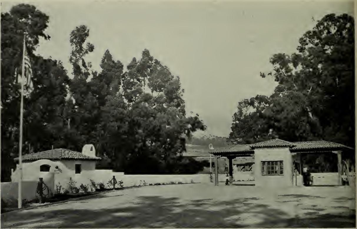
STANDARD OIL SERVICE STATION, SANTA BARBARA Edwards, Plunkett & Howell, Architects
