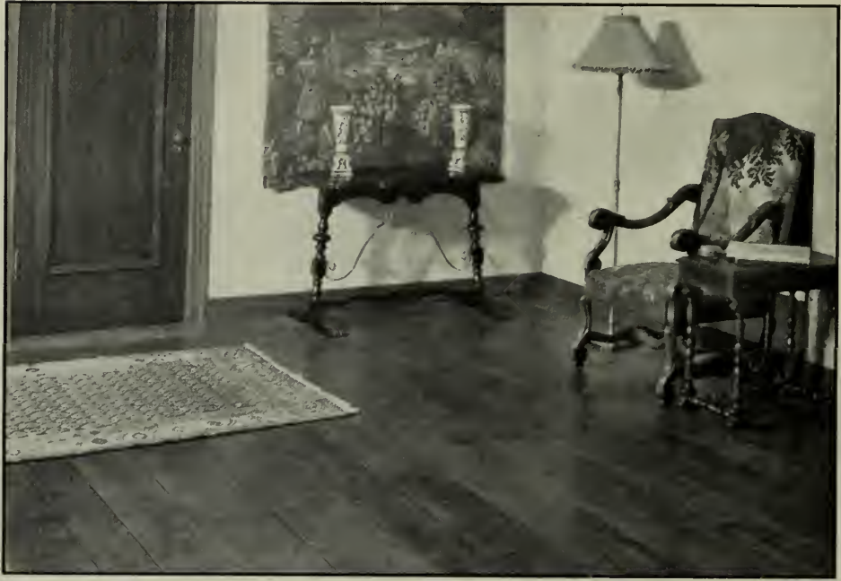
PLANK FLOORING LAID IN MASTIC
