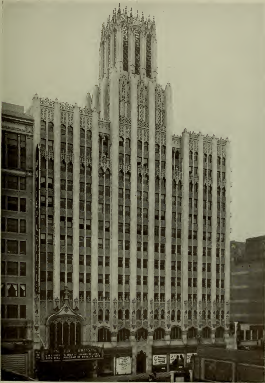
UNITED ARTISTS THEATER AND OFFICE BUILDING, LOS ANGELES WALKER AND EISEN AND C. HOWARD CRANE, ARCHITECTS
