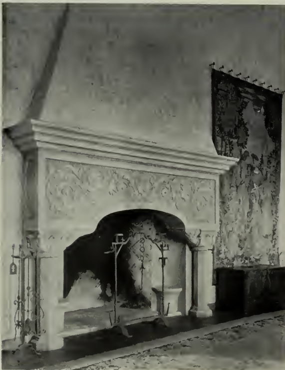
FIREPLACE, HOUSE FOR MR. RALPH LEE, HILLSBOROUGH A. F. Leicht, Architect
