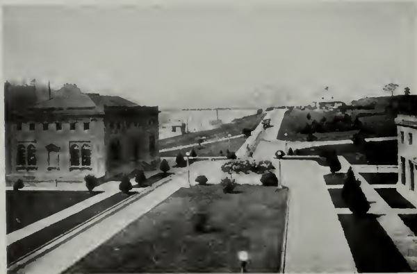
GOVERNMENT LOCK-SITE, SEATTLE Bebb and Gould, Architects
