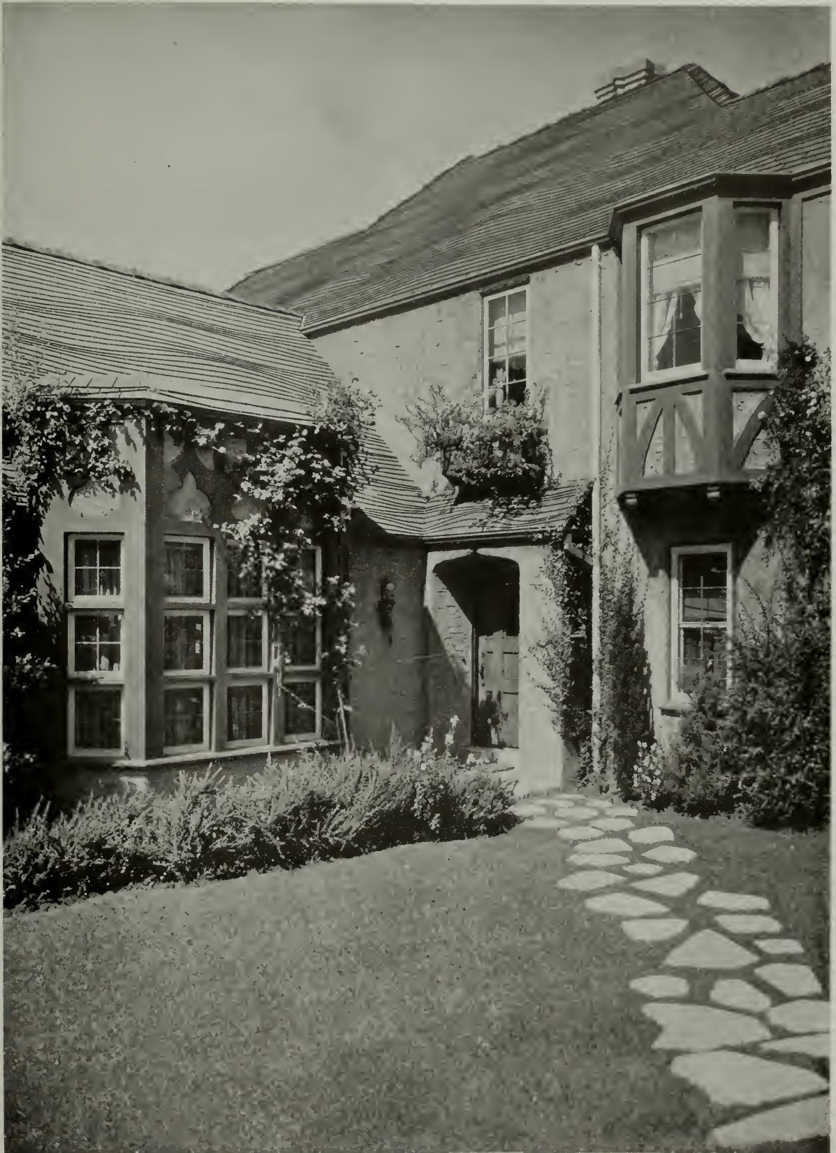
HOUSE FOR MR. R. W. OSBORN, BERKELEY, CALIFORNIA SIDNEY B. NOBLE AND ARCHIE T. NEWSOM, ARCHITECTS
