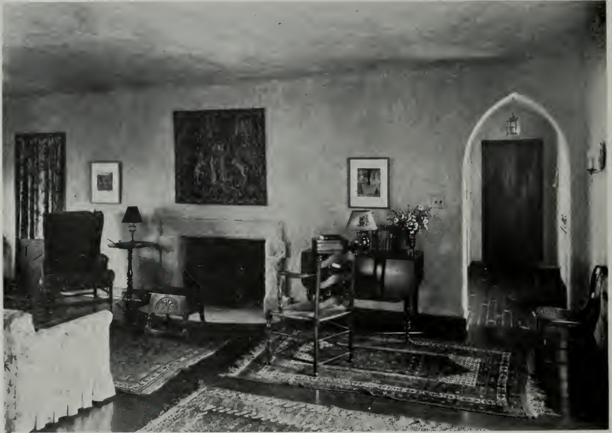
LIVING ROOM, HOUSE OF DARRAH CORBET, SEATTLE, WASHINGTON
