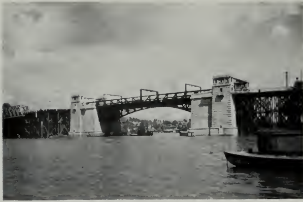
PIER OF LATONA BRIDGE, SEATTLE Daniel R. Huntington, Architect
