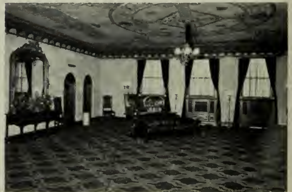
LOUNGE, BROADWAY THEATER, TACOMA Heath, Gove & Bell, Architects
