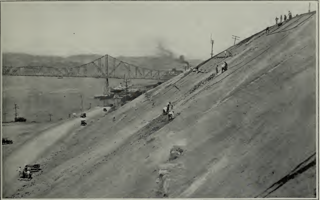
OVER AN ACRE OF CEMENT CONCRETE NOW WILL KEEP THE CONTRA COSTA HILLS FROM SLIDING OVER THE STATE HIGHWAY AT VALONA. THE NEW $8,000,000 CARQUINEZ HIGHWAY TOLL BRIDGE APPEARS IN THE VIEW.
