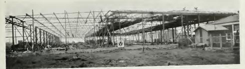
STEEL FRAME (ALL ELECTRICALLY WELDED) SHOP BUILDING FOR ASSOCIATED OIL COMPANY
