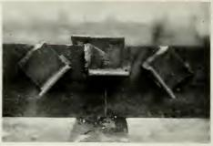
CLIPS FOR CROSS BRACING ON BOTTOM CHORD
