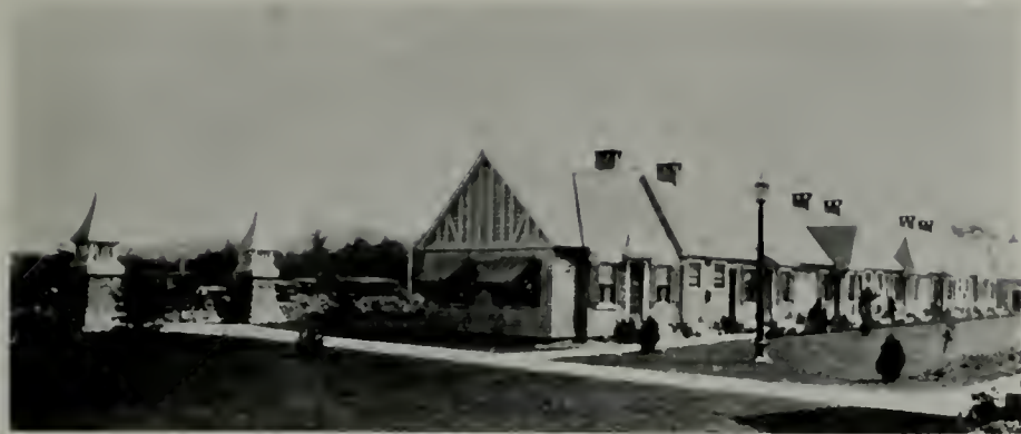
GATE ENTRANCE, APARTMENT COURT, SEASIDE, OREGON
