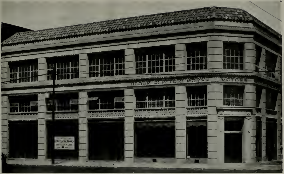
NEW HOME OF GLOBE ELECTRIC WORKS, SAN FRANCISCO Mark T. Jorgensen, Architect
