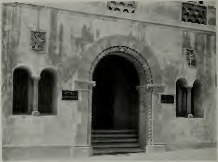
ENTRANCE, HOTEL CONSTANCE, PASADENA McNeal Swasey, Architect
