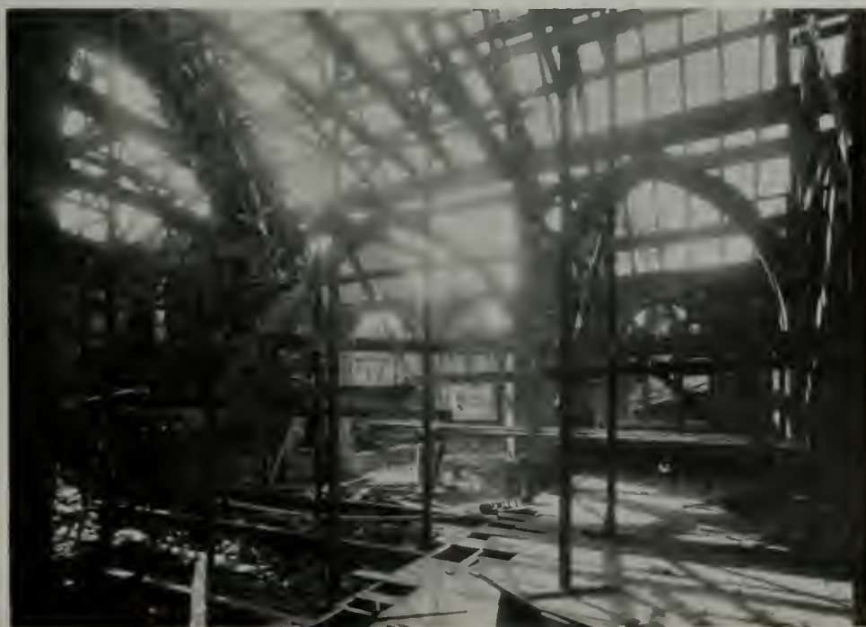
PROGRESS PICTURE, INTERIOR OF ST. PAUL'S CHURCH
