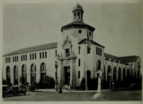
Automobile Club, Los Angeles Construction is concrete with portland cement stucco. Filler walls are monolithic auth concrete structural frame Architectis Hunt and Burns, Los Angeles. Contractor: C. J. Kubach Co., Los Angeles
