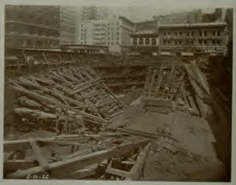
FIG II - STREET WALLS SHORED WITH HEAVY TIMBERS
