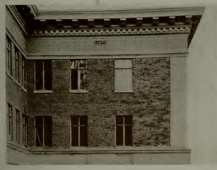
DETAIL OF CORNICE, MADE OF ARMCO SHEET METAL, BELVEDERE APARTMENTS
