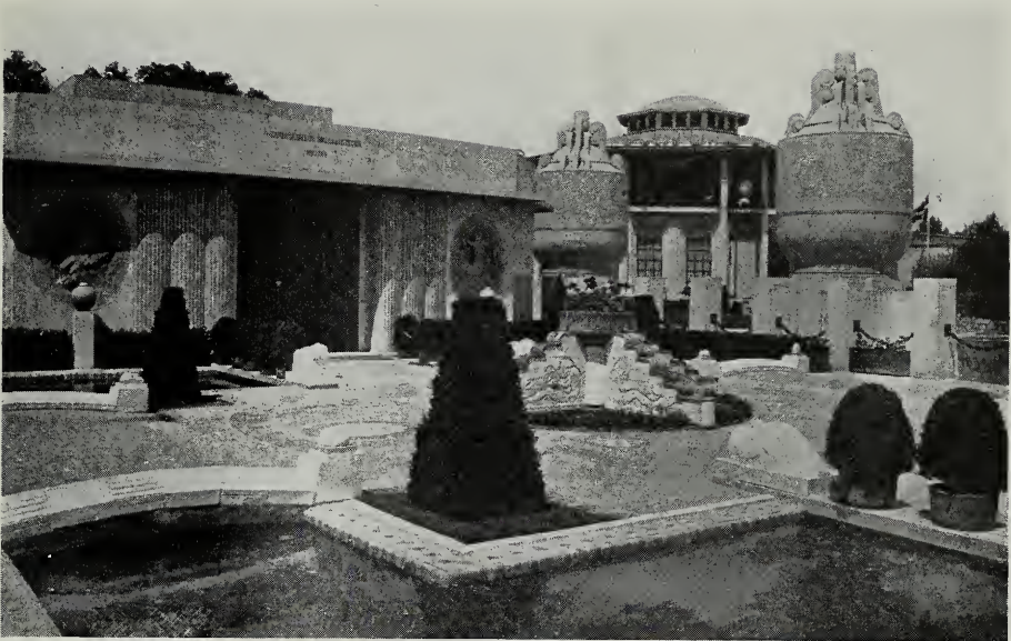
SEVRES PORCELAIN EXHIBIT M. Patout, Architect
