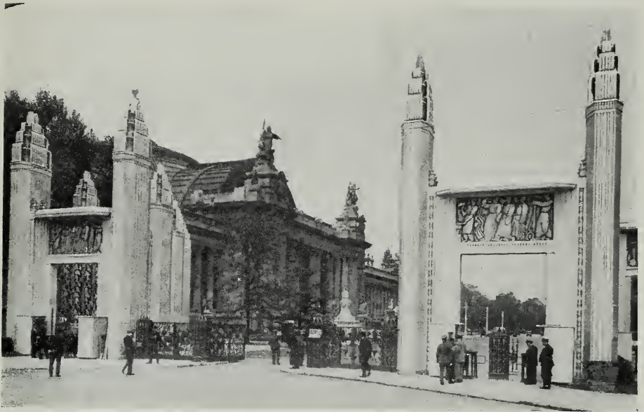
THE MAIN ENTRANCE GRILLE M. Brandt, Iron Worker
