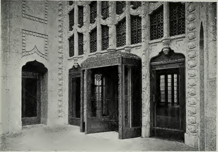
BRONZE DOORWAYS, FRONT ENTRANCE, TELEPHONE BUILDING
