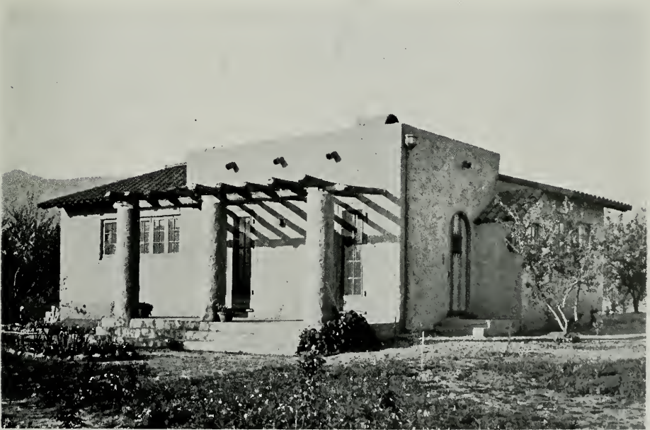
WEST VIEW OF COTTAGE NO. 3, KROTONA INSTITUTE OF THEOSOPHY Robt. B. Stacy-Judd, Architect
