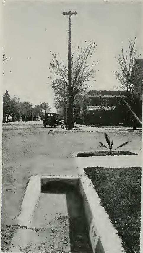
(Fig. 5) SHOWING ARMO PART CIRCLE CULVERT, REPLACING DIP AT B AND 18TH STREETS, BAKERSFIELD.
