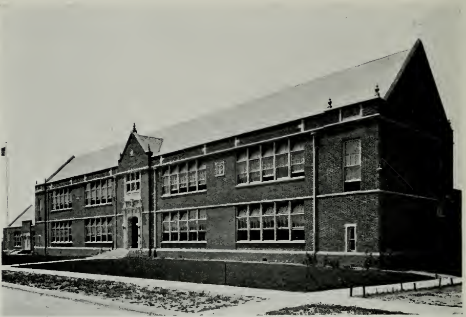
VAN NESS SCHOOL BUILDING, LOS ANGELES Noerenberg and Johnson, Architects
