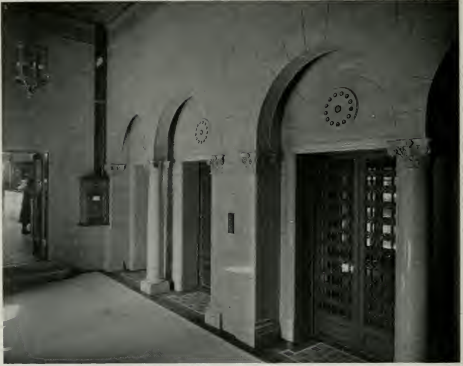
ELEVATOR LOBBY, TAFT BUILDING, HOLLYWOOD Walker and Eisen, Architects and Engineers
