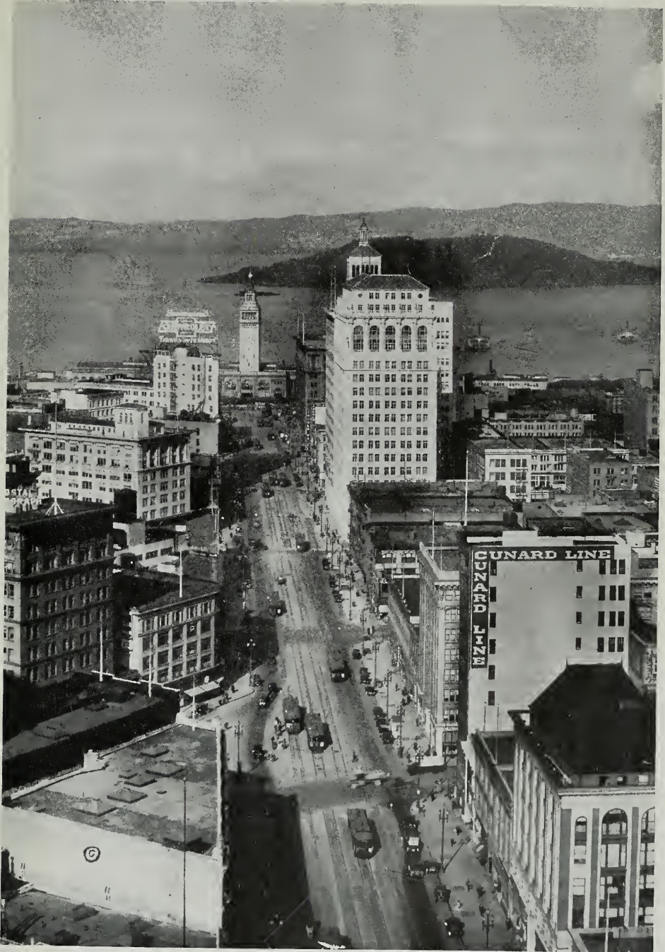
LOOKING DOWN MARKET STREET FROM SUTTER, SAN FRANCISCO P. G. & E. BUILDING ON THE RIGHT
