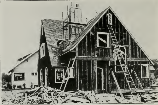
HOUSE COVERED WITH HERRINGBONE METAL LATH, READY FOR PLASTER
