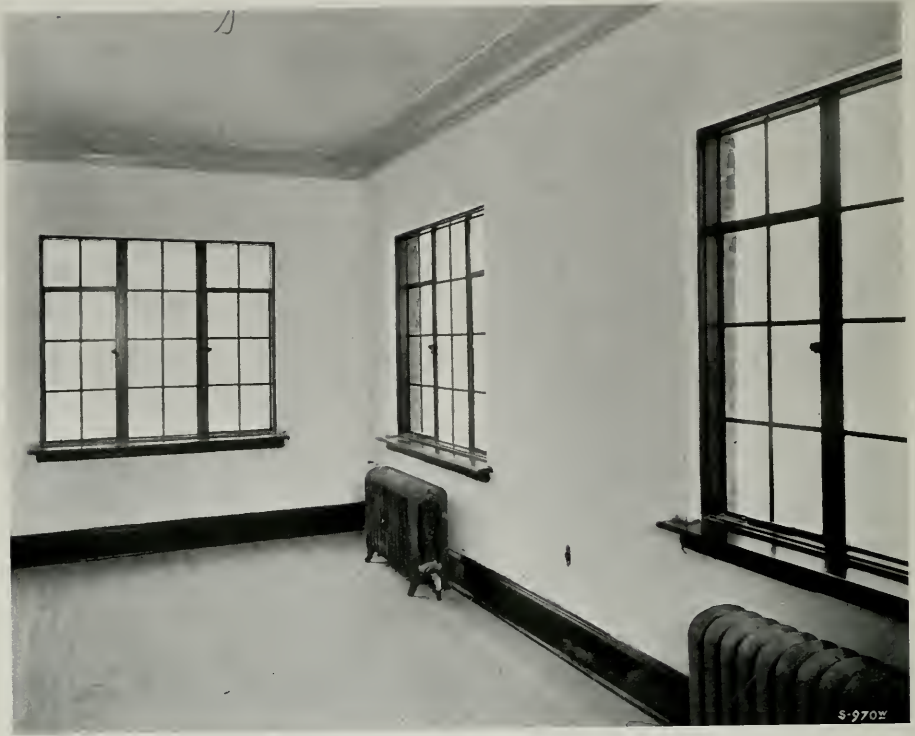
UNFINISHED STEEL CASEMENT INSTALLATION, SHOWING SCREEN STOPS IN PLACE
