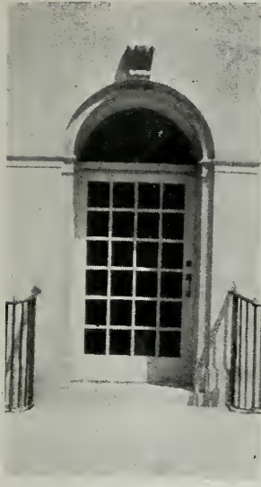
A French doorway with simple architectural treatment.
