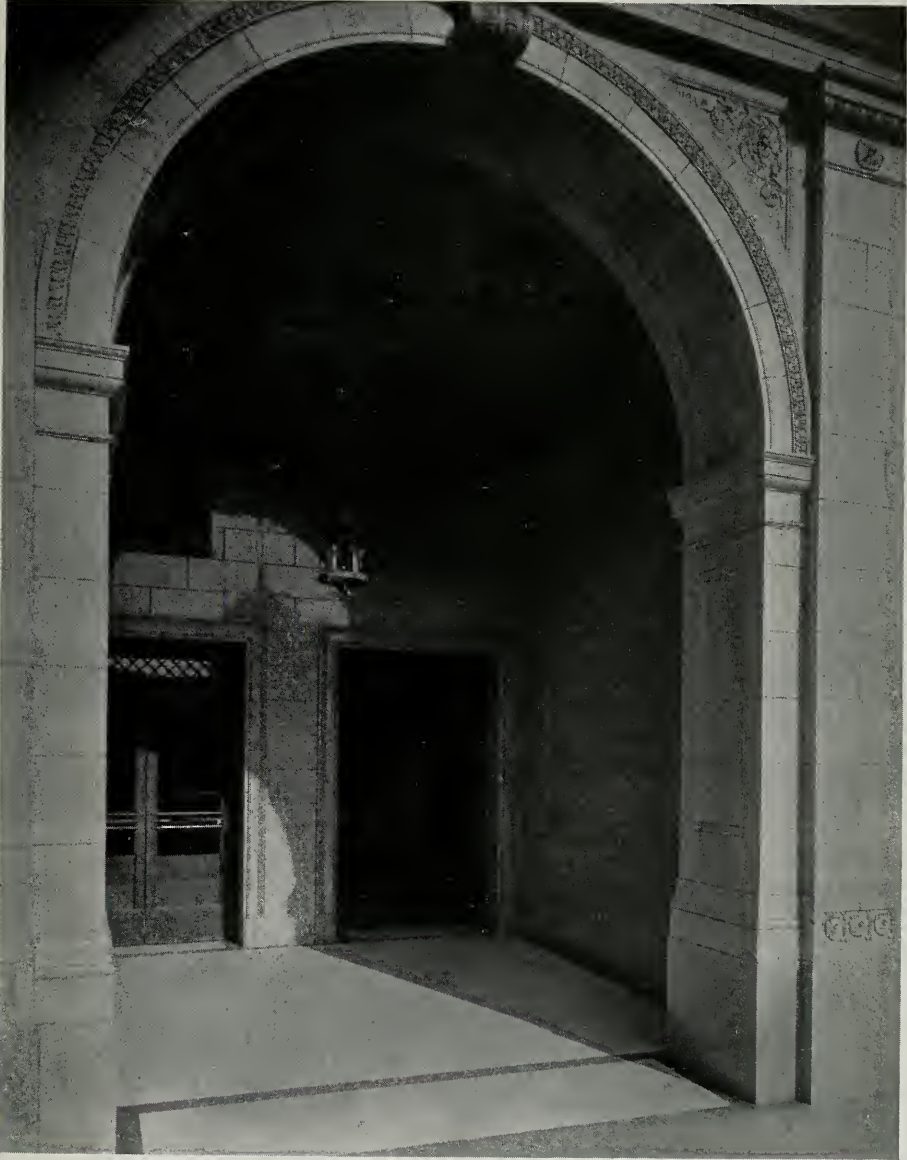
ENTRANCE DETAIL, TAFT BUILDING, HOLLYWOOD Walker and Eisen, Architects and Engineers
