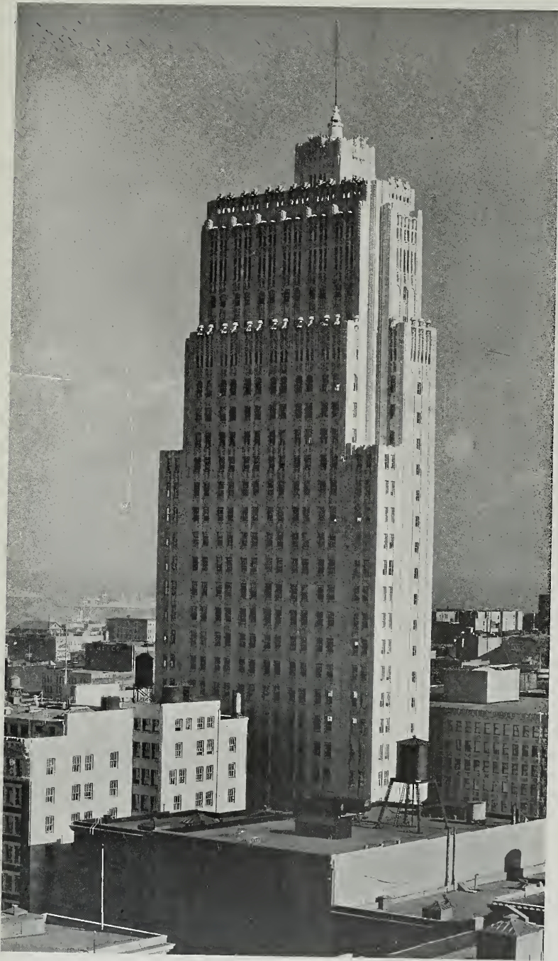
NEW MONTGOMERY STREET FACADE, TELEPHONE BUILDING, SAN FRANCISCO J. R. MILLER AND T. L. PFLUEGER, A. A. CANTIN, ASSOCIATED ARCHITECTS
