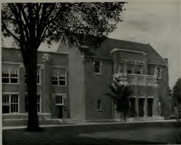
West Side Junior High School, Bay City, Michigan Perkins, Fellows & Hamilton, Architects Unglazed Terra Cotta used for ornamental trim throughout
