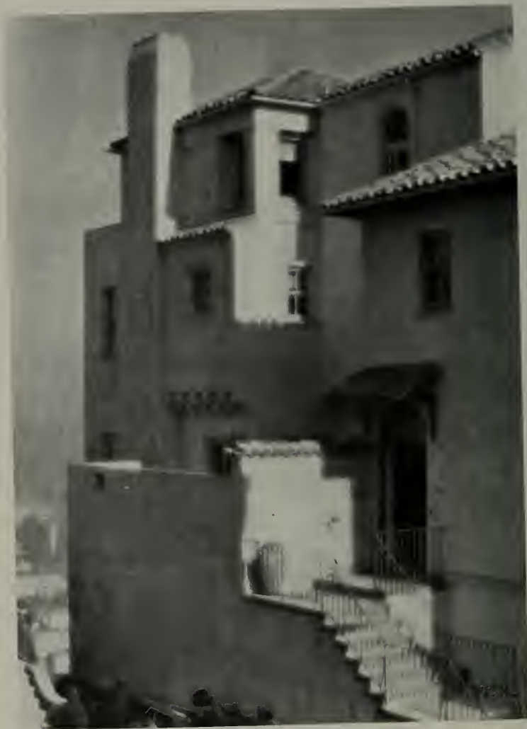
HOUSE OF MR. CHARLES LUX LEWIS, SAN FRANCISCO JOHN K. BRANNER, ARCHITECT
