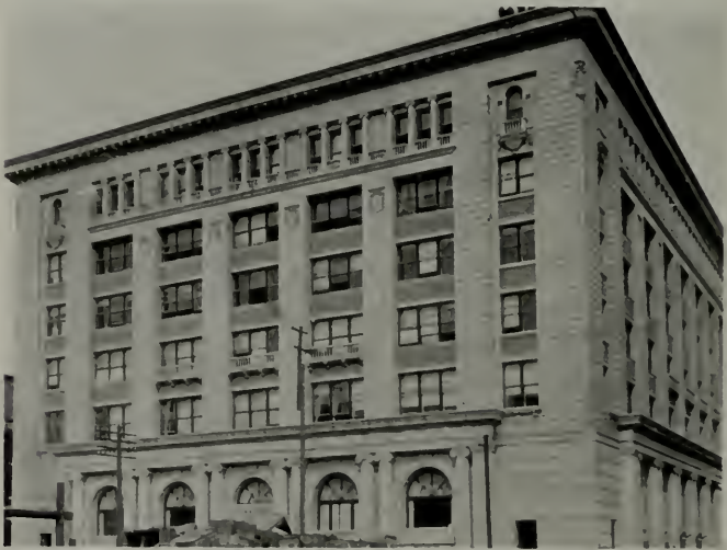
INDUSTRIAL BANK OF JAPAN, TOKYO Structural steel frame and reinforced concrete wall construction. Undamaged.
