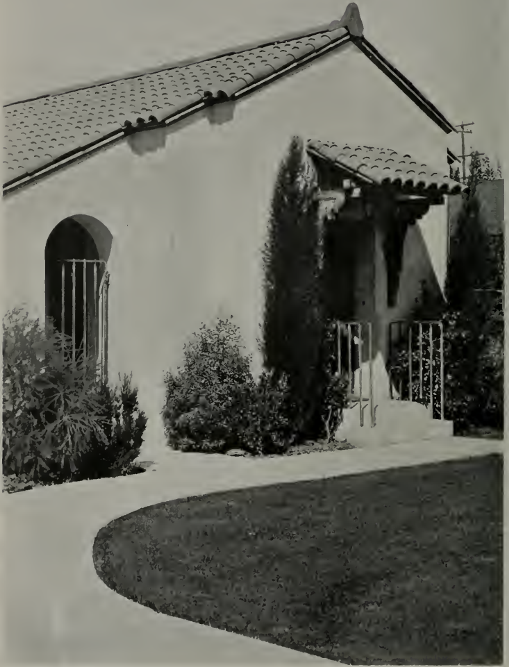
HOUSE AT ST. ANDREWS PLACE, LOS ANGELES ERNEST IRVING FREESE, ARCHITECT
