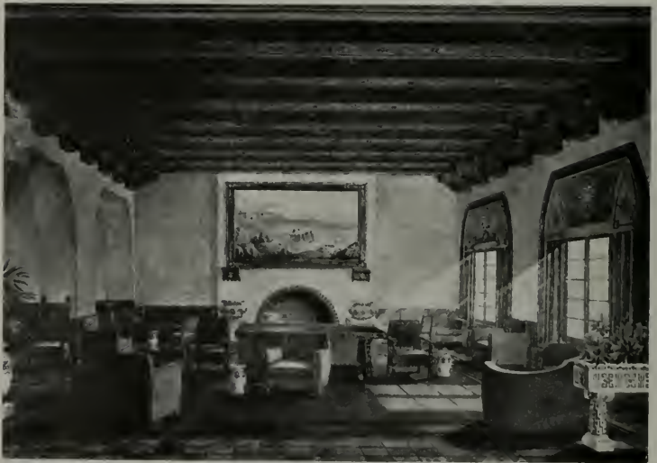
INTERIORS, HOTEL FRANCISCAN, ALBUQUERQUE TROST AND TROST, ARCHITECTS
