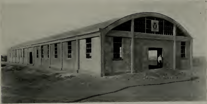
CONCRETE STOREHOUSE FOR ASSOCIATED OIL COMPANY, AVON
