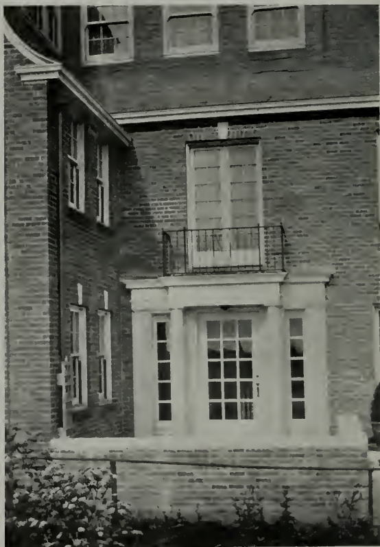
ENTRANCE DETAIL, RESIDENCE OF H. H. ASHLEY, SAN FRANCISCO Ashley and Evers, Architects
