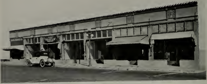
STORE BUILDING FOR LESLIE R. WILSON, OAKLAND Designed by Hutchison and Mills
