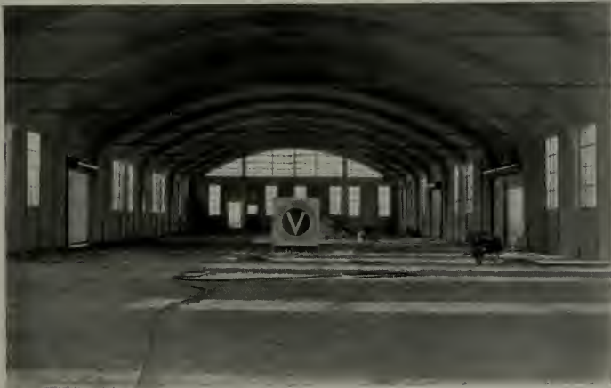
INTERIOR STOREHOUSE FOR ASSOCIATED OIL COMPANY, AVON
