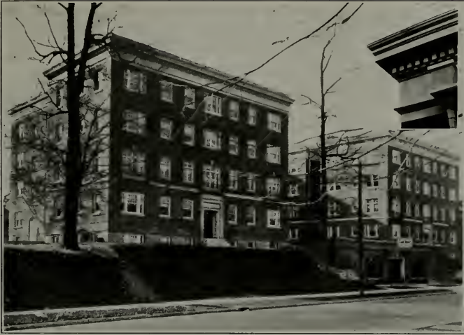
GRAND APARTMENT, DAYTON, OHIO H. C. Smith, Architect A. A. Smith, Sheet Metal Contractor. ARMCO-Ingot Iron sheet metal work throughout. Three and one-half tons used in cornice alone.
