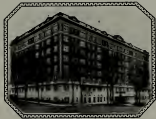
The Bellerive Apartments, Kansas City, use a Wayne Rapid-Rate Water Softener to free them from the expenses which hard water causes.
