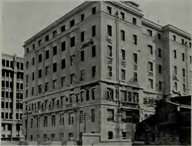
NATIONAL BANK OF JAPAN, TOKYO Reinforced concrete skeleton, brick walls, stone veneer. Slightly damaged.
