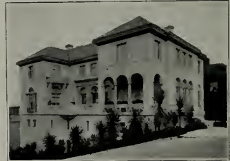
HEUTER RESIDENCE, SAN FRANCISCO Louis M. Upton, Architect
