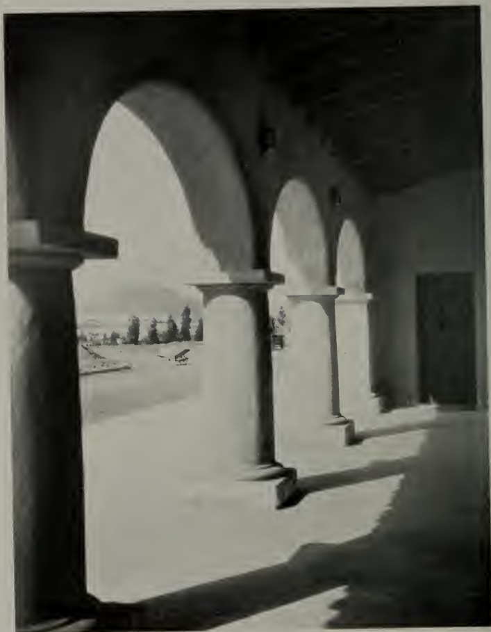
ARCADE, COMMERCIAL BUILDING, RANCHO SANTA FE, DEL MAR, CALIFORNIA REQUA AND JACKSON, ARCHITECTS
