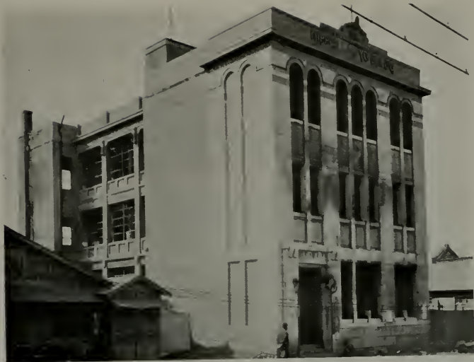
NIPPON KAIJO BUILDING, YOKOHAMA Reinforced concrete. Undamaged by earthquake.
