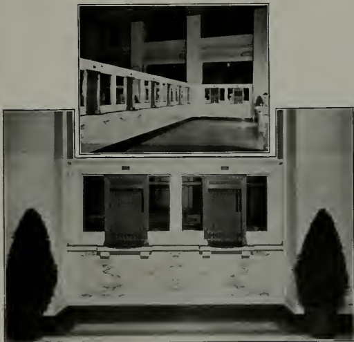
Matched panels of Madre Veined Alabama Marble in the Madison-Kedzie State Bank, Chicago, Ill. Cady & Crosby, Architects. Henry Marble Co.—Contractors.
