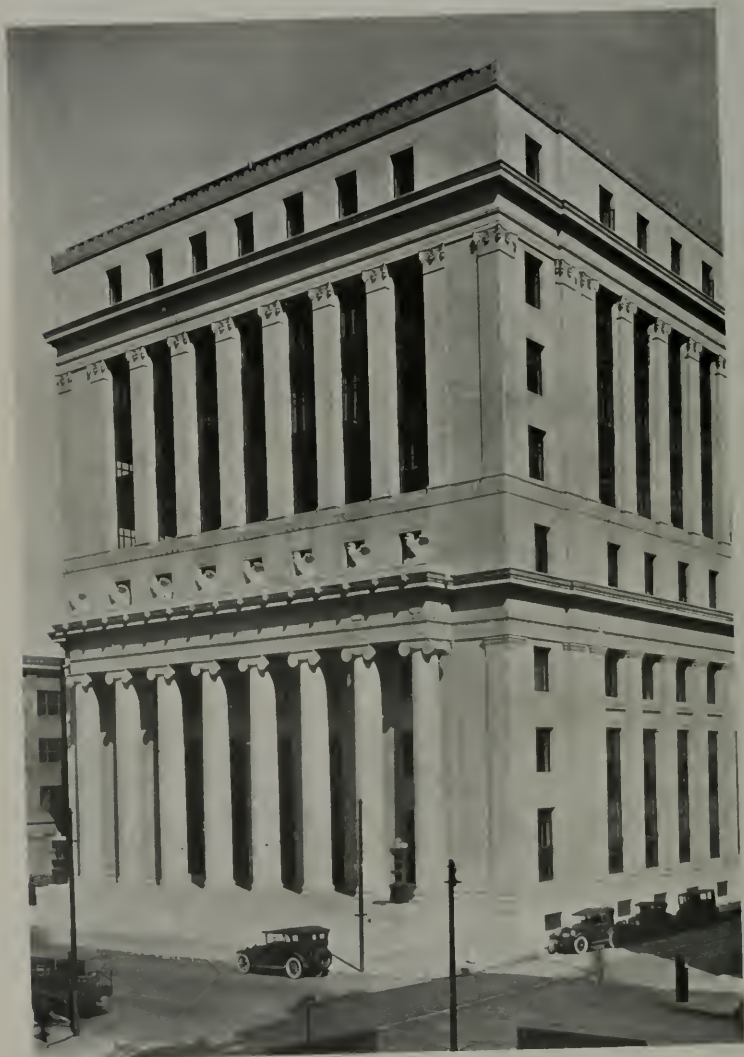
FEDERAL RESERVE BANK OF SAN FRANCISCO GEORGE W. KELHAM, ARCHITECT
