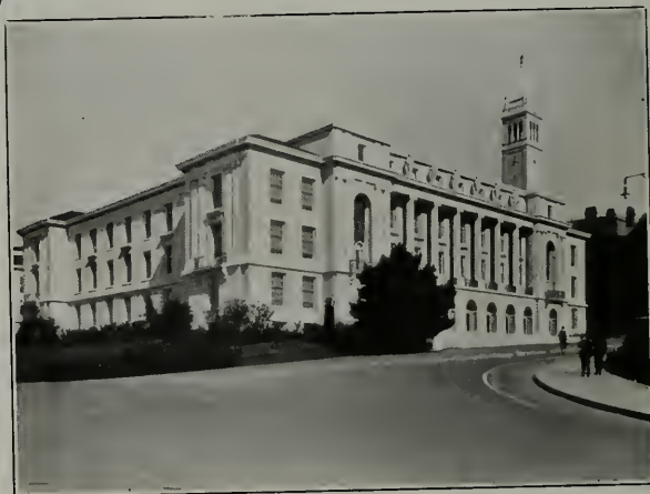
Wheeler Hall, University of California. John Galen Howard, Architect
