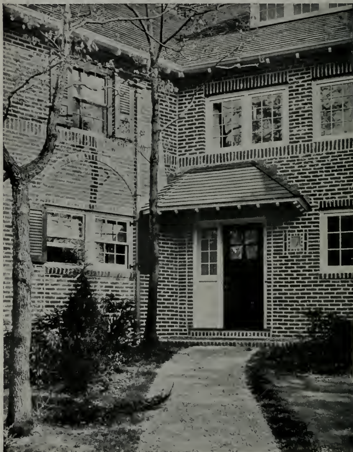
Detail of Residence, Newtonville, Mass., Frank Chouteau Brown, Architect
