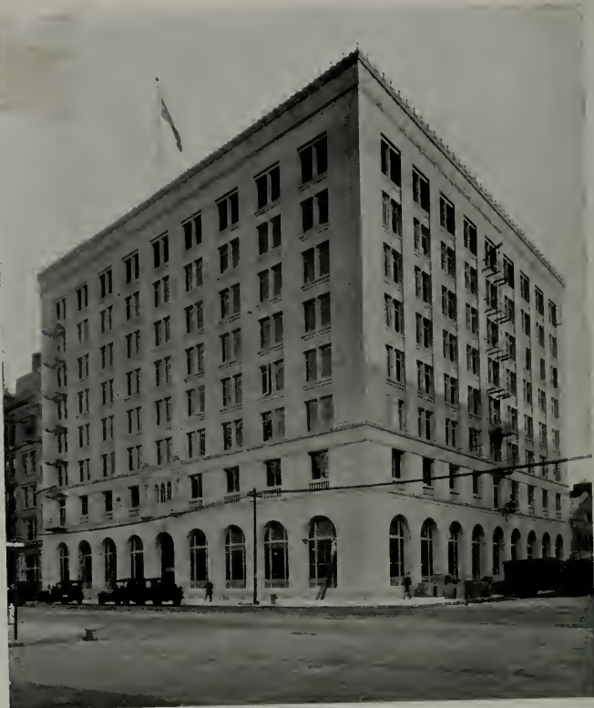
BUILDING FOR WALTON N. MOORE DRY GOODS COMPANY, SAN FRANCISCO Geo. W. Kelham, Architect Foundation Company, Builders
