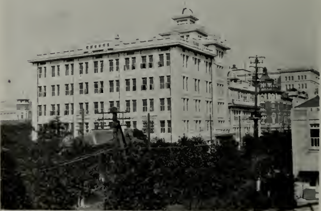
NICHI NICHI BUILDING, TOKYO, OF REINFORCED CONCRETE. UNDATED.
