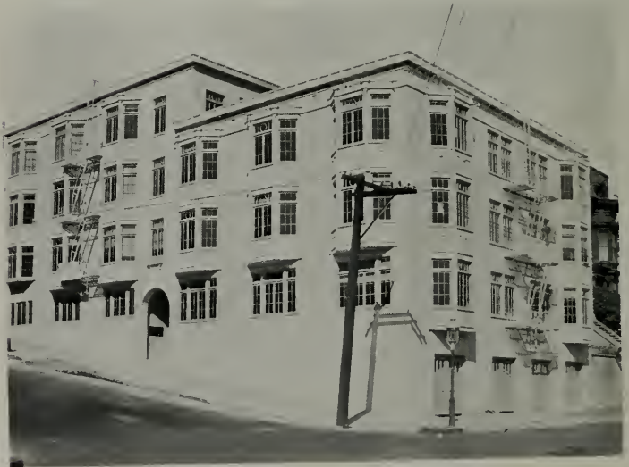
APARTMENTS FOR MR. DANIEL McKILLOP, SAN FRANCISCO Baumann and Jose, Architect and Engineer
