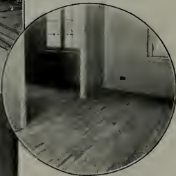
1/2" x 2" No. 1 Common oak flooring was laid over terrazzo in this modern 33 apartment building in St. Louis. Details on request.
