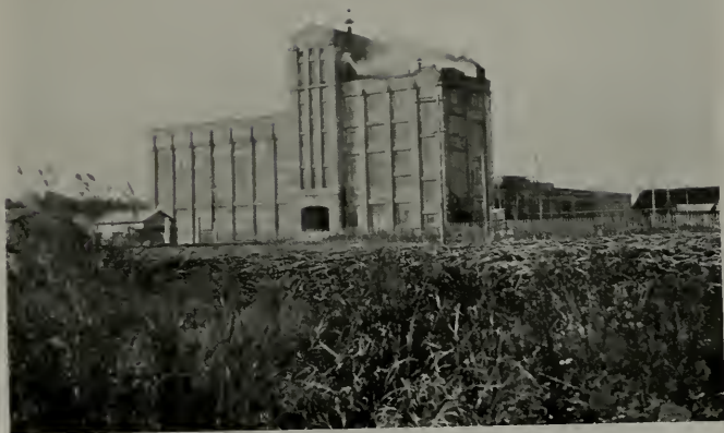
CASCADE BREWERY, TSURUMI, OF REINFORCED CONCRETE. UNDATED.
