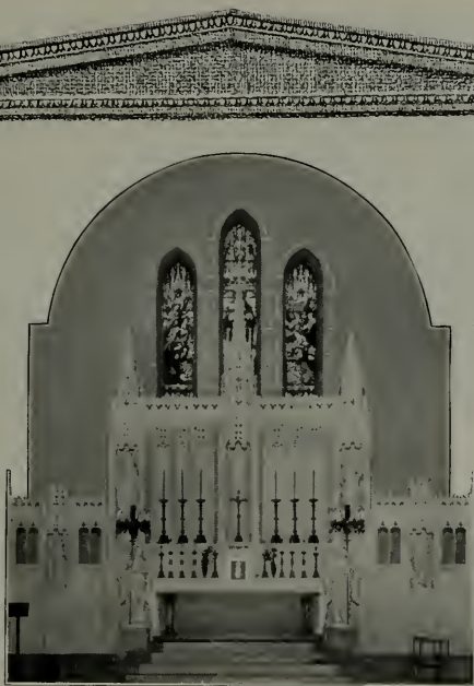
American Cream White Lens altar with Pink Tennessee Marble steps and base, in Holy Name Church, Philadelphia, Pa. Maginnis & Walsh, Architects. J. Hegerty, Marble Contractor.
