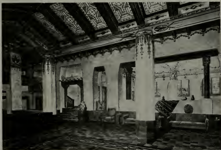
INTERIORS, HOTEL FRANCISCAN, ALBUQUERQUE TROST AND TROST, ARCHITECTS
