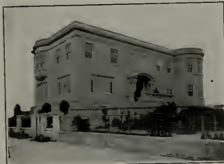
Residence, 21st and Fair Oaks Streets San Francisco Theo. Lenzen, Architect
