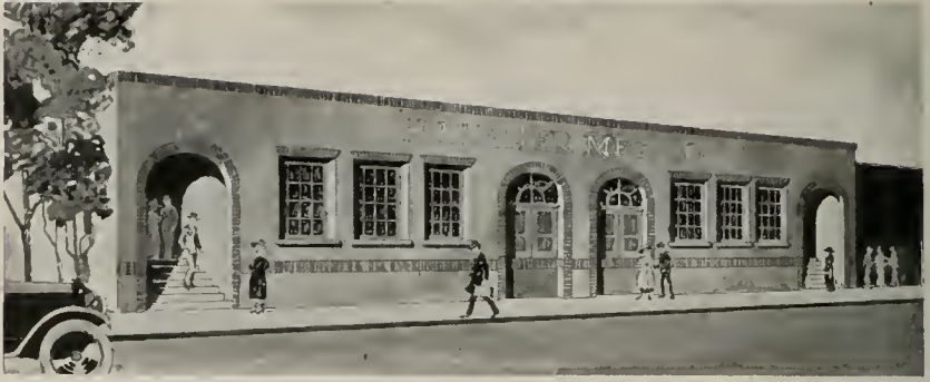
BUILDING FOR H. MUELLER MFG. CO., LOS ANGELES
