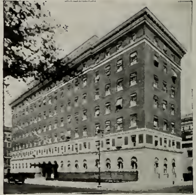
MT. SINAI HOSPITAL, NEW YORK Arnold W. Brunner, Architect
