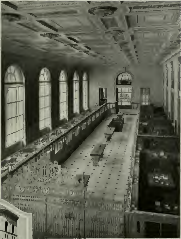
Main Banking Room—Bank of Italy, San Francisco Bliss and Faville, Architects
