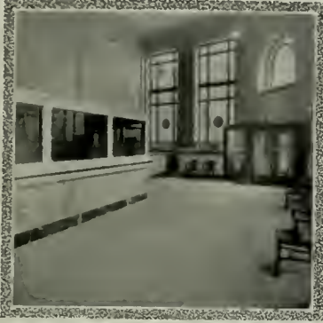
Cleveland Trust Branch Bank A. G. Hall, Architect Matched panels of Madre Veined Alabama on Imported Verde An- tique Base
