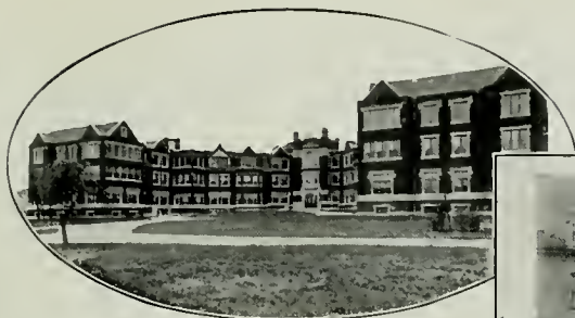
OAK FLOORS are today giving satisfactory service in the Presbyterian Home for the Aged, Evanston, Ill., shown at left, in the Nurses' Home, Robinwood Hospital, Toledo, Ohio, shown next below, and in the Masonic Memorial Hospital, Utica, N.Y.
