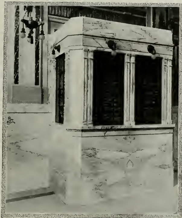
MATCHED PANELS OF MADRE VEINED ALABAMA KEITH'S THEATRE, CLEVELAND, O. C. L. and G. W. Rapp, Architects
