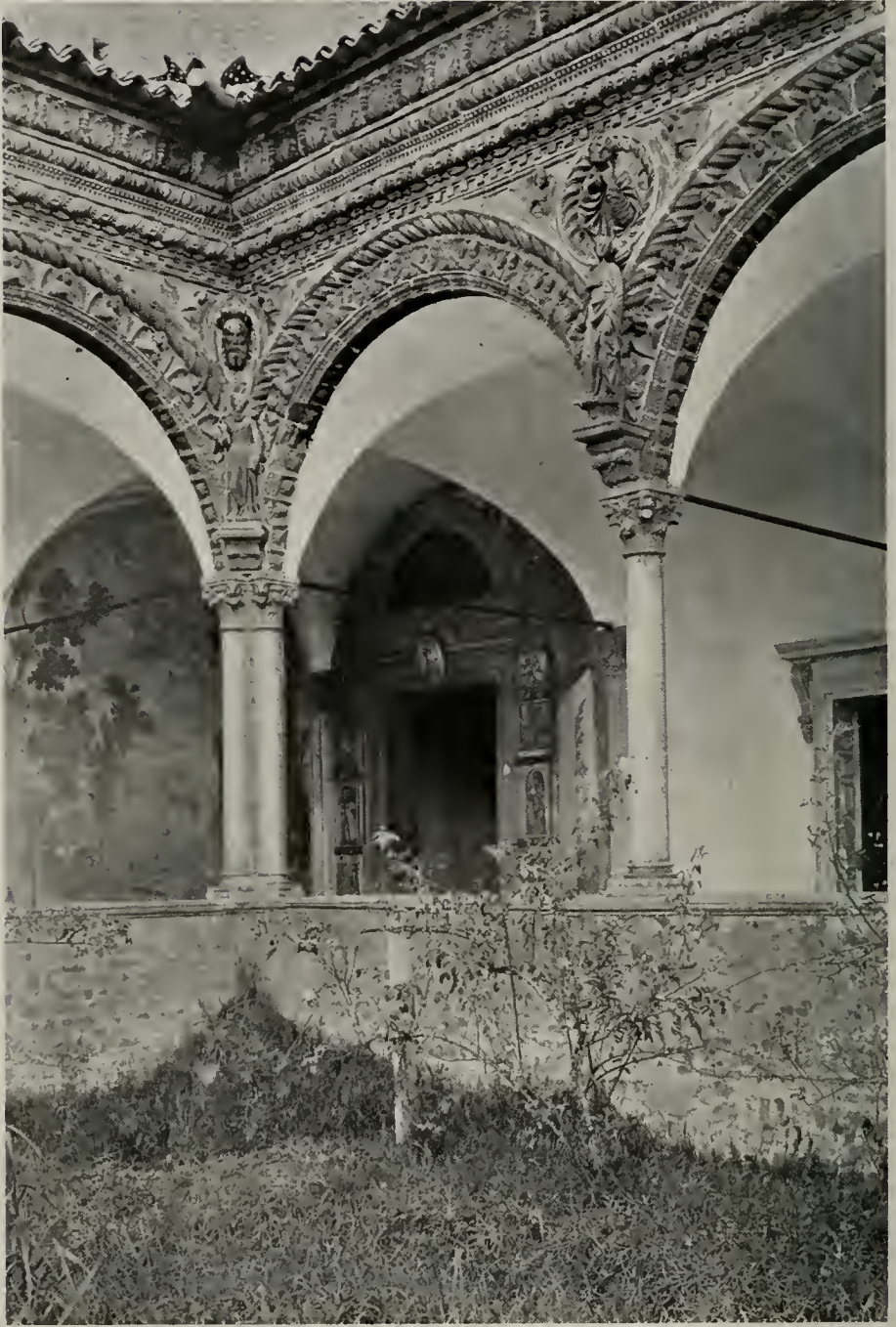
CORNER IN COURT OF MONASTERY, CERTOSA OF PAVIA, ITALY, (1523) COLOR RED, UNGLAZED; TYPICAL OF EARLY ITALIAN TERRA COTTA WORK
