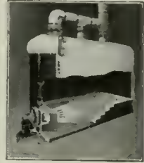
BURNER IN OPERATION
