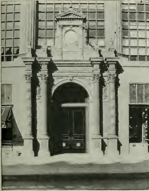
Main Entrance, Brownstein-Louis Company's Factory Building, Los Angeles, California, John Parkinson, Architect: Executed in dark standard buff Terra Cotta with white mottling. Columns above entrance also Terra Cotta.
