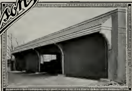
Garage at the Metropolitan Coal Co., Brookline, Mass.
