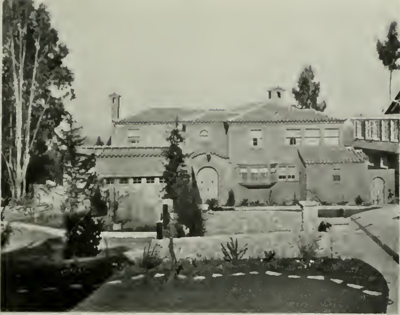
HOUSE OF MR. E. J. SCHNEIDER, CLAREMONT Albert Farr, Architect and J. F. Ward, Associate Horace George Cotton, Landscape Architect
