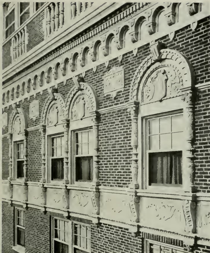
Detail of Terra Cotta, Upper Stories, Chase Hotel, St. Louis, Mo. Preston J. Bradshaw, Architect
