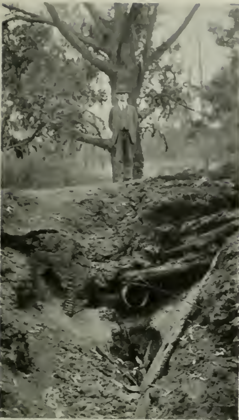
ARMCO CULVERT ON WILDCAT CANYON ROAD. UNDAUNED BY BERKELEY FIRE. SEPT. 1923. NOTE CONDITION OF WOODEN HEADWALL.
