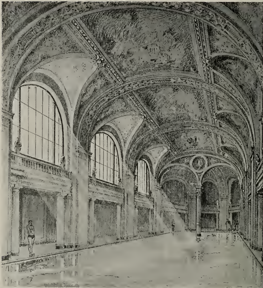
INTERIOR, ELKS CLUB BUILDING, SAN FRANCISCO F. H. Meyer & A. R. Johnson, Architects
