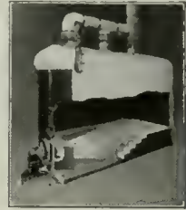
BURNER IN OPERATION
