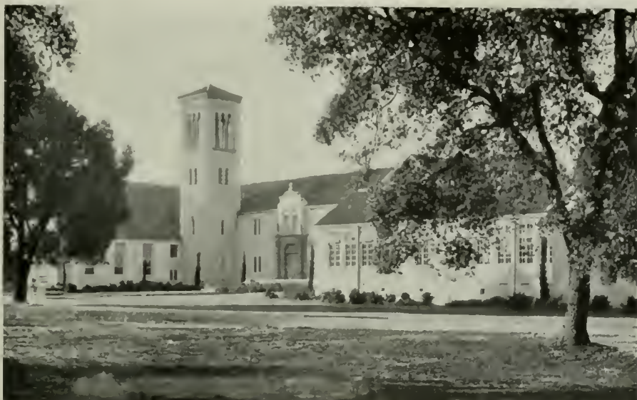
PALO ALTO UNION HIGH SCHOOL BUILDING
