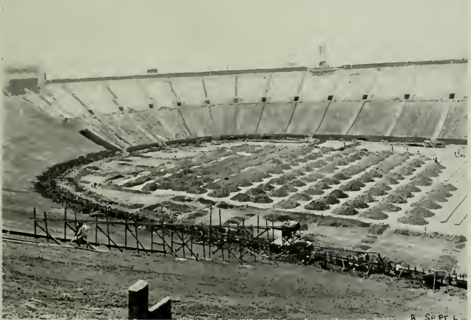
CALIFORNIA MEMORIAL STADIUM, BERKELEY Photo taken September 6th, 1923
