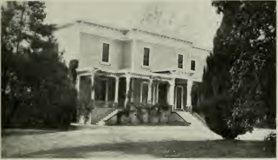
HOUSE OF MR. J. S. McCLYMONT, MENLO PARK, BEFORE ALTERATIONS
