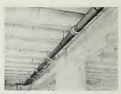
CORROSIRON DRAIN LINE IN PROCESS OF INSTALLATION, NEW OAKLAND TRIBUNE BUILDING E. T. Foulkes, Architect. Scott Co., Plumbers
