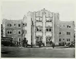
Showing Interlocking Tile Walls of Bennett Apartment House after fire Not a tile cracked—not even a crack in the stucco
