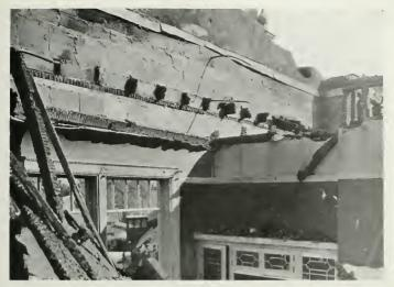
BENNETT APARTMENT HOUSE, STOCKTON Roof and partitions destroyed. Hollow tile walls intact
