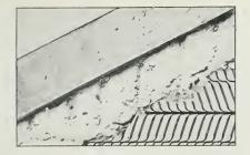
Herringbone Lath keys the plaster solidly and prevents cracks and falling
