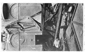
Truss T-12 up against the 18th St. wall. Note ventilating fan at left, which was carried down by collapse of the concrete roof.
