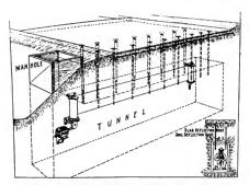
OBSERVATION TUNNEL BUILT UNDER TEST HIGHWAY
