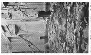
Showing truss T-12 against the 18th Street wall. Note terra cotta above ceiling line upon which truss rested.
