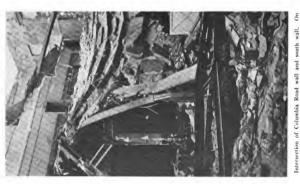
the left, column C2 and that part above the joint whether C4 column C2 and that part above the joint whether off. Here is an excellent presentation of what came down on the beeds of the spectators. The concrete roof is only three inches thick.
