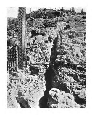
HETCH-HETCHY DAM CONSTRUCTION, SOUTH ABUTMENT AND CONCRETING PLANT AUGUST, 1921
