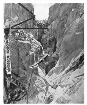
HETCH-HETCHY DAM CONSTRUCTION, SHOWING BOTTOM OF FOUNDATION
