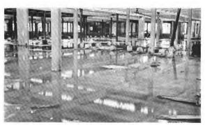
CONCRETE FACTORY FLOOR PROTECTED WHILE HARDENING BY "PONDING"
