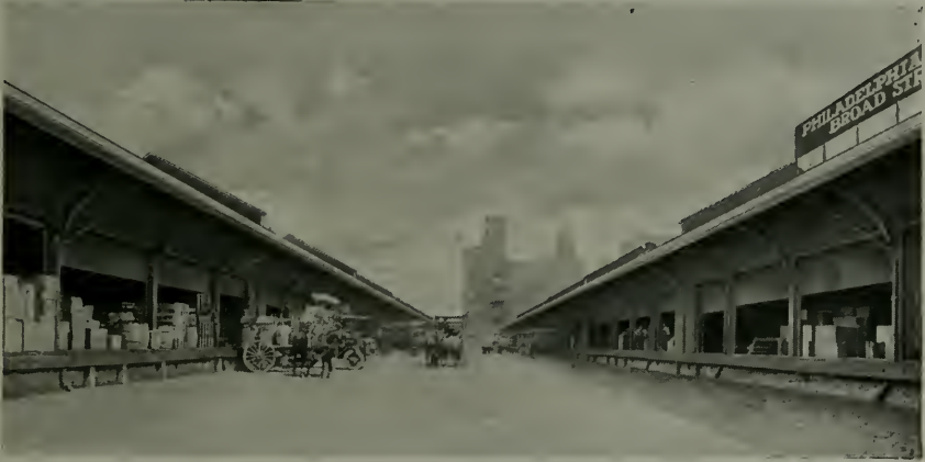
Wilson Rolling Steel Doors—Pennsylvania R. R. Freight Sheds, Philadelphia, Pa.
