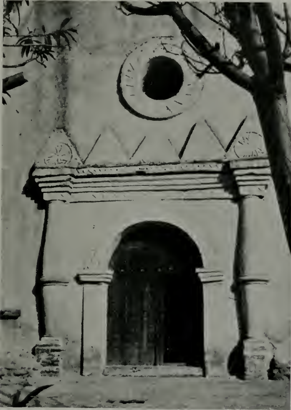
ENTRANCE DOORWAY, SAN IGNACIO DE CABURICA
