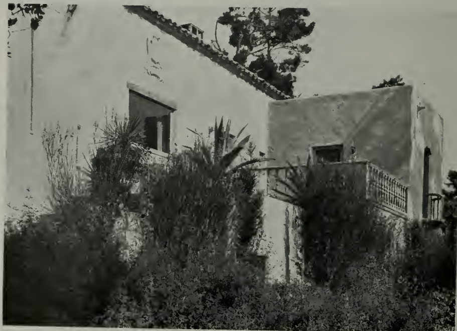
HOUSE FOR MR. GEORGE T. COOK, PEBBLE BEACH, CAL. Pierpont & Walter S. Davis, Architects
