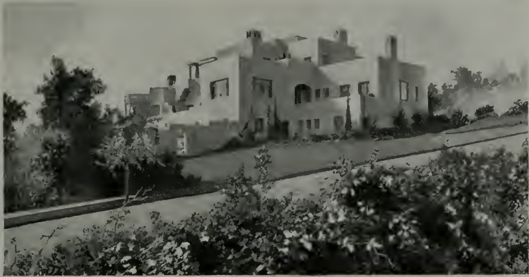
RESIDENCE OF HON. HERB. HOOVER, SECRETARY OF COMMERCE, STANFORD, CAL A. B. Clark, Architect Frederick W. Snook Co., Plumbing Contractors
