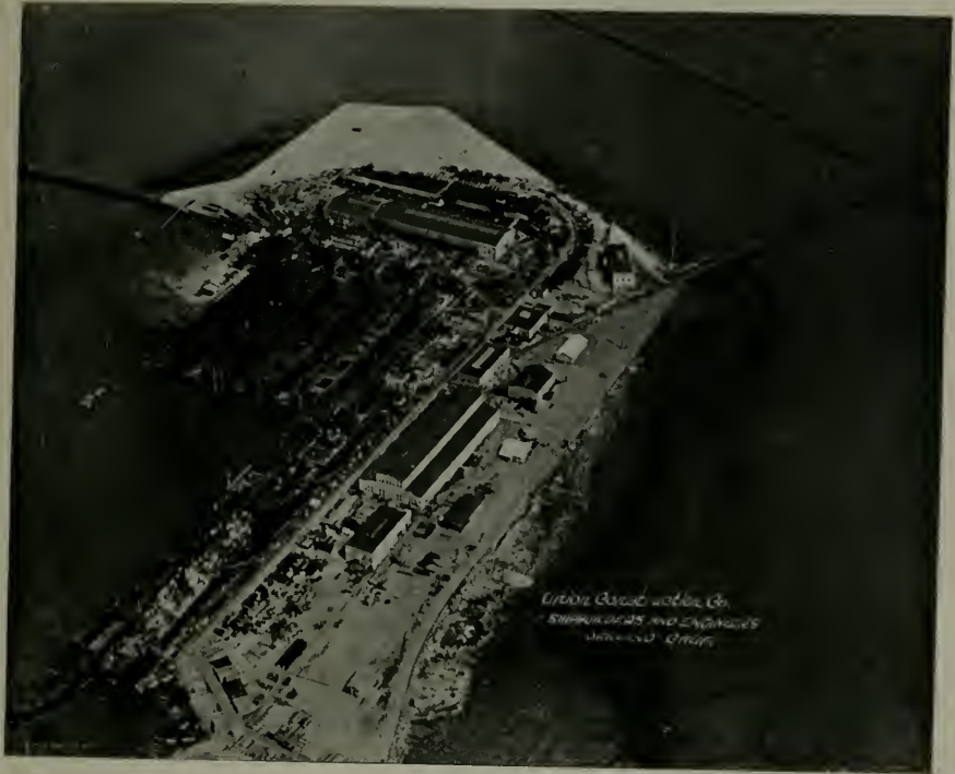
AIRPLANE VIEW, UNION CONSTRUCTION PLANT, OAKLAND
