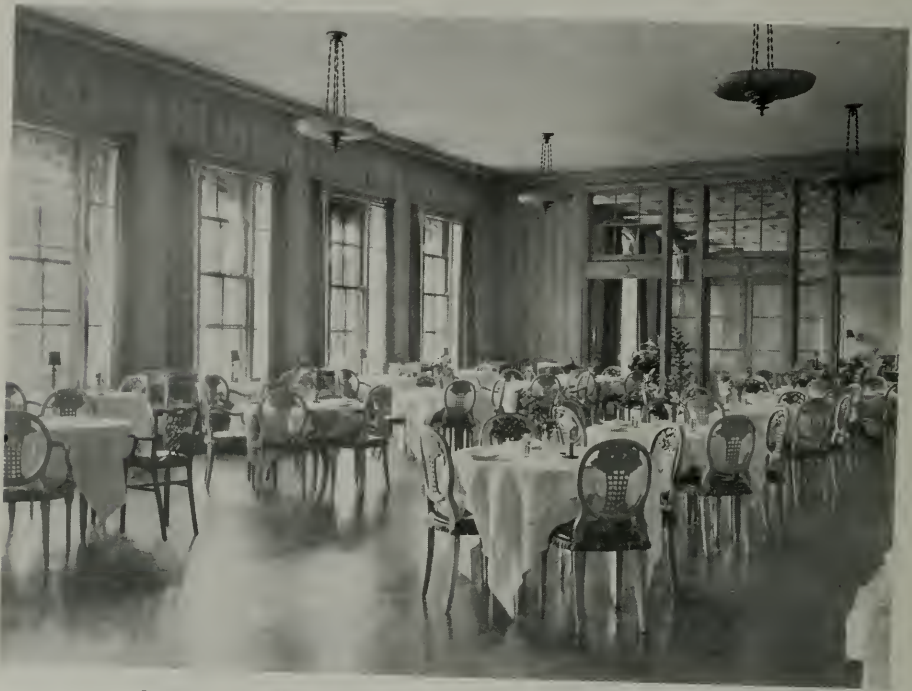
DINING ROOM, DEL MONTE LODGE, PEBBLE BEACH, CAL. Lewis P. Hobart, Architect
