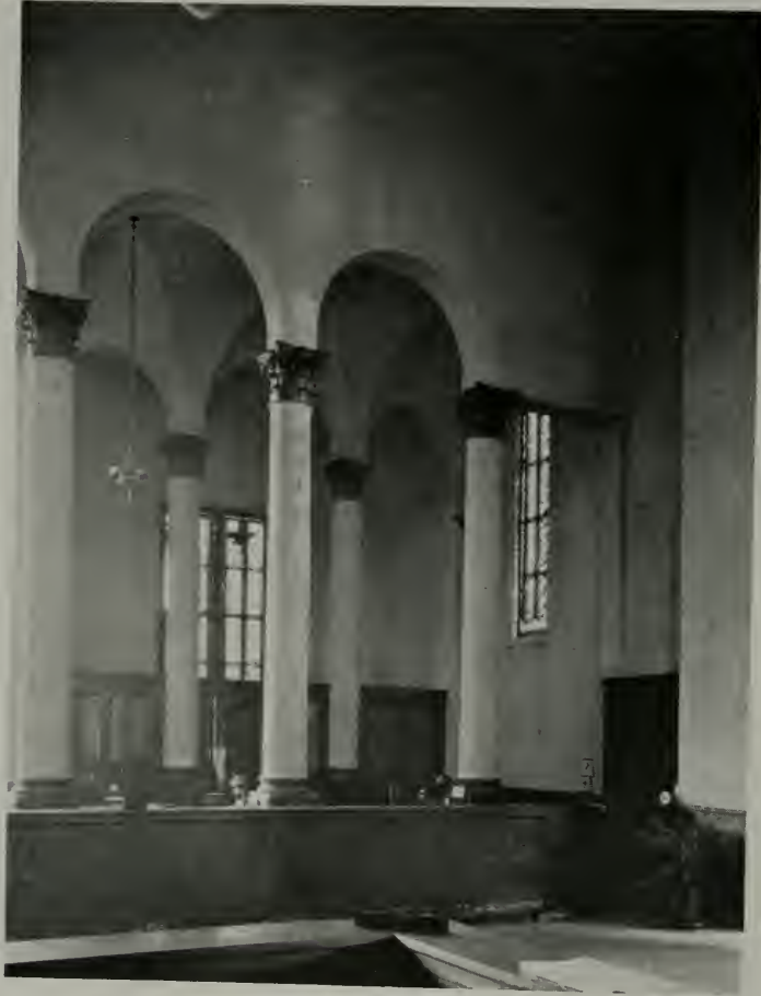
COUNTY NATIONAL BANK AND TRUST COMPANY, SANTA BARBARA, CAL. Myron Hunt, Architect
