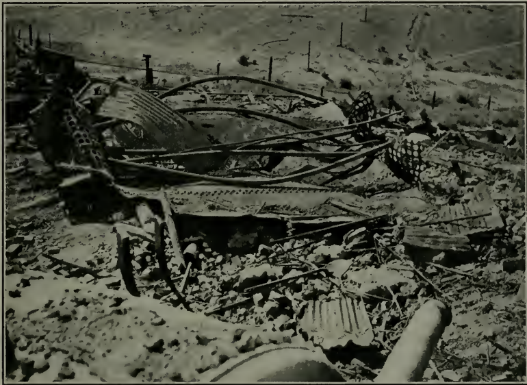
FIG. 2—VIEW OF THE EXPLODED BOILER
