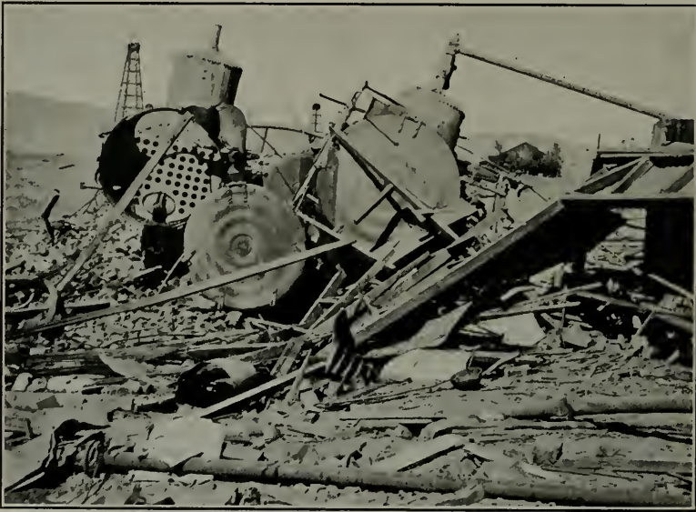
FIG. 1—VIEW OF NUMBER 2 AND NUMBER 3 BOILERS
