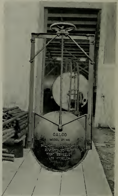
CAST IRON SLIDE GATE EMPLOYED IN RECLAMATION WORK, MT. EDEN
