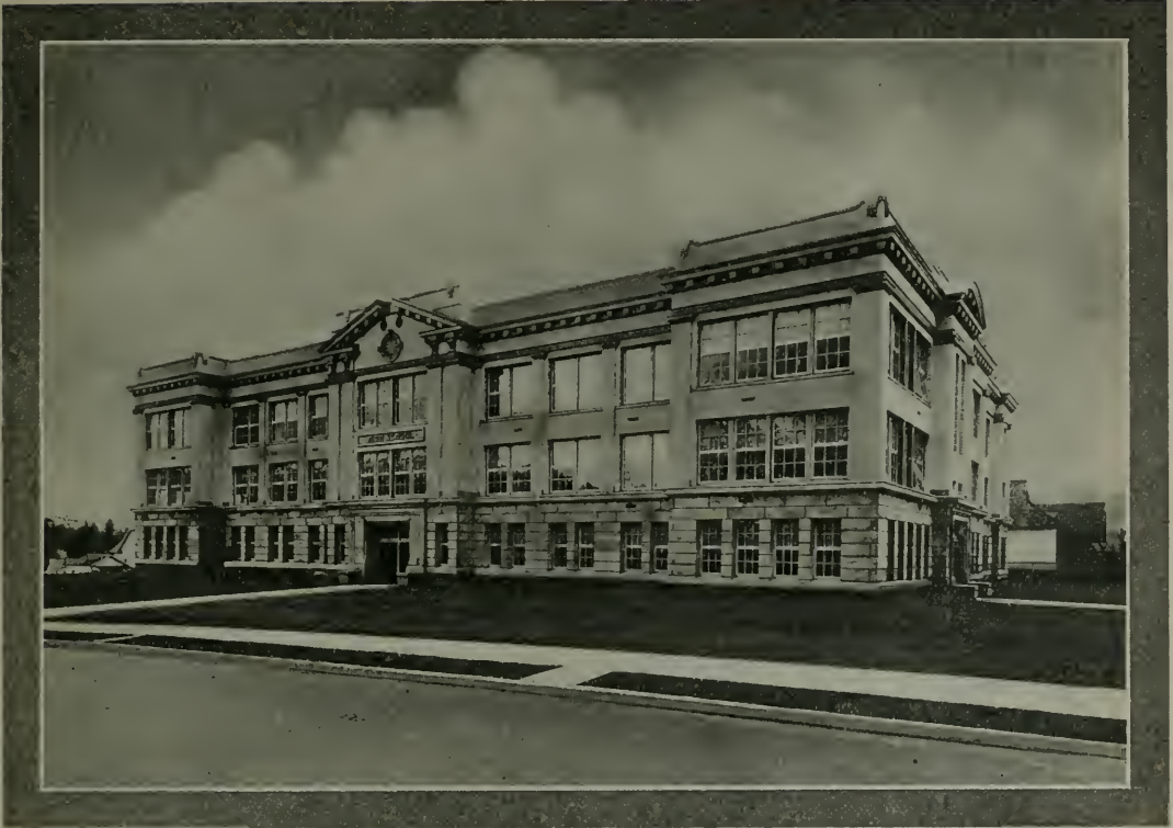
ROSEBURG, OREGON, HIGH SCHOOL. F. MANSON WHITE, Portland, Oregon, Architect
