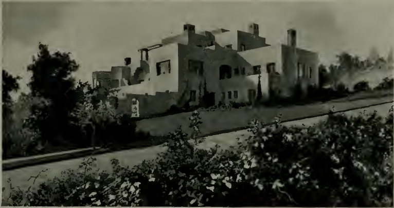
RESIDENCE OF HON. HERB. HOOVER, SECRETARY OF COMMERCE, STANFORD, CAL A. B. Clark, Architect Frederick W. Snook Co., Plumbing Contractors
