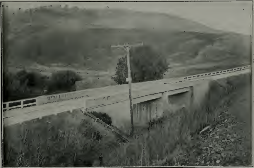
BRIDGES ON STATE HIGHWAY, SANTA BARBARA COUNTY, OVER CANADA DEL REFUGIO
