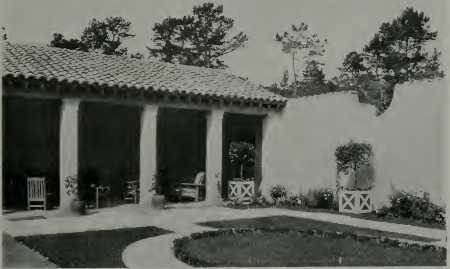
PATIO, HOUSE FOR MR. JOHN S. CRAVENS, PEBBLE BEACH, CAL. Lewis P. Hobart, Architect
