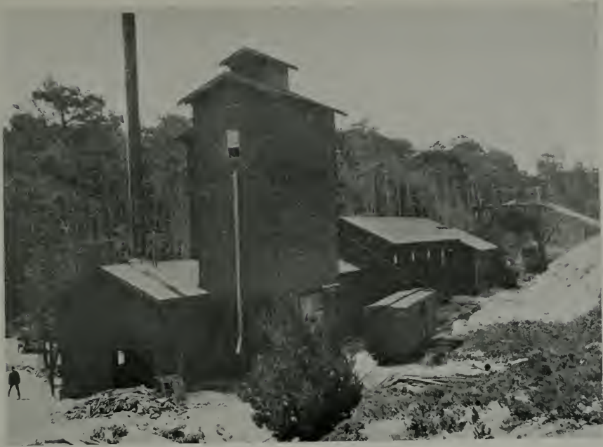
PLANT AT LAKE MAJELLA
