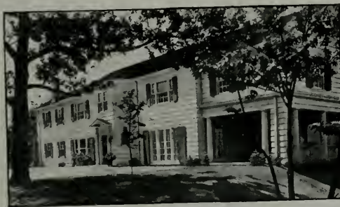
House at Cornwall-on-Hudson, N. Y. Finished with Old Virginia White. Rogers & Zogbaum, Architects, New York
