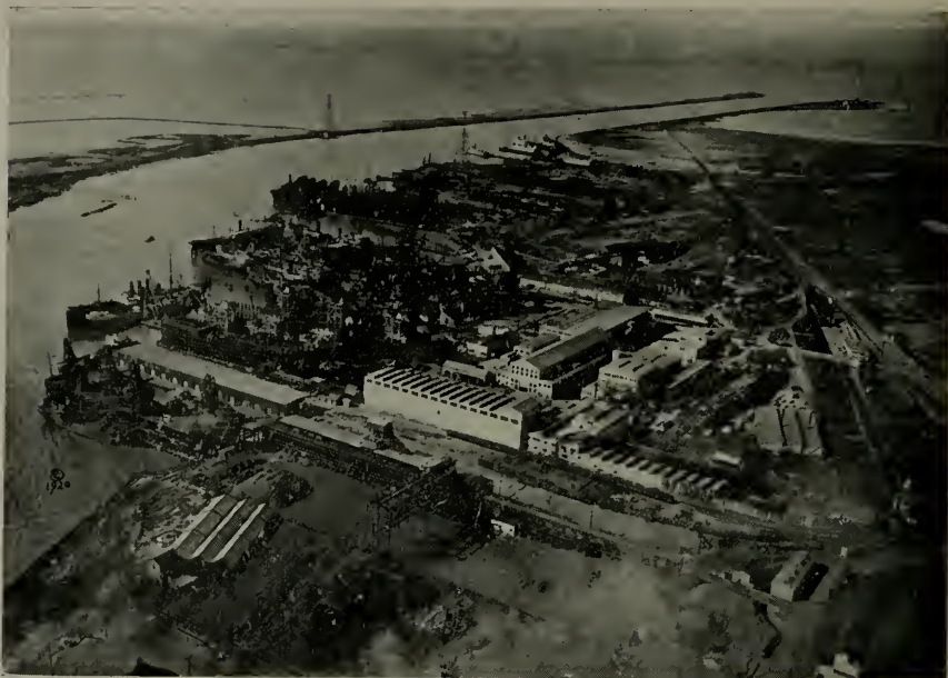
PLANT OF THE MOORE SHIPBUILDING COMPANY, OAKLAND
