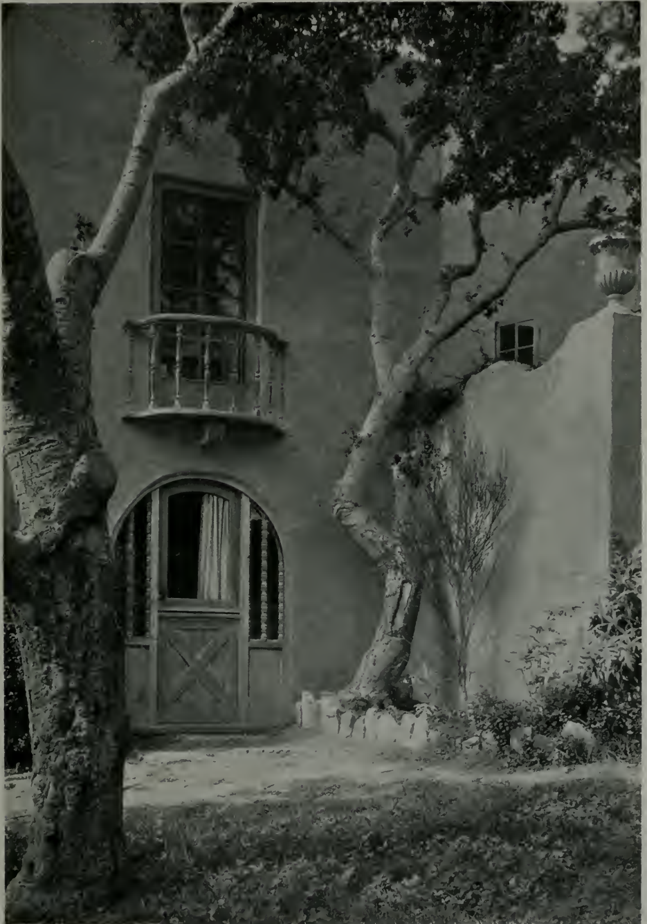
HOUSE FOR MR. GEORGE T. COOK, PEBBLE BEACH, CAL. PIERPONT & WALTER S. DAVIS, ARCHITECTS
