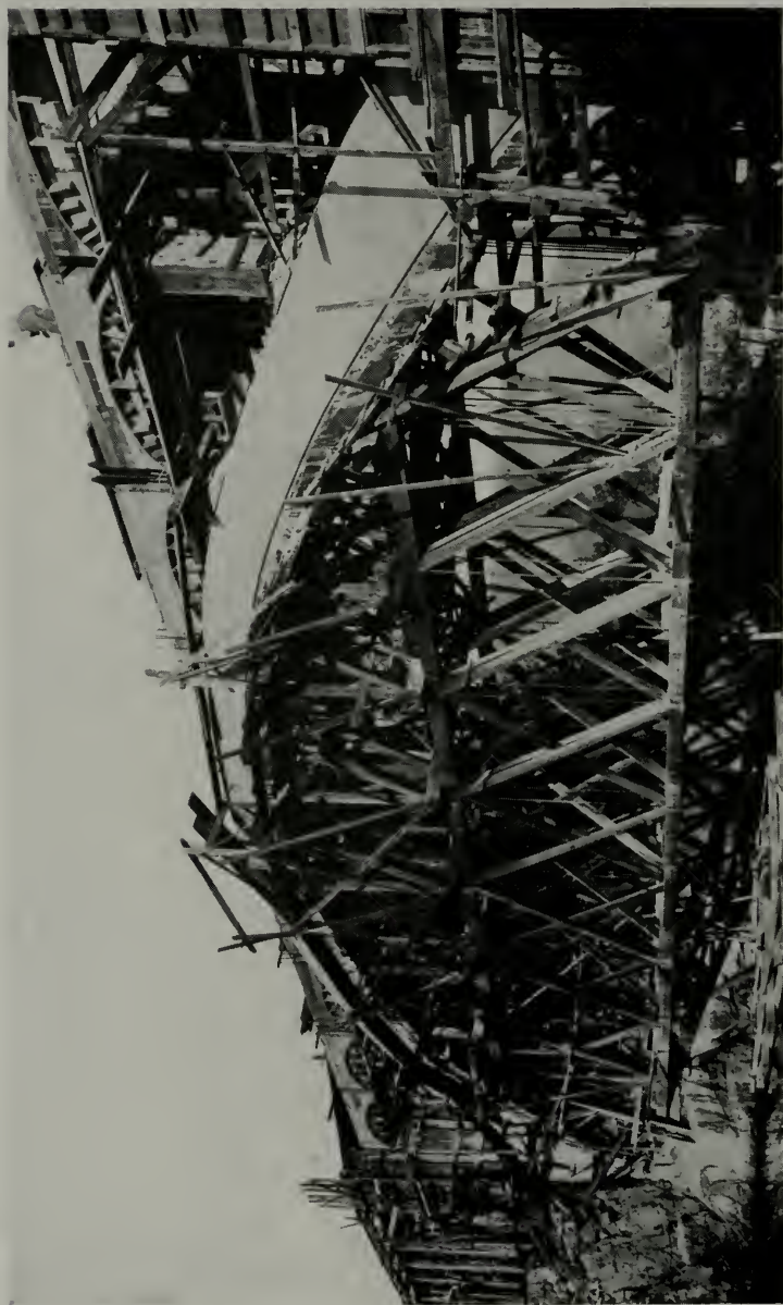
ROGUE RIVER BRIDGE, OREGON, SHOWING HOWE TRUSS SUPPORTING FRAMEWORK OF ARCH SPAN. HERBERT NUNN, HIGHWAY ENGINEER; C. B. McCULLOUGH, BRIDGE ENGINEER
