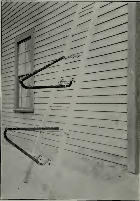
FIG. 1—CHICAGO AND LOS ANGELES LADDER BRACKETS
