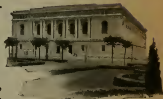
Carnegie Library San Francisco; all sheet metal and iron grills on windows are of Armco Ingot Iron. Geo. W. Kelham, Architect.
