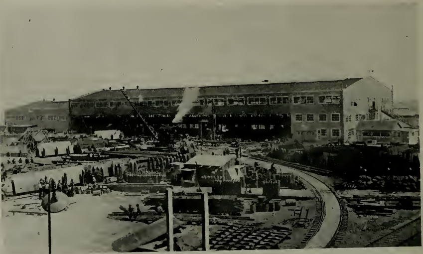
VIEW OF FABRICATING SHOP, UNION CONSTRUCTION COMPANY, OAKLAND
