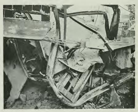
ARROW POINTS TO BREAK IN BOTTOM CHORD OF TRUSS D, REFERRED TO IN TEXT
