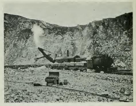
PIEDRA ROCK COMPANY'S PLANT Close-up of quarry face, showing No. 70 Bucyrus steam shovel loading train enronte to crusher.
