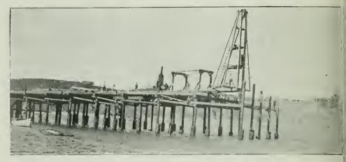
Fig. 1—This photograph shows the use of Armco ingot iron corrugated pipes to protect a wharf, recently built at Port Orford, Curry County, Oregon, from the ravages of the teredo.
