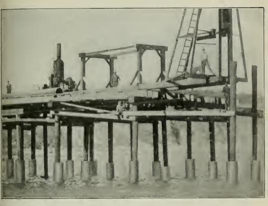
Fig. 3—A close-up view of the wharf recently constructed by the port of Port Orford, Curry County, Oregon, showing how ingot iron corrugated pipes were installed to prevent attacks by marine woodberers.
