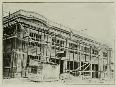
FLIMSILY CONSTRUCTED SCAFFOLD WITHOUT RAILINGS OR TOEBOARDS.
