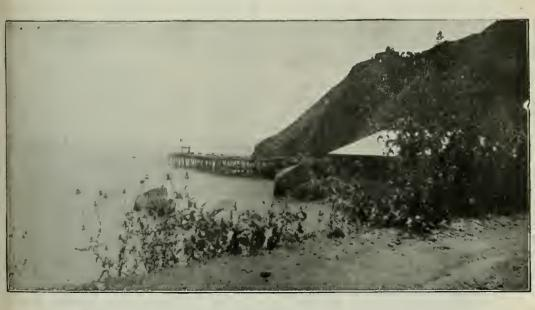
Fig. 4—Wharf recently erected at Port Orford. The piles are protected from marine borers by corrugated iron pipes.
