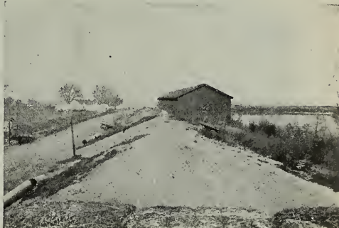
Reclamation District Camp, Sacramento River, and Armco Pipe
