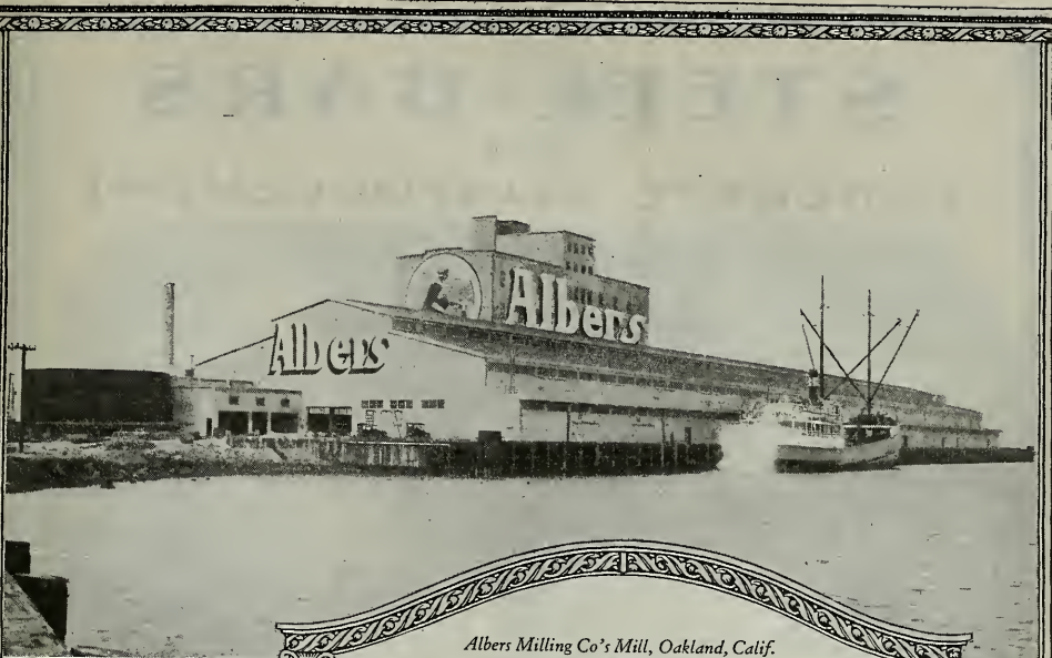
Albers Milling Co's Mill, Oakland, Calif. Covered with a PABCO 10 Year Roof.
