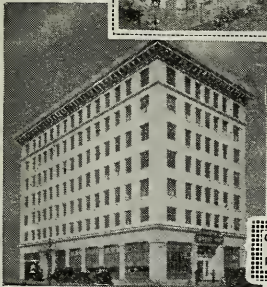
CITIZENS SAVINGS BLDG. PASADENA, CAL.
