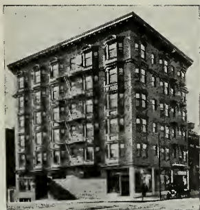
Crescent Apartments, Ellis and Hyde Streets, San Francisco Equipped with WALL BEDS
