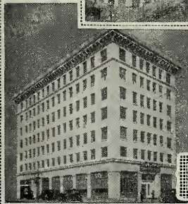
CITIZENS SAVINGS BLDG. PASADENA, CAL.
