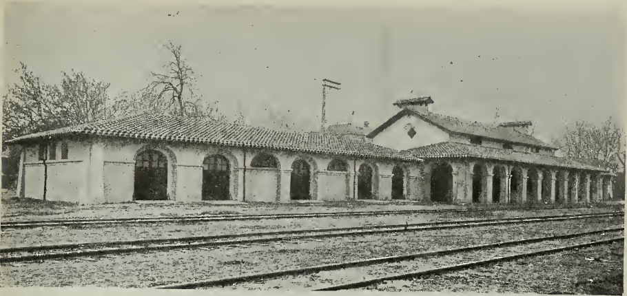
WESTERN PACIFIC DEPOT, SACRAMENTO Willis Polk & Company, Architects
