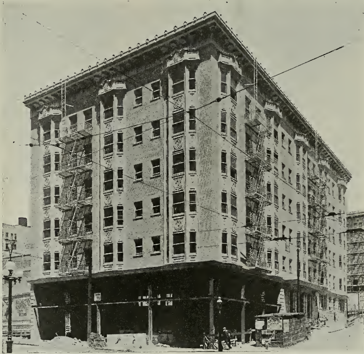
Apartment House Taylor and Geary Streets San Francisco For Mr. I. Rosenberg MR. JOSEPH CAHEN, Architect
