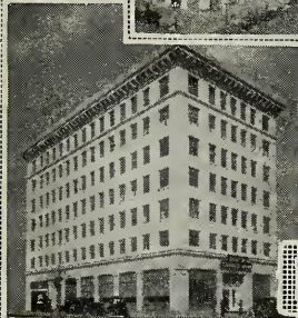
CITIZENS SAVINGS BLDG. PASADENA, CAL.
