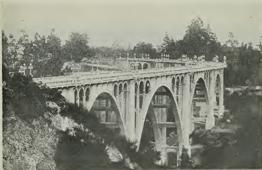
ARROYO SECO BRIDGE, PASADENA Harrington, Howard and Ash, Engineers
