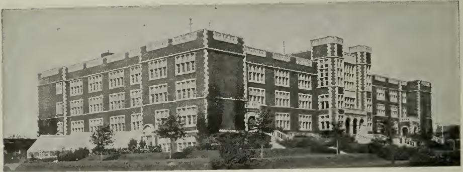
CENTRAL HIGH SCHOOL, MINNEAPOLIS, MINN.
