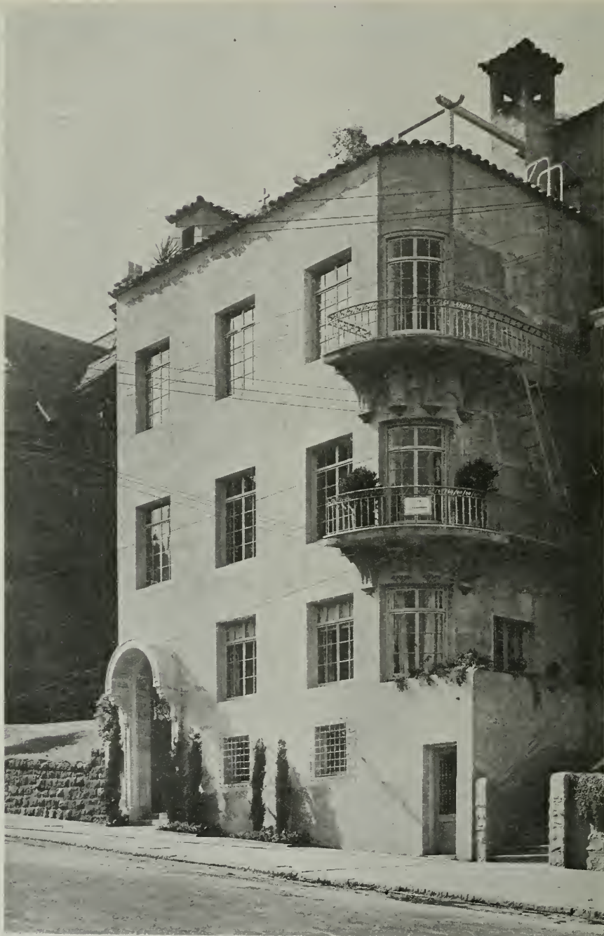
APARTMENTS FOR MR. NATHAN L. BELL. SAN FRANCISCO. J. F. DUNN, ARCHITECT
