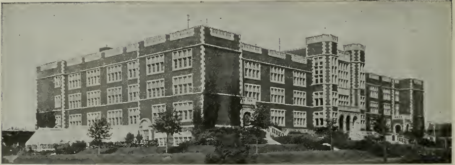
CENTRAL HIGH SCHOOL, MINNEAPOLIS, MINN.
