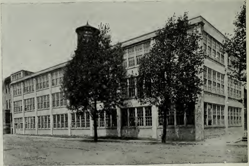
MILL OF THE NIAGARA SILK CO., NORTH TONAWANDA, N. Y. G. Morton Wolf, Architect
