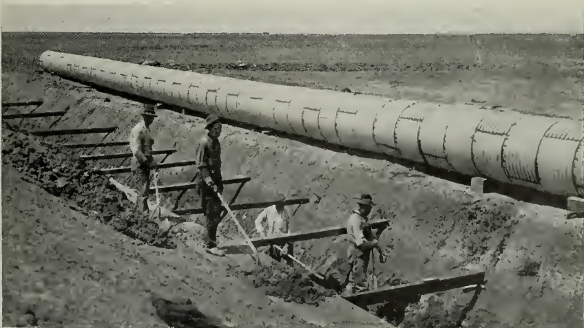
FORTY-EIGHT INCH ARMCO PIPE BEING INSTALLED IN IRRIGATION DITCH, RECLAMATION DISTRICT NO. 1500
