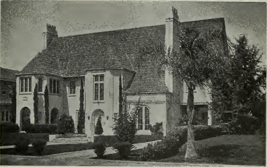
RESIDENCE OF W. H. GLOVER, 327 SOUTH NORMANDIE STREET De Remer & Hewitt, Architects
