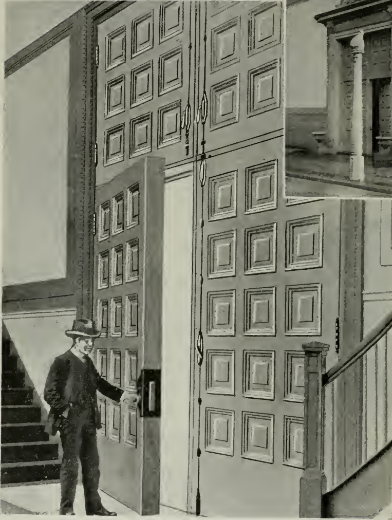
DOOR HUNG ON STANLEY BALL BEARING BUTTS IN THE PACIFIC GAS AND ELECTRIC COMPANY'S BUILDING, SAN FRANCISCO
