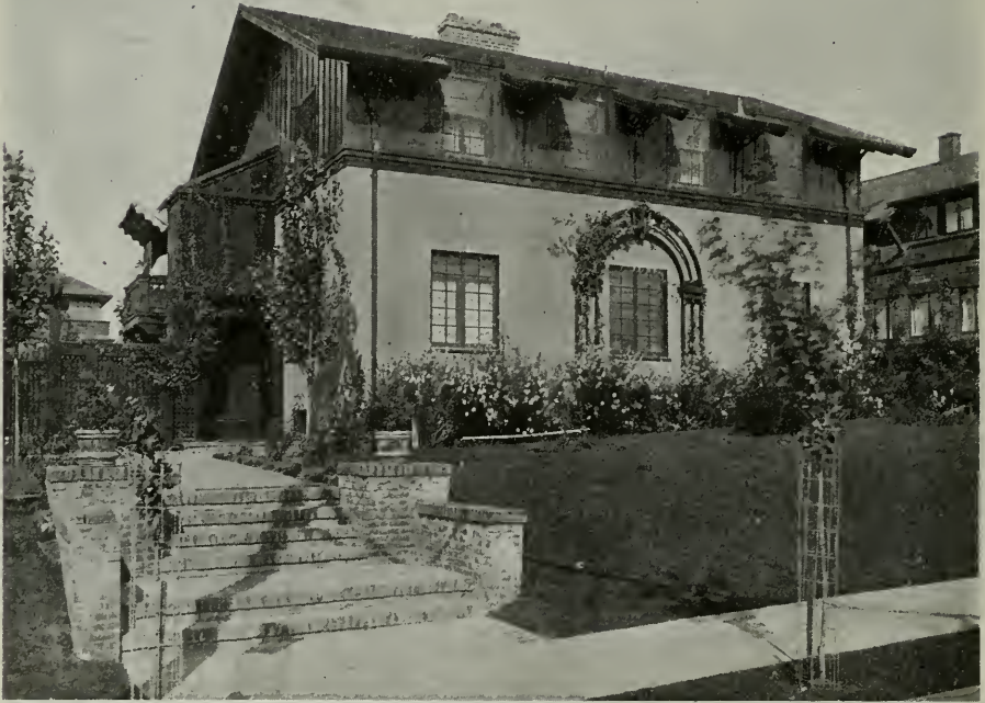
HOUSE FOR MR. A. H. MARKWART, OAKLAND, CALIFORNIA Wm. C. Hays, Architect
