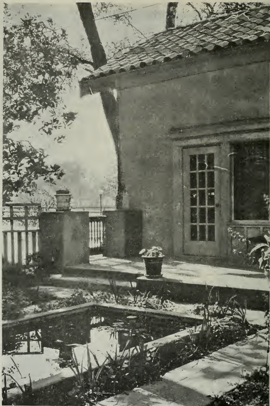
HOUSE OF MR. EDWIN J. SYMMES, ALAMEDA, CALIFORNIA EDWIN J. SYMMES, ARCHITECT
