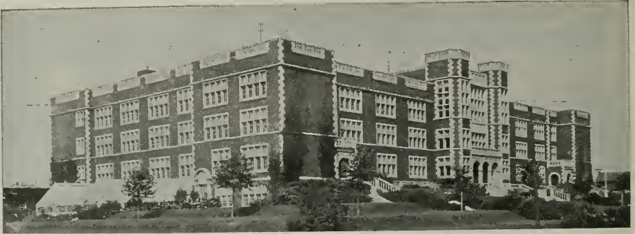
CENTRAL HIGH SCHOOL, MINNEAPOLIS, MINN.
