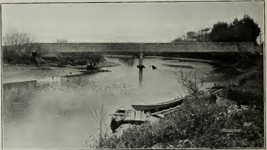
VIEW OF HIGHWAY BRIDGE OVER SALT RIVER, HUMBOLDT COUNTY, CALIFORNIA H. J. Brunnier, Engineer
