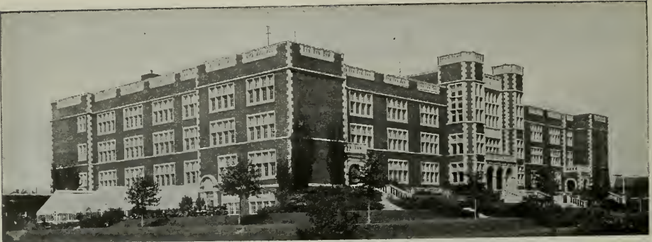
CENTRAL HIGH SCHOOL, MINNEAPOLIS, MINN.
