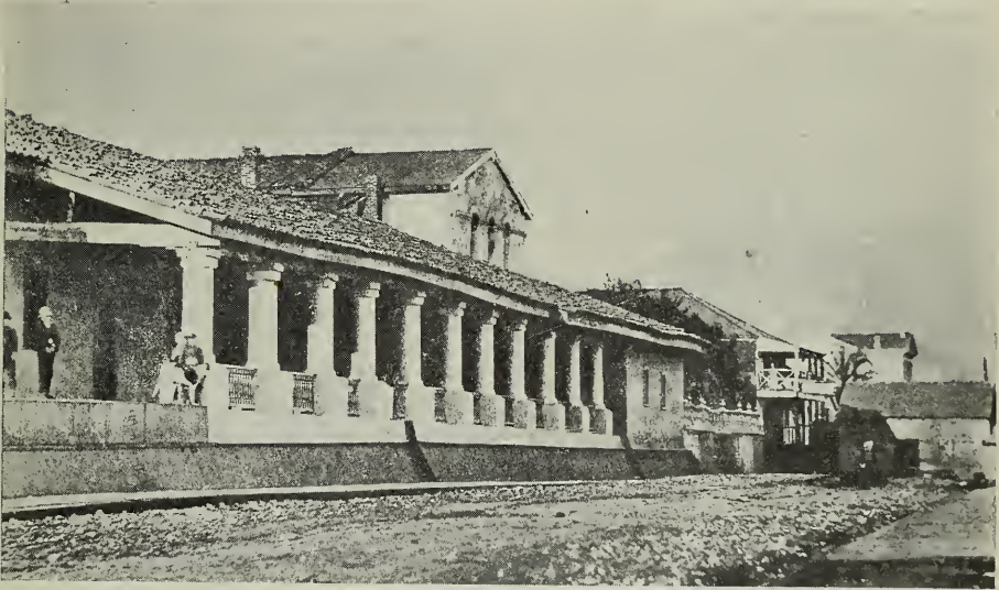
SAN LUIS OBISPO MISSION—AFTER GRADING OF STREET, RECONSTRUCTION OF WALL TO CHURCH FORECOURT, AND REMOVAL OF TILES FROM BELFRY
