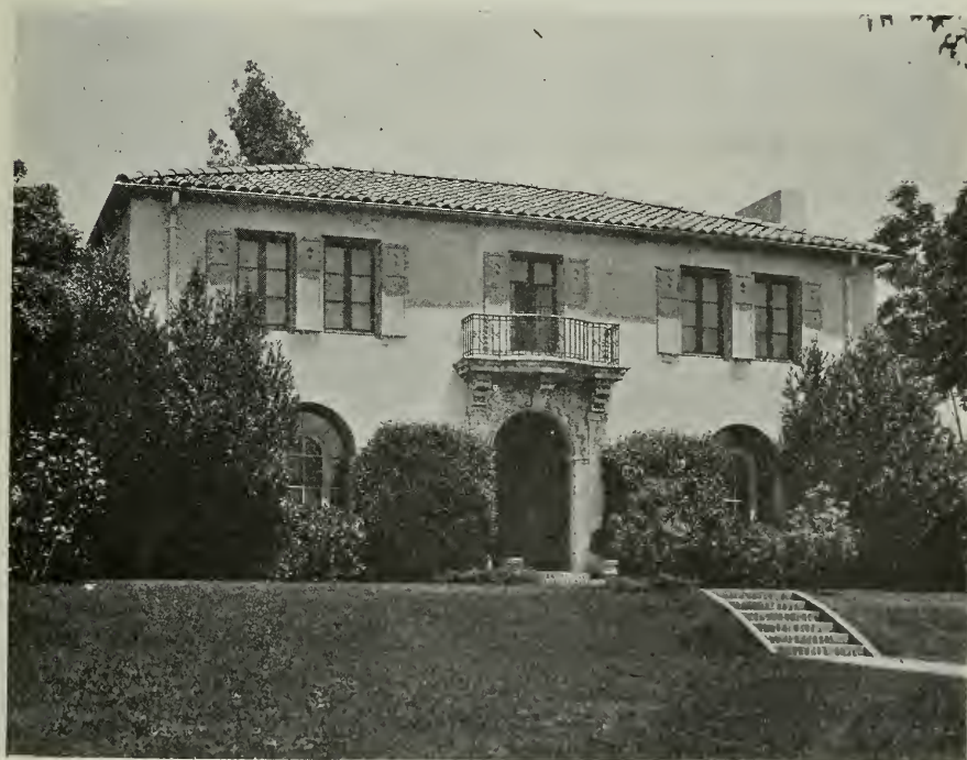
RESIDENCE OF BRIGGS C. KECK, OAK KNOLL, PASADENA Reginald D. Johnson, Architect
