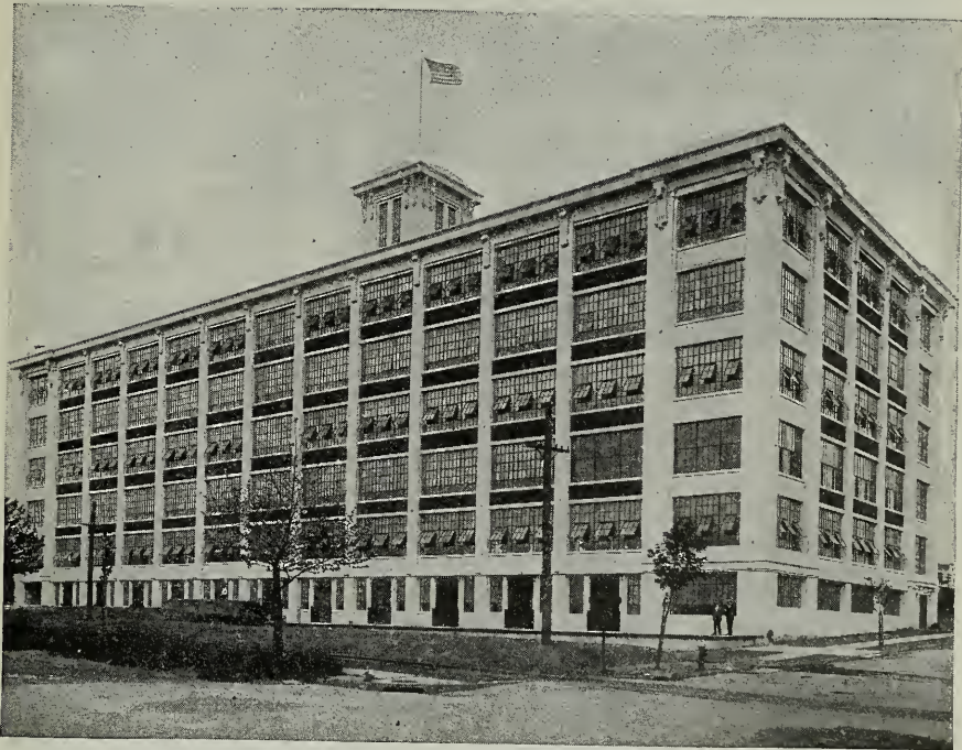
CONCRETE FACTORY, ALUMINUM GOODS CO., NEWARK, N. J. Lockwood, Green & Co., Engineers
