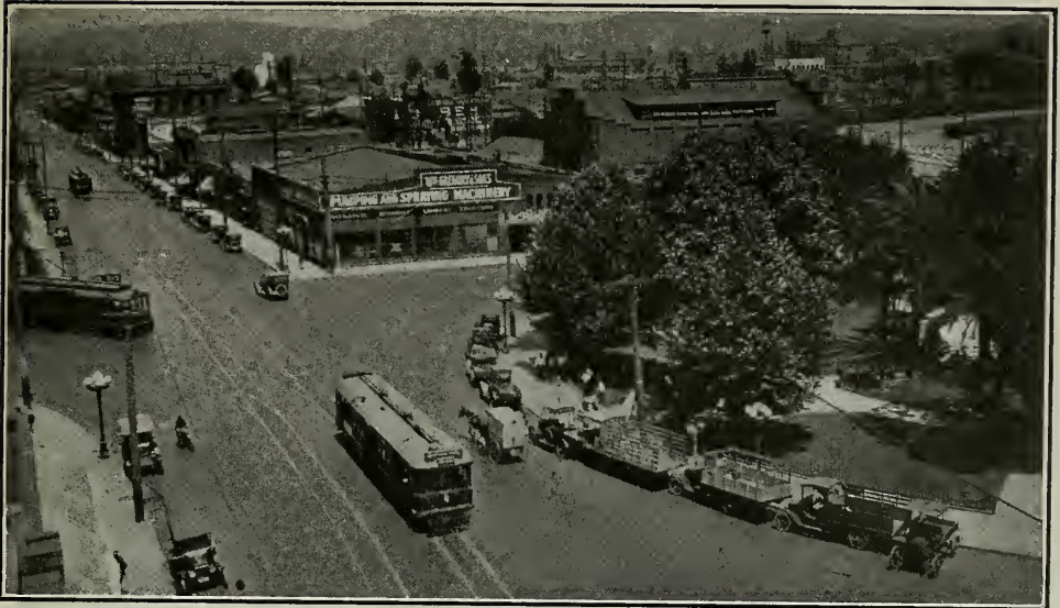
MAIN STREET, LOOKING NORTH FROM THE PLAZA, LOS ANGELES All buildings in the immediate foreground lie within the proposed station zone.
