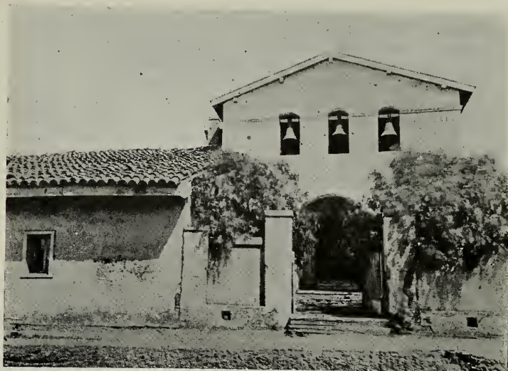
SAN LUIS OBISPO MISSION—ORIGINAL ENTRANCE AND FACADE TO CHURCH, AFTER REMOVAL OF ROOF TILES OVER BELFRY
