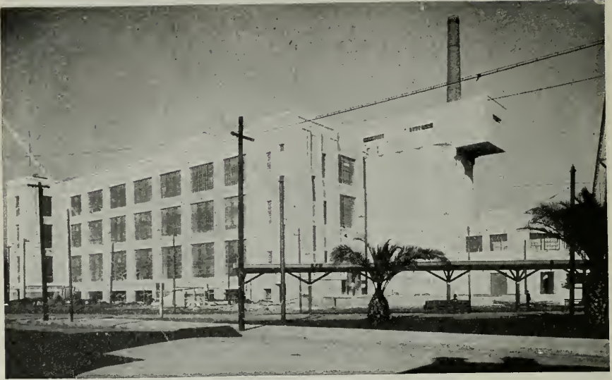
PACIFIC COAST SHREDDED WHEAT CO., OAKLAND Lewis P. Hobart and C. H. Cheney, Architects H. J. Brunner, Engineer
