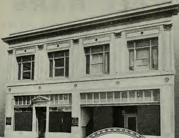
The First National Bank of Fairfield, California covered with a PABCO 20-Year Roof.
