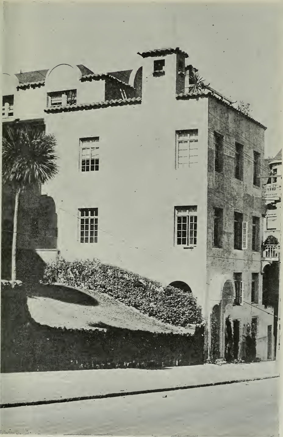
APARTMENTS FOR MR. NATHAN L. BELL, SAN FRANCISCO. J. F. DUNN, ARCHITECT
