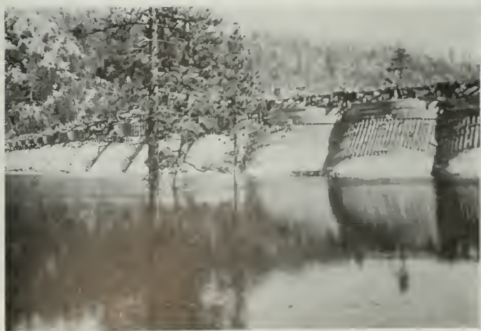
ELEANOR DAM LOOKING DOWN STREAM.
