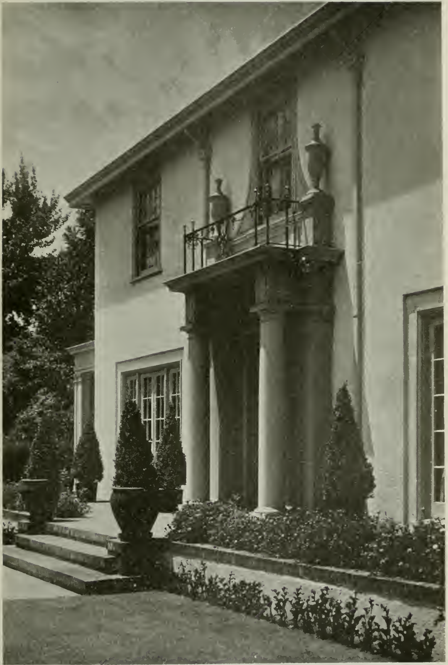
HOUSE OF MRS. HUGHES AND MRS. KENNEDY, PALO ALTO, CALIFORNIA JOHN K. BRANNER, ARCHITECT
