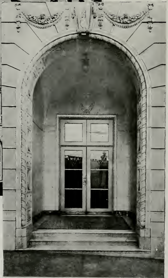
DETAIL OF ENTRANCE, Y. W. C. A. BUILDING, SAN FRANCISCO
