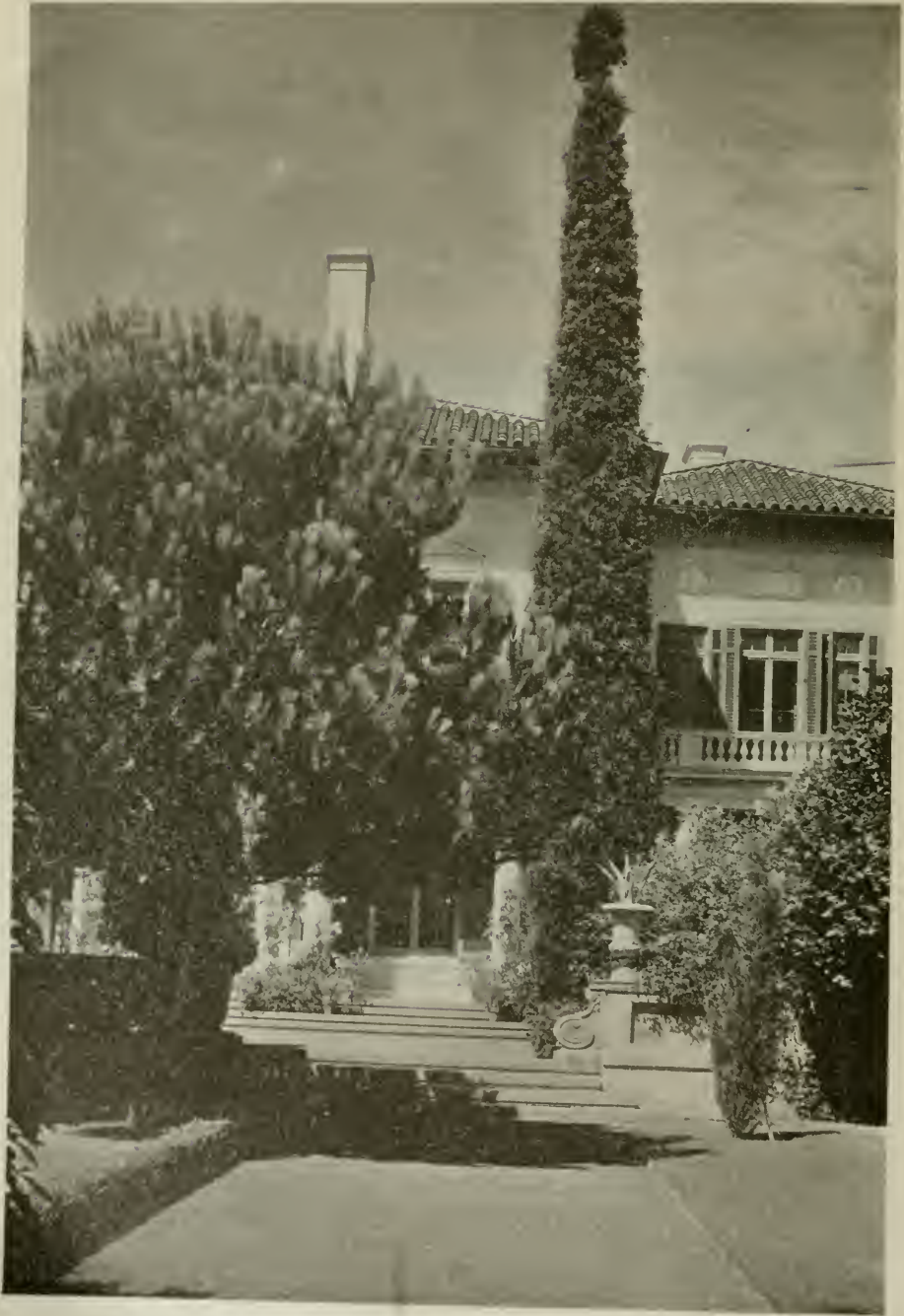
HOUSE OF MR. WM. H. CROCKER, BURLINGAME, CALIFORNIA LEWIS P. HOBART, ARCHITECT
