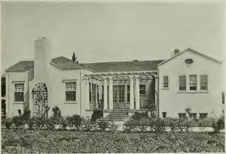
HOUSE OF MISS EMMA CHURCH, PALO ALTO, CALIFORNIA Charles K. Sumner, Architect
