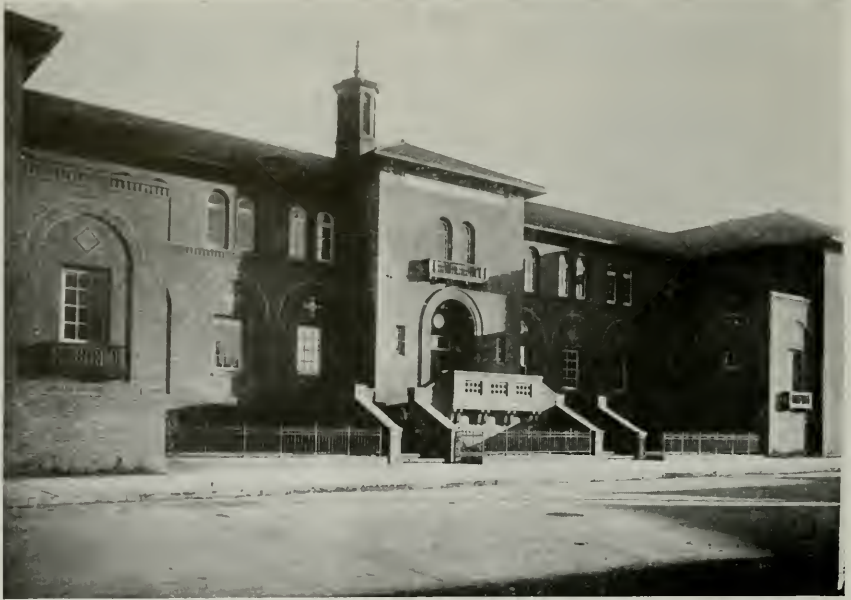
[ Monroe School Building—John Reid, Jr., Architect, San Francisco
