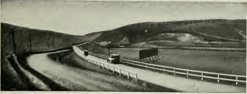
Stretch of concrete highway on the Lincoln Way, Altamont Pass, Alameda county, California.
