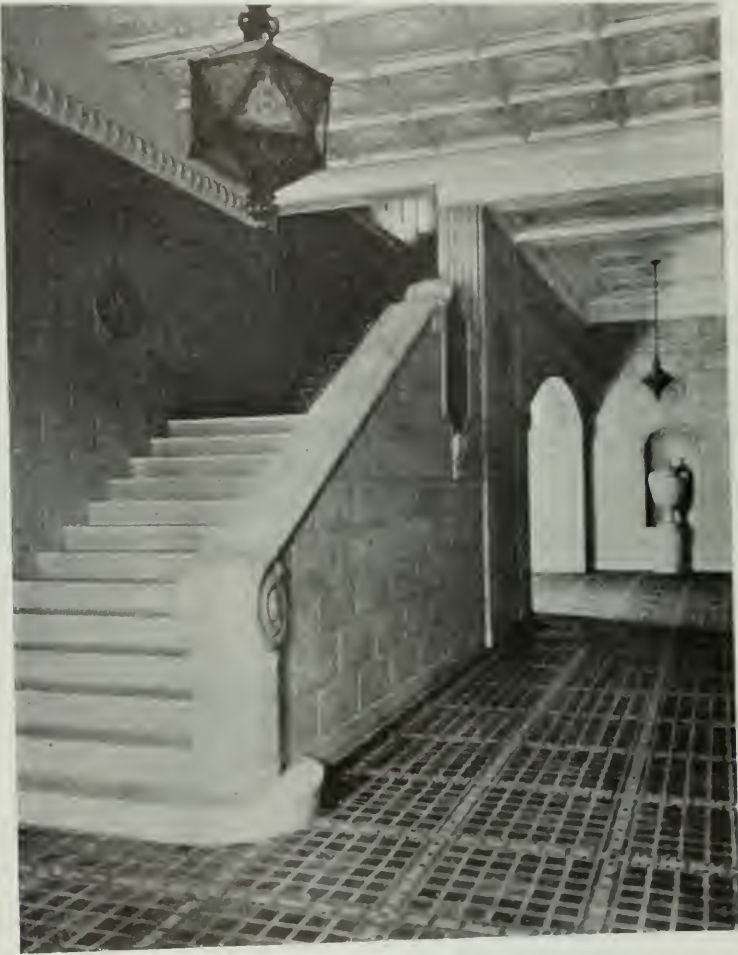
LOBBY, MASONIC TEMPLE, SACRAMENTO R. A. Herold, Architect
