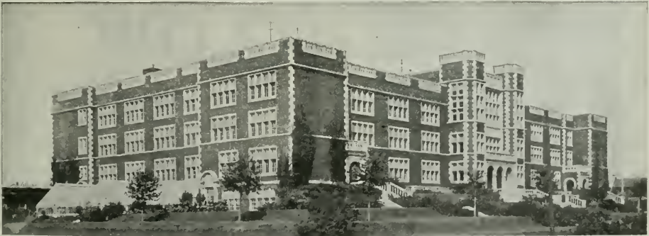
CENTRAL HIGH SCHOOL, MINNEAPOLIS, MINN.
