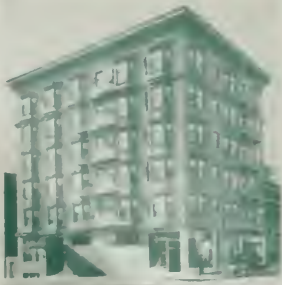
Crescent Apartments, Ellis and Hyde Streets, San Francisco Equipped with WALL BEDS
