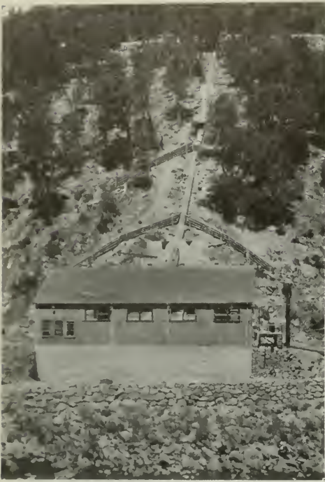
Power House at Early Intake from Across River
