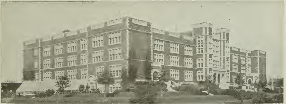
CENTRAL HIGH SCHOOL, MINNEAPOLIS, MINN.
