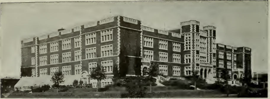
CENTRAL HIGH SCHOOL, MINNEAPOLIS, MINN.
