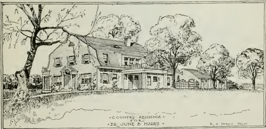
COUNTRY HOUSE FOR DR. JUNE B. HARRIS, NEAR SACRAMENTO R. A. Herold, Architect
