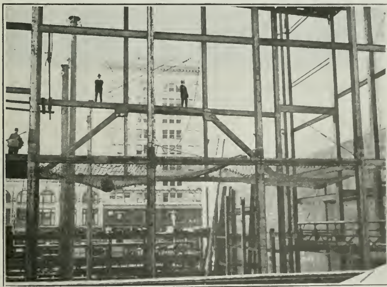
SAFETY NETS TO CATCH FALLING WORKMEN
