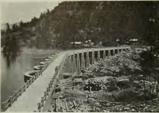
ELEANOR DAM. HETCH HETCHY WATER SUPPLY PROJECT.
