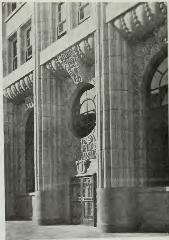
ENTRANCE, CAPITAL NATIONAL BANK, SACRAMENTO R. A. Herold, Architect
