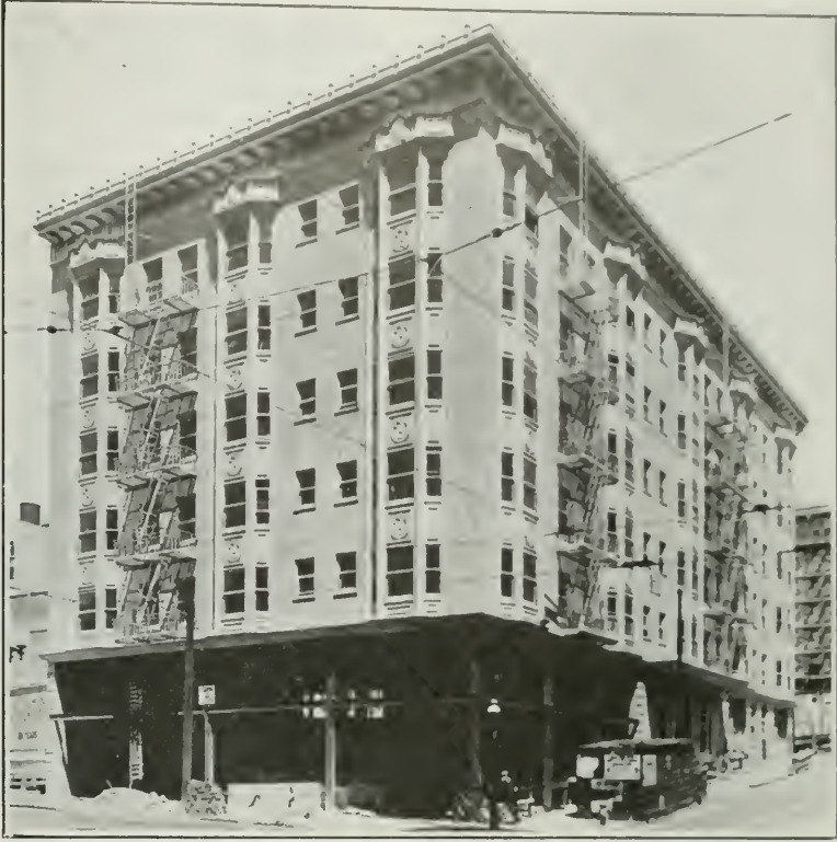
APARTMENT HOUSE, TAYLOR AND GEARY STREETS, SAN FRANCISCO FOR I. ROSENBERG - JOSEPH CAHEN, ARCHITECT This high class apartment building is equipped with a "Kerner Built-in-the-Chimney Incinerator"
