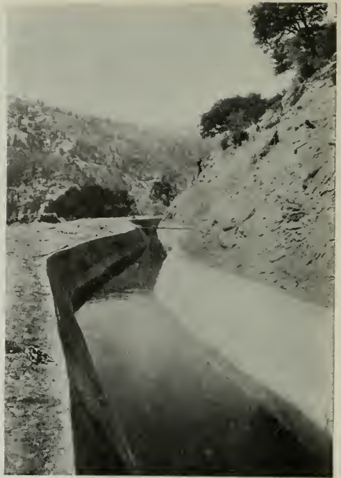
Aqueduct at Early Intake.
