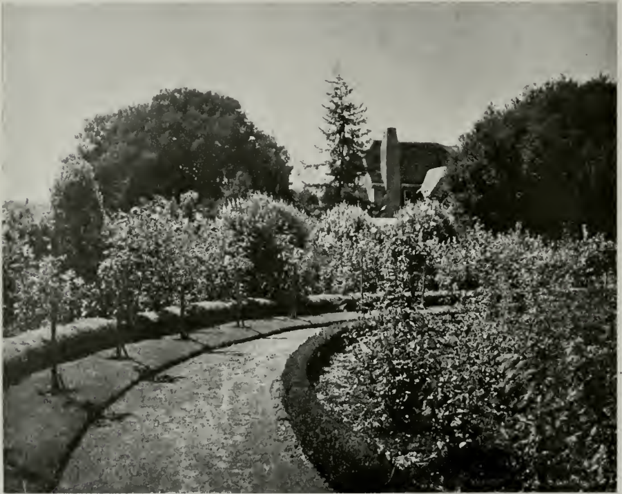
VIEW IN GROUNDS, HOUSE FOR E. J. McCUTCHEN, ESQ., LOS ALTOS, CALIFORNIA
