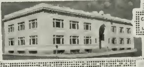
CITIZENS SAVINGS BLDG. PASADENA, CAL.
