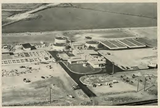
AERIAL VIEW of Cantra Costa Sewage Plant addition. The lake adjacent to the plant was farmed by flood waters. The 78" outfall line from the sedimentation tanks farms on integral part of the dyke protection system. (Brown and Caldwell, Engineers.)
