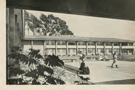
tectural firm of Stone, Mulloy, Marraccini, and Patterson found that by using a steel framework an extra floor could be added. The steel system allows the use of lighter walls and floors, saving from 35 to 50 pounds per square foot of floor area. Smith and Moorehead are the structural engineers. One floor providing approximately 65 additional beds will be completed by
