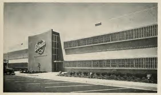
EITEL-McCULLOUGH, INC. is another addition to the rapidly expanding industrial area south of San Francisco. Exterior of 2-story office is surfaced with ceramic veneer of  $\frac{3}{4}$ " square tiles applied to the slab while being poured. (Vincent G. Raney, Architect. Hall, Pregnaff & Matheu, Structural Engineers.)
