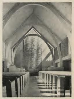
glu-lam wood arches in lieu of the precast concrete. The alternate bid proved to be considerably less expensive and we were happy to honor the substitution, Mr. Jones states, as it resulted in a much more refined cross vaulting due to the reduction in the mass of the
