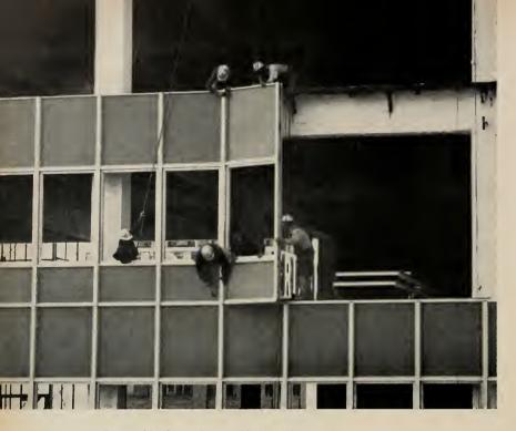
INSIDE SETTING No scaffolding installed in installation of this woll. Note interior back-up pon primed at factory, ready for fnish.
