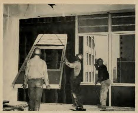
Maximum flexibility for expansion and cantraction during thermal changes is made possible by split mullians. Nate the studs far fastening inta angle clips in upper left of frame.
