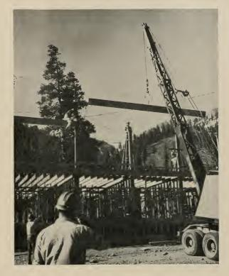
girders, and inclined eable tension members. Each half of the main frame acts independently in somewhat the manner of a guy derrick, with the roof girder functioning as the boom, the column as the mast, and the inelined cables as the guys.
