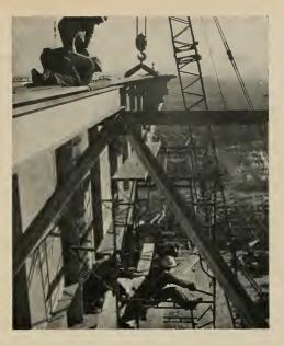
TESTING CALIBRATIONS on high tensile bolts used to splice flanges of 365-ft. girders which cantilever 142-ft. each way.
