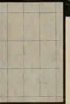
Detail shows how large scale appear-ance is accomplished by surrounding a group of pieces with a wide, slightly concave, contrasting color, accent joint. Smaller flush inter-mediate joints harmonize with the Ceramic Veneer color.
