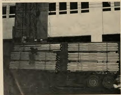
Factory prefabricated fromes delivered to jobs on pallets bundled six to each pallet and hoisted to floors.
