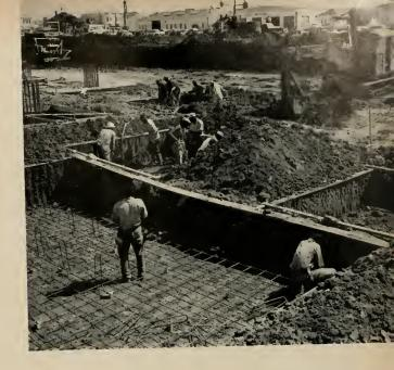
BELOW: First floor of new building as seen from roof of adjacent building, showing supports for a plywood base serving as the first "layer" of the lower floor of the Factory section . . . reinforcing steel is placed on top of the plywood then a layer of concrete is poured . . . concrete columns will extend upward as supports for the second floor.
