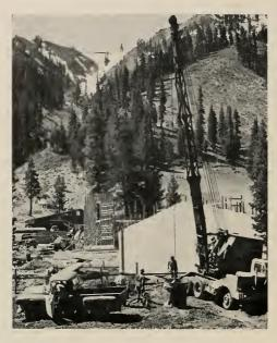
PRESS BUILDING: Takes form as workmen prepare to pour cancrete wall.
