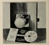
Incorporates many new labor-saving features, simplifies installation with only three preassembled units and no knob screw is required to fasten the knob to the spindle. An important safety feature is the panicproof locking button which is automatically released when the knob is turned. Known as the 5280 series, complete data is available from the manufacturer, Yale & Towne Mig. Co., Chrysler Bldg., New York 17, N. Y.
