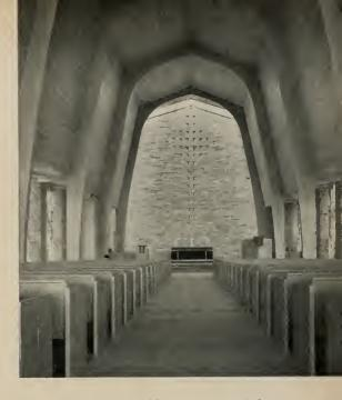
glu-lam beams are supported by a tension ring at the eave line to make up the dramatic roof of the structure.
