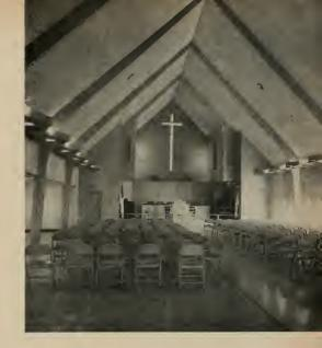
doubling the membership. Glu-lam arches form an attractive structural shape for the nave, and exposed wood decking and exterior cedar siding relate it with the surrounding wooded countryside.
