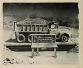
Additional scale sections may be joined for greater length and capacity, requiring only 9 standard bolts, and can be relocated as the job requires. These portable vehicle scales incorpo-
