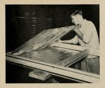
Right View shows the workman completing a maximum prefabrication: frames are assembled complete except for glass.
