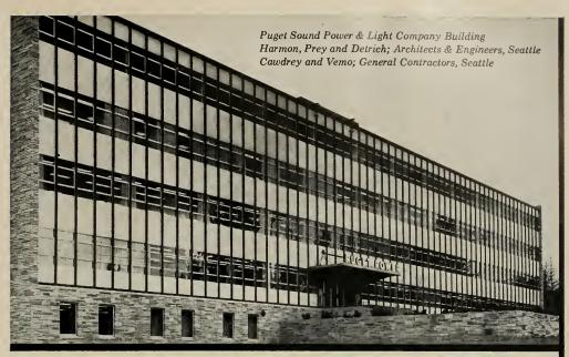
The exterior face of the Fentron panel is porcelain enamel over 16-gauge USS Vitrenamel Sheet. Interior is 14-gauge USS Cold Rolled Sheet with insulation sandwiched between. "u" factor is .104. These panels are effective as covers for spandrels and columns, and as mullions complete with windows.
