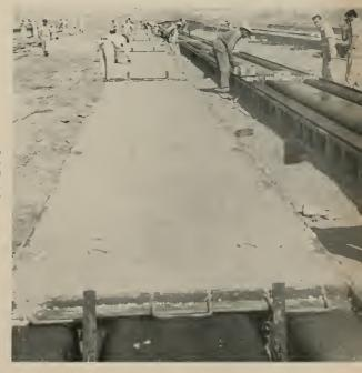
AT RIGHT: Finishing crew puts final touches an pre-tensioned, prestressed concrete panels while another 350 ft. casting bed (right) is prepared for pour. Each bed accommadates eight 40-ft. panels, maintaining a 56-ton stress during the  $2^{1/2}$  day curing period.
