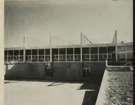
**STEEL FOR VERSATILITY!** Exposed steel trusses solved a problem in the construction of the Green River School's gymnasium ... and saved about \$30,000 in building costs! Since soil conditions required the building to be founded on pilings, the gym could be recessed half its height into the ground. This unique design allowed for a continuous roof plane. For your next project, consider the advantages of steel—United States Steel.
