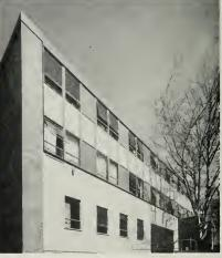
Illustrated: Ariston steel curtain walls with insulated panels. Phi Kappa Sigma Fraternity, Berkeley, California. F. P. Lathrop Construction Co., Contractors Ratcliff and Ratcliff, Architects
