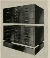
Lyon flat drawer files are provided with hinged paperweight on front and protecting hood on back of drawer to prevent edges of paper from curling. Stops prevent drawers from being pulled out accidentally, but easily released when desired. Each cabinet has five drawers; may be stacked one above the other to any desired height. Available in three sizes and with a variety of drawer divider arrangements. Complete data from the manufacturer, the Lyon Metal Products Inc., Aurora, Illinois
