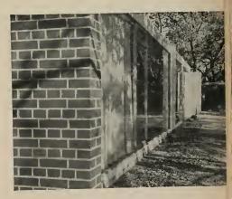
Steel is complementary to any building material. Here the steel frame is set off at either end with English Bond brick bearing walls. The architects favor white painted frames so that shadows will give the structures a "sculptured look."
