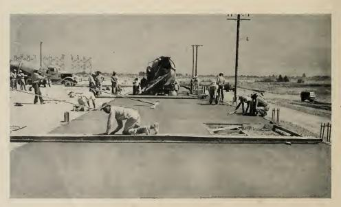
REINFORCING STEEL—for the continuous framing shown (right) protruding from acres of concrete floor slobs.
