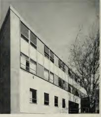
Illustrated: Ariston steel curtain walls with insulated panels. Phi Kappa Sigma Fraternity, Berkeley, California. F. P. Lathrap Construction Co., Contractors Ratcliff and Ratcliff, Architects
