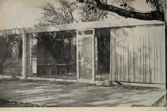
The steel framing of this building has an 8-inch WF 48-pound member running through the center, supported on a  $5 \times 5$  16-pound column. The front and rear members are 12-inch 10.6-lb. steel channels. These are supported on the  $5 \times 5$  center column and masonry end walls. Intermediate roofing members are 6-inch channels and 8-inch wide flanges.
