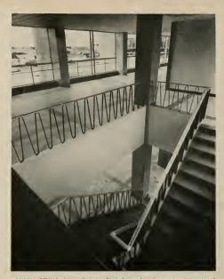
MAIN STAIR from 1st to 2nd floor is of steel with aluminum rail, with Red Verona Marble freads and risers. The lobby floor is af Verona in a field of white Columbia Marble.
