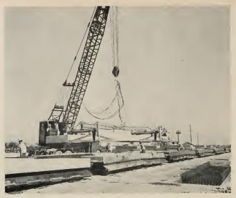
PRE-CAST, Thin shell roof panels (left) being removed from forms. Stripping process requires obout three minutes.
