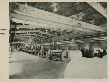
LOOKING down production line of paper-making machines—side walls and raaf strongly reinforced for large overhead crane.
