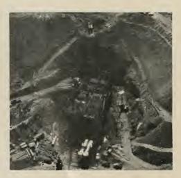
In California's Mojave Desert the Air Force is completing a giant concrete test stand which will provide the means to test rocket engines and missile components having up to 1,000,000 pounds of thrust. The new stand, an important addition to America's missile testing program, is the largest stand constructed by the Air Force to date.
