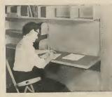
The "wall-hung" system offers full flexbility for installing, rearranging and re-moving shelving, display boards, black-boards, coat racks, lightweight desks and other similar furnishings. Using vertical, slotted steel columns that are easily in-stalled at 36" intervals along walls, any standard bracket-equipped fixture can be quickly set in position, readjusted or inter-
