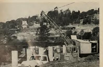
Erecting rigid steel frames; floor joists of steel ribs were landed on concrete piers and wall of 45 degree lot, ceiling joists bolted to seven concrete block pillars; 12 foot by 1-foot sheer wall connected to two of the interior frames will provide lateral support.
