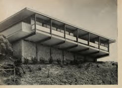
Cantilever extending 11 fect over supporting foundation and wall is made possible by using steel sections. Structure utilizes skeleton of steel ribs which support roof and floor without load bearing walls.
