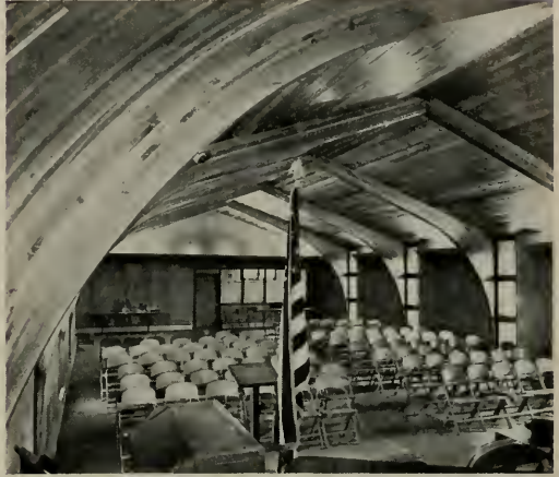
Heavy haunches of the fir arches provide support for this church.
