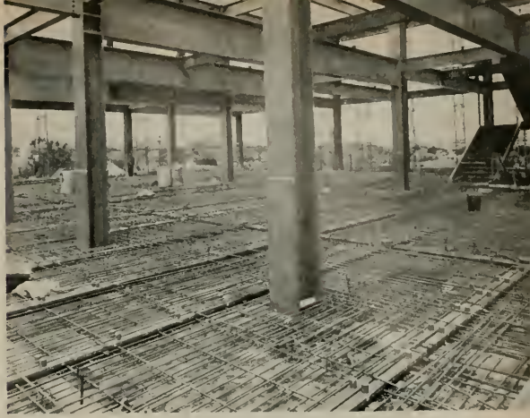
STEEL in place for concrete pouring.
