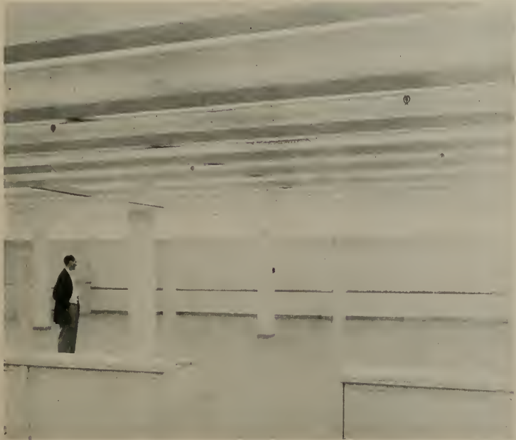
FIG. 3 Note the exceedingly low contrasts, and how the ceiling is cut off by the fixtures themselves at high angles. This is a case where fixtures, reflectances and distributions were all carefully matched for best seeing conditions.
