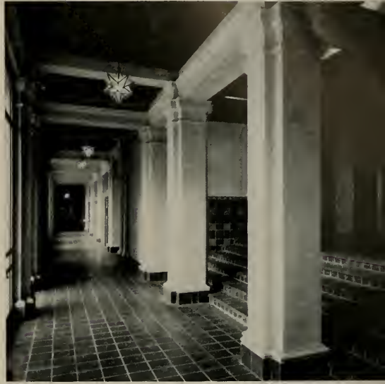
INTERIOR VIEW of the Main Corridor of the Chapel entrance, showing combination use of wood panel ceiling, tile floors and decorative tile wainscoting.
