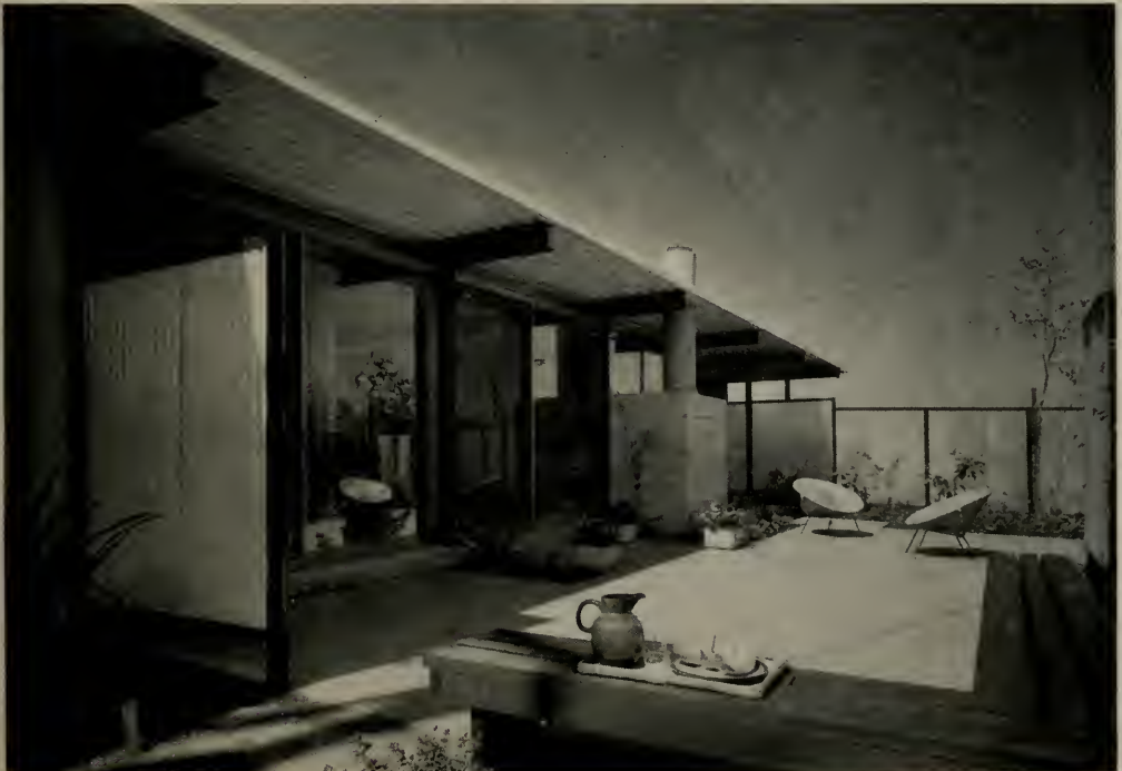
A STEEL HOUSE FOR MASS PRODUCTION: In this residence, designed for mass production, Architect Soriano has utilized 10 ft. by 26 ft. module steel, plus a 1½ in. steel decking. I-beams extend beyond walls, with steel sash and floor to ceiling windows, to provide roof extension for shade and protection. Interior has exposed steel beams. (1955)
