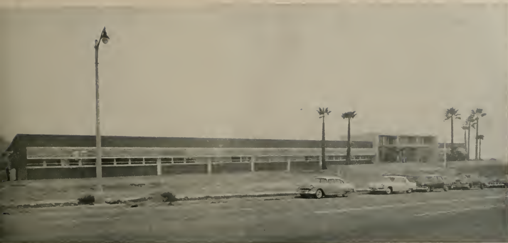
NEW $1,175,000 Allstate Insurance Company Regional Office Building
