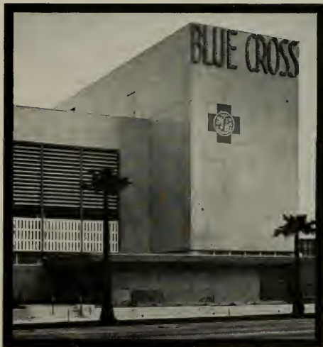
• Architectural Porcelain Enamel used for veneer, louvers, soffits, sills, jambs and headers.
