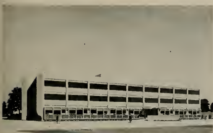
SANTA CLARA COUNTY JAIL AND SHERIFF'S DEPARTMENT ERNEST F. TRESEDER, A.I.A., ARCHITECT 30 LAFAYETTE SQUARE SAN FRANCISCO, CALIF.
