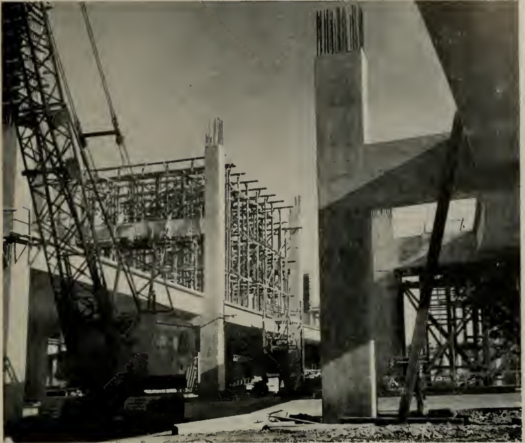
SHOWN ABOVE are separation structures, San Francisco Bay Bridge approach.
