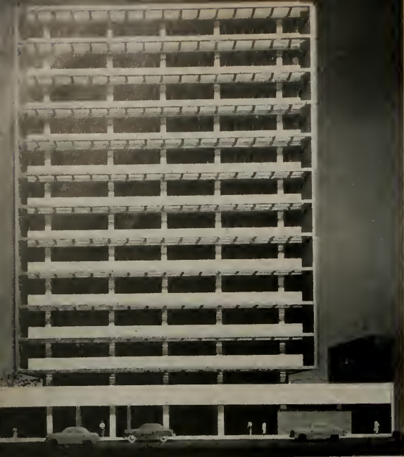
ELEVATION , showing horizontal sunshades. Vertical louvers indicated as projected beyond wall of building. Glass walls surround each floor. Floors are concrete poured on corrugated metal forms.
