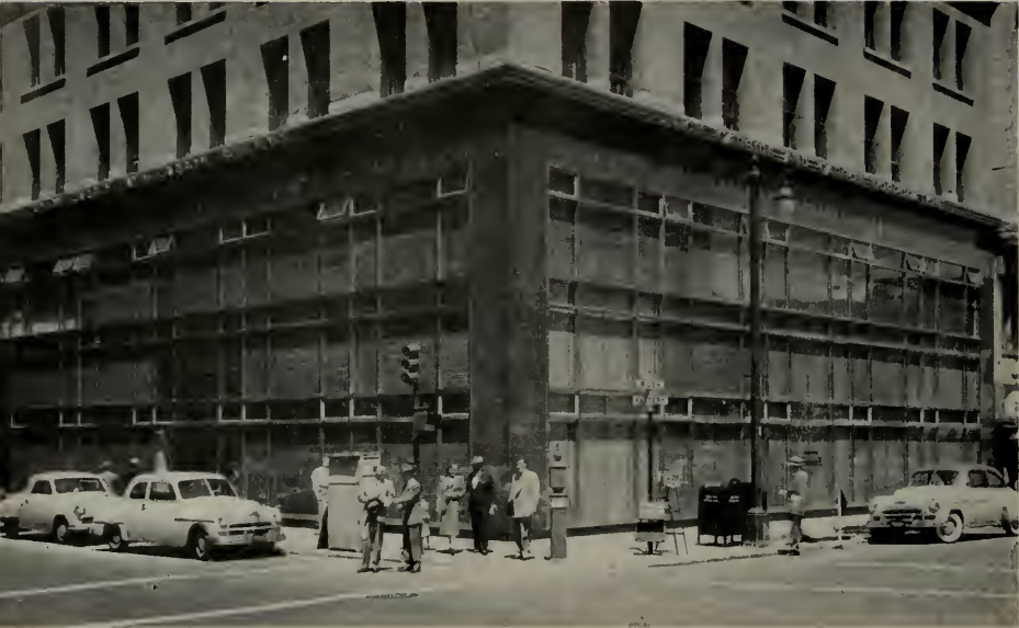
UNION CARBIDE BUILDING, 22 Battery Street, San Francisco, remodeled and refaced with stainless steel and glass, and trimmed with red Swedish granite. THOMPSON & WILSON, Architects
