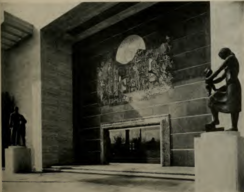
ENTRANCE close-up showing colorful mural constructed over doorway
