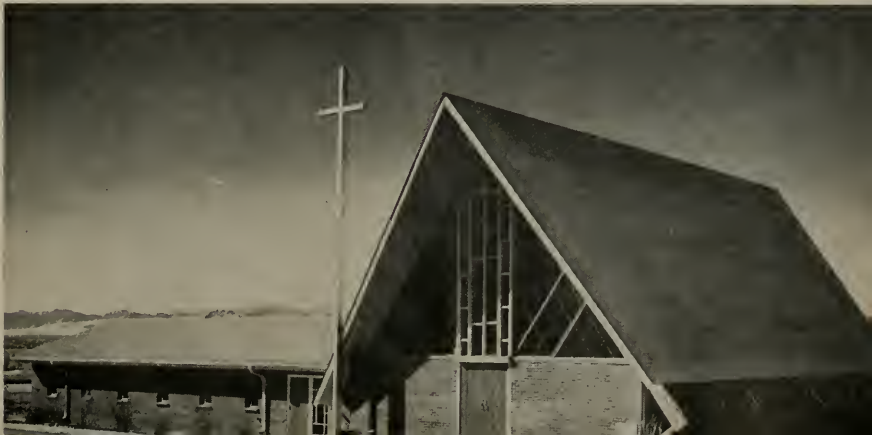
ADVENT EVANGELICAL LUTHERAN CHURCH, Westminster, Colorado, designed by Orrie Joel Holman and Associates, Architects. A church of charm indeed.
