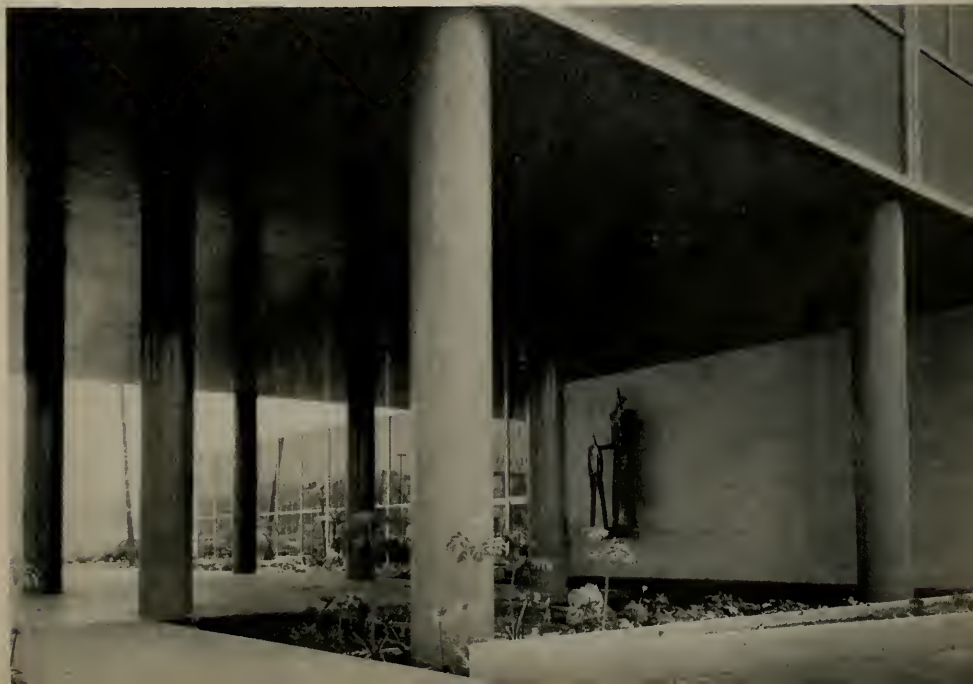
West entrance foyer showing glazed ceramic tile soffit and column facing with anchor type ceramic veneer wall as background for planting and for bronze sculpture.
