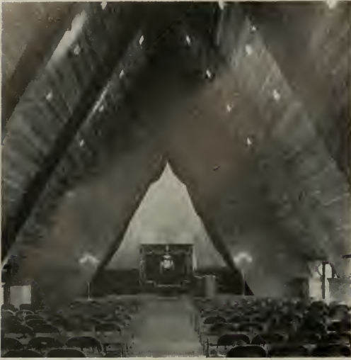
TEMPLE BETH JACOBS CHURCH, Oakland, California, designed by Albert Hunter, Architect. The wedge shaped roof offers beauty and simplicity.
