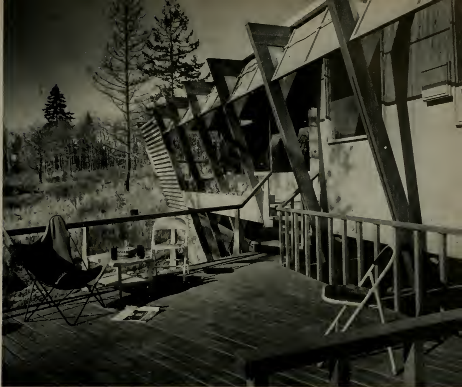
Attractive rustic, rough-textured decking and frame work of Douglas Fir in the Eugene, Oregon, residence of Dr. and Mrs. Robert E. Nye. Norris M. Gaddis, Architect.
