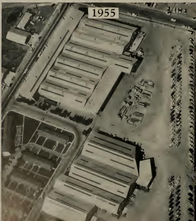
AIR VIEW of 3½ acre plant. Note provision for customer parking.
