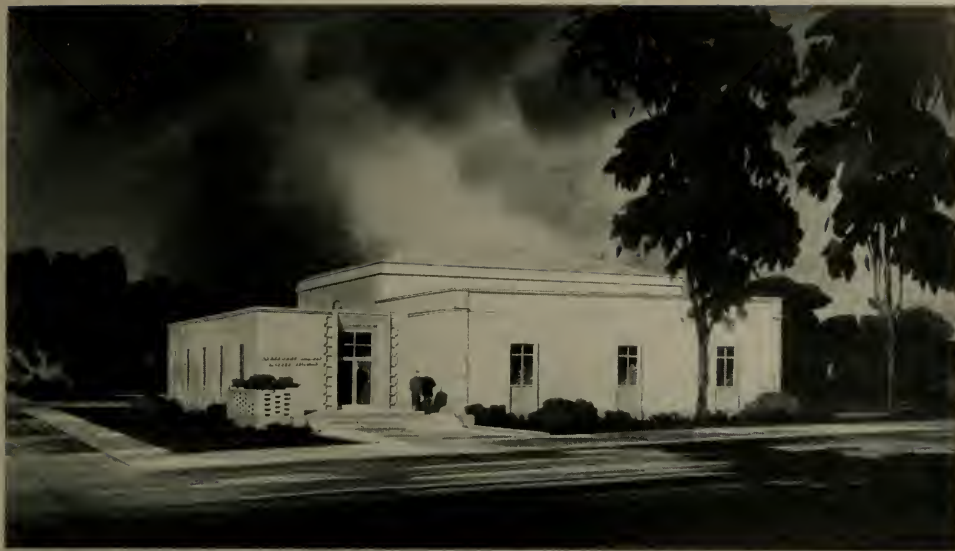
CLAREMONT COLLEGE SCIENCE BUILDING
