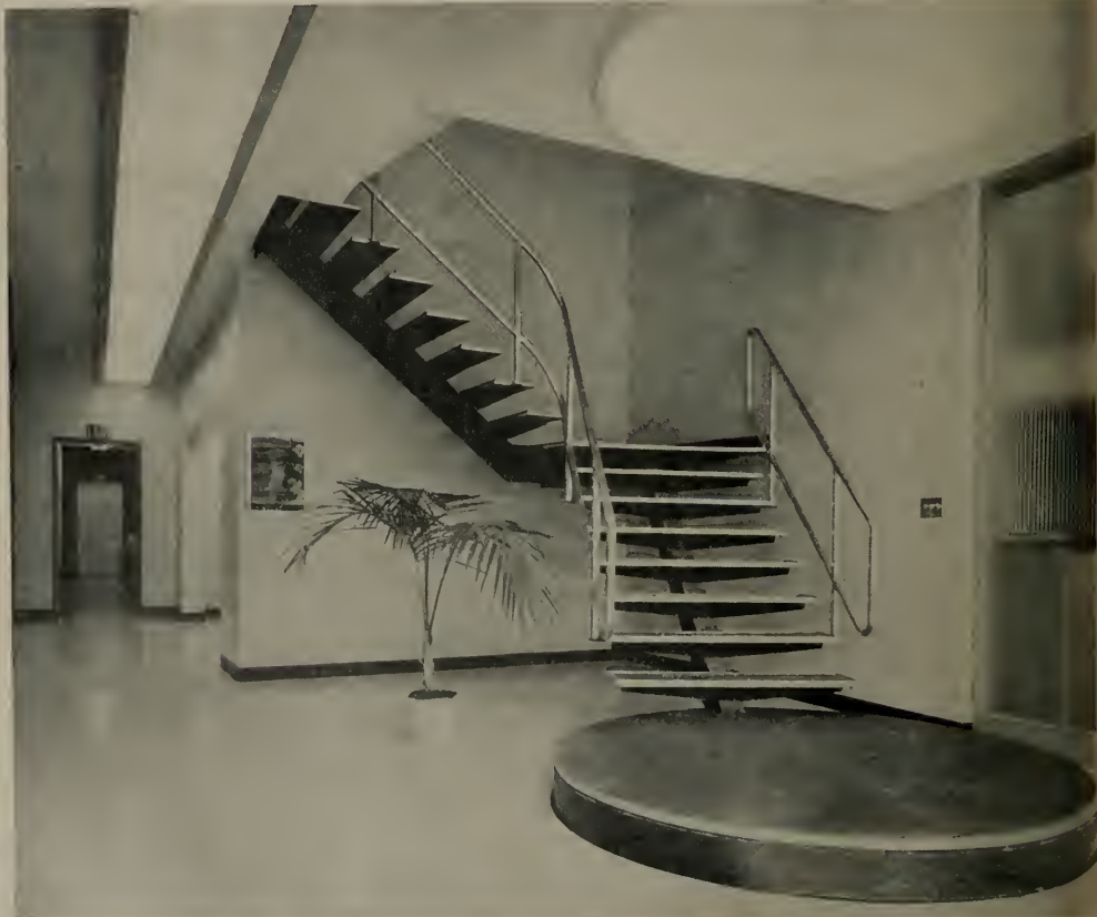
SPACIOUS LOBBY showing interesting and unusual stair treatment.
