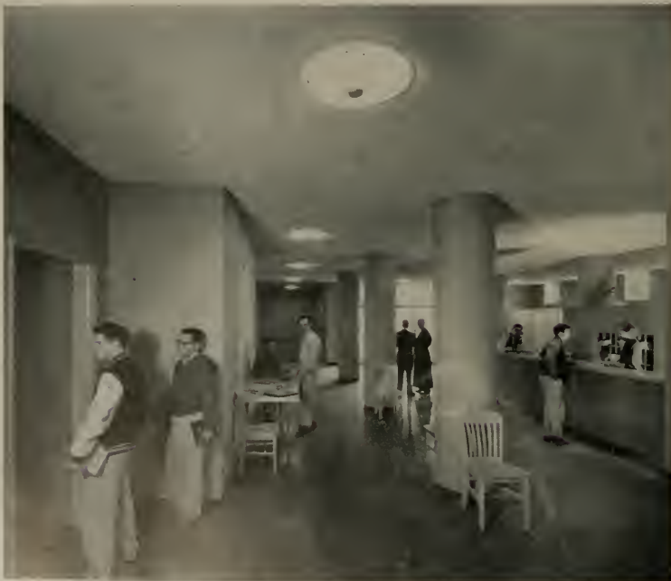
ANOTHER VIEW OF MAIN LOBBY Shows entrance of the seven story steel and concrete student residence. Walls are covered in gray and green, floors in red asphalt tile, and woodwork is natural finish birch.
