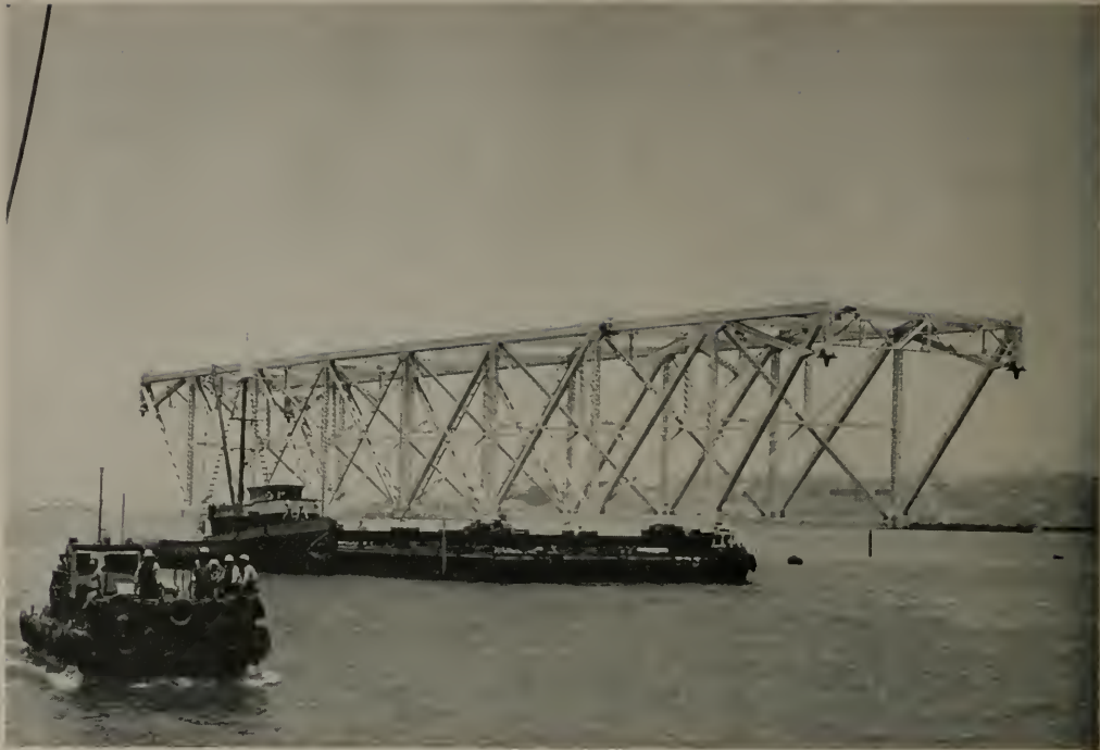
Fig. 1—Aluminum Falsework Truss Being Towed Into Position.
