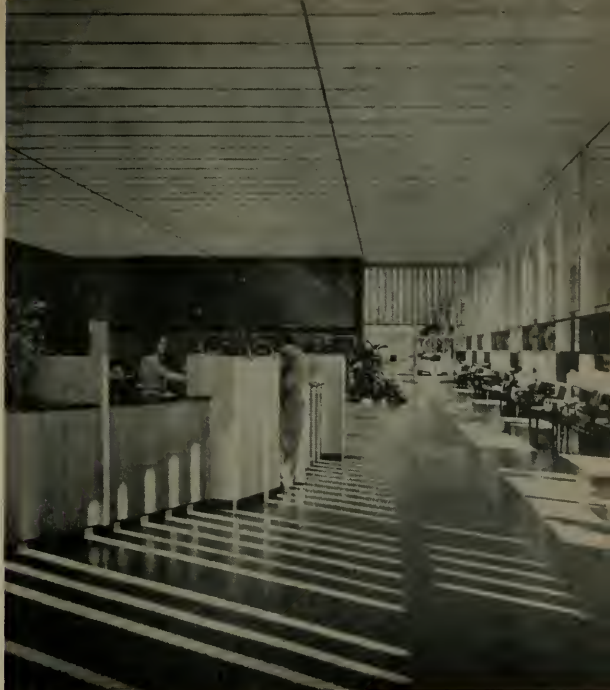
LUMINOUS CEILING illustrated above is implemented with instant-start fluorescent lamps above corrugated plastic.
