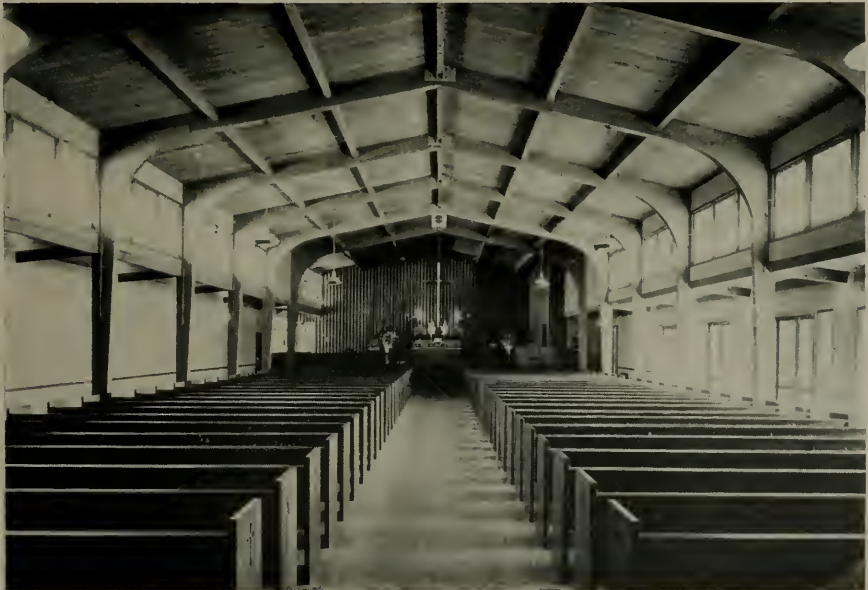
FIRST LUTHERAN CHURCH . . . Tarrence, California. Edward David Davies, Architect.
