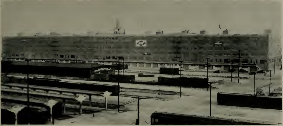
ONE of first Dinwiddie Construction Company jobs in San Francisco . . . the Southern Pacific Terminal Warehouse.
