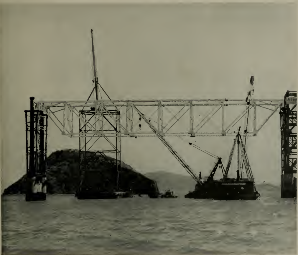
Fig. 2—Aluminum Falsework Truss Raised Into Position and Ready for Steel Erection.
