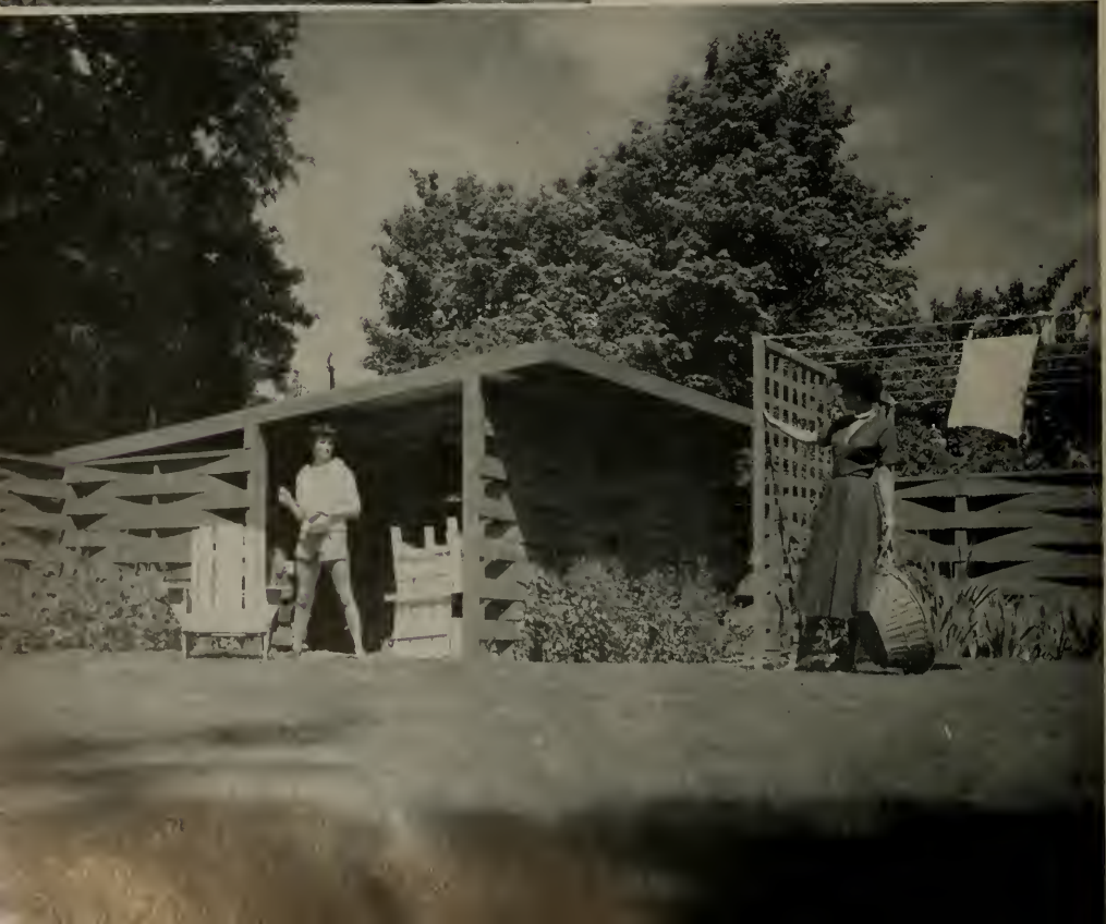
ANOTHER example of clever use of rough sawn lumber with simple design lines to create an outdoor garden area is seen in the illustration below of the M. C. Evans residence in Forest Grove, Ore.
