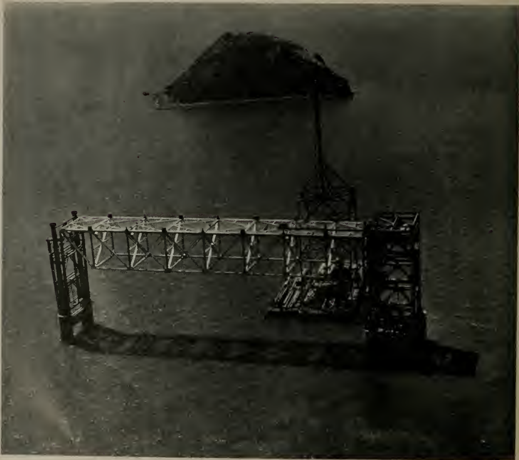
Fig. 3—Erecting First Piece of Steel Upon Aluminum Falsework Truss.
