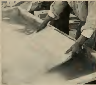
1 Ceramic Veneer units must be soaked in clean water for one hour before using. Wall surface should also be damp at time of setting.
