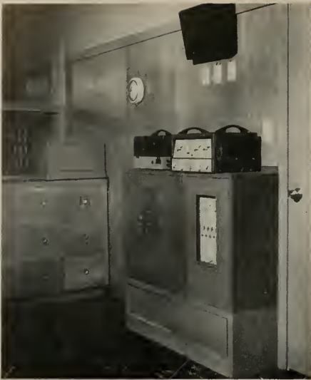
Heart of system is located in Sacristy. Automatic roll player sits on counter top to left. In center is bell cabinet; matching cabinet to right contains clock and timer mechanism.
