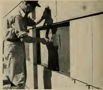
3 To insure permanent bond between Veneer and structure, the wall surface is also brushed with the same Portland cement mixture.
