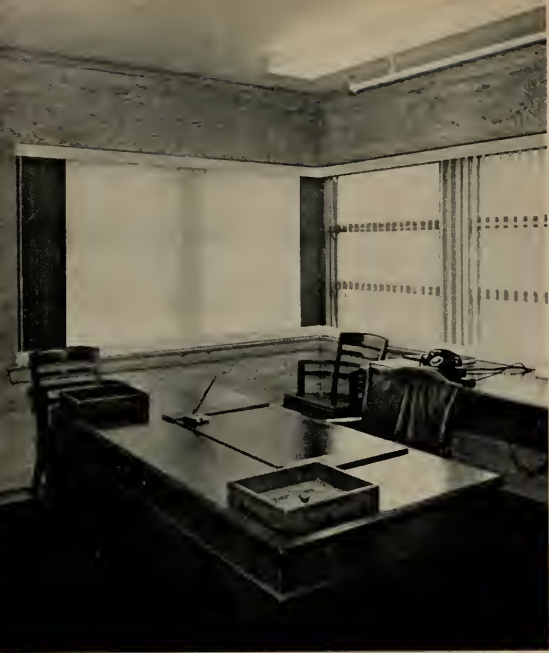
Decorative Douglas Fir plywood in 3-D effect installed in a private office.
