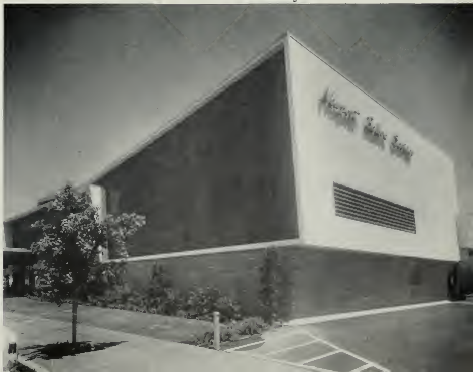
VIEW of new building from "boy side".
