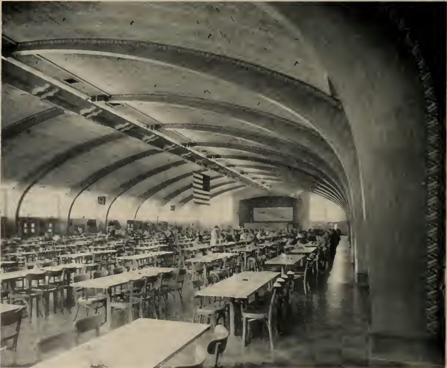
BOEING CAFETERIA—Shows how architects can design shop-grown arches and trusses to span tremendous widths and at the same time achieve striking beauty.
