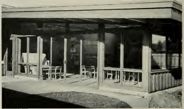
Arislide steel sliding doors as used in the New Annex to the White Oaks School, San Carlos. John Carl Warnecke, Architect
