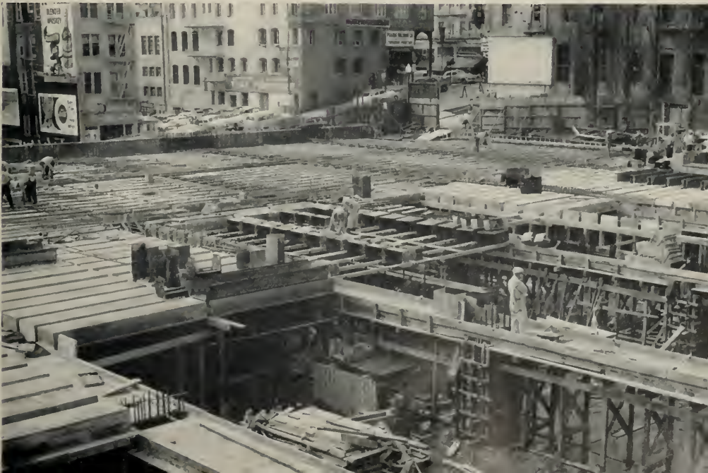
General view of roof framing.
