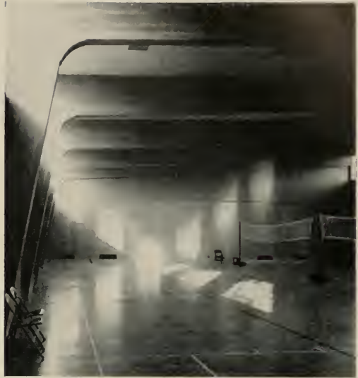
CURVED BOOMERANG TRUSSES seen here create a striking effect in this multi-purpose school room.
