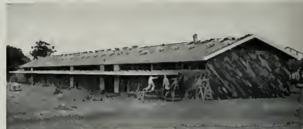
To protect against termite damage for the life of the buildings, BAXCO Chemonited (pressure treated) Lumber was used for sill plates, wall studs, rafters, and sheathing.
