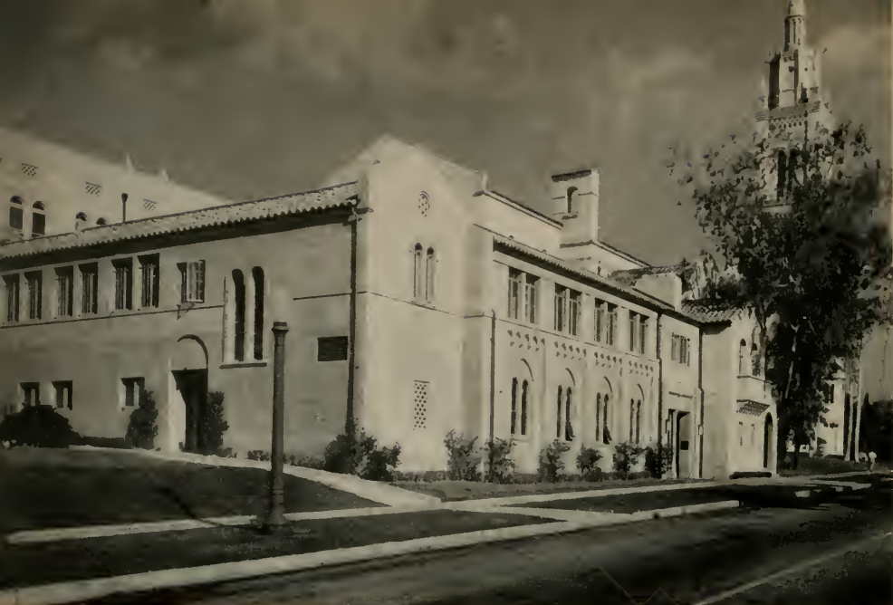
ADDITION TO WILSHIRE METHODIST CHURCH — Wilshire Boulevard
