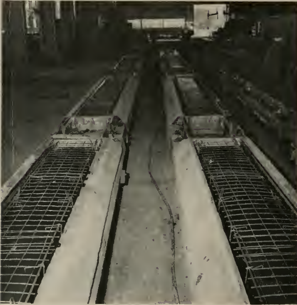
BATTERY OF CHANNEL SLAB MOLDS
