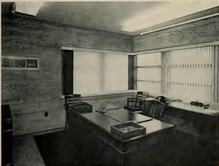
Random length panels have been used (below) with a pleasing and unusual effect in this Charlotte, North Carolina, office.
