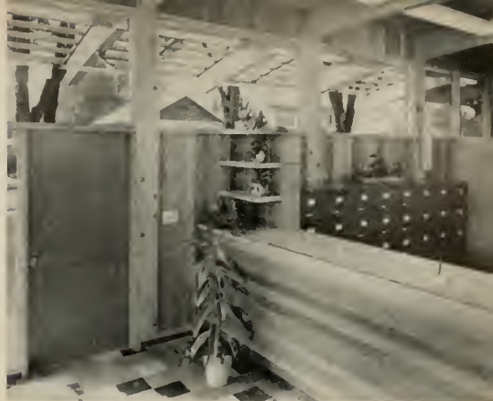
LOOK AT THE LOBBY —from the front street window side, shows the handling of arches as exposed roof members; high windows and fluorescent light to develop light.
