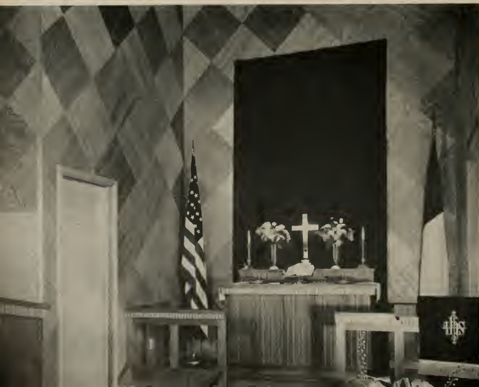
3-D Plywood not only gives three dimensional effect to this Church nave, but has good acoustical properties as well.
