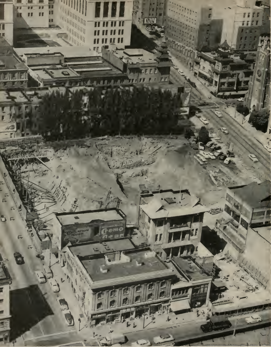
SITE CLEARED—EXCAVATION WELL STARTED
