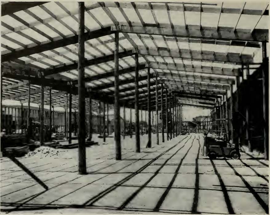
CONSTRUCTION PHASE—United States Products Corp. Warehouse
