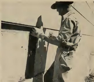
5 The C.V. unit is then set in place. Excess of mortar will be forced out of joints from the back, leaving a \frac{3}{4} inch mortar bed.
