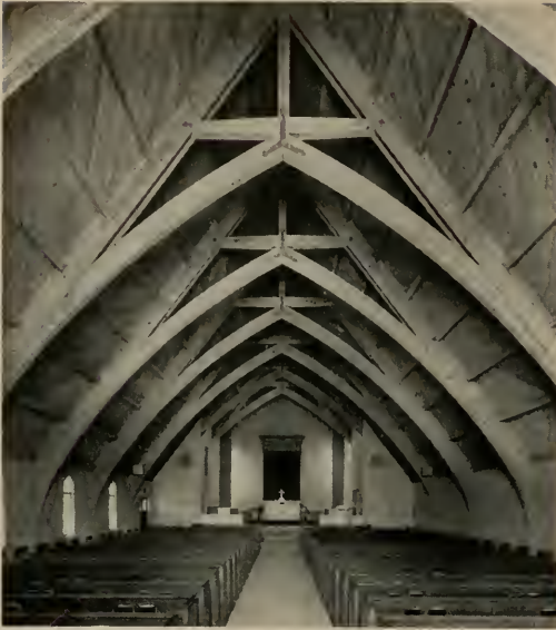
First Methodist Church, San Gabriel, California. Sandblasting of all wooden arches, decking, purlins and superstructure followed by overglazing retains texture and grain of wood in this church by Edwin Westberg of Quintin-Westberg, Architects.
