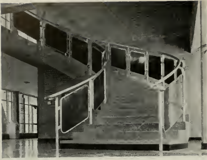
Aluminum and porcelain rails, by Michel and Pfeffer, San Jose High School. Kump Associates, Architects
