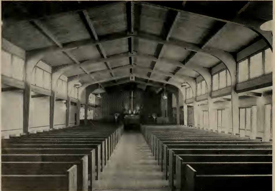
First Lutheran Church, Torrance, California (below) by Edw. David Davies, Architect and Murray K. Goldsmith, Engineer, shows large, span-free naves are no problem to achieve with modern techniques.
