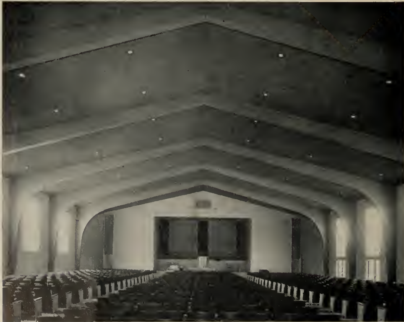
FIRST BAPTIST CHURCH (Van Nuys, California) AUDITORIUM — These V-type arches with built-up heels permit the design of simple, yet distinctive roof structures with pleasing lines.
