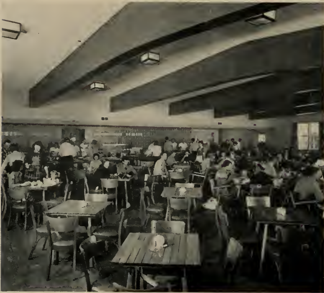
BOEING CAFETERIA—Shows how architects can design shop-grown arches and trusses to span tremendous widths and at the same time achieve striking beauty.
