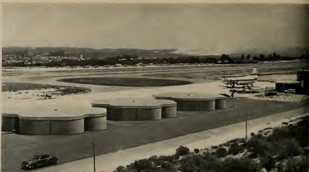
Six Cloverleaf Quad Hangars provide space for twenty-three standard private airplanes. Twenty-fourth quad serves as waiting room and utility area for pilots.
