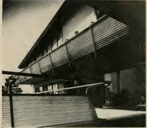
A new function is performed as part of a guard-rail on the lanai of a large apartment hotel — shatterproof and fire resistant, it meets safety code requirements.
