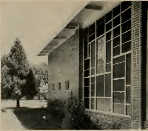
Reinforced brick exterior wall.
