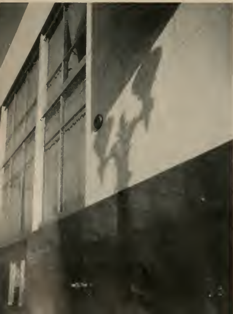
MAIN FACADE details of the Alameda County-East Bay Title Insurance Company—Oakland.
