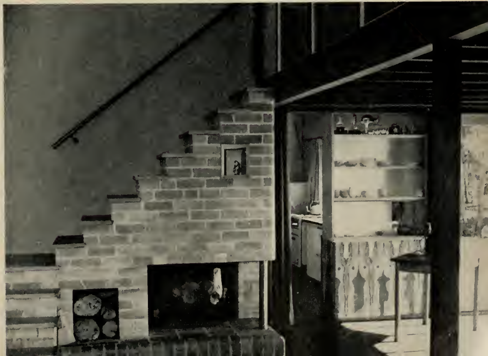
THE GALLERY is reached by these open stairs at one end of the living room. Fireplace chimney is an asbestos pipe fixed to the outside of the building.
