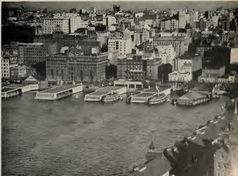
RAILWAY STATION being built on Circular Quay , links Sydney's network of underground electric trains with suburb routes.
