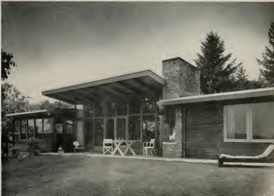
Wide overhang of roof extension shelters patio in all kinds of weather. Lovely Swedish fireplace at right of glass wall has decorative and utilitarian value.
