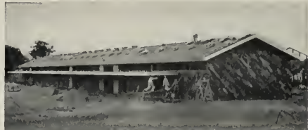
To protect against termite damage for the life of the buildings, BAXCO Chemonited (pressure treated) Lumber was used for sill plates, wall studs, rafters, and sheathing.
