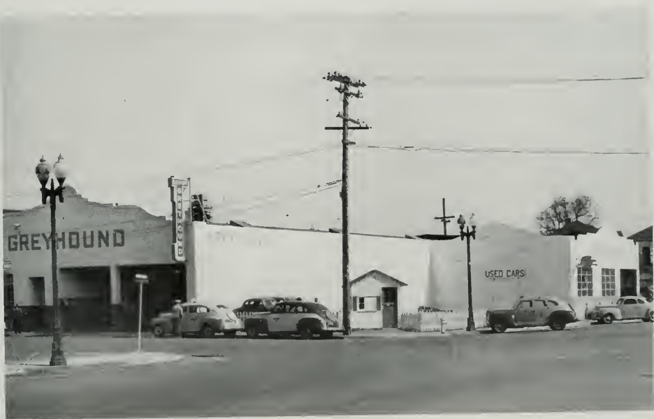
BEFORE REMODEL . . . Old building was bus-garage combination.
