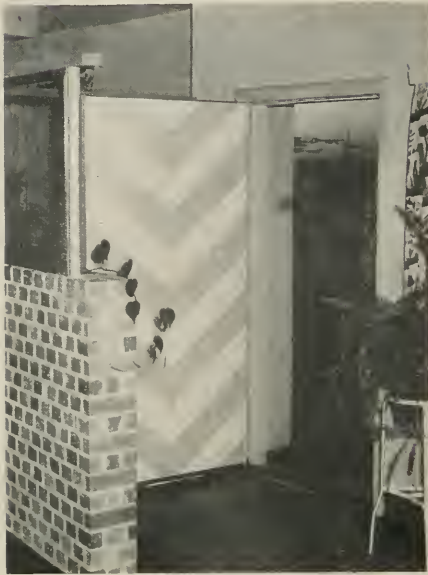
SCREEN - forming shelter at front entrance.
