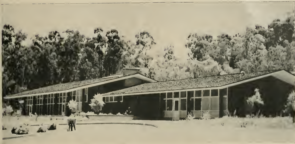
HILLSBOROUGH ELEMENTARY SCHOOL —Designed by the architectural firm of Kump & Falk and constructed for the City of Hillsborough, San Mateo county. It is an eighth grade school comprising a multiple purpose room, eight classrooms, and a cafeteria. Exterior is wood facing, roof is shake wood.
