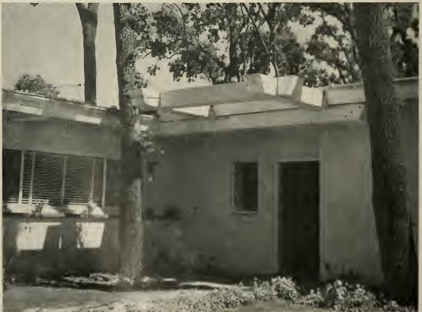
FRONT ENTRANCE - Showing large timbers extending over doorway to form canopy. Timbers were taken from Sacramento River pier.
