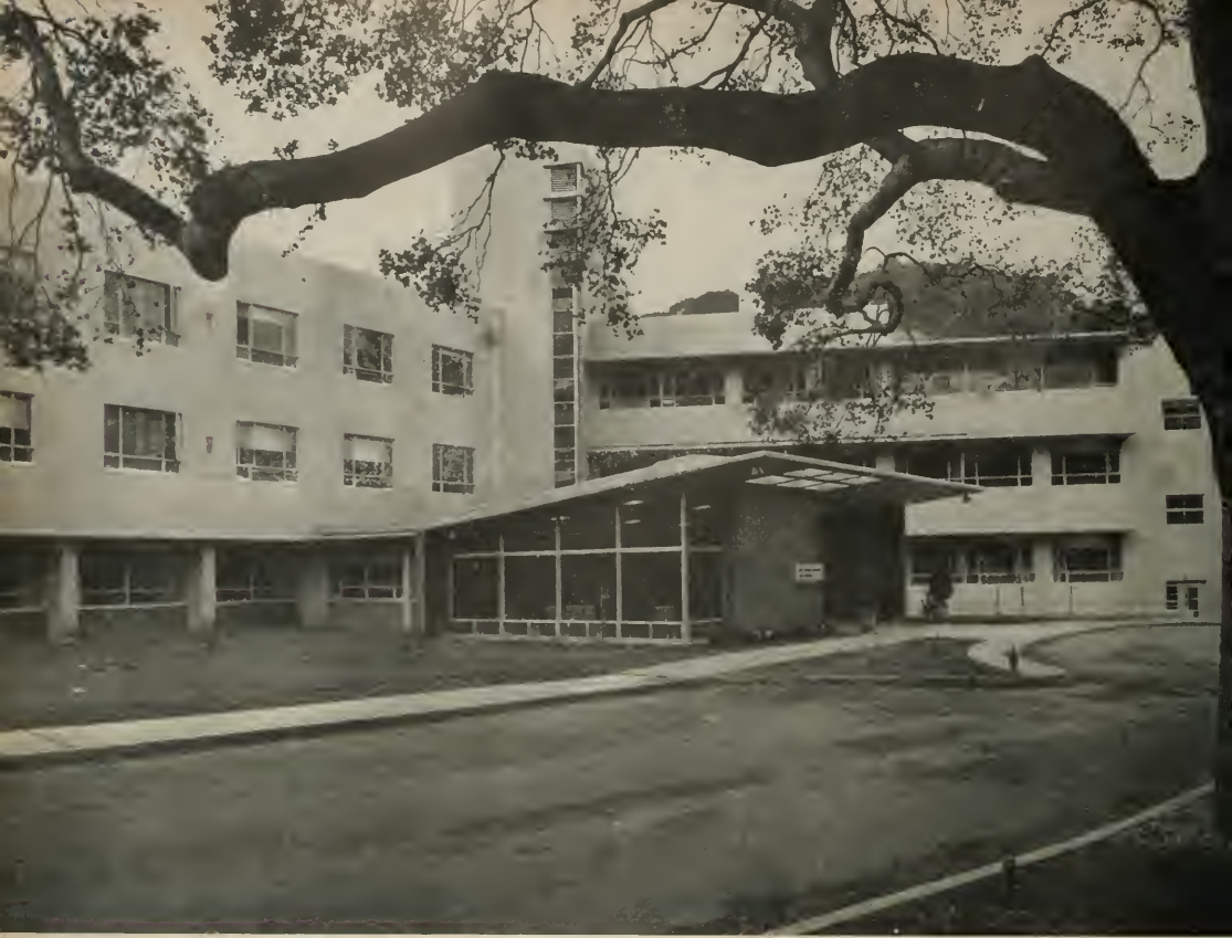
SOUTHEAST ELEVATION SHOWING MAIN ENTRANCE
