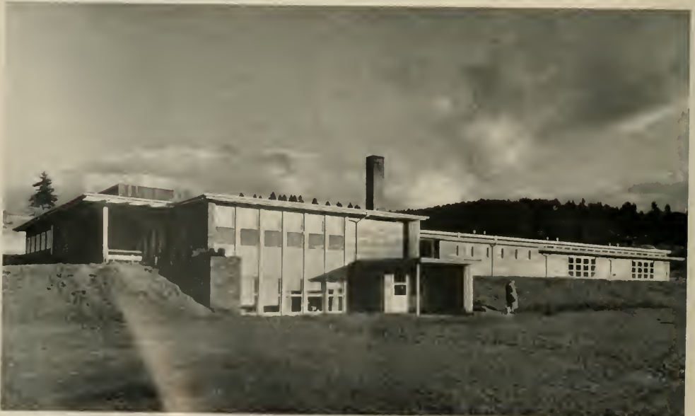
Core of school from lower level. Play field opens directly into first aid room. Final wing of school will connect with core by covered arcade.
