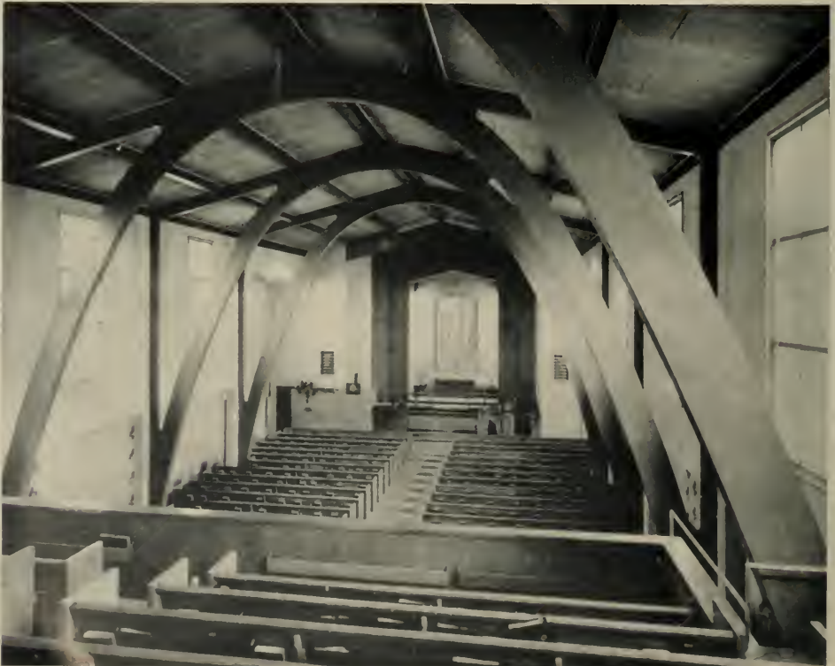
FIRST LUTHERAN CHURCH OF ALHAMBRA, Alhambra, California. Culver Heaton, AIA, Architect. Remarkable effect of a double structure is realized by curving arch members away from side walls.
