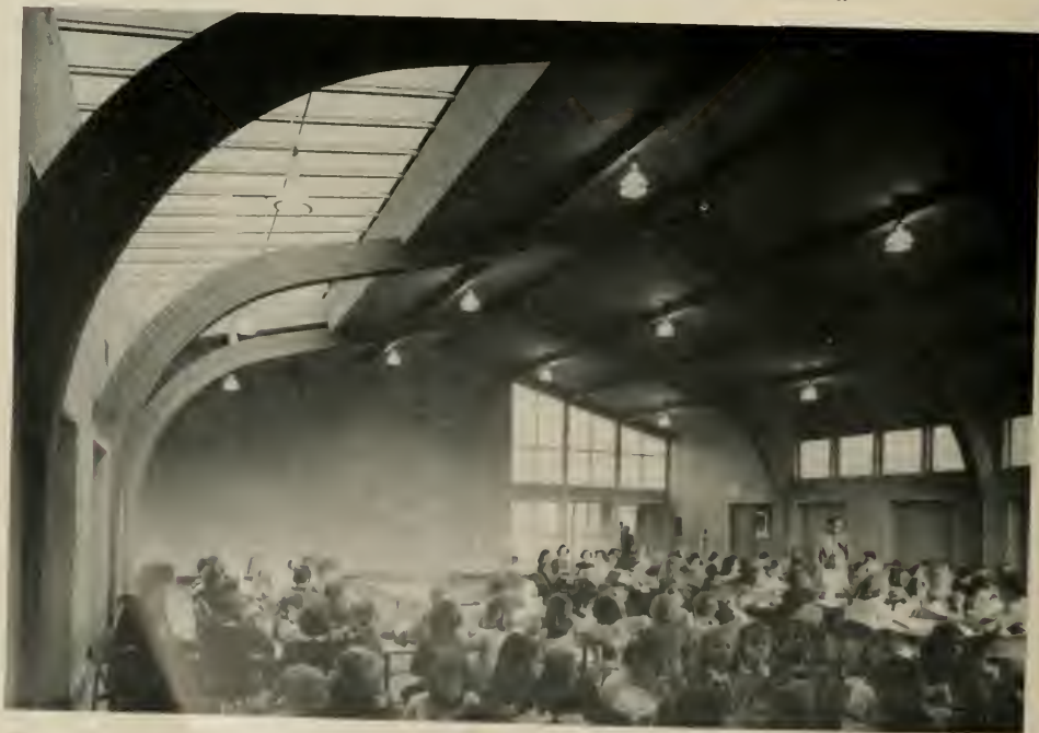
Multi-Use Building (below) . . . Auditorium and Cafeteria, exposed laminated wood trusses, skylight, partial glass ends of building, portable tables and asphalt tile floors.
