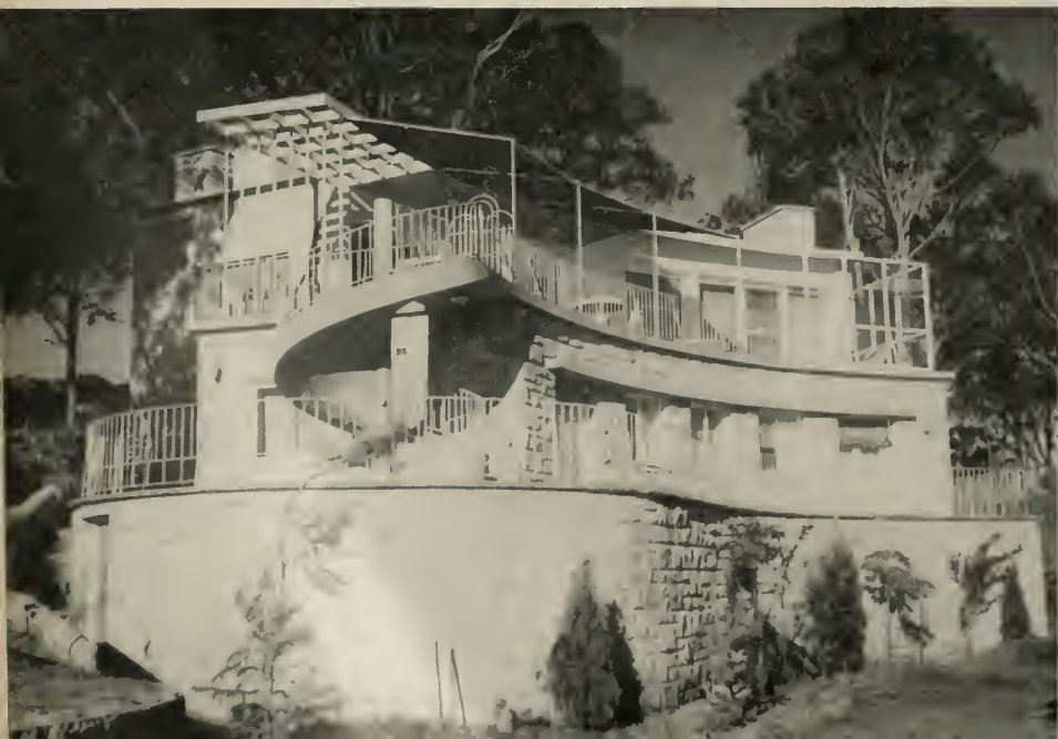
Architects Bunning & Madden designed this house to take advantage of scenic beauty and land-locked waters at Newport, near Sydney. Built on curve following contours of hillside and beach. Sandstone walls; bedrooms lower level, living and dining above. Spiral stairs to top veranda which is furnished with deck chairs and lounges.
