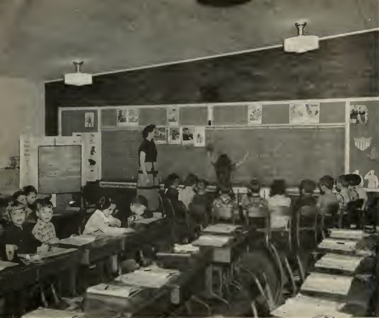
Economy roof rafters become ceiling joists for classrooms. Note pitch of roof against far wall. Acoustical tile ceilings give good results here . . . blackboards placed against end brick wall.
