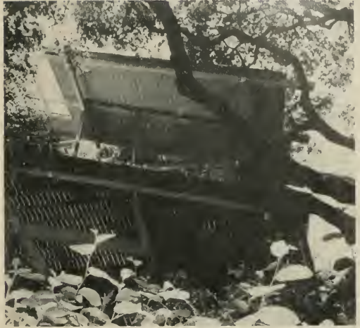
View from Canyon side shows how living space was extended by cantilevering the wood deck out into the tree tops.
