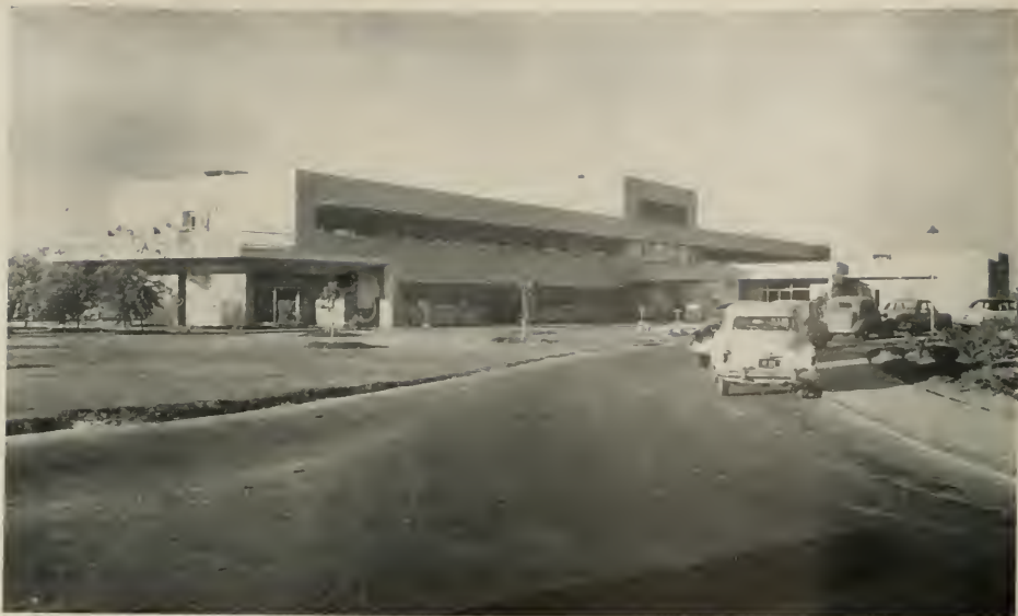
ENTRANCE DRIVEWAY to the new Pioneers Memorial Hospital
