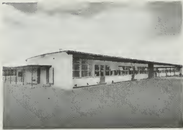
Mayfair School, Fresno Franklin & Simpson, Architects
