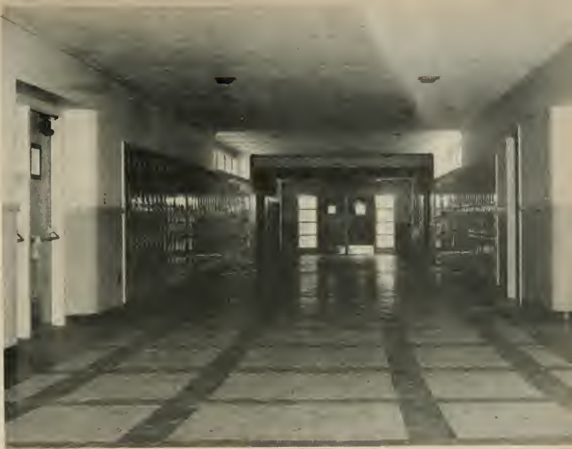
ABOVE VIEW —Shows main corridor of the Dr. James Hogan, Jr., High School, Vallejo. It is 700 feet long and 18 feet wide. Flooring is ceramic and asphalt tile. Lockers are a part of 1200 installations.
