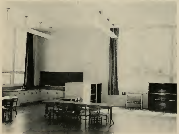
Multi-purpose room is shown above: Large windows for natural lighting, plus overhead lights and draw curtains on windows to regulate light. Acoustic ceiling, asphalt tile floor.
