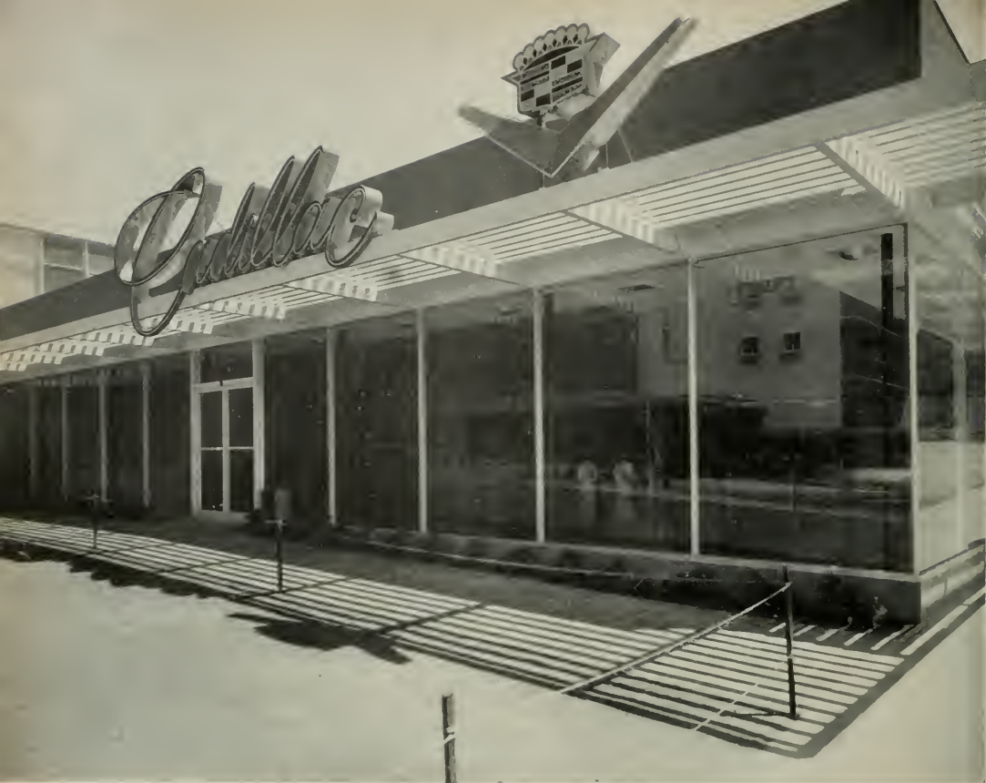
Showroom with glass front and anti-sun glare louvered canopy.
