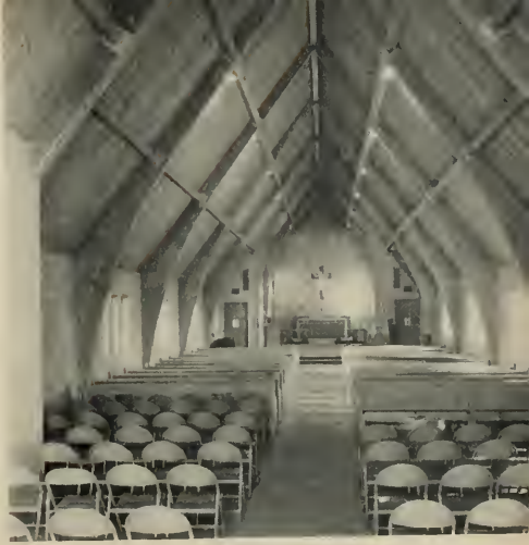
HOLY CROSS LUTHERAN CHURCH, Portland, Oregon. James L. Payne, Architect. Narrow Churches can have lofty height when arches are designed with proper camber and delicate taper.
