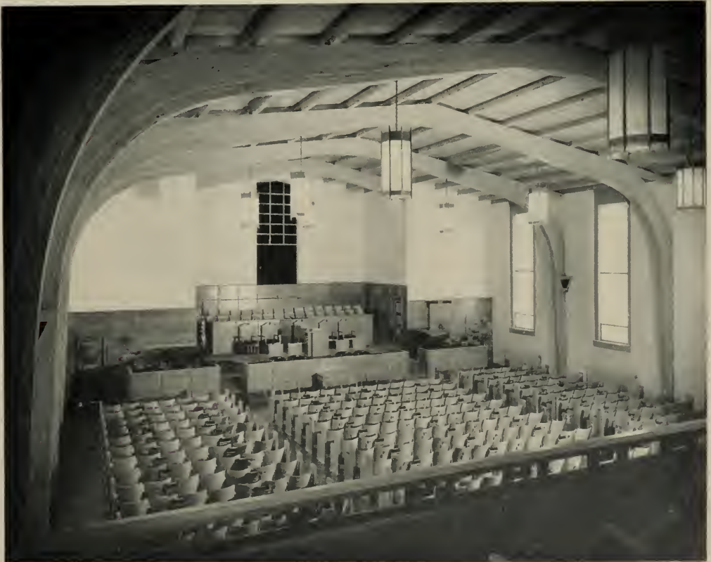
SEVENTH DAY ADVENTIST CHURCH—Boulder, Colorado. Jones and Hunter, Architects. Sweeping arches provide a nave to accommodate one thousand worshippers.
