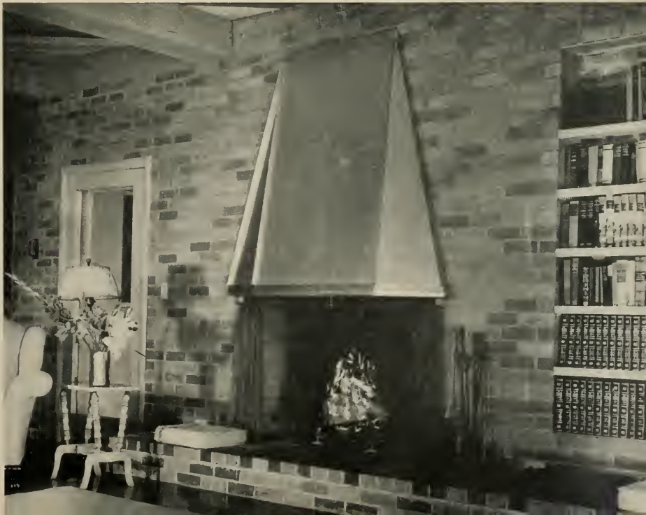
FIREPLACE - with chrome metal hood. Raised brick hearth skirts along base of brick wall and across end of the living room.
