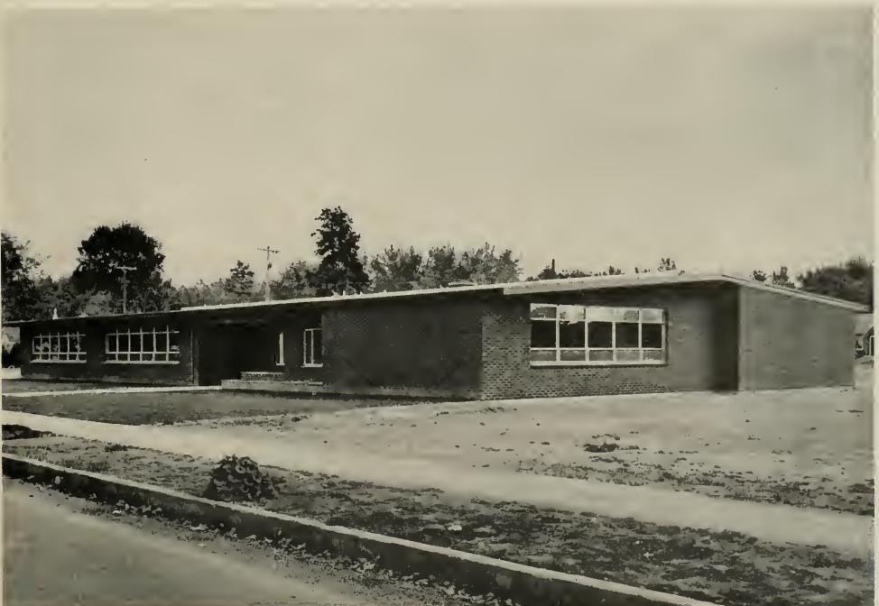
Front view of novel Madison Elementary School at Boise, Idaho—A "little" school designed to be converted to other uses when classroom demand has passed.
