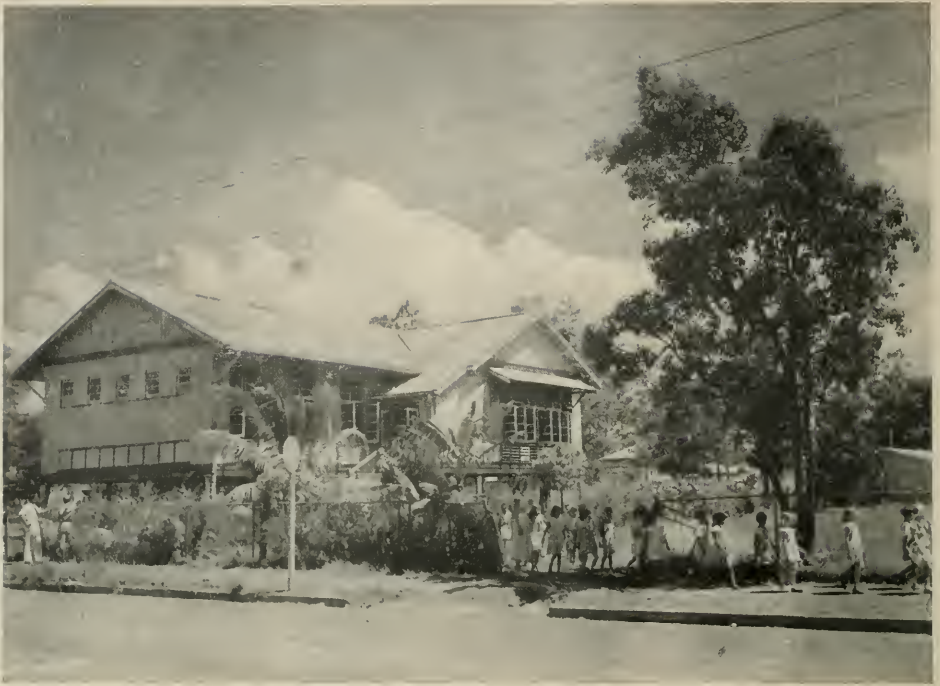
Infant School Building of Darwin's Primary School—Lower Louvers, Extensive Windows and High Piles Provide Tropic Climate Ventilation.
