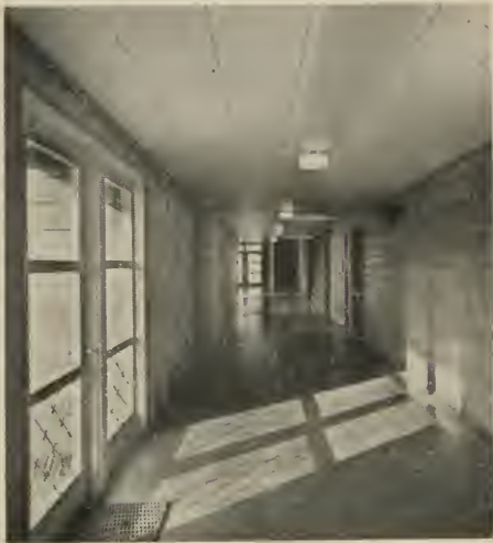
STANDARD corridor built as single loaded section paralleling each classroom wing. Note fir panelling used along walls to withstand heavy use.
