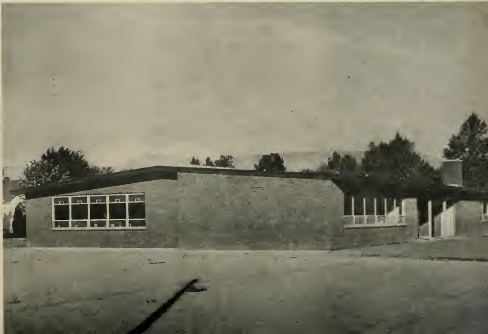
View of rear—and one side of brick building. Note uniformity of window arrangement for each of the six classrooms.
