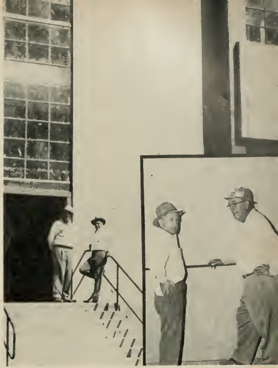
Roland Cowles, Bechtel Corp'n and Carl W. Gott of Continental Can Co. standing by 17-ton tilt-up panel. Inset - Carl W. Gott and Roland Cowles beside smooth panel cast on concrete floor. (See photo below.)
