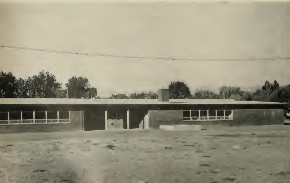
Rear view of this unusual school building shows how compact and un-institutional it looks in center of residential district of Idaho's state capital city, Boise.
