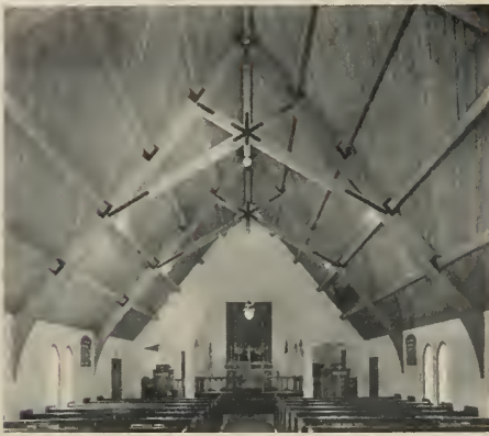
LUTHERAN CHURCH OF THE REDEEMER, Van Nuys, California. John Fleming, Architect. Interesting use of cross members & king bolt reaching to roof apex which serve to ornament the simple arches.
