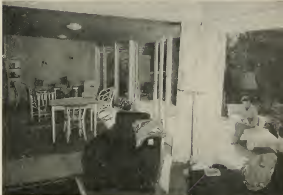
Rear wall, providing windows and doors for sunroom, living room, kitchen, study and two bedrooms. Glass doors fold for use of room and porch as sundeck.
