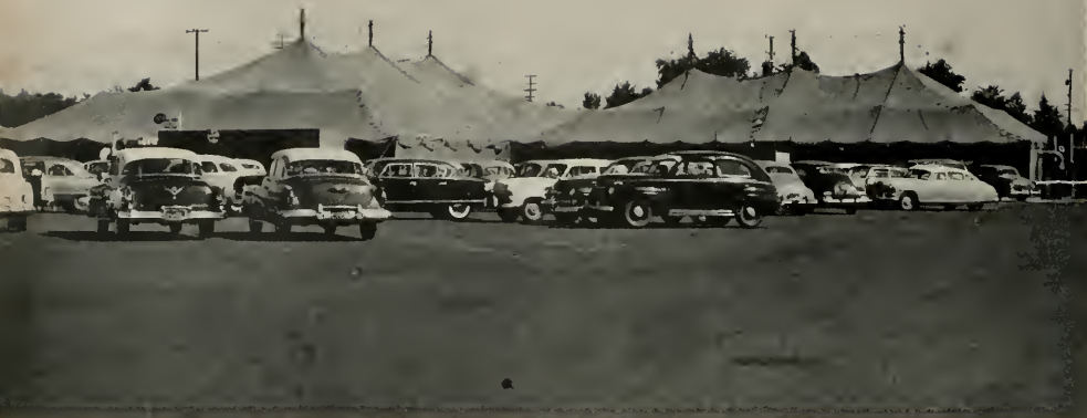
THIS IS BROCK'S DEPARTMENT STORE FOLLOWING DISASTROUS 1952 EARTHQUAKE ... Following Pictures Tell Rehabilitation Story
