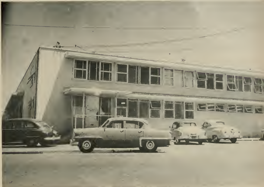
COMMERCIAL—Among commercial type buildings constructed is the warehouse for the Redwood Wholesale Grocery Company at Redwood City.
