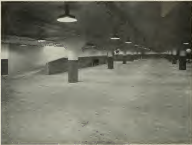
Entrance to Lower Floor
