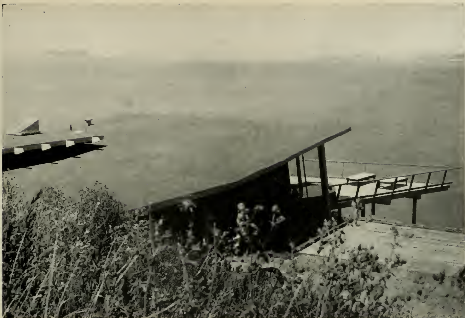
VIEW OF HOME AND PANORAMA OF BAY FROM APPROACH DRIVE
