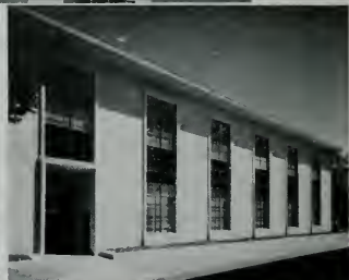
Marysville: Ariston steel sash, stainless steel entrance and door, steel stair rail.
