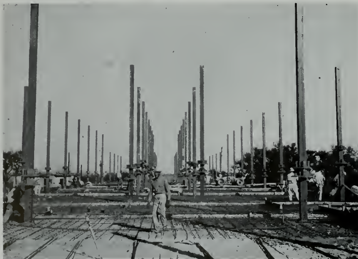
◀ Hydraulic Lifting Unit atop steel column.
