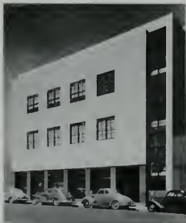
Watsonville: Ariston steel sash with stainless steel trim on ground floor and stair well, and stainless steel doors and entrance.
