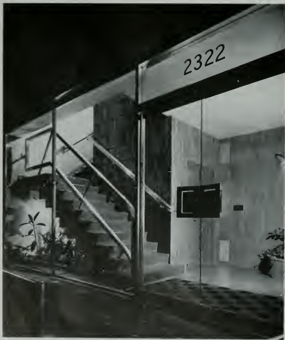
Main portal detail showing veneer application of Roman brick laid vertically with stacked joints to give illusion of greater expanse. Stairway and floor are terrazzo finished. Area is enclosed in 9 ft. high plate glass panels inset with double glass doors.
