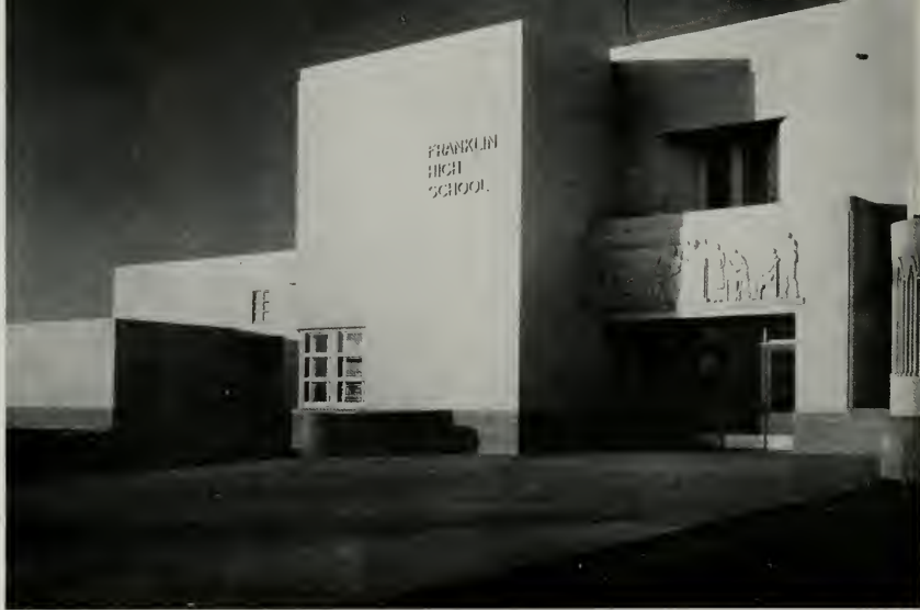
DETAIL of the new $2,500,000 Franklin High School at Stockton which represents one of the largest high schools in the nation.
