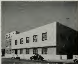
Richmond: Ariston bronze entrance and doors, miscellaneous steel and steel stairs.
