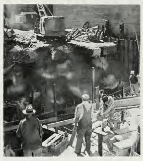
Moke-Ready-Steel mat reintorcing in toreground ... Foundations of old five story building may be seen in center bock around steel sheet piling to left and right.
