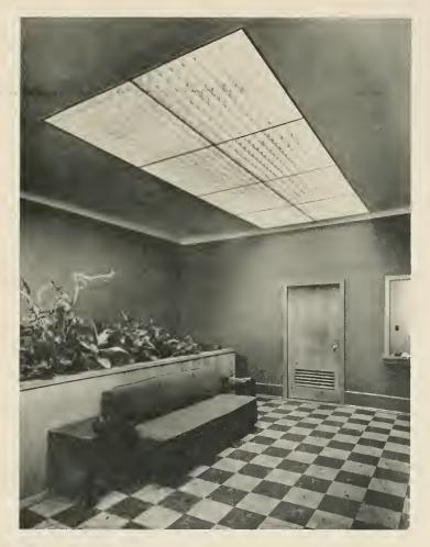
AFTER—The entire skylight area is hidden behind panel of aluminum louvered grid section set flush with ceiling. Satin finish aluminum distributes light evenly, eliminating shadaws and glare.
