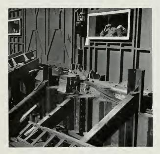
HEAVY timber shoring of steel sheet piling is blacked against chip angles . . . note the interlocking piling is burned off even at top.
