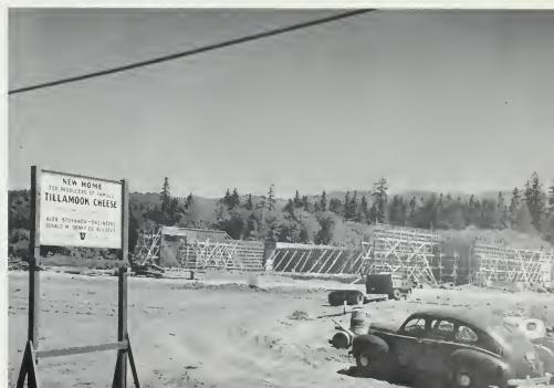
CONSTRUCTION progresses ropidly with foundations in place and concrete forms, with reinforcing steel, in place for pouring of concrete.
