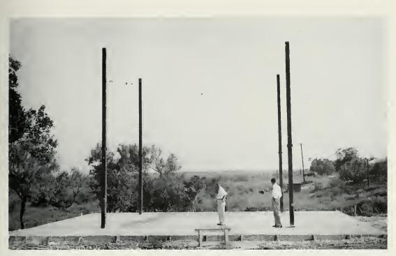
SECOND FLOOR reinforced concrete slab has been laid on top of the base slob of the experimental building being constructed by the Institute.
