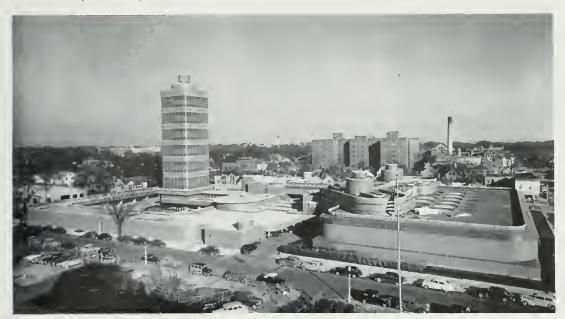
on their particular tasks, and each floor is cantilevered from the central core which is a cluster of circular, reinforced concrete shafts, and rises 156 feet above the ground and is anchored to a concrete foundation which penetrates fifty-four feet into the earth. The main or square floors are cantilevered  $21\frac{1}{2}$  feet to each corner, while the circular floors are cantilevered  $12\frac{1}{2}$  feet.
