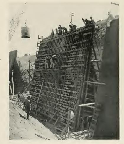
COUNTERFORT WALLS on the Los Angeles River Flood Control Channel . . . Note depth to which vibrators reach.
