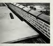
Extending 4 in. up the wall and 4 in. over the deck, they are available in lengths of 40 in. or 47 in., packaged 32 pieces to the carton. Easy to handle and cut, they are protected from attack by termites, dry ot or fungus growth.
