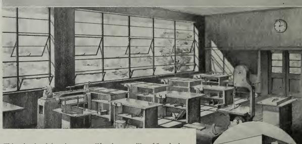
This school training shop exemplifies the versatility of Standard Fencraft Windows. It calls for abundant daylight . . . plenty of ventilation and good control of it. The use of medium size panes is recommended for easy, low-cost glass replacement. Sill vents that discourage leaning out of windows are desirable.
