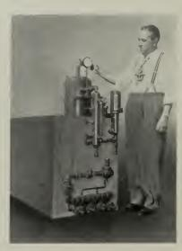
The Model "A" boilers are now available in  $3\frac{1}{2}$  h. p., 5 h. p., and  $7\frac{1}{2}$  h. p. capacities, and represent the best of Steamaster's 30 years of design and engineering experience within the small boiler field. A few of the design features are new burner shapes and two pass
