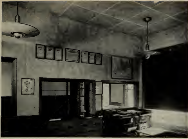
View at left: Interior of radio operations room showing Fiberglas acoustical board on walls and ceiling.
