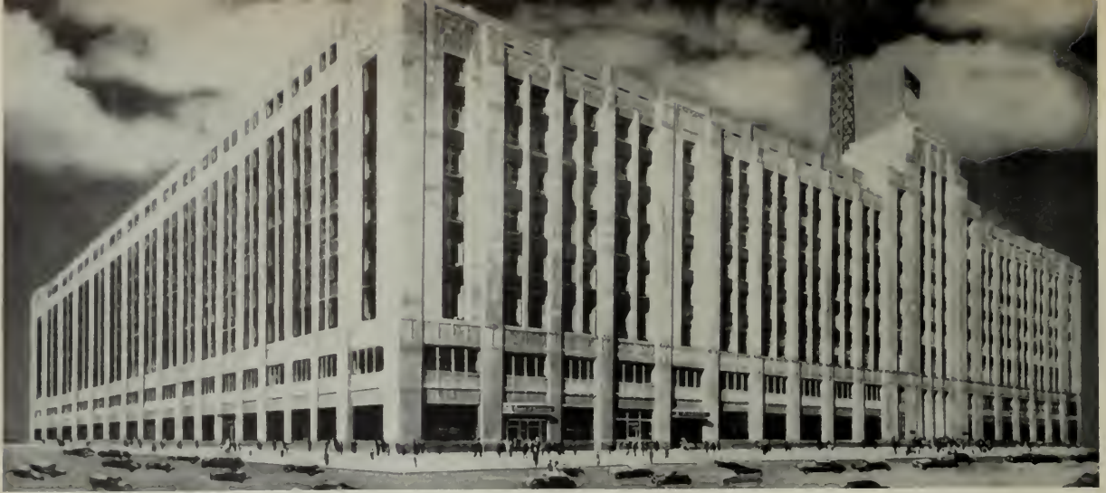
L. J. HENDY, Architect for Capitol Company
