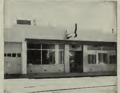
A new store front was an important part of Blewett's remodeling program (Ray Stirm, Mason Contractor, and W. C. Hoegerman, General Contractor). Salt Glazed tile was specified because of its permanent attractiveness.
