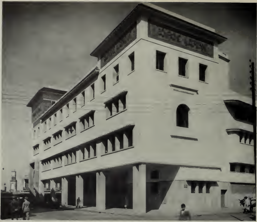
SIDE ELEVATION of the bank and office building of the Compagnie Algérienne in Casablanca, Morocco.
