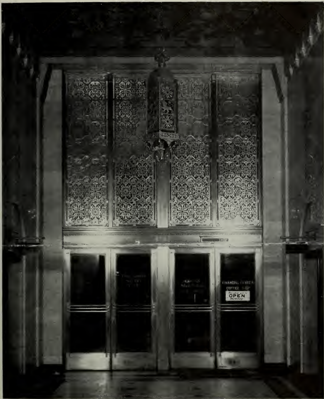
Lead overlay transom light, designed and executed for the Financial Center Building, San Francisco. An extremely rich design was achieved by the bold use of sheet lead over glass. The lights are composed of leaded glass panels in alternate squares and rectangles of octagonal shape. The sheet lead is pierced in a design of stylized leaves and heraldic animals and soldered to the main leads between the panels. The entire effect is that of a completely weatherproof and translucent grille. The leadwork is designed to harmonize with the bronze lamp and general architectural ornamentation of the foyer.
