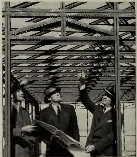
STRAN-STEEL PRE-CUT FRAMING in place. Inspecting framing for 24-foot by 36-foot home recently erected at Pittsburg demonstration are, Chas. W. Kraft, President (left), Joe Peebles, Manager, Kraftile's Stran-Steel Division, and Jim Crawford, Vice President and Sales Manager of Kraftile Company.
