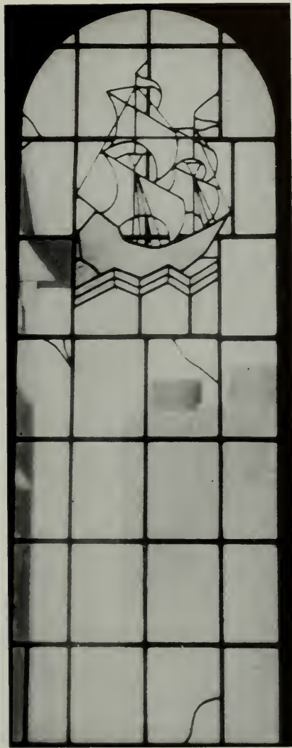
This is an example of what can be done with an unattractive window opening. The problem in this case was to treat the large area decoratively, and at the same time to admit full daylight. This has been solved with a simple design in lead and textured glass, with a few "breaks" scattered in the field to add interest. This window is in the penthouse of Mrs. Mayes, Telegraph Hill, San Francisco.
