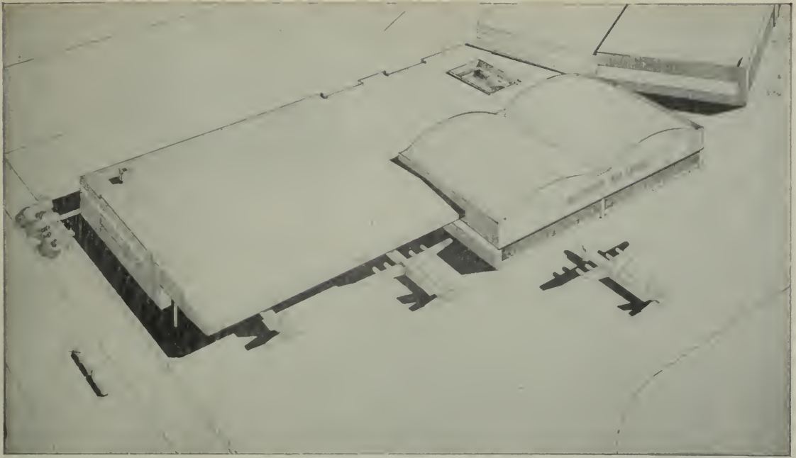
REAR ELEVATION showing airport side of two closed hangars and two nose-hangars being built by Western Air at Los Angeles at a cost of $1,500,000. Minor repairs to the luxurious DC-6's are made in the nose-hangars and overhaul jobs are done in the closed areas. Roof garden for employees is shown at top.
