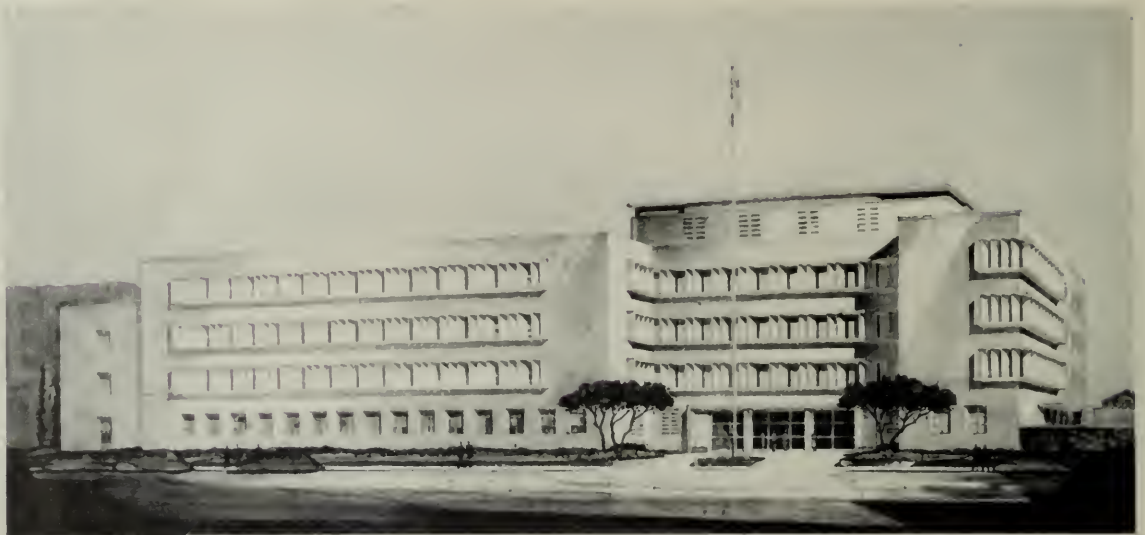
West laboratory building showing new office wing
