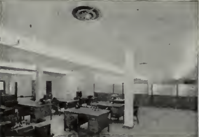
Acousti-Celotex provides quiet in these offices, Kraft Cheese Co., San Francisco
