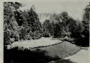
Earth Forming Stage of on outdoor theatre
