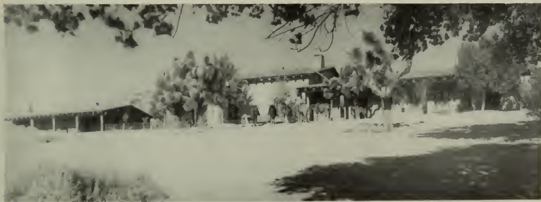
AN ADDITIONAL adobe unit now joins the two buildings shown here
