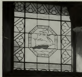
Light over entrance to Bank of America, Napa branch. In this example the ship emblem, background and borders are all executed in textured glasses in simple modern lines, designed to admit full daylight but to diffuse harsh glare.
