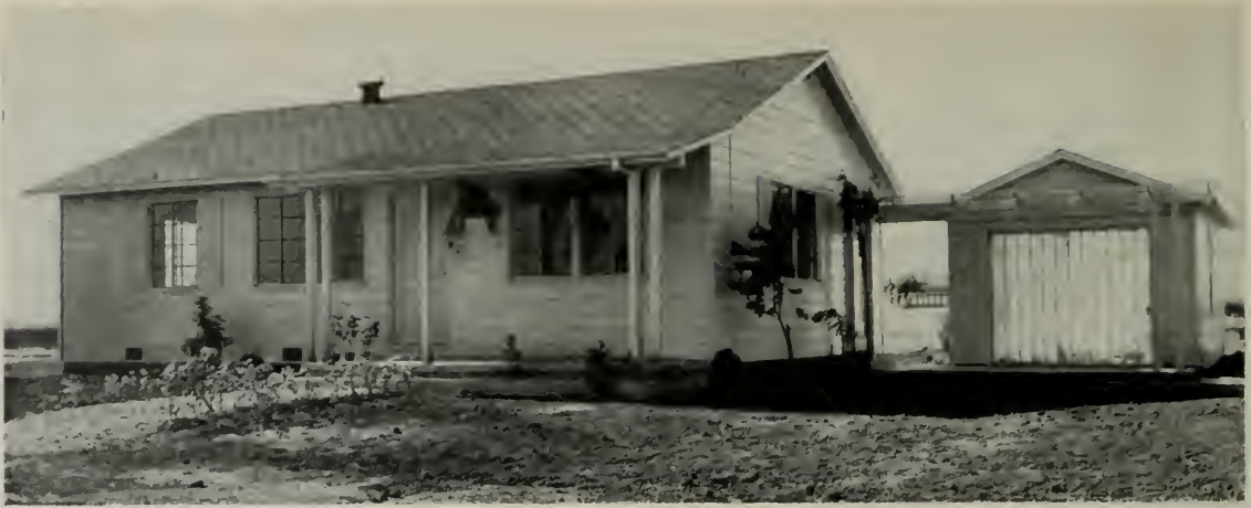
"KRAFTILE" PACKAGED STEEL FRAME HOME COMPLETED
