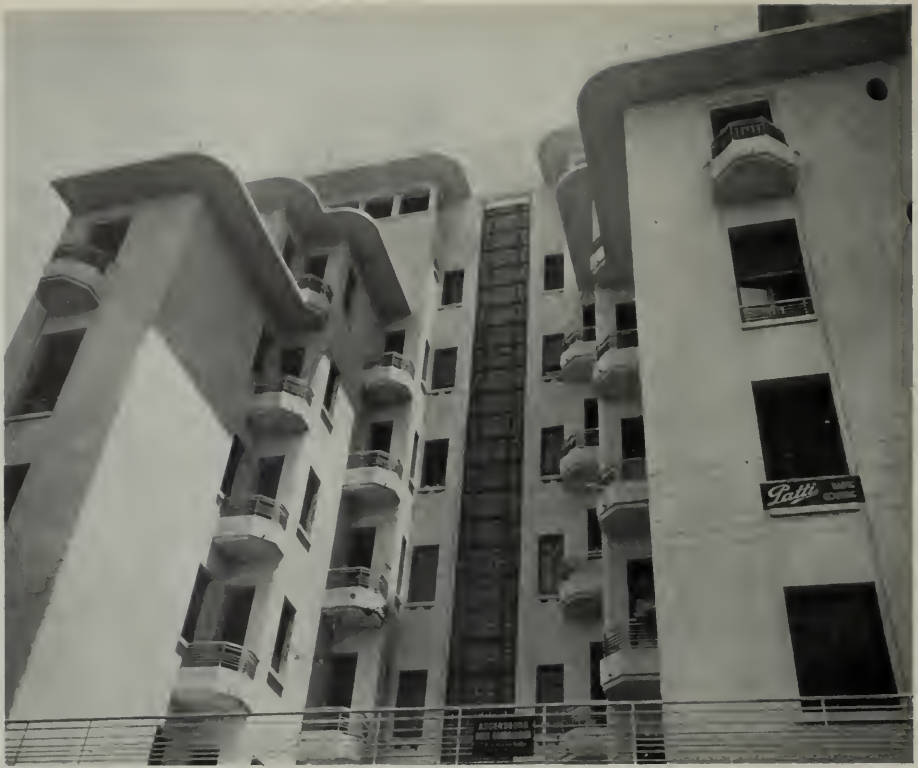
Above: A lovely Tunisian Apartment House. View is a side elevation showing vertical setbacks in the court which permit ample light to enter. Note the wrought iron grille in elevator shaft, and welded steel rail in the foreground.
