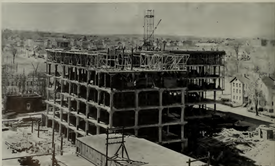
LOWER VIEW shows the new six-story building of the STANLEY Company which is being constructed of concrete and brick to house the Stanley Electric Tool Division.
