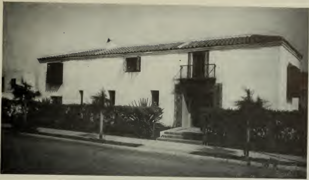
ABOVE: Street view of the Louis Bradbury adobe house. Note lateral roof ridges which divide rather yellow field tiles into panels. Raised ridges are of gun metal for contrast.
