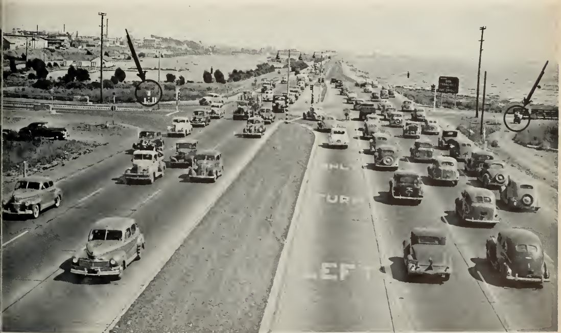
MATIC HIGHWAY CROSSING SIGNAL at intersection on East Shore Highway (left circle) between Oakland and Richmond. More than 45,000 vehicles per day are governed by this electric monitor. Note Highway Patrolman at right (in circle) governing flow of traffic. (Photo California Highways & Public Works.)
