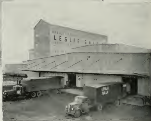
Leslie Salt Company, Newark, California, a recent Corrugated Transite installation by Western Asbestos Co.
