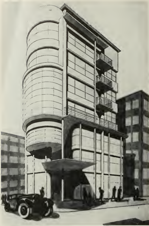
Department Store Project in Algiers. The building is of concrete with exterior in heat resisting glass.
