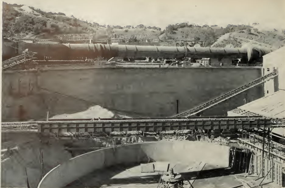
Above: Retaining Wall 3rd Kiln, Permanente
