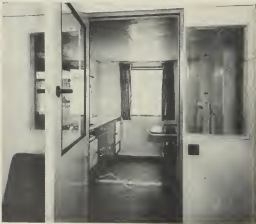
Interior of a British emergency prefabricated "Portal" house. Kitchen and bathroom appliances, with dividing wall, are turned out as a single unit. Illustration shows kitchen viewed from the living-room, with refrigerator, sink, and gas cooker. British Official Photo
