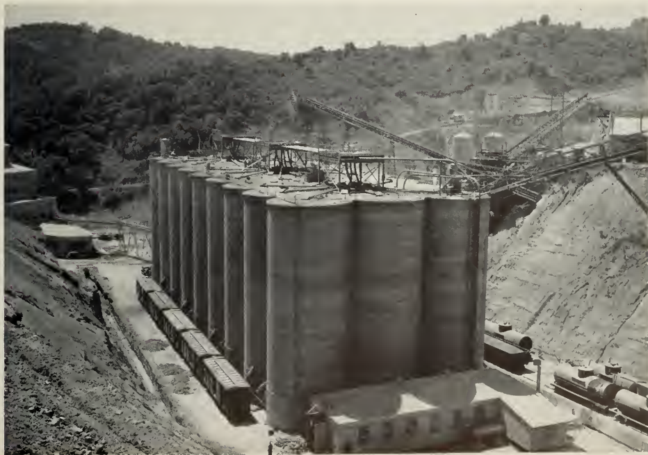
BATTERY OF CEMENT SILOS AT PERMANENTE
