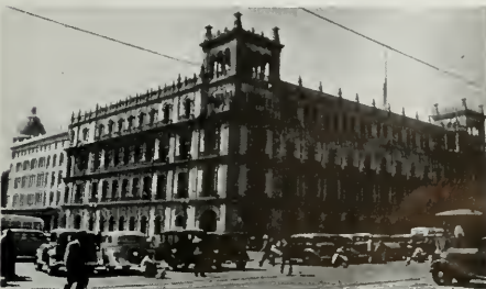
City Hall in Mexico City, D.F.
