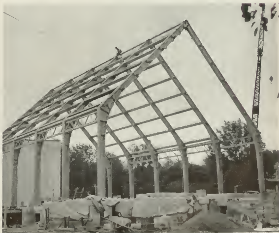
WELDED free standing framework of Church structure showing unusually high pitch of roof design.
