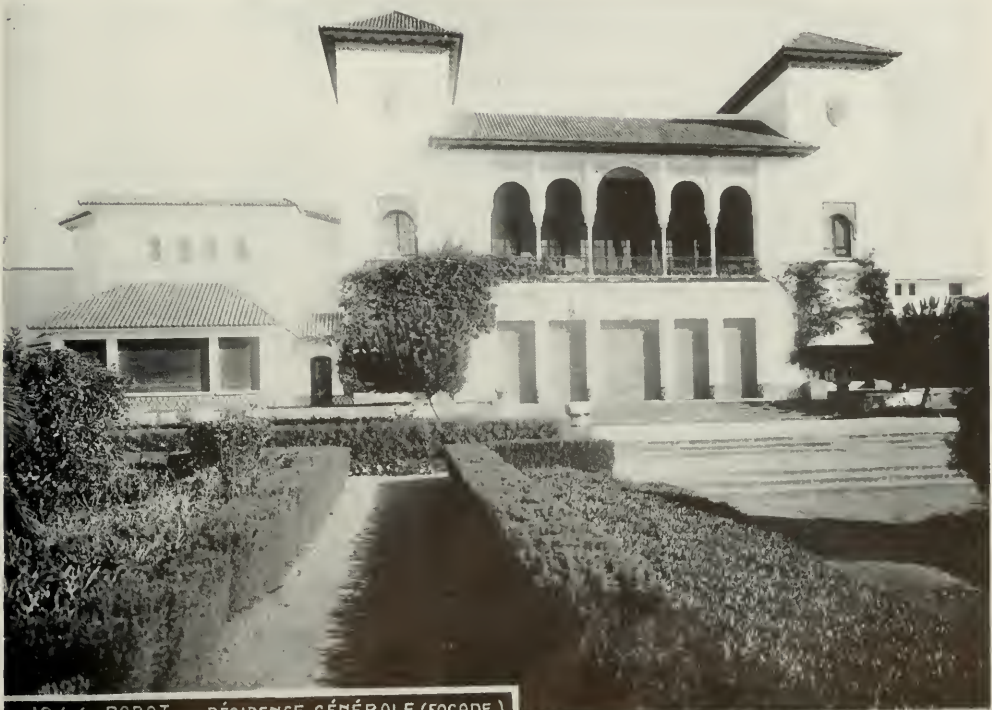
Residence of the Governor General of Morocco at Rabat—note the cast grilles and rolling-wood blinds at the left and center, ground floor. The roof is of green glazed tile, while the base is formed of faïence mosaic. The two odd shaped blocks by the garden steps are old Moorish column caps. All details of this building are typically Moroccan.
