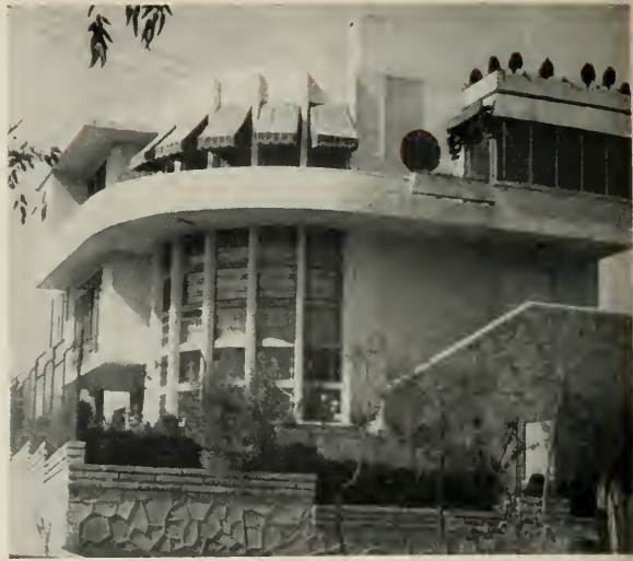
LOWER: Details of the Artistic Modern Mexico Casa of which Ramon Carlos Aguayo was the Architect. Basement, First and Second Floor Plans Shown.
