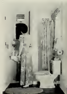
Complete Standard Size Fixture Bathroom
