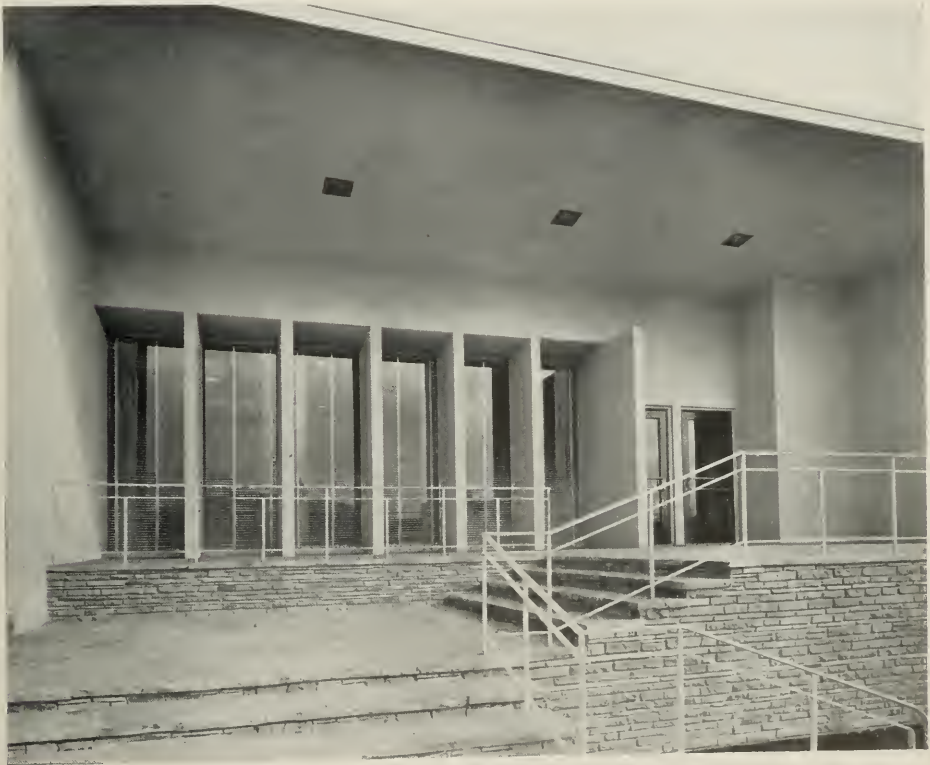
FLAGSTONE STEPS and Porch of MacArthur Boulevard Entrance to Kaiser's Permanente Foundation Hospital at Oakland, California
