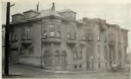
Prior to conversion . . . old, outdated.
