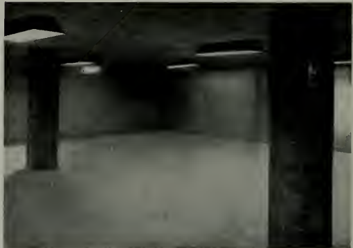
Above: Employees' Locker Room (before locker installation). Partitions for personnel rooms and offices, employees' dressing rooms and lunch room are 6" x 12" Kraftile "Salt-Glazed" Structural Units, 4" thick with vertical cellular construction reinforced with cement grout where necessary. Partitions are glazed from floor to ceiling
