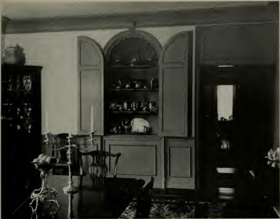
COE RESIDENCE ALTERATION—1939—DINING ROOM An extraordinary commission wherein the owners had complete furnishings of rare and valuable Georgian antiques V.G. fir wainscot and trim painted Williamsburg lead-blue; maple floors stained black; plaster walls oyster white.
