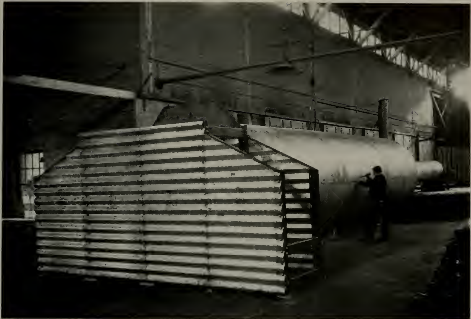
This Armo iron air-raid shelter is 50 ft. long and 7½ ft. high and will accommodate 50 persons. Four unskilled workmen can erect the shelter with simple tools in a few hours.
