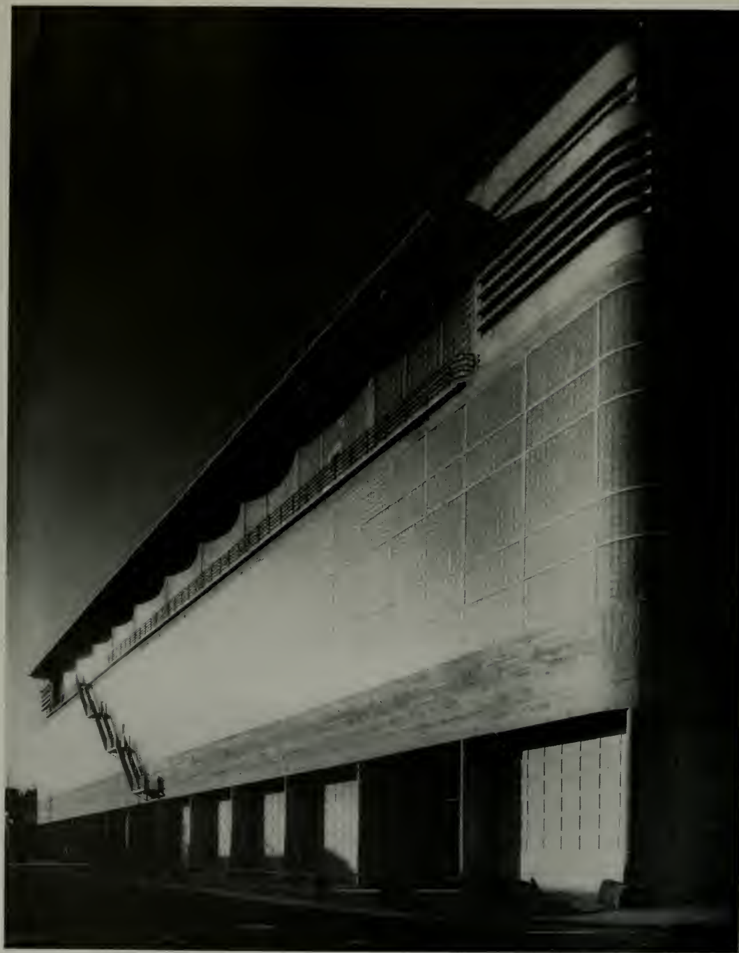
BOTTLING PLANT FOR ACME BREWERIES, SAN FRANCISCO, CALIFORNIA William G. Merchant, Architect
