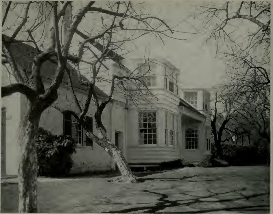
NEU RESIDENCE, PORTLAND, OREGON—1930 TERRACE SIDE
