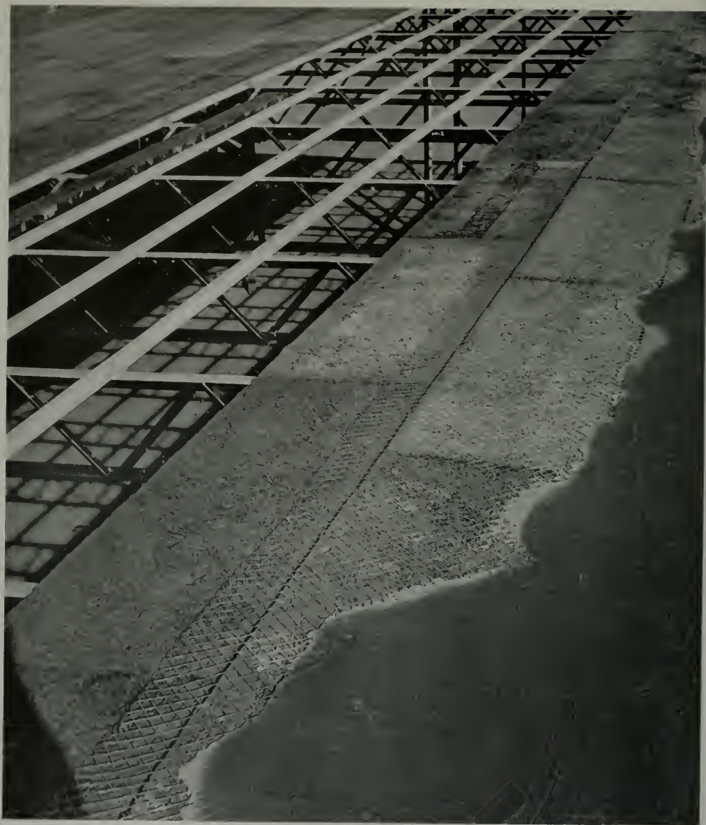
ROOF CONSTRUCTION OF INDUSTRIAL PLANT, SHOWING STEEL, THERMAX, WIRE AND CEMENT TOPPING
