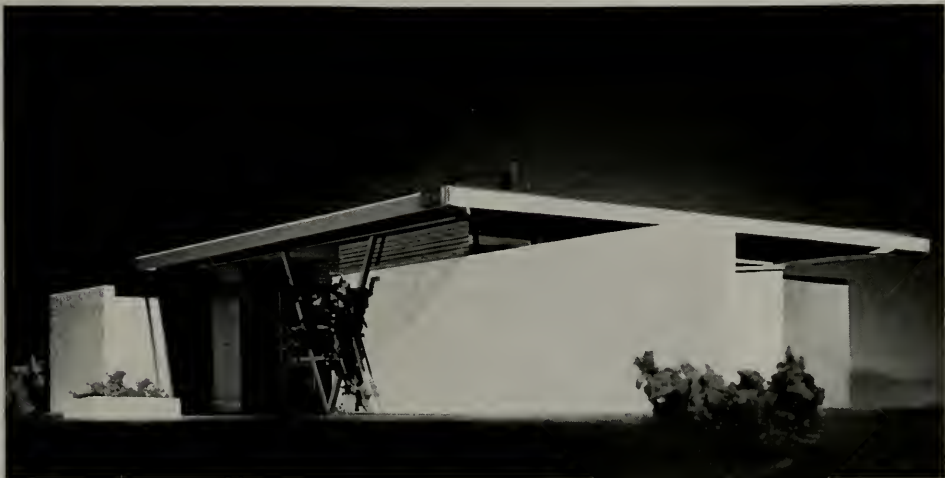
THE "V" HOUSE, WITH ITS GRACIOUS ENTRANCE AND PRIVATE PATIO. ITS MASSIVE WALLS ARE GROUPED FOR PRIVACY AND RELATIVE PROTECTION AGAINST BOMB FRAGMENTS AND FIRE
