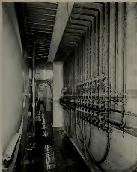
The gleaming Kraffled Government Celler where Acme beer awaits bottling in large one-piece, glass lined tanks
