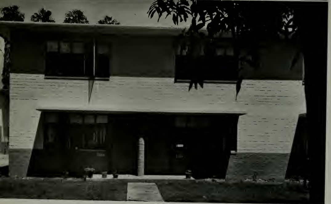
Close up of a twin apartment unit showing wide overhang flat roof and hooded entrances, the latter formed by a cantilevered extension of the second floor slab
