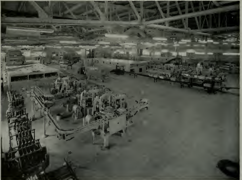
MACHINERY HALL, THE FIFTH FLOOR OF THE NEW BOTTLING PLANT, WHERE ALL BOTTLING, LABELING AND PACKAGING OPERATIONS ARE CONCENTRATED
