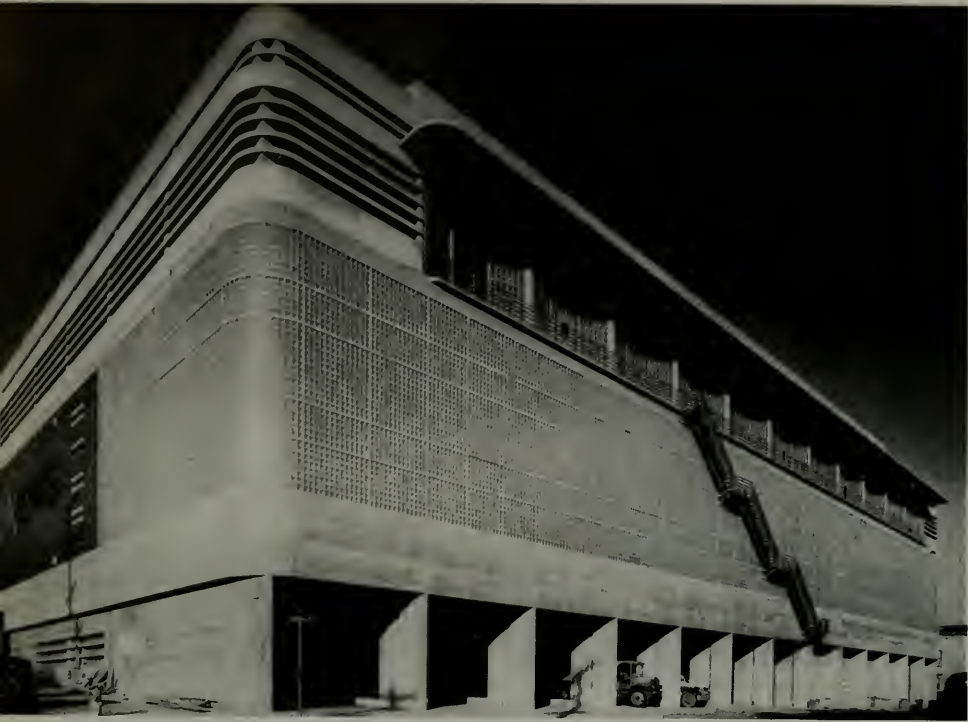
RIBBONS OF GLASS BLOCKS DOMINATE THREE FACADES OF ACME BOTTLING PLANT, SAN FRANCISCO
