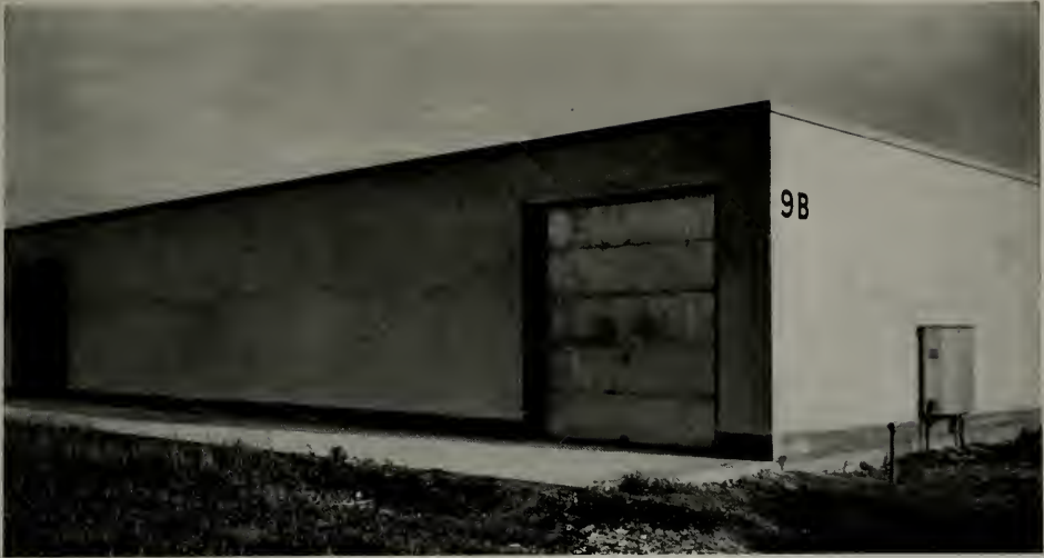
TYPICAL BUILDING OF INDUSTRIAL GROUP
