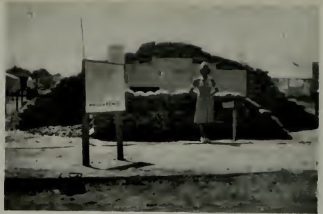
CALIFORNIA ARCHITECTS' AIR RAID SHELTER AT STATE FAIR
