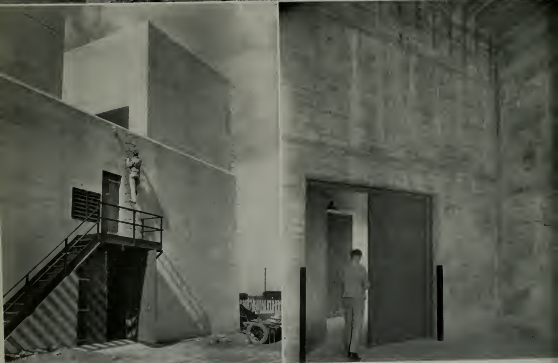
(Top) Exterior view of test stand building. Inlet stacks for the four test cells are on the corners of the structure; outlet stacks in the center each serve two test cells. (Above—left) Exterior view of inlet stacks. (Above—right) Interior view of test cell, showing height from the cell floor that sound-absorbing baffles of Fiberglas pads are installed in an inlet stack.
