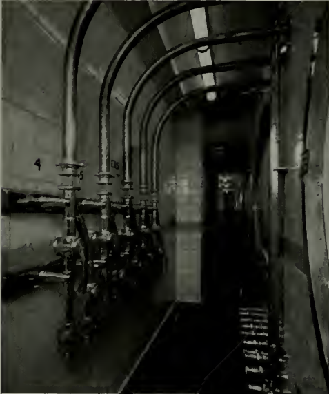
Government Celler contains four 100-barrel and eleven 250-barrel glass lined tanks. The Wall Units are Kraftile Ceramic Glazed, Cellular, they are ideal for a refrigerated room like this. Kraftile Vitreous 8 x 8 Quarry Tile is used to finish the floor here, in the Meter Room, and the entire working area of Machinery Hall. 13,300 square feet were used—the largest quarry tile installation in San Francisco last year
