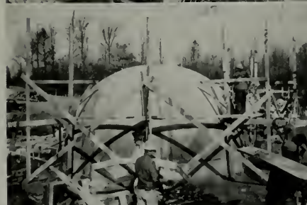
Construction methods: Pictured from top down—(1) Laying out the balloon form; (2) Method of anchoring; (3) Inflating canvas with compressed air; (4) Mounting window frames and dusting balloon so cement won't stick to it.
