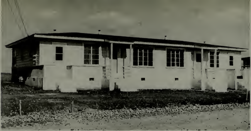
One of the completed two family dwellings
