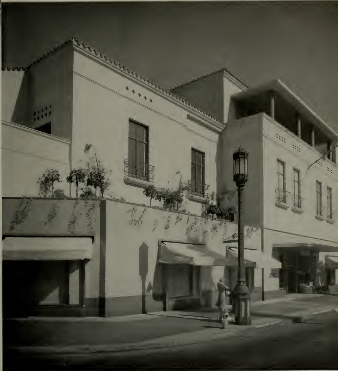
AT LEFT—PERINO'S RESTAURANT, LOS ANGELES, CALIFORNIA. J. R. DAVIDSON, ARCHITECT. FINISHED WITH ADHESION TYPE CERAMIC VENEER, IN FLESH AND WARM BUFF, WITH BASE OF HAND-MADE BLACK WITH GOLD LUSTER.
