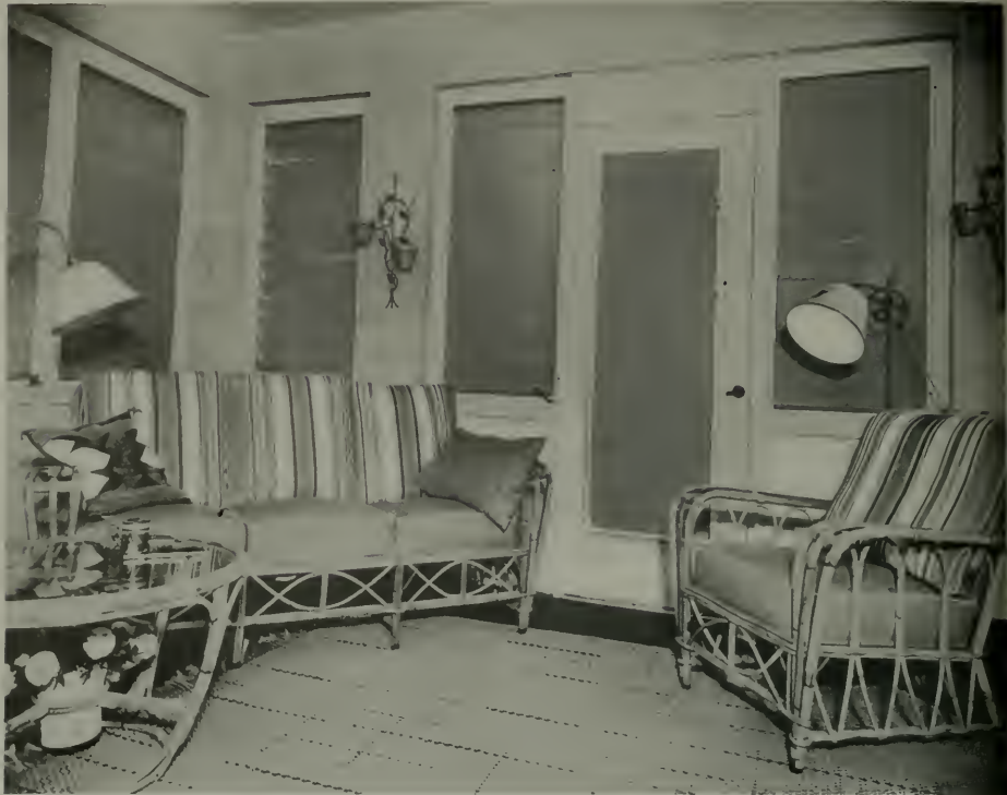
Porch equipped with all-metal jalousies, providing adequate shade and complete inside control of ventilation, visibility and sunlight.
