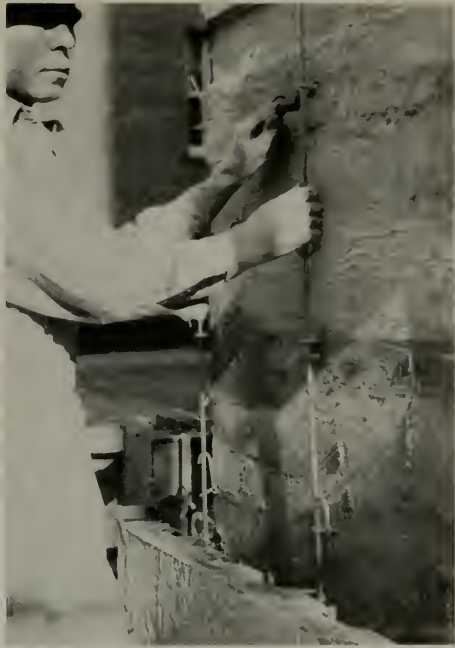
SETTING THE ANCHORED TYPE OF CERAMIC VENEER. NOTE SPACE BETWEEN ANCHOR ROD AND CONCRETE. BELOW, A UNIT SET IN PLACE, READY FOR TIEING AND GROUTING.
