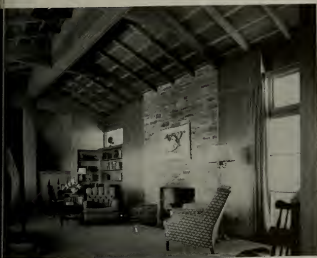
LIVING ROOM is paneled in Philippine mahogany with redwood and pine ceiling. Note gusset roof construction in place of customary trusses.
