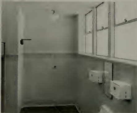
Entrance corner of girls' toilet room, Ross Grammar School. Particularly attractive is the tile coloring, the field being Kraftile's Monterey Buff, a delicate shade, with a bull-nose capping and sanitary cove base of Kraftile's Seafoam Green. Architect: Carl Gromme; general contractor, Carico & Gautier; tile contractor, Donlon Tile Company.
