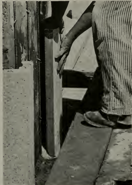
SETTING THE ANCHORED TYPE OF CERAMIC VENEER. NOTE SPACE BETWEEN ANCHOR ROD AND CONCRETE. BELOW, A UNIT SET IN PLACE, READY FOR TIEING AND GROUTING.
