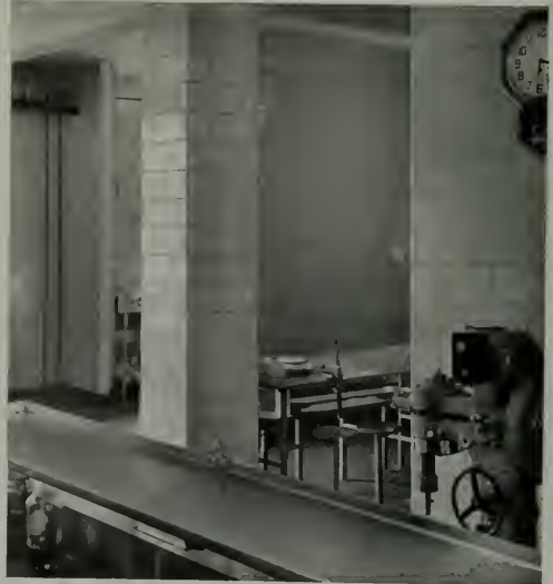
Ceramic Glazed Wall Units (Unsize) are widely used in industrial plants and commercial structures where beauty as well as utility is important. Laid with a nominal \frac{1}{4} -in. joint. Triple-glazed surfaces available in a variety of colors—bright, mat, mottled or clay-coated.
