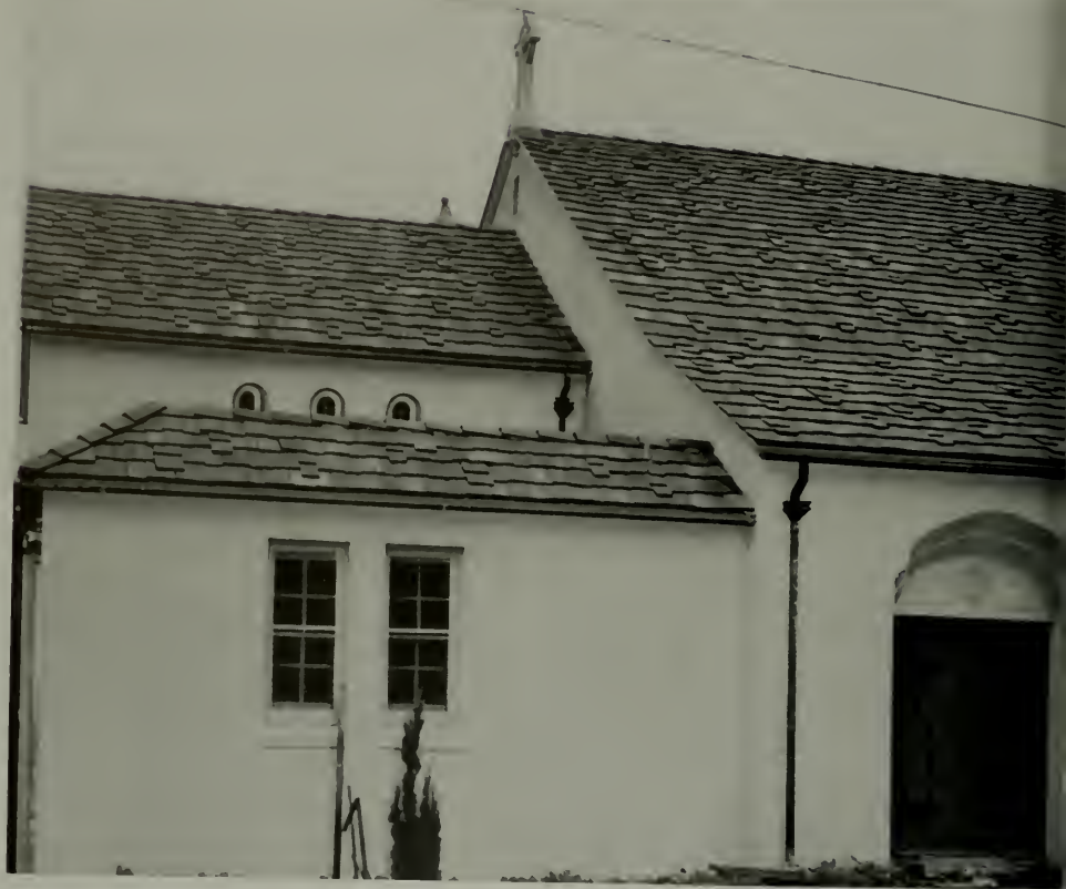
SHINGLE TILE ROOF, ST. PATRICK'S CHURCH, LARKSPUR, CALIFORNIA
