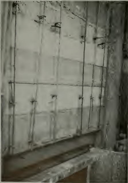
SETTING THE ANCHORED TYPE OF CERAMIC VENEER. THE PICTURES ABOVE AND BELOW SHOW THE ANCHOR RODS HELD OUT FROM THE CONCRETE STRUCTURE BY BENDING PROJECTING END OF ANCHOR BEHIND ROD.
