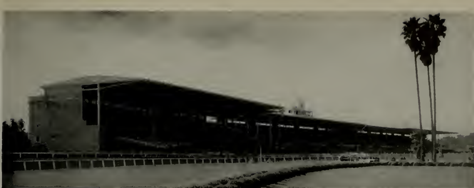
GENERAL VIEW OF SANTA ANITA RACE TRACK, SANTA ANITA PARK, CALIFORNIA. CLUBHOUSE GRANDSTAND IN FOREGROUND
