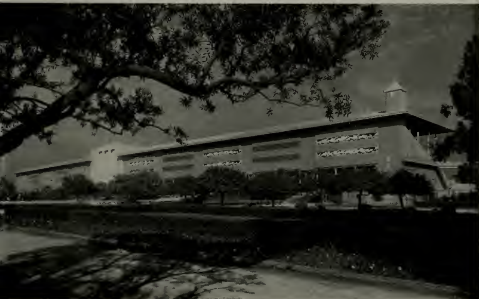
ENTRANCE FRONT TO GRANDSTAND, SANTA ANITA RACE TRACK Gordon B. Kaufmann, Architect
