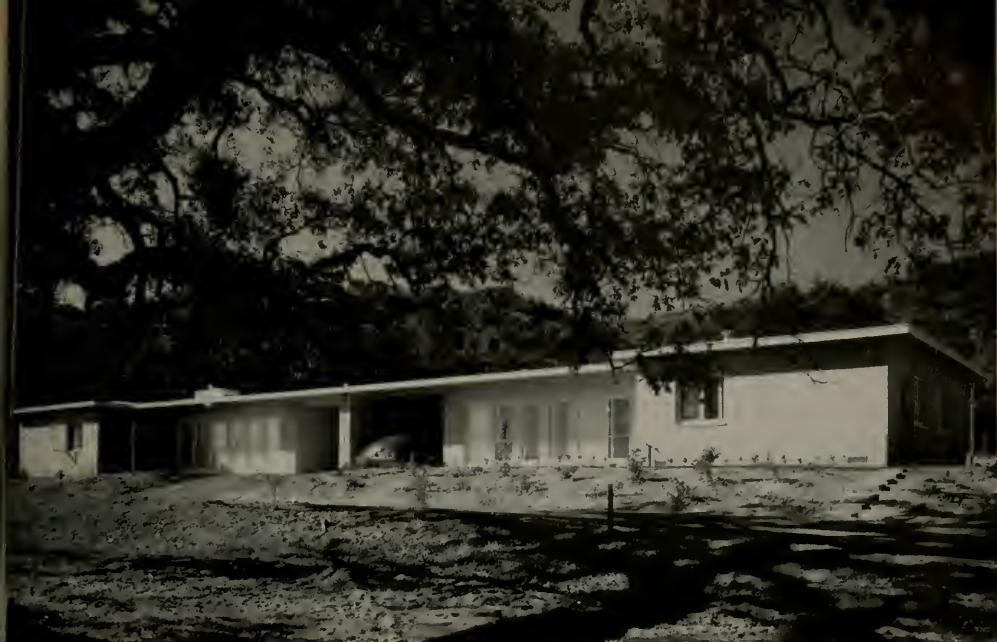
General Construction by C. M. Tieglund
