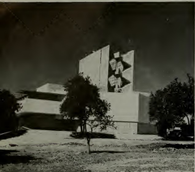
Shrine for Florida Southern College, Lakeland. Dominating the mass is a 63 ft. tower of poured concrete on two sides with three concrete "bow ties" at either end to provide flower boxes. The tower supports 18 bronze gongs shaped like jingle bells. A rigid skylight at the level of the third deck protects the auditorium (pictured below) since there is no roof over the tower. Note diamond shape block construction in auditorium.
