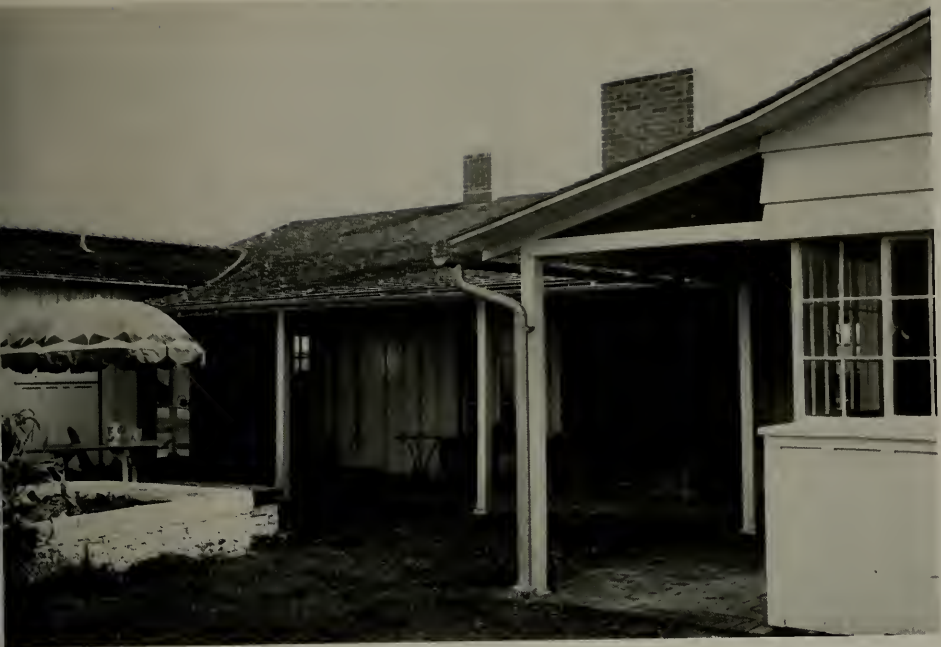
RANCH HOUSE FOR MR. AND MRS. JOHN P. McNEIL, ATHERTON, CALIFORNIA Wallace H. Hubbert, Architect
