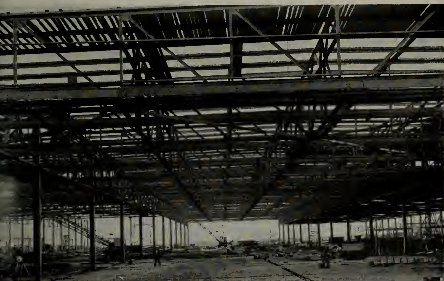
Steel frame of one of the huge assembly buildings under construction for the Douglas Aircraft Company, Inc., at North Long Beach, California. Outside bays are 30 feet and are increased to 60 feet on the inside to provide clear assembly areas.
