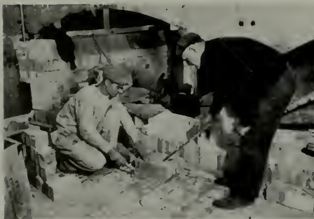
Apprentice of Birmingham plant of the Tennessee Coal, Iron and Railroad Company, learning how to lay brick.
