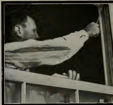
SHOWING EASE WITH WHICH WINDOW IS BALANCED
