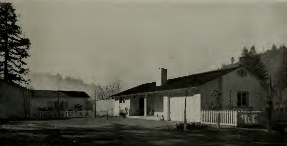
houses in Redwood City; designed for vacation use but adequate for all year living. Blanchard and Maher, Architects
