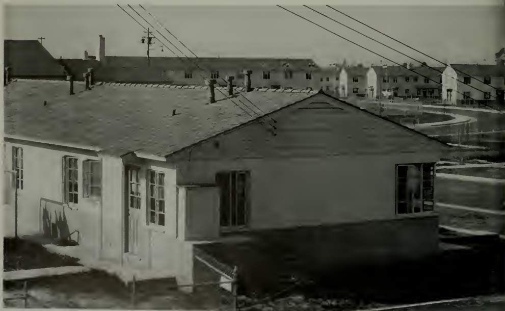
A DETAIL OF THE SAME. ARTHUR SCHILLING WAS CHIEF ENGINEER; CLARENCE STEIN, HOUSING CONSULTANT; RALPH D. CONNELL, LANDSCAPE ARCHITECT.
