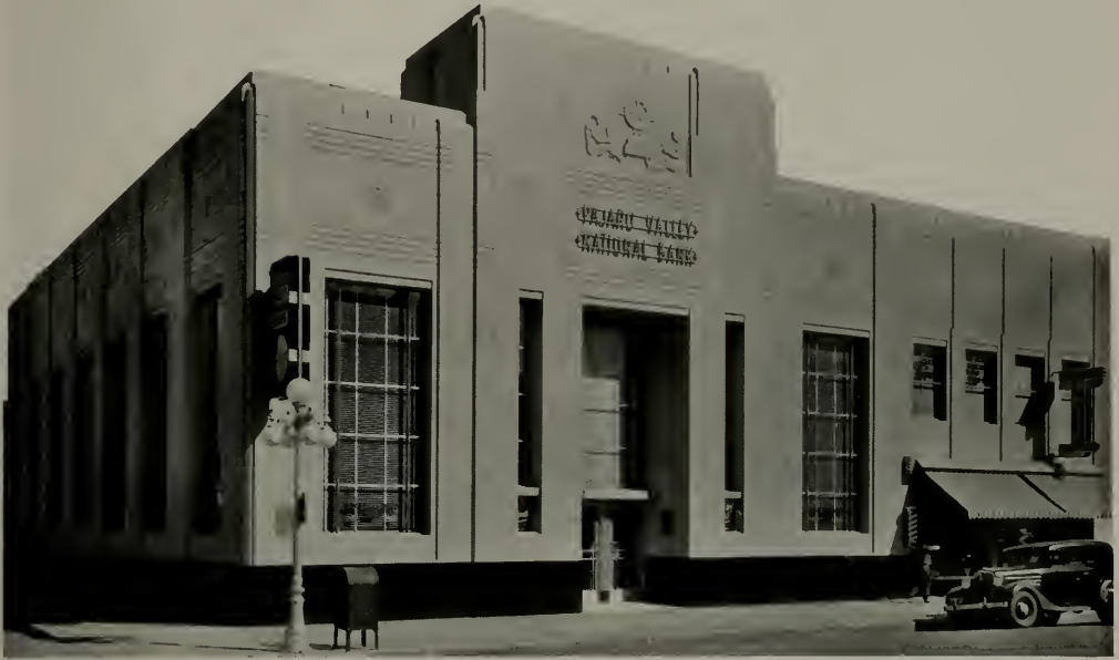
N. Clark & Sons' Adhesion Type Ceramic Veneer was chosen by Architect H. H. Winner in the execution of the new Pajaro Valley National Bank at Watsonville, California.
