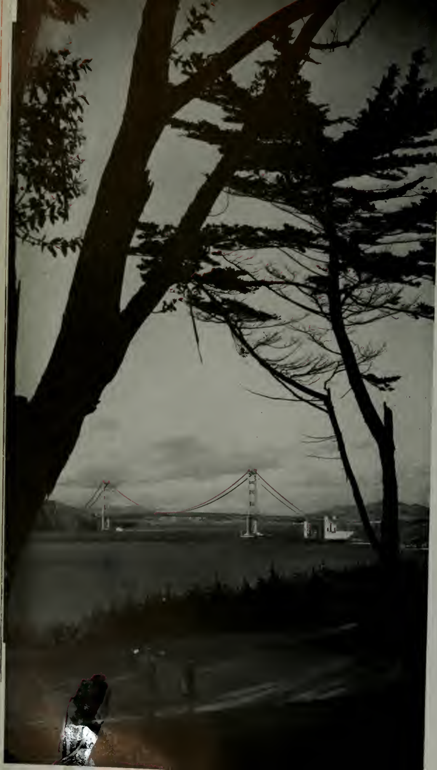
STRIKING VIEW OF THE GOLDEN GATE BRIDGE TAKEN FROM LINCOLN PARK GOLF COURSE. THE 4200 FOOT SPAN IS THE LARGEST BRIDGE SPAN IN THE WORLD.
