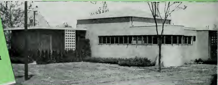
Don't miss seeing this beautiful Plywood House if you visit the New York World's Fair. Send for free manual which tells about Dri-Bilt with Plywood construction.
