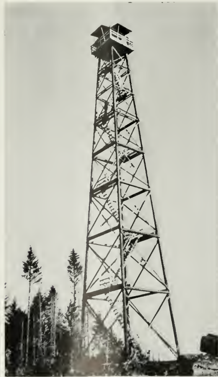
TYPICAL FOREST FIREMAN'S LOOKOUT TOWER. ORIGINALLY THESE WERE BUILT OF STEEL; LATER A STANDARD TIMBER DESIGN WAS ADOPTED
