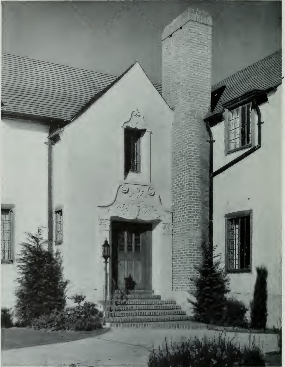
ENTRANCE DETAIL, RESIDENCE OF WILLIAM JENKINS, SEATTLE, WASHINGTON Roi L. Morin, Architect
