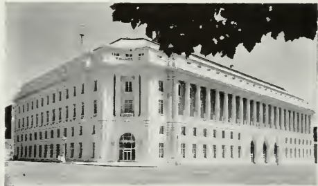
FEDERAL BUILDING • CIVIC CENTER • SAN FRANCISCO
