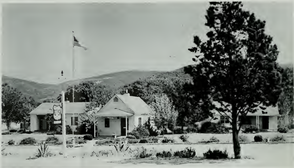
DISTRICT RANGERS' HEADQUARTERS, ANGELES NATIONAL FOREST, NEWHALL, CALIFORNIA Group consists of 2-Room Office, Guard Dwelling, Ranger Dwelling and Fire Crew Barracks.
