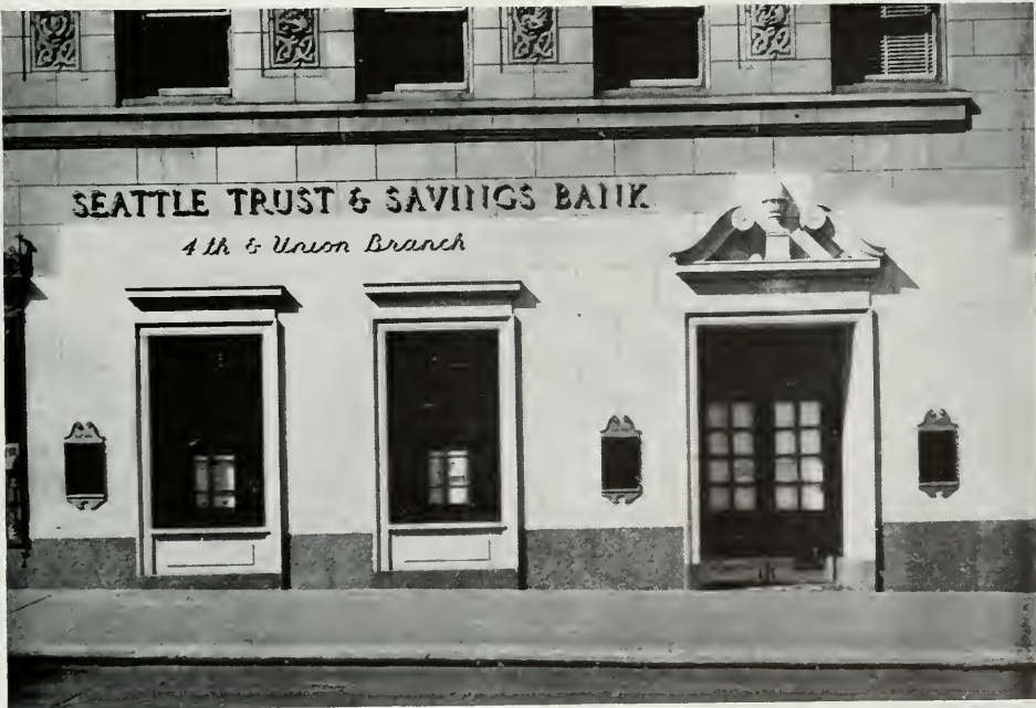
SEATTLE TRUST & SAVINGS BANK, SEATTLE, WASHINGTON McClelland & Jones, Architects
