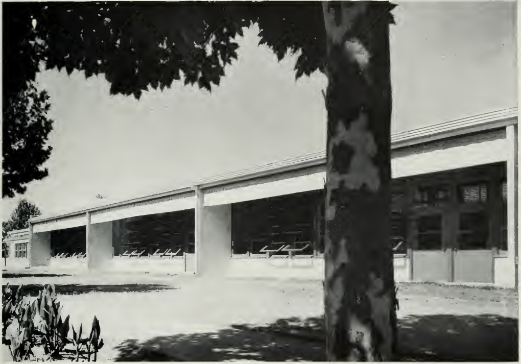
FOWLER ELEMENTARY SCHOOL, FOWLER, CALIFORNIA Chas. H. Franklin and Ernest J. Kump, Jr., Architects
