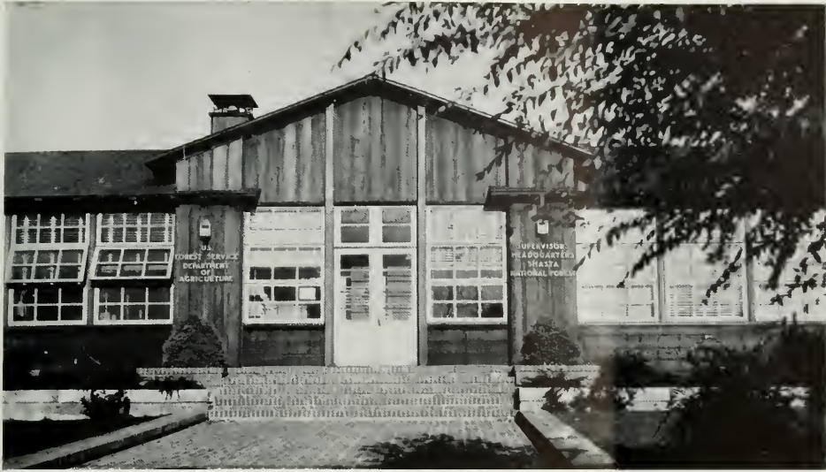
ENTRANCE DETAIL, SUPERVISOR'S OFFICE, NATIONAL FOREST, MT. SHASTA CITY, CALIFORNIA
