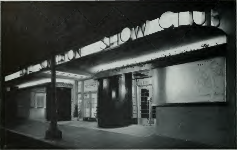
NIGHT VIEW OF SHOW CLUB, HOTEL SOMERTON, SAN FRANCISCO Williams & Grimes, Albert R. Williams, Architect Indirect Neon lighting
