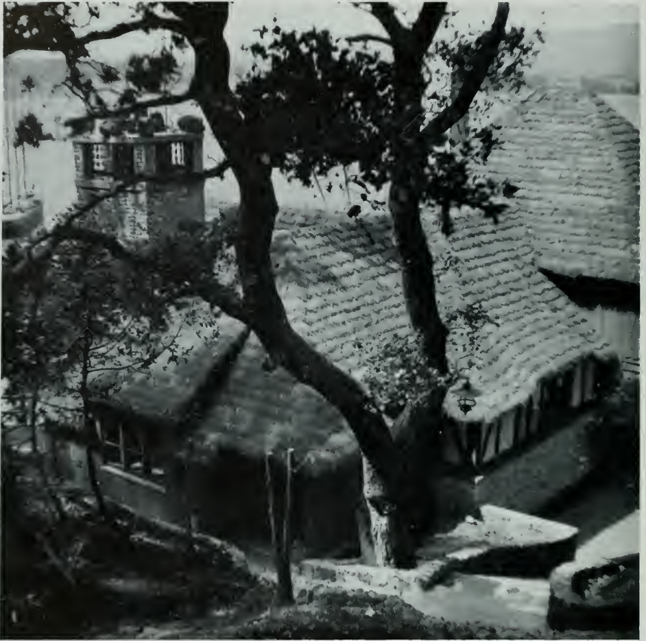
A STUDY IN THATCHED ROOF, HOUSE FOR MR. AND MRS. CARL W. REBMANN, BELVEDERE ISLAND, CALIFORNIA
