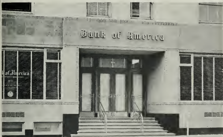
Entrance detail, faced with N. CLARK & SONS CERAMIC VENEER. Also showing use of Alameda Quarry Tile for stair treads and risers.
