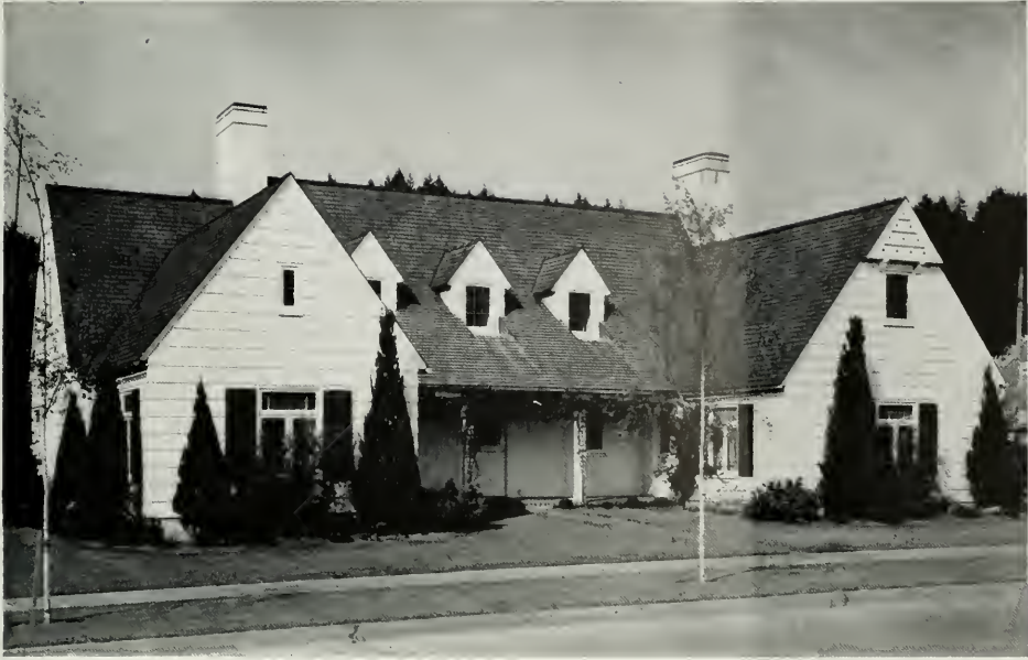
RESIDENCE OF G. L. DRAKE, SHELTON, WASHINGTON George W. Stoddard, Architect Double coursed shingle side-walls
