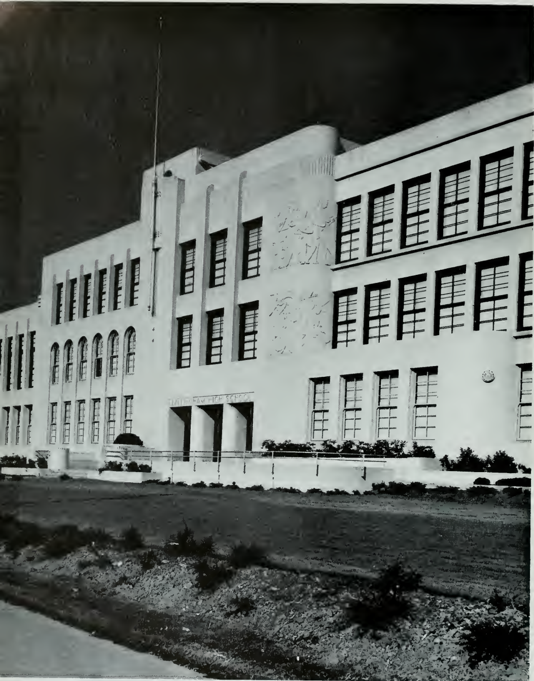
BELLINGHAM HIGH SCHOOL, BELLINGHAM, WASHINGTON F. A. NARAMORE, ARCHITECT
