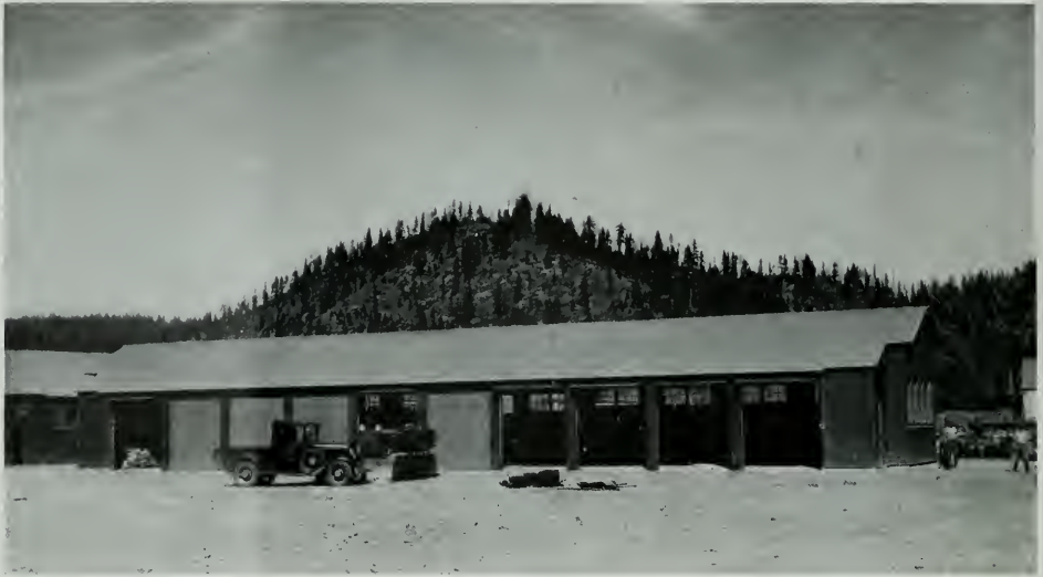
STANDARD 10-STALL 26-FT. SPAN GARAGE, PLUMAS NATIONAL FOREST, QUINCY
