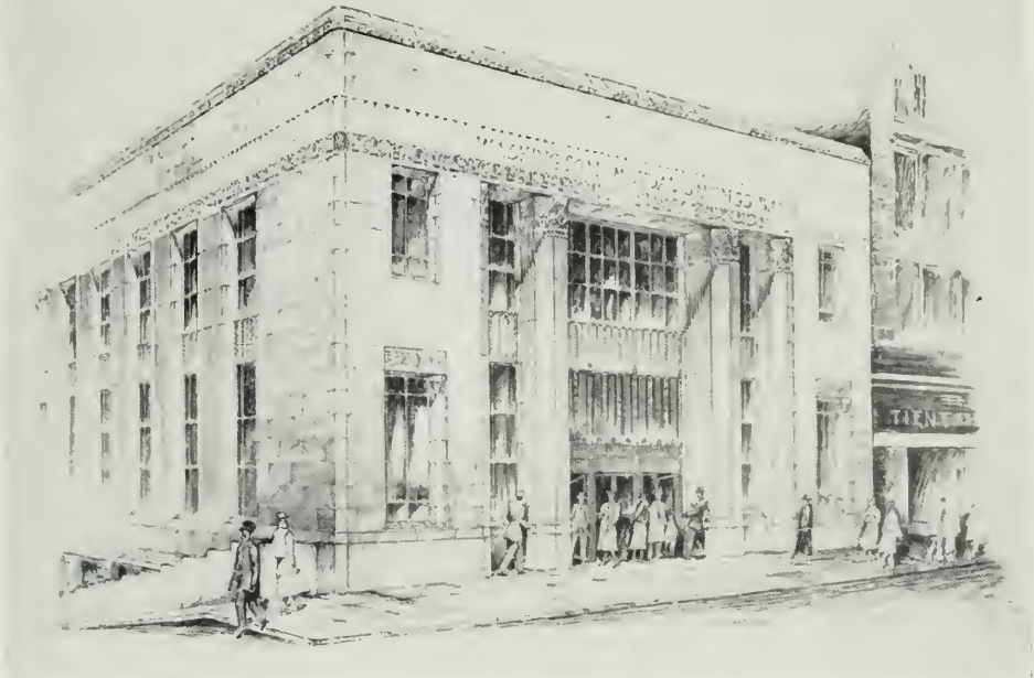
WASHINGTON MUTUAL SAVINGS BANK, SEATTLE C. A. Merriam, Architect
