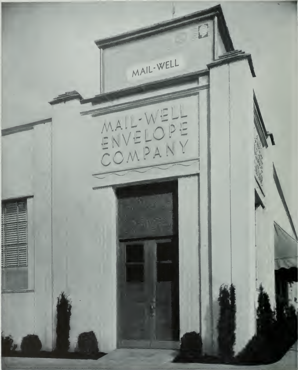
DETAIL OF ENTRANCE, MAIL-WELL ENVELOPE COMPANY, PORTLAND Richard Sundeleaf, Architect
