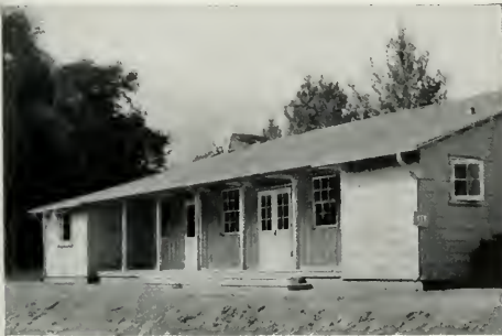
MESS HALL, CALIFORNIA F. & R. EXPERIMENT STATION, ANGELES NATIONAL FOREST
