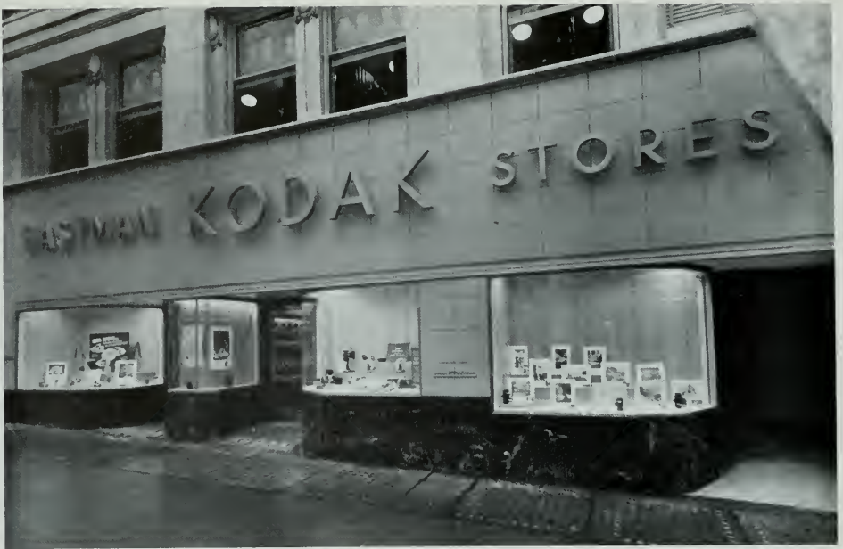
EASTMAN KODAK STORES, SEATTLE, WASHINGTON McClelland & Jones, Architects
