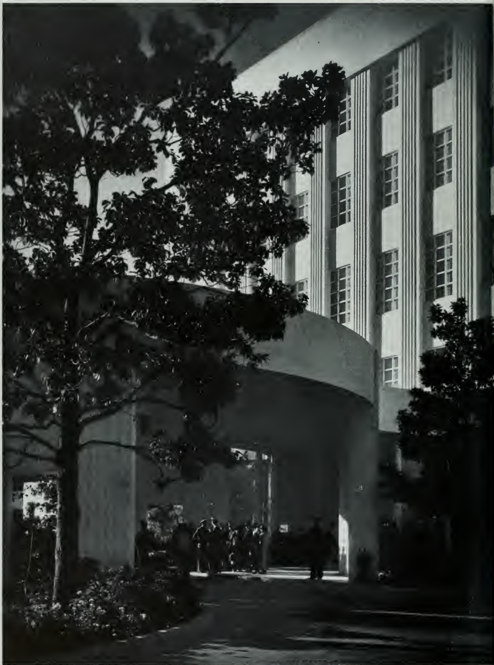
STORE BUILDING FOR I. MAGNIN & COMPANY, LOS ANGELES, CALIFORNIA Hunt & Chambers, Architects; T. L. Pflueger, Architect of Interior
