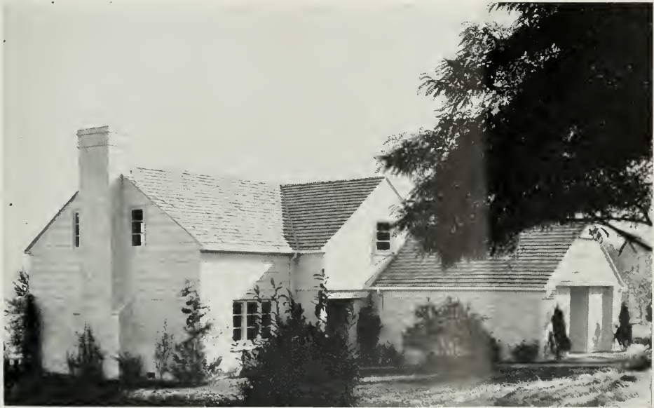
RESIDENCE AT SHERIDAN BEACH, SEATTLE, WASHINGTON William J. Bain, Architect Horizontal siding with V-joint vertical board siding on entrance gable
