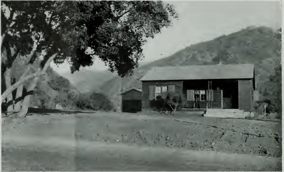
TYPICAL FOREST GUARD DWELLING, ANGELES NATIONAL FOREST, SOUTHERN CALIFORNIA Blanchard & Maher, Architects
