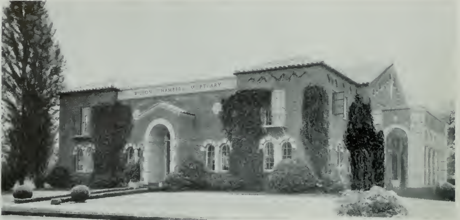
WILSON-CHAMBERS MORTUARY, PORTLAND, OREGON Richard Sundeleaf, Architect
