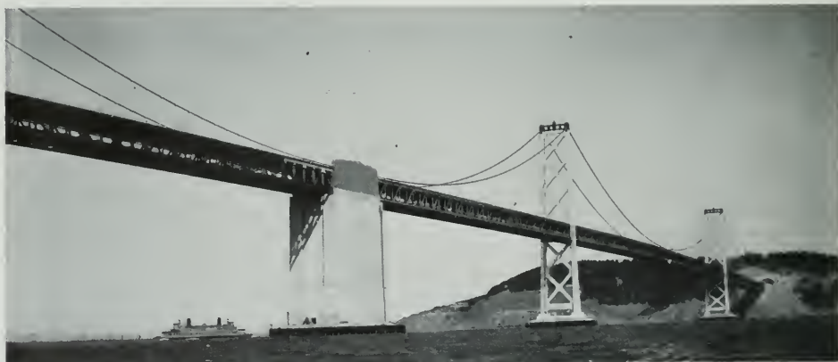
CENTER ANCHORAGE OF SAN FRANCISCO BAY BRIDGE; A POINT OF INTEREST AND COMMENT BY ENGINEERS
