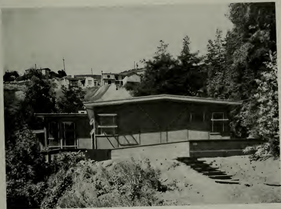
HOUSE FOR PROFESSOR ROBERT TRYON, BERKELEY, CALIFORNIA MICHAEL GOODMAN, ARCHITECT Exterior of \frac{1}{4} " plywood panels over sheathing used experimentally.
