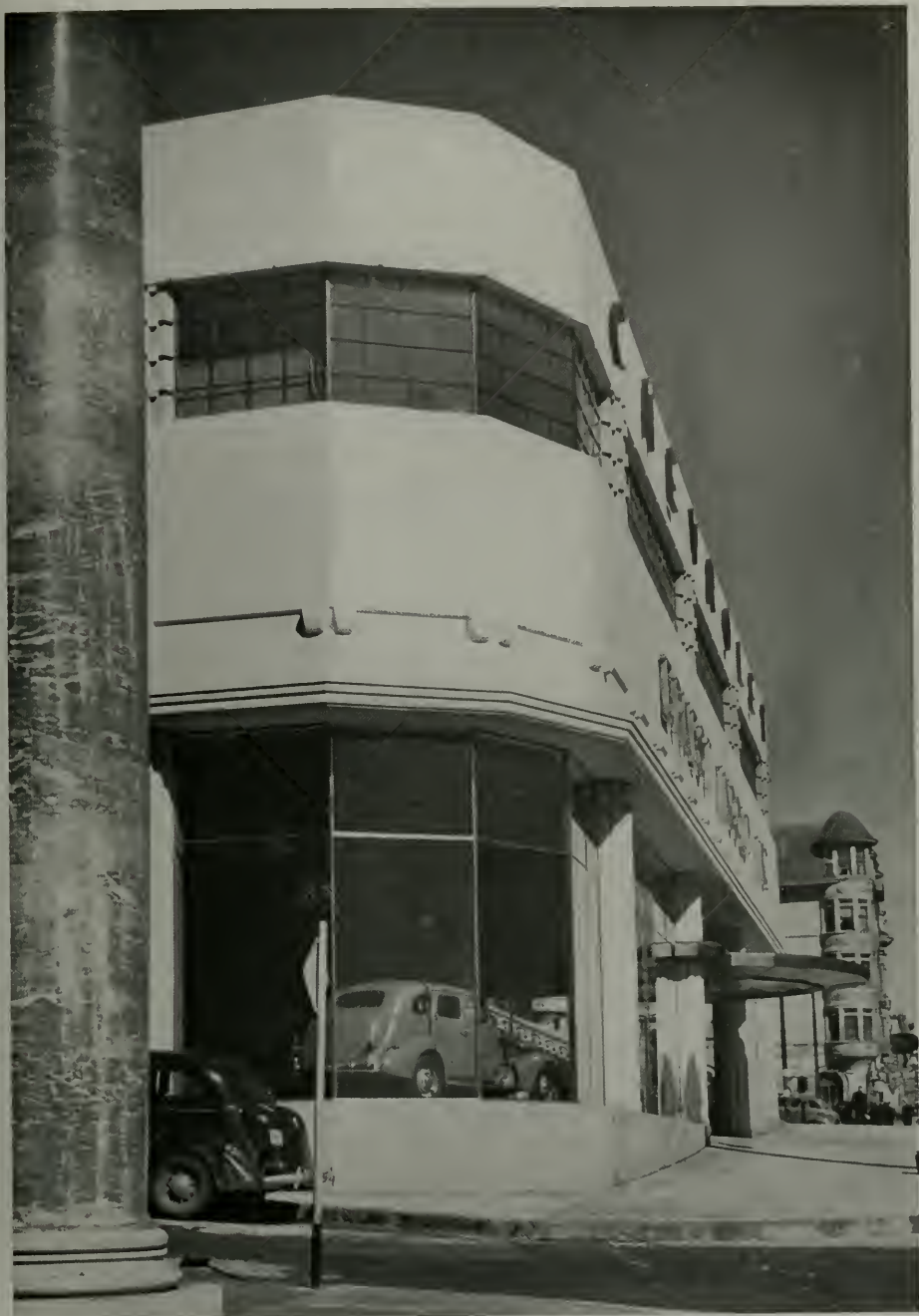
VAN NESS AVE. FRONT, ERNEST INGOLD AUTOMOBILE DISPLAY AND SERVICE BUILDING, SAN FRANCISCO John E. Dinwiddie, Architect
