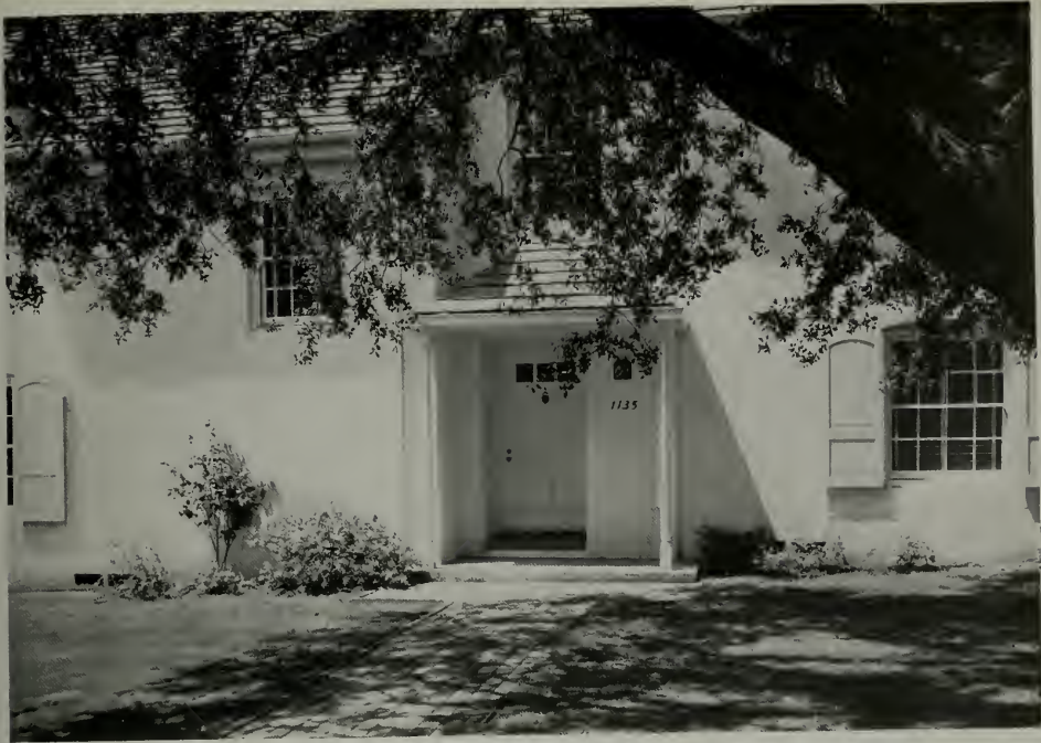
DETAIL OF ENTRANCE, RESIDENCE FOR MR. AND MRS. JOHN HOLMAN, SAN MARINO, CALIFORNIA
