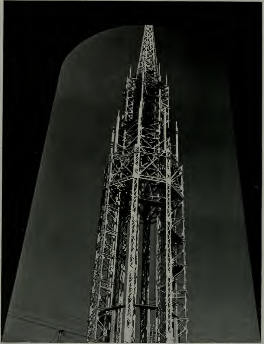
STRUCTURAL STEEL FRAMING OF CENTRAL THEME TOWER, GOLDEN GATE INTERNATIONAL EXPOSITION, TREASURE ISLAND
