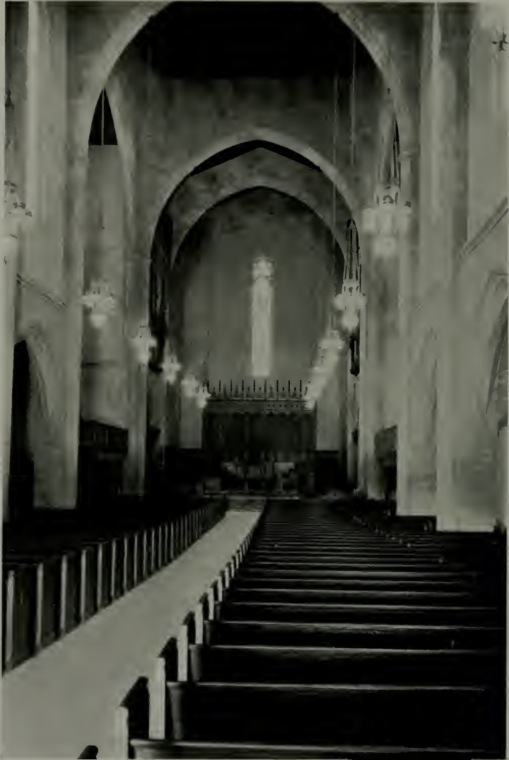
NAVE, LOOKING TOWARD THE CHANCEL, FIRST CONGREGATIONAL CHURCH OF LOS ANGELES ALLISON & ALLISON, ARCHITECTS
