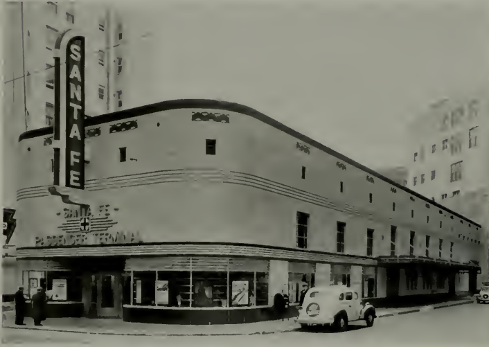
SANTA FE PASSENGER TERMINAL San Francisco
