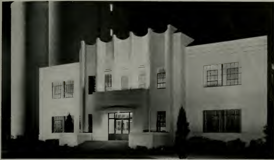
ADMINISTRATION UNIT, SPRECKELS SUGAR REFINERY
