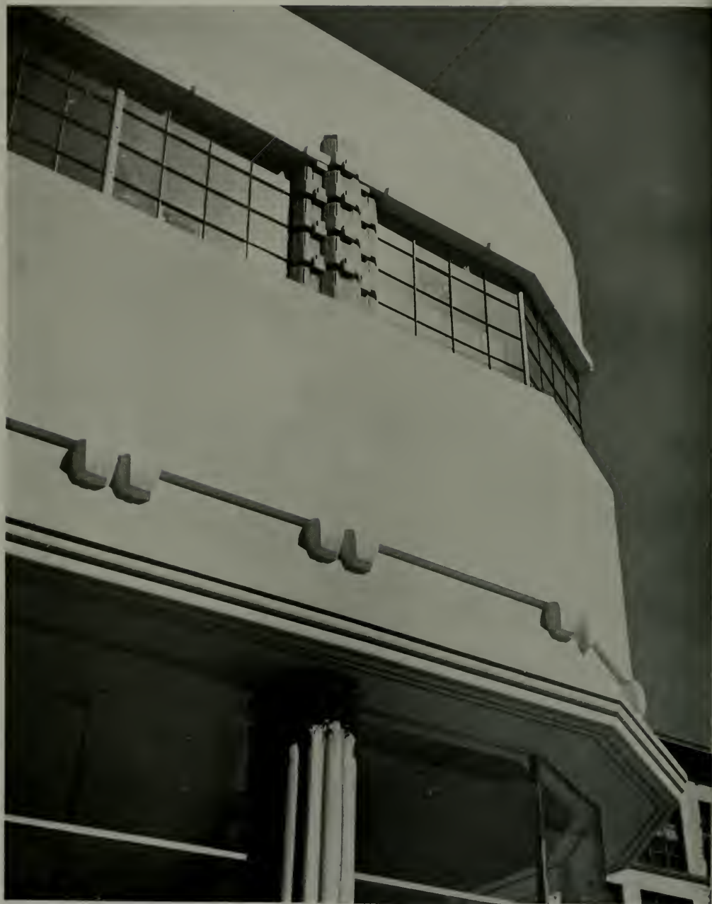
DETAIL, ERNEST INGOLD AUTOMOBILE DISPLAY AND SERVICE BUILDING, SAN FRANCISCO JOHN E. DINWIDDIE, ARCHITECT
