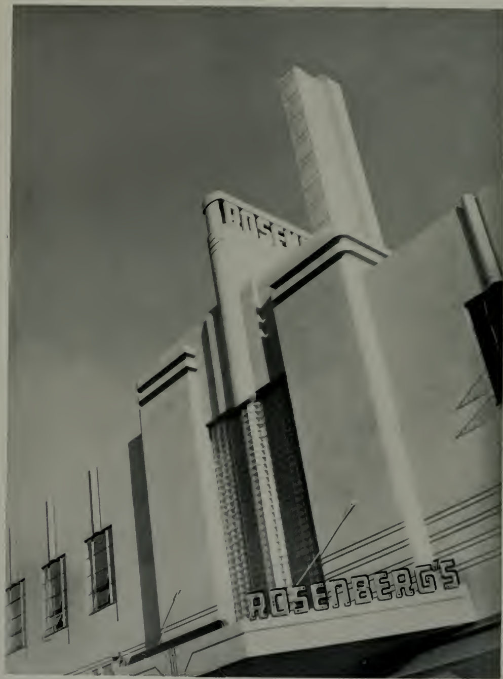
DETAIL OF TOWER, ROSENBERG'S DEPARTMENT STORE, SANTA ROSA, CALIFORNIA HERTZKA AND KNOWLES, ARCHITECTS
