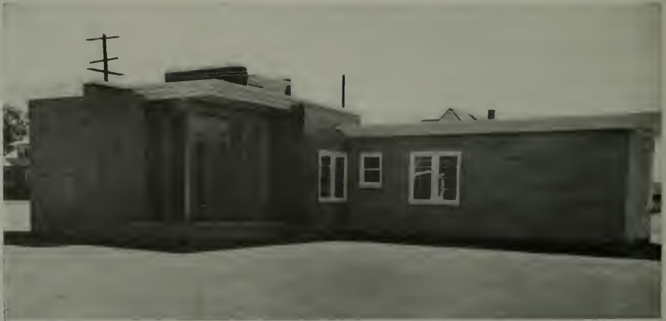
ULTRA MODERN HOUSE FOR R. A. SWANSON, ALBANY, OREGON, FROM PLANS BY FRANK LLOYD WRIGHT; R. C. MILLER, BUILDER Exterior of brick and hot pressed resin-bonded Douglas fir plywood with redwood face ply.
