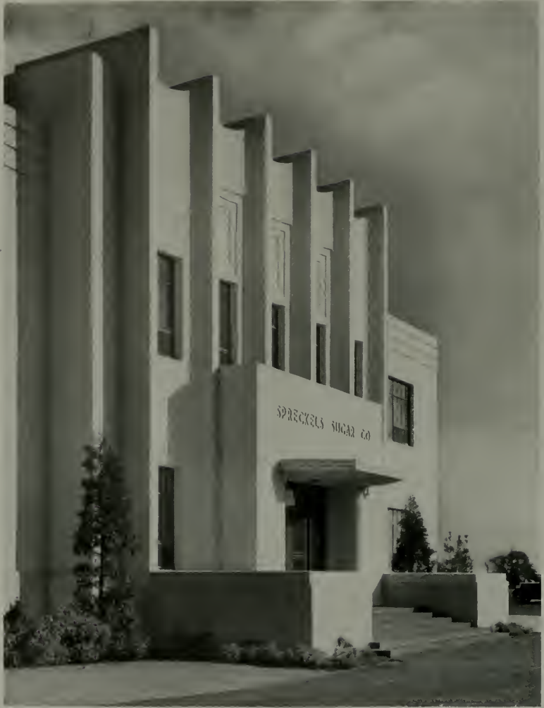
DETAIL OF ENTRANCE, SPRECKELS SUGAR PLANT, NEAR WOODLAND, CALIFORNIA Geo. W. Kelham, Harry A. Thomsen, Jr., Architects
