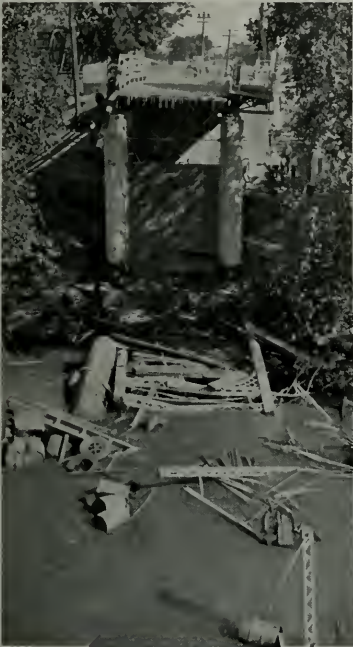
LEFT—SACRAMENTO RIVER BRIDGE AT RED BLUFF COLLAPSES. TRUCKS AND STEEL FRAMEWORK ARE SHOWN IN RIVER. RIGHT—TOWER ON SAN BENITO RIVER BRIDGE NEAR HOLLISTER DAMAGED BY TRUCK.
