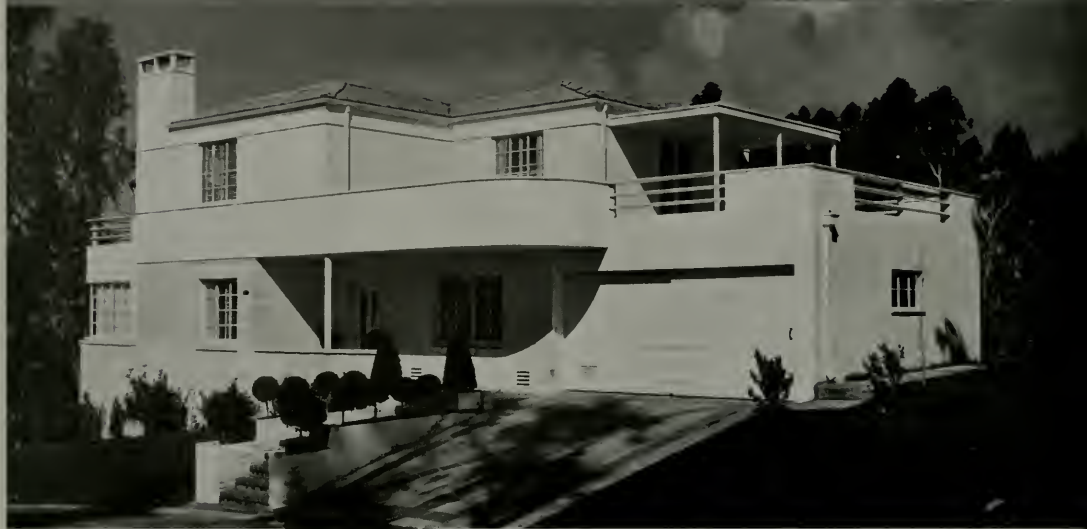
General Electric Model Home, Berkeley, California. John Ekin Dinwiddie, Architect J. M. Walker, Builder
