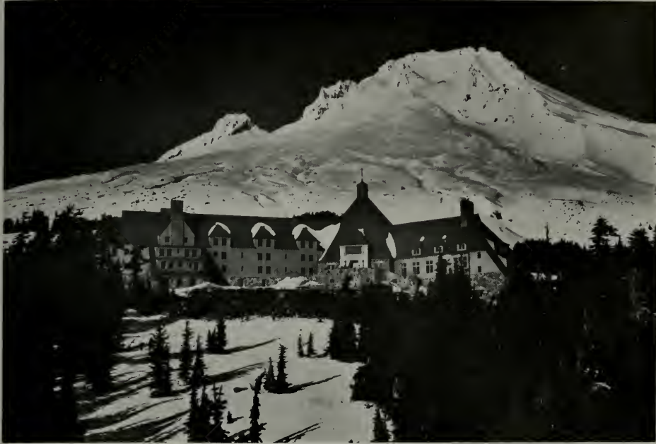
GENERAL VIEW, TIMBERLINE LODGE, MT. HOOD, OREGON U. S. FOREST SERVICE, ARCHITECTS GILBERT STANLEY UNDERWOOD CO., ASSOCIATE ARCHITECTS
