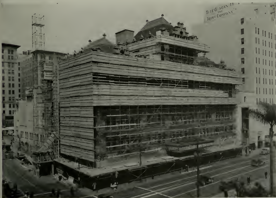
NEW PHILHARMONIC BUILDING, FORMERLY THE AUDITORIUM, LOS ANGELES Douglas fir plywood protective covering used while old face of building is being lifted for new.
