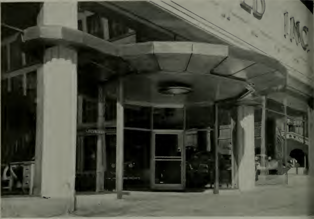
ENTRANCE, ERNEST INGOLD AUTOMOBILE DISPLAY AND SERVICE BUILDING, SAN FRANCISCO John E. Dinwiddie, Architect
