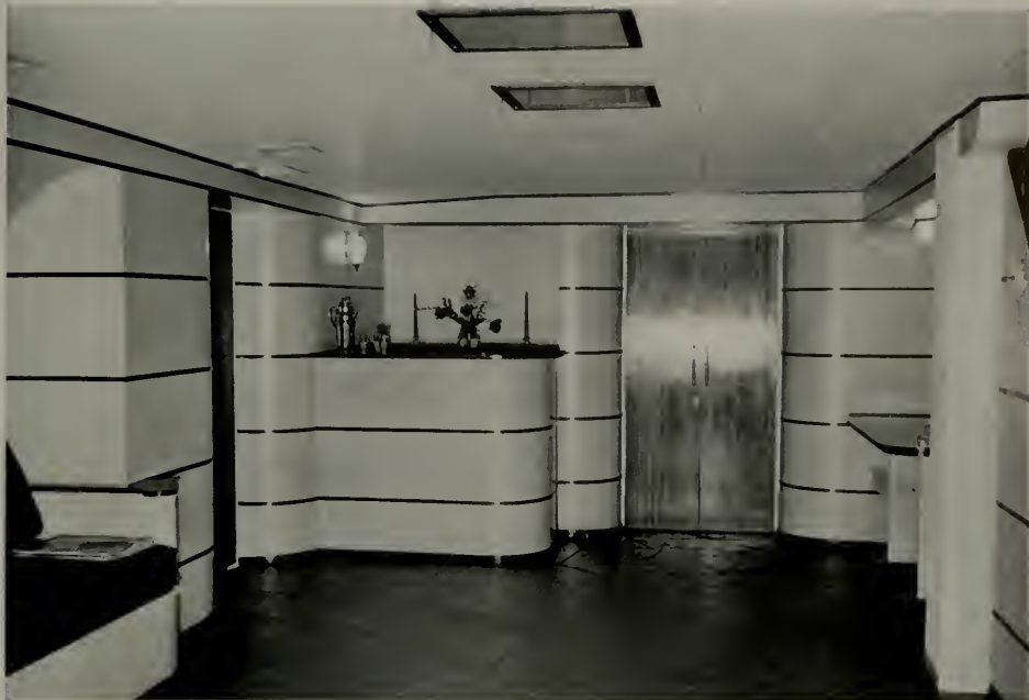
A RECREATION ROOM FINISHED IN GLOSS ENAMEL, THE DOUGLAS FIR PLYWOOD PANELS BEING PAINTED. CURVED SURFACES ACHIEVED BY BENDING THE 3/16" PLYWOOD TO FIT REQUIREMENTS.
