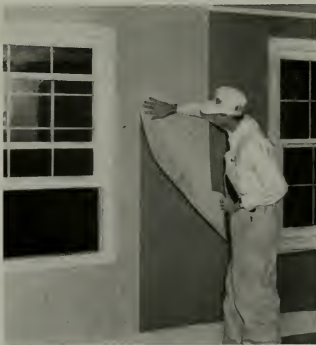
UNDER WALLPAPER, THE SKILLED DECORATOR PREFERS A BASE OF FIR PLYWOOD. IT IS BEST TO USE A 3/4 LB. DEADENING FELT OVER THE PLYWOOD.
