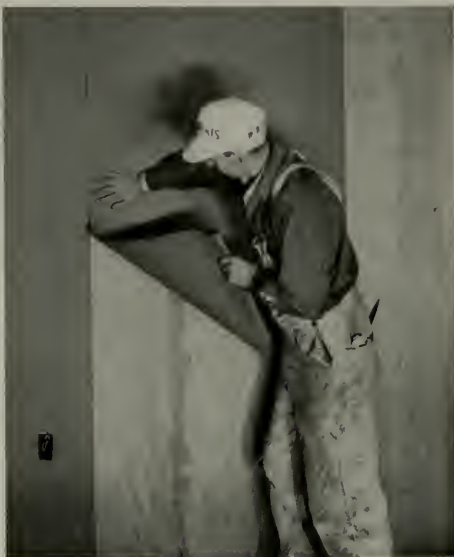
THE STRAIGHT EDGED FELT IS TIGHTLY BUTT-JOINTED, PROVIDING A SMOOTH SURFACE FOR THE PAPER.
