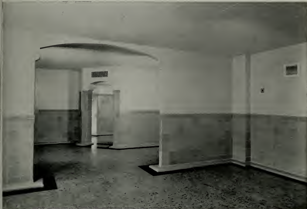
Typical Wards—showing use of Glazed Terra Cotta Wall Units
