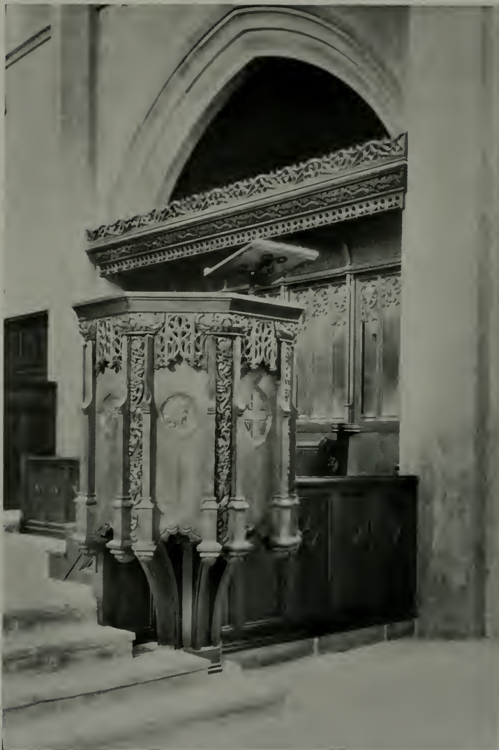
ARCHIBALD MEMORIAL PULPIT, FIRST CONGREGATIONAL CHURCH OF LOS ANGELES (Other photos Pages 32, 33, 34) ALLISON & ALLISON, ARCHITECTS
