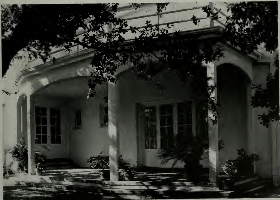
PORCH, RESIDENCE FOR MR. AND MRS. JOHN HOLMAN, SAN MARINO, CALIFORNIA
