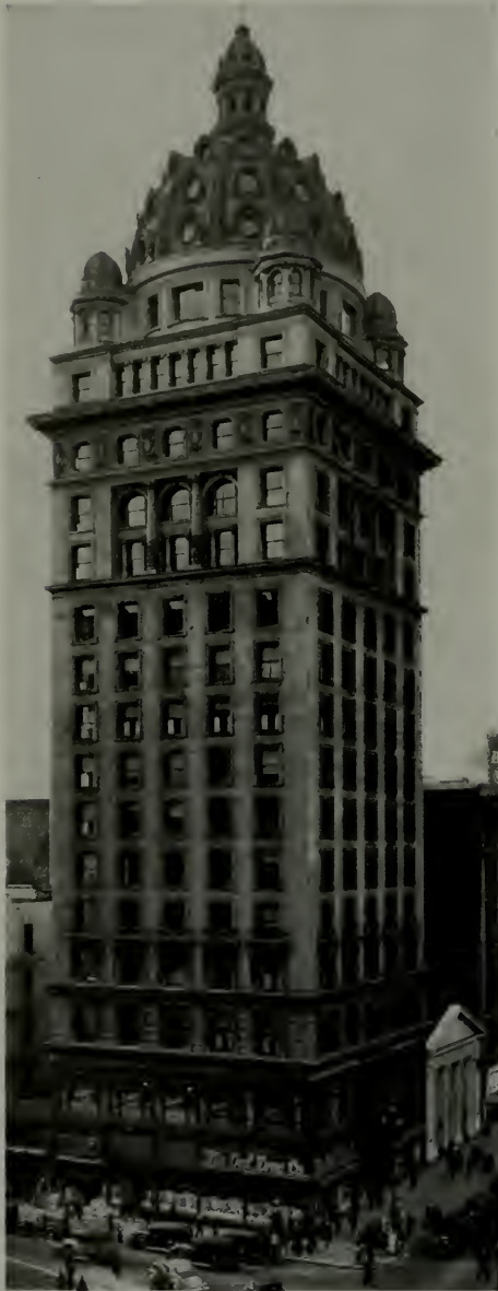
CLAUS SPRECKELS BUILDING AS IT LOOKED BEFORE MODERNIZATION. ORNAMENTAL DOME HAS BEEN REPLACED WITH SIX FLOORS OF RENTABLE OFFICE SPACE.
