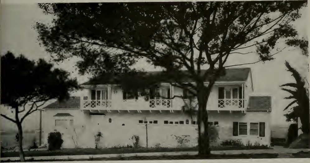
HOUSE FOR EARL L. HOFFMAN, LOS ANGELES, CALIFORNIA LEO F. BACHMAN, ARCHITECT
