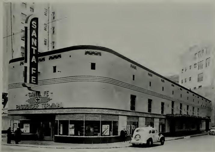
Santa Fe Passenger Terminal, San Francisco
