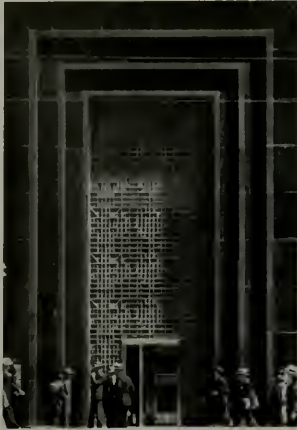
Entrance Detail, Central Tower, San Francisco Albert F. Roller, Architect
