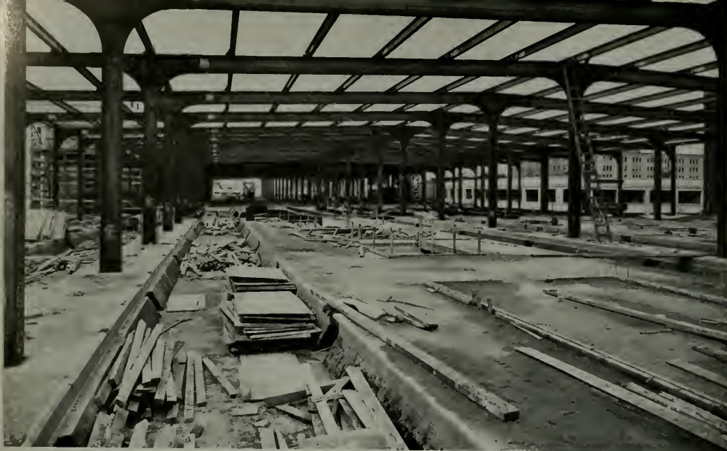
Trains will roll in the San Francisco Terminal over six tracks arranged in pairs. View of the elevated track level.
