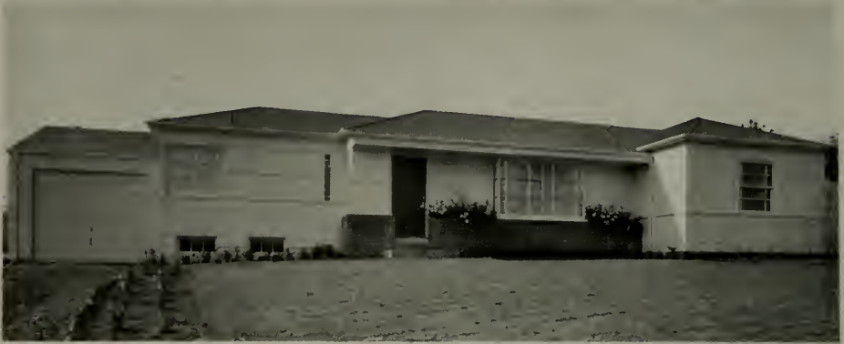
HOUSE OF A. P. TANSCHER, PORTLAND, OREGON DESIGNED BY J. WAYLAND OWEN Exterior covering is Harborside
