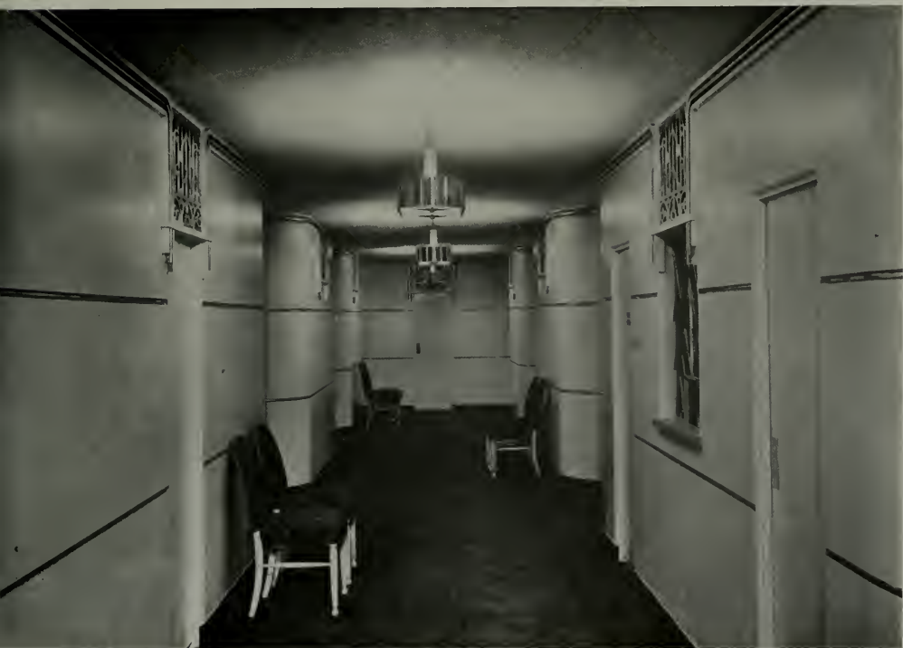
A RECREATION ROOM FINISHED IN GLOSS ENAMEL, THE DOUGLAS FIR PLYWOOD PANELS BEING PAINTED. CURVED SURFACES ACHIEVED BY BENDING THE 3/16" PLYWOOD TO FIT REQUIREMENTS.
