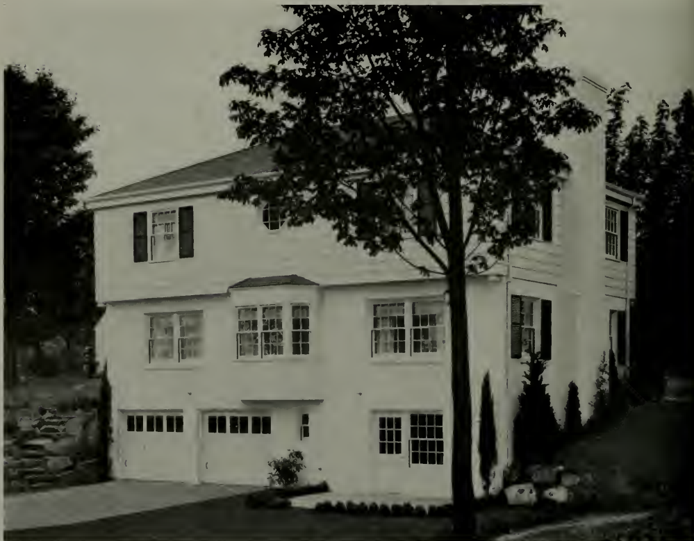
REAR VIEW OF BLUE RIDGE MODEL HOME, NEAR SEATTLE, WASHINGTON T. FRANCIS BELLAMY, ARCHITECT
