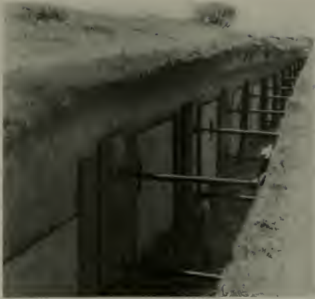
SEWER TRENCHES SHEETED WITH PLYWOOD PANELS. INSTEAD OF THE CUSTOMARY SUPPORT OF TIMBER SHEETING. STANDARD 4 x 8 FT. CONCRETE FORM PANELS OF 3/4 IN. DOUGLAS FIR PLYWOOD.
