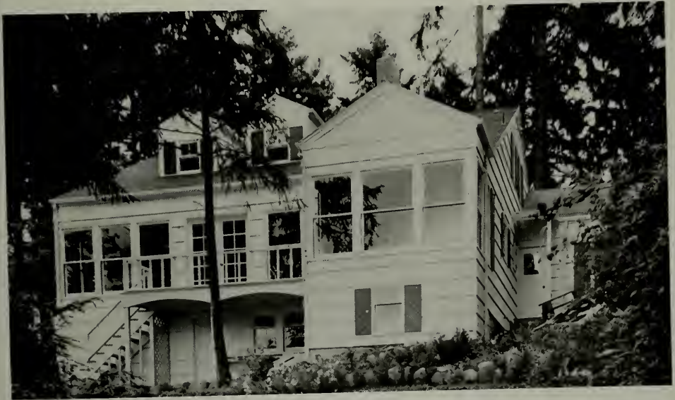
THE CLARK HOUSE AFTER ALTERATIONS AND ADDITIONS. ROOF IS RED CEDAR SHINGLES APPLIED TO 5/16" DOUGLAS FIR PLYWOOD SHEATHING SILAS E. NELSON, ARCHITECT
