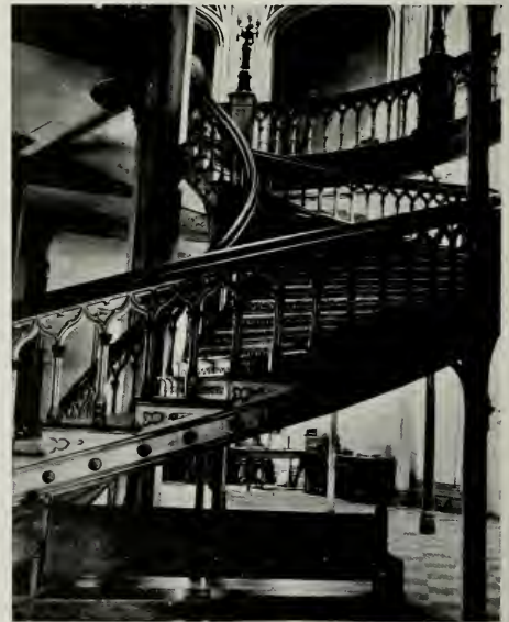
Great circular staircases are outstanding features of the old Louisiana State Capitol Building now being renovated by a group of Works Progress Administration employees. Replaced by a $5,000,000 skyscraper state office building, the old Capitol is being converted into a museum.
