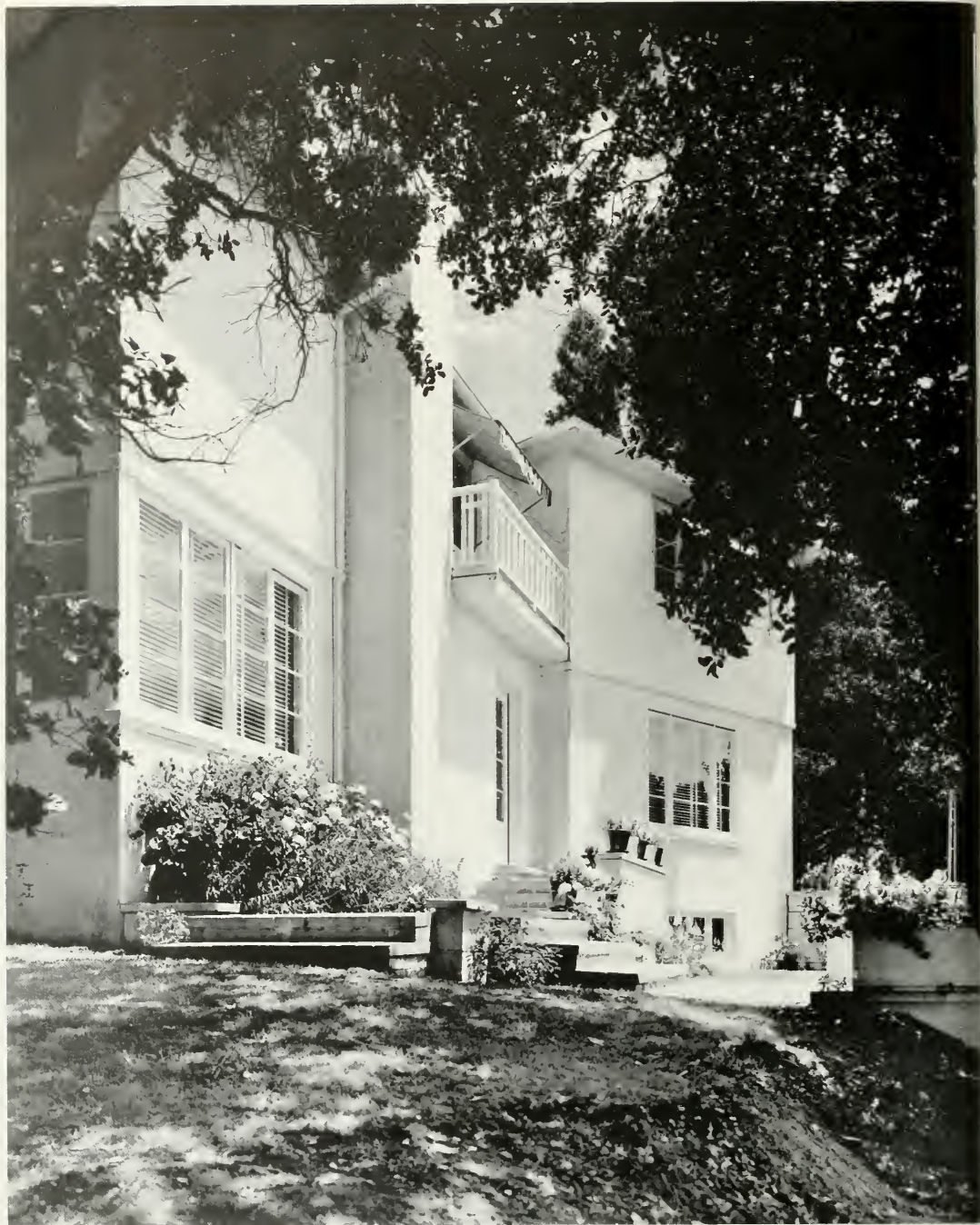
GARDEN VIEW, RESIDENCE OF CARL F. GROMME, ROSS, MARIN COUNTY, CALIFORNIA
