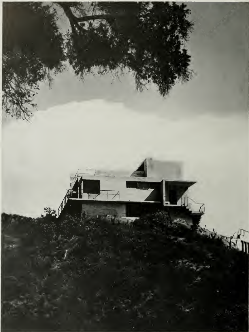
REINFORCED CONCRETE HOUSE FOR RICHARD HALLIBURTON, LAGUNA BEACH, CALIFORNIA
