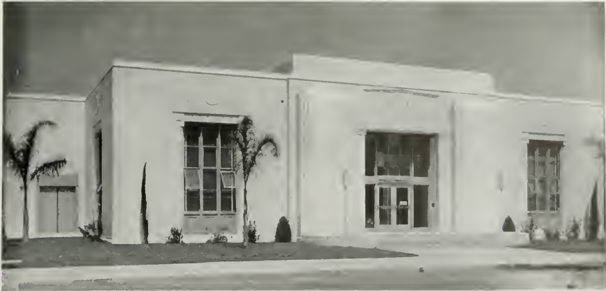
PUBLIC LIBRARY, TORRENCE, LOS ANGELES COUNTY, CALIFORNIA Walker and Eisen, Architects
