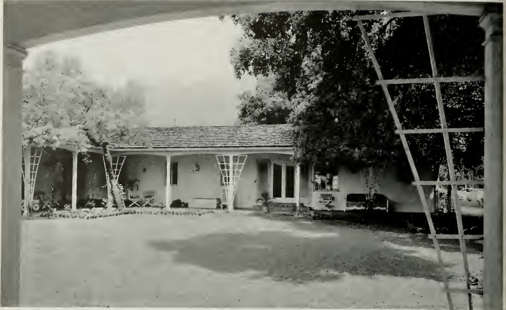
REINFORCED CONCRETE HOUSE FOR JOHN D. GREGG, ARCADIA, CALIFORNIA GARRETT VAN PELT, ARCHITECT
