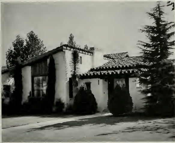
Residence of J. W. Hall, Fresno, California
