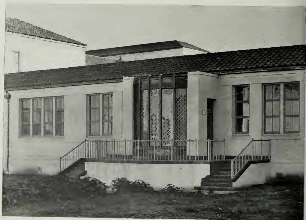
THE DOMESTIC SCIENCE DINING ROOM BAY OVERLOOKS THE FOUNTAIN COURT
