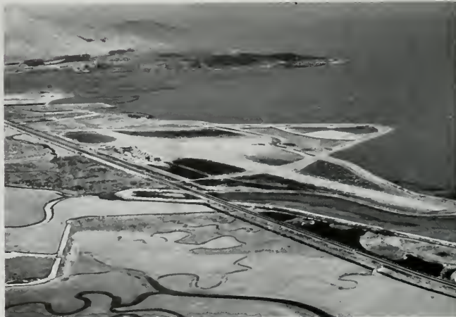
SAN FRANCISCO AIRPORT AFTER COMPLETION OF RECLAMATION, FINANCED BY $260,000 PWA BOND ISSUE
