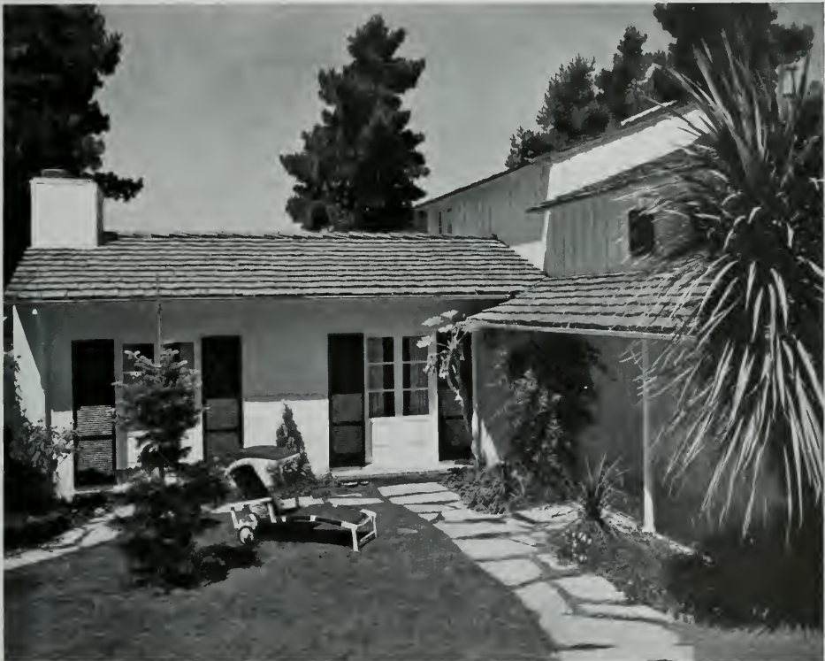
HOUSE IN PIEDMONT PINES, OAKLAND, CALIFORNIA Miller and Warnecke, Architects
