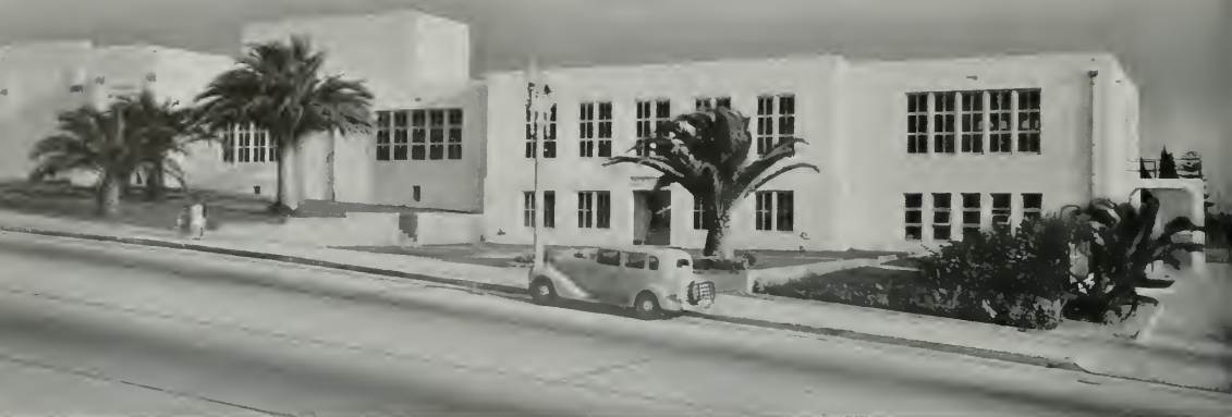
HERMOSA BEACH SCHOOL, SHOWING CLASSROOM WING; WINDOWLESS AUDITORIUM ON THE LEFT, HIGH STAGE LOFT NEAR THE CENTER Samuel E. Lunden, Architect
