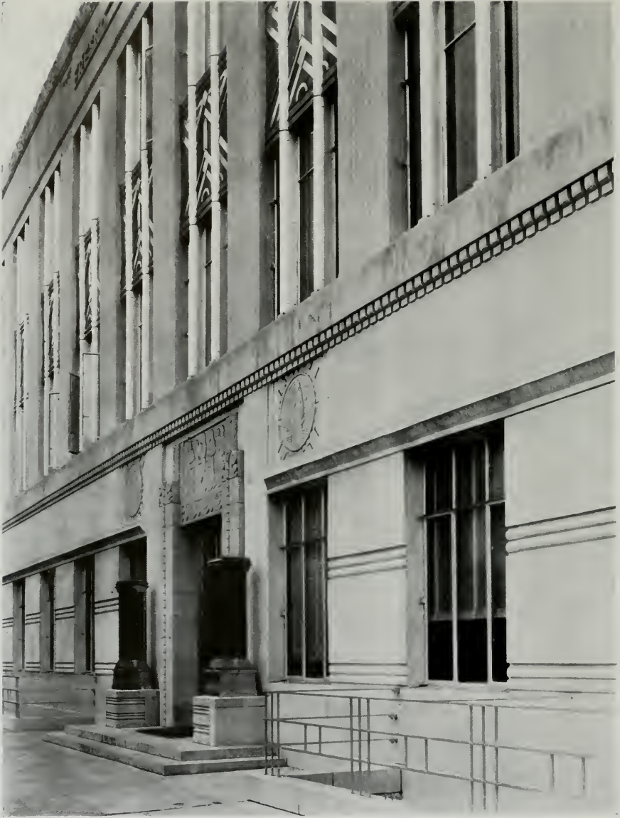
DETAIL OF FACADE, FRESNO COUNTY HALL OF RECORDS, FRESNO, CALIFORNIA W. D. COATES, FRED L. SCHWARTZ, H. RAPHAEL LAKE, CHARLES H. FRANKLIN, E. J. KUMP AND E. W. PETERSON, ALLIED ARCHITECTS.
