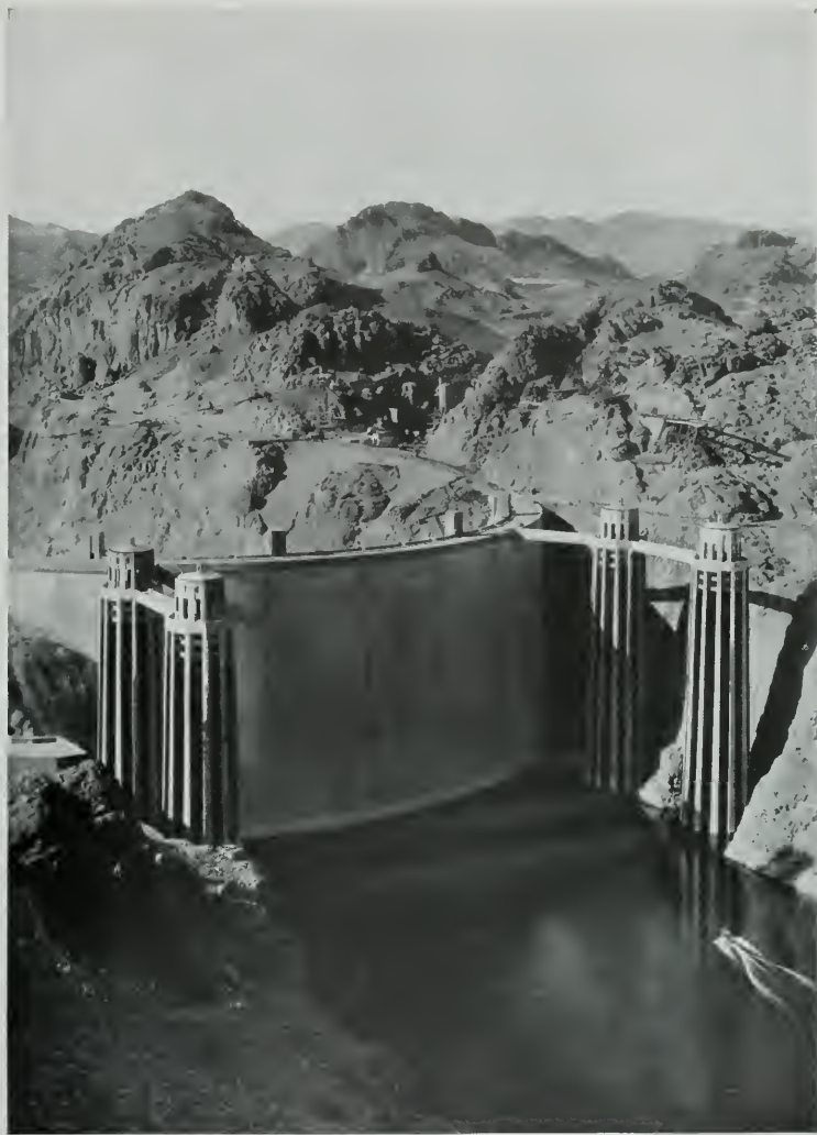
INTAKE TOWERS, UPSTREAM FACE OF DAM GORDON B. KAUFMANN, ARCHITECT
