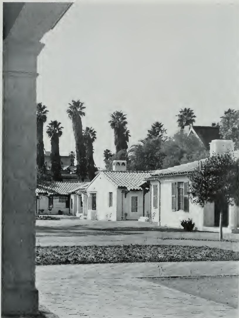
LOOKING SOUTHWEST TOWARD THREE OF THE BUNGALOWS, CHAPMAN PARK HOTEL PUEBLO, LOS ANGELES
