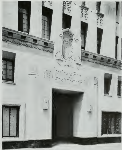
ENTRANCE DETAIL, HILL CASTLE APARTMENTS OAKLAND, CALIFORNIA
