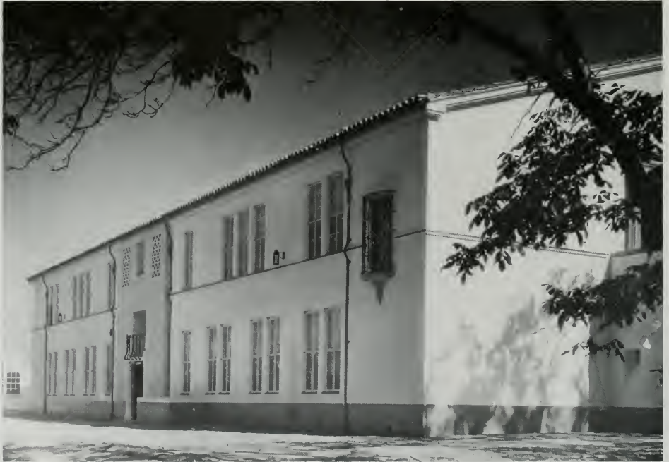
SOUTHWEST FACADE, FULLERTON JUNIOR COLLEGE Harry K. Vaughn, Architect
