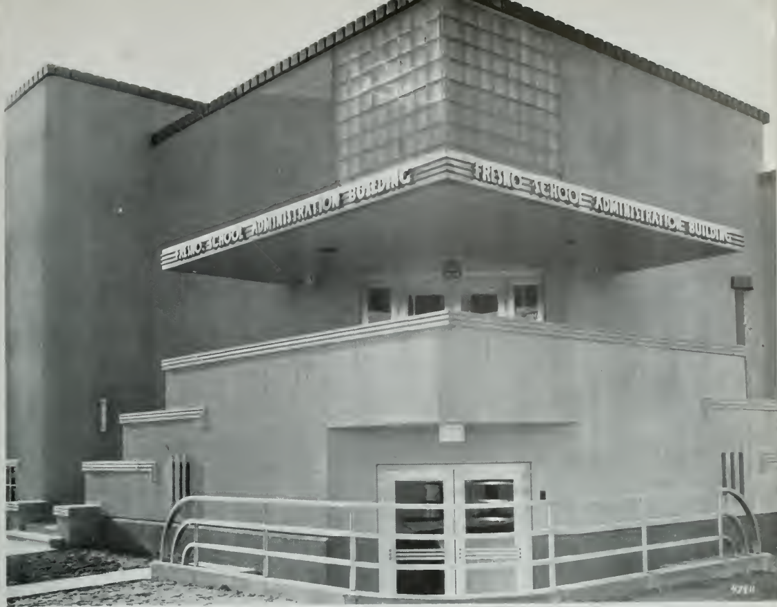
SCHOOL ADMINISTRATION BUILDING, FRESNO, CALIFORNIA OFFICE OF CHARLES H. FRANKLIN, FOR ALLIED ARCHITECTS OF FRESNO.
