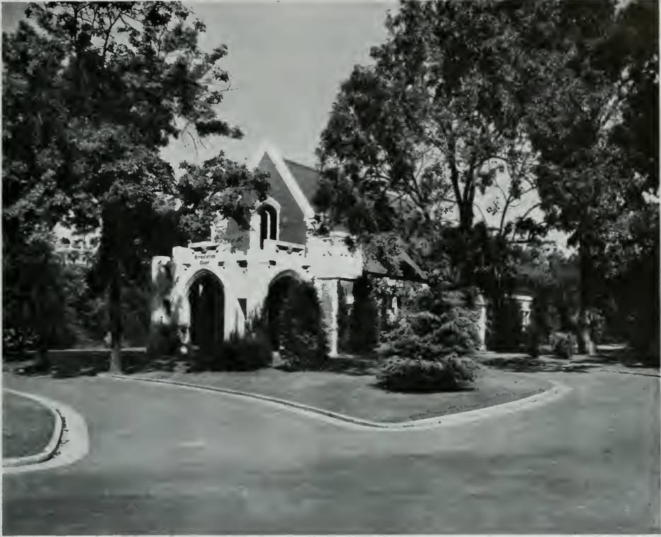
CREMATORIUM CHAPEL, MOUNTAIN VIEW MEMORIAL PARK, OAKLAND, CALIFORNIA W. P. Day, Architect
