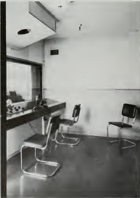
Typical of the individual control rooms for the different studios in KFWB at Hollywood.
