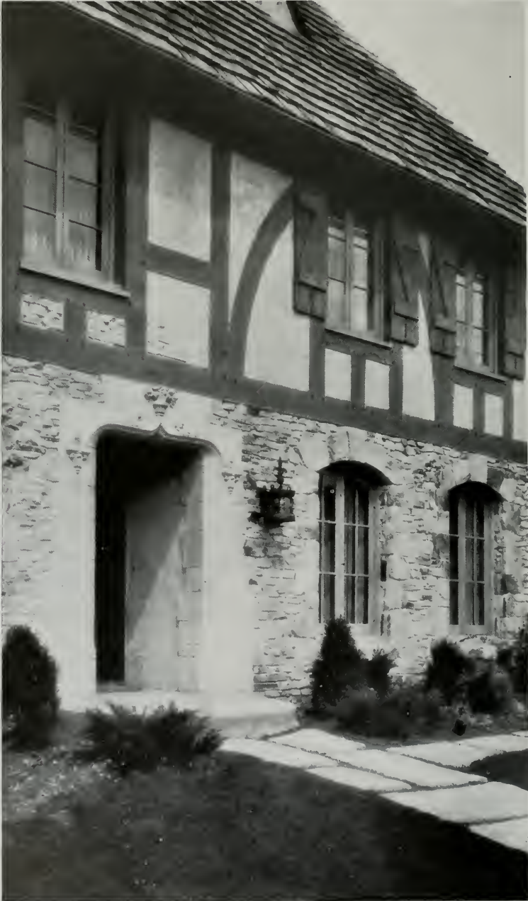
DETAIL OF FRONT, RESIDENCE OF GEORGE BEAN, PIEDMONT Miller and Warnecke, Architects
