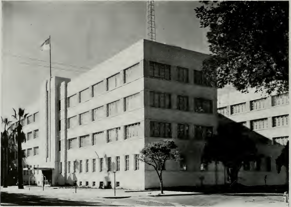
MOTOR VEHICLE OFFICE BUILDING, SACRAMENTO, CALIFORNIA
