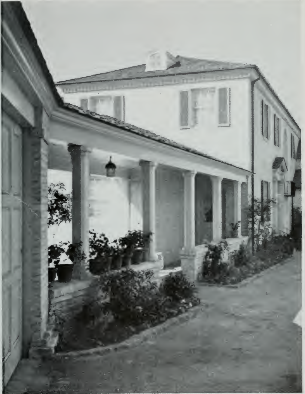
LOGGIA, RESIDENCE OF STANLEY HILLER, BERKELEY, CALIFORNIA JOHN KNOX BALLANTINE, JR., ARCHITECT
