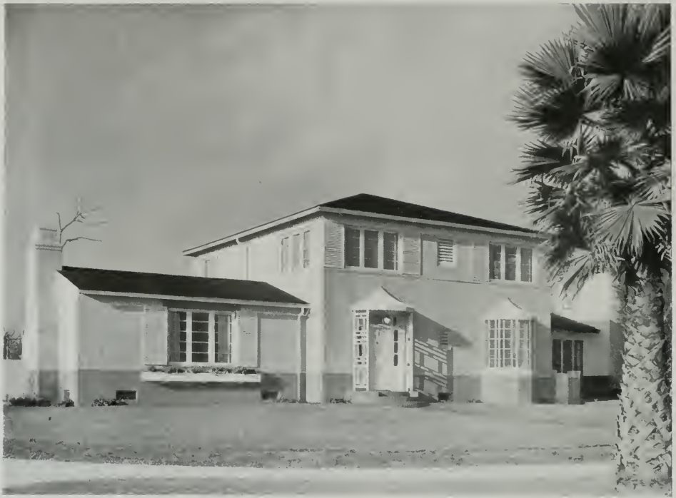
RESIDENCE OF DR. C. R. HOWSON, SAN MARINO, CALIFORNIA GORDON B. KAUFMANN, ARCHITECT
