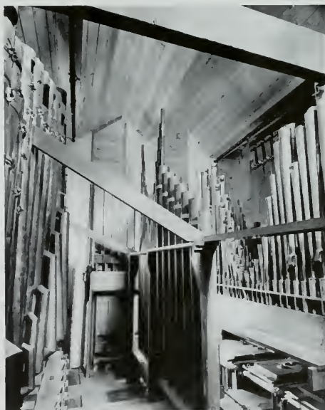
The interior of one of the two organ reverberation rooms showing the introduction of "splayed" ceiling to eliminate any parallel surfaces.
