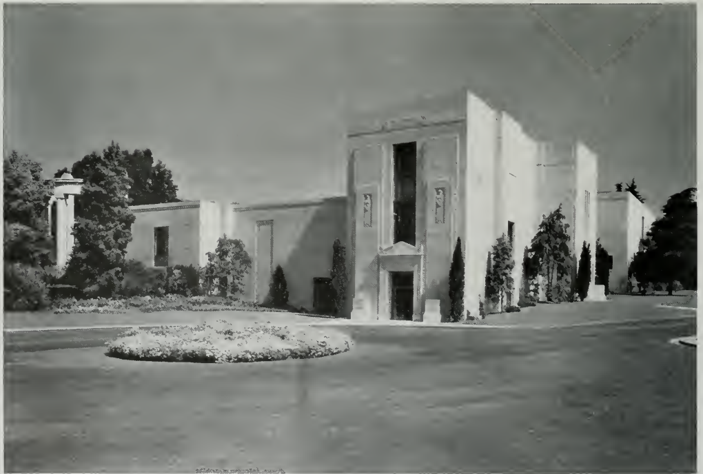
MAIN MAUSOLEUM, MOUNTAIN VIEW MEMORIAL PARK OAKLAND, CALIFORNIA W. P. Day, Architect
