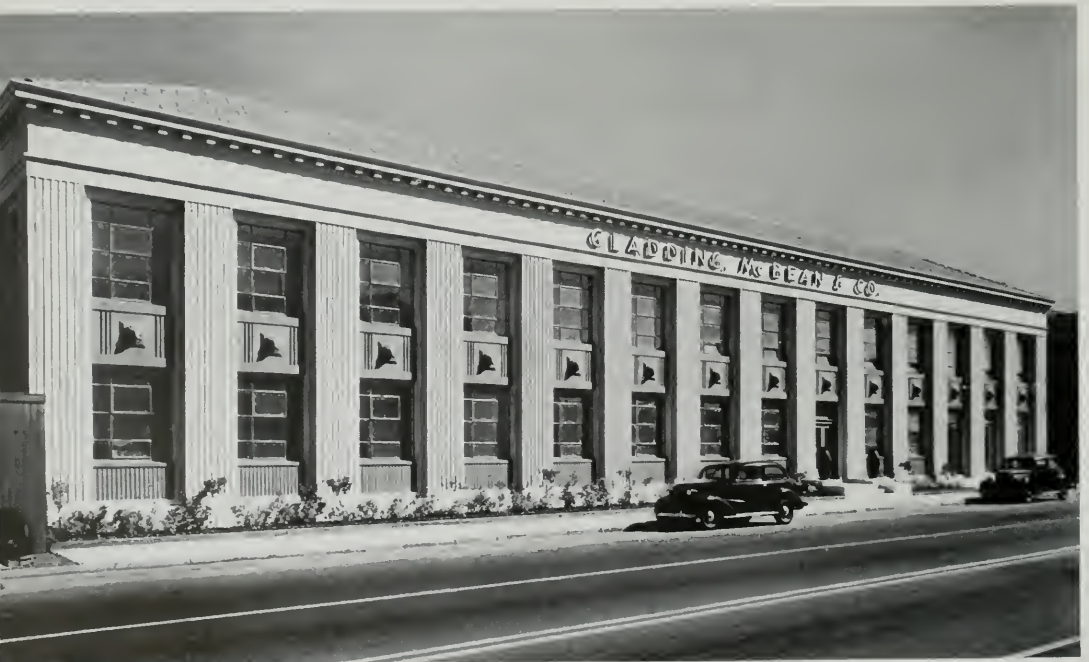
NEW BUILDING FOR GLADDING, McBEAN & COMPANY, SAN FRANCISCO, CALIFORNIA
