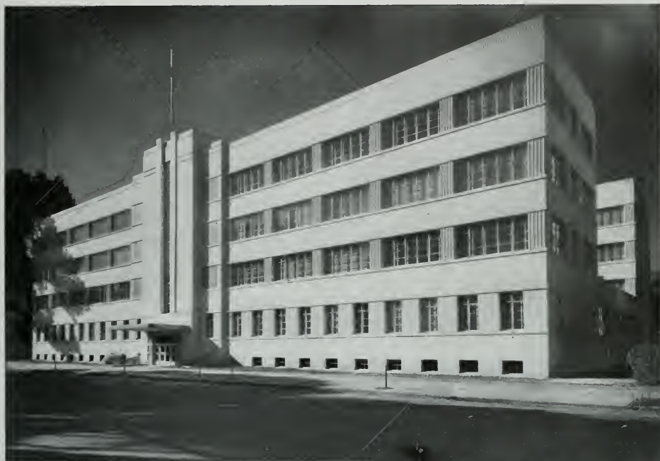
BUILDING FOR PUBLIC WORKS DEPARTMENT, SACRAMENTO Geo. B. McDougall, State Architect
