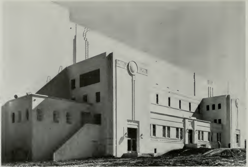
REAR VIEW, FRESNO MEMORIAL AUDITORIUM, FRESNO, CALIFORNIA
