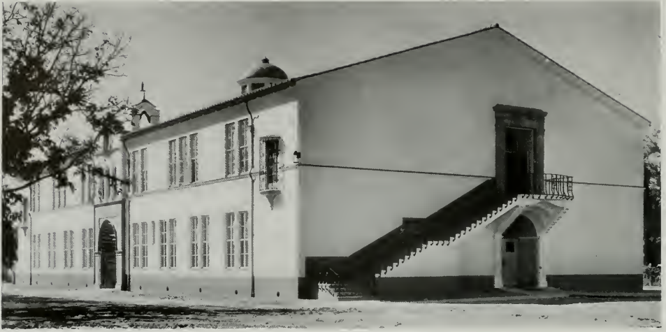
NORTHEAST CORNER, FULLERTON JUNIOR COLLEGE Harry K. Vaughn, Architect
