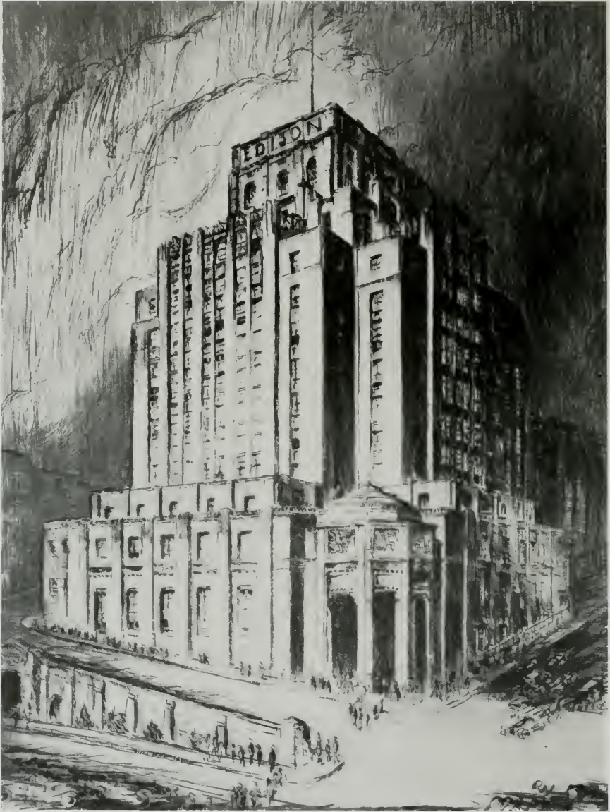
SOUTHERN CALIFORNIA EDISON BUILDING, LOS ANGELES, CALIFORNIA ALLISON & ALLISON, ARCHITECTS.
