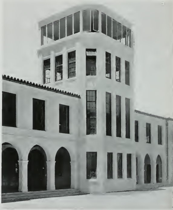
TOWER, ADMINISTRATION BUILDING, SAN FRANCISCO AIRPORT, SAN FRANCISCO
