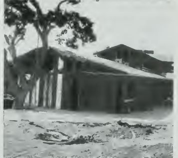
Note roof built around tree
