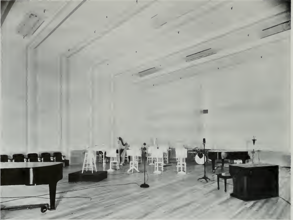
Studio Five in Warner Brothers KFWB at Hollywood was planned for the presentation of orchestra and choruses without audience, and its acoustical design allows placing the source of sound to any point desired in the room. Six different materials were used in the wall construction. Elimination of the wainscoting proved a distinct aid in the control of flutter echoes.
