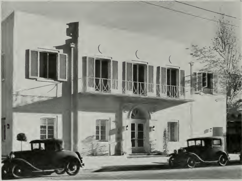
ASSEMBLY HALL, LOS ANGELES COUNTY MEDICAL ASSOCIATION, LOS ANGELES, CALIFORNIA GORDON B. KAUFMANN, ARCHITECT
