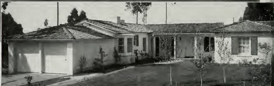
Residence of Mr. and Mrs. Vernon Ball, Creston Road, Berkeley. Edwin Lewis Snyder, Architect; J. M. Walker, Builder.
