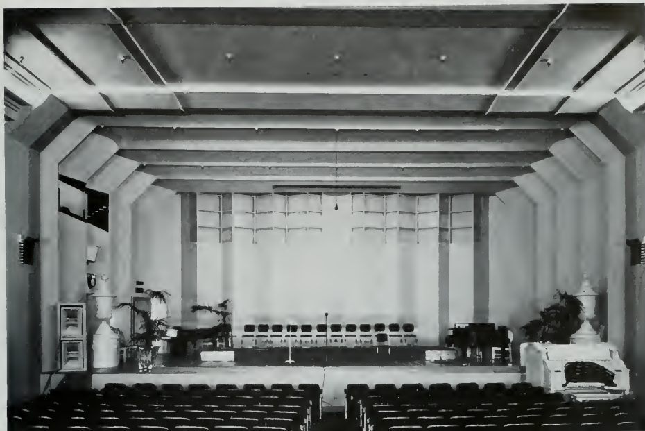
Auditorium and stage of Warner Brothers new KFWB at Hollywood, showing in detail the "splayed" wall treatment which was used to back up the musicians. At the back center is seen the penthouse from which the motion picture screen is dropped. At the right of the stage is the manual of the Wurlitzer organ and at the upper left hand side are seen the sponsors' booth and the studio control room. This differs from ordinary construction in that the auditorium and stage are built as a single room, instead of being two acoustically coupled units.
