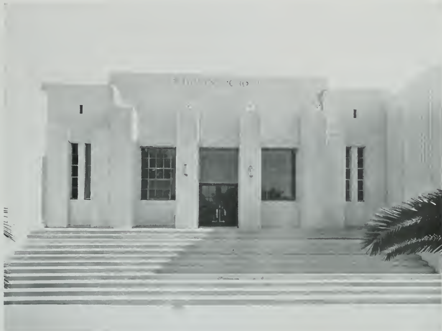
FRONT ELEVATION, CONLEY GRAMMAR SCHOOL, TAFT, CALIFORNIA Charles H. Biggar, Architect L. H. Nickkian, Structural Engineer
