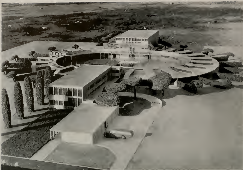
RING PLAN SCHOOL INTENDED TO SERVE A WIDELY DISTRIBUTED POPULATION Richard J. Neutra, Architect Each classroom, with free grouping of children, opens into a private schoolroom patio.
