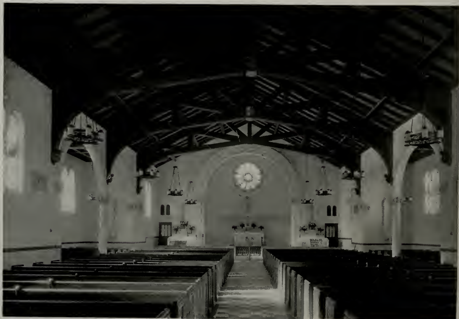
AUDITORIUM, ST. PETER MARTYR CHURCH, PITTSBURG Arnold Constable, Architect
