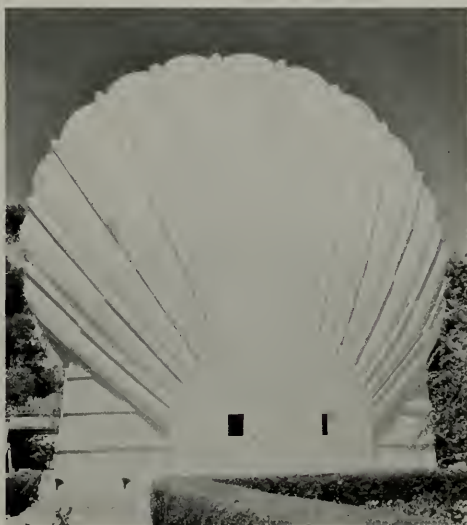
REAR VIEW OF SHELL OIL BUILDING, EXPOSITION GROUNDS, SAN DIEGO
