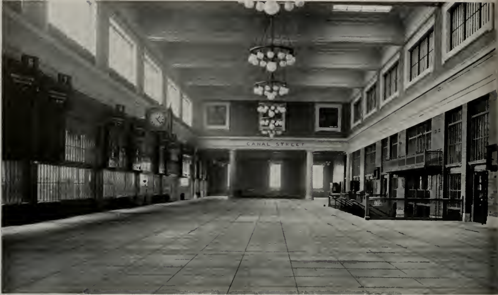
CONCRETE FLOOR IN CONCOURSE, CHICAGO AND NORTHWESTERN RAILWAY TERMINAL, CHICAGO Frost & Granger, Architects
