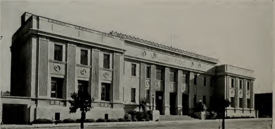
VETERANS MEMORIAL BUILDING, BERKELEY, CALIFORNIA Henry H. Meyers, Architect George R. Klinkhardt and Mildred S. Meyers, Associate Architects
