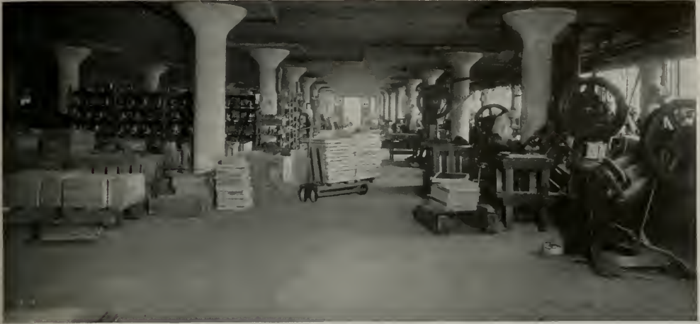
TEN YEARS OF TRUCKING HEAVY LOADS HAS NOT MARRED THIS CONCRETE FLOOR FINISH Crushed trap rock aggregate was used in this wearing course and the surface was finished by troweling. The hard wearing quality of the floor is largely due to the control of the water-cement ratio in mixing and adequate curing.
