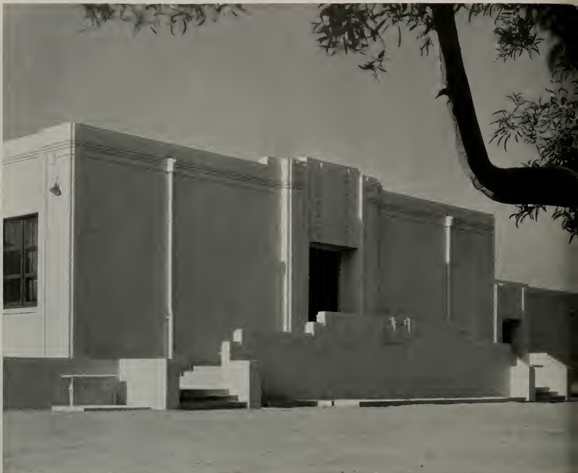
GROVER CLEVELAND ELEMENTARY SCHOOL, PASADENA, CALIFORNIA ROBERT H. AINSWORTH, ARCHITECT
