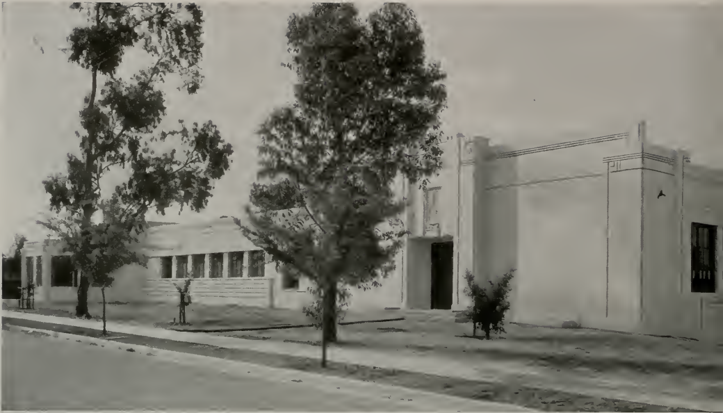
GROVER CLEVELAND ELEMENTARY SCHOOL, PASADENA, CALIFORNIA Robert H. Ainsworth, Architect
