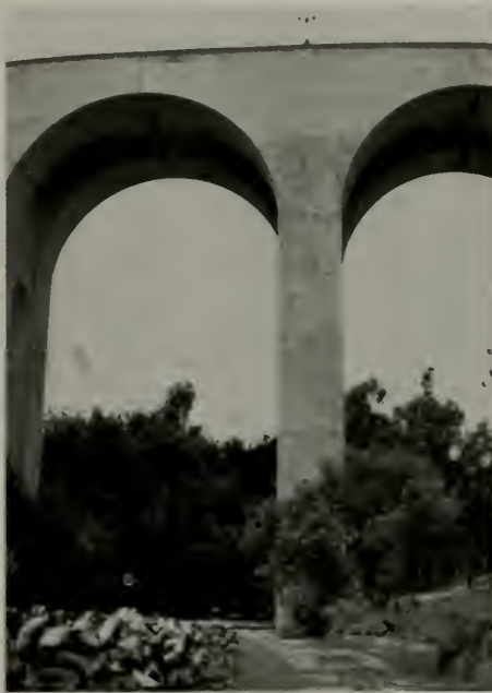
CLOSE-UP OF CABRILLO BRIDGE, BALBOA PARK, SAN DIEGO
