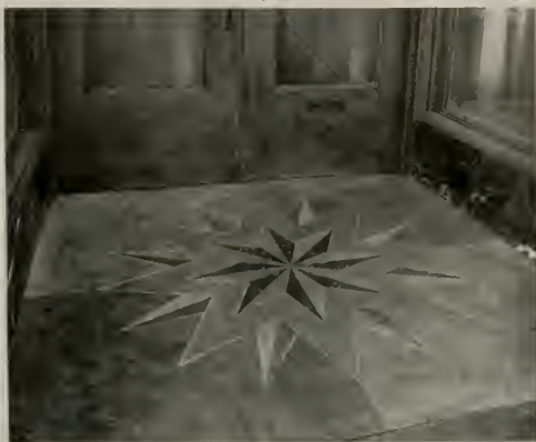
VARICOLORED FLOOR FINISH, COOPER BUILDING, LOS ANGELES
