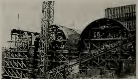
FORM WORK FOR SUPERSTRUCTURE, CABRILLO BRIDGE, BALBOA PARK, SAN DIEGO
