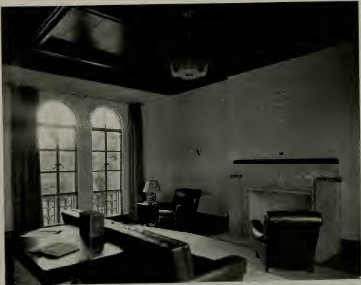
MEN'S CLUB ROOM, VETERANS MEMORIAL BUILDING, SAN LEANDRO Henry H. Meyers, Architect George R. Klinkhardt and Mildred S. Meyers, Associate Architects
