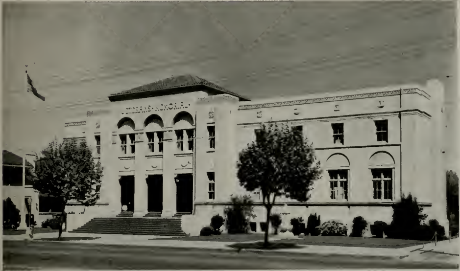
VETERANS MEMORIAL BUILDING, ALAMEDA, CALIFORNIA Henry H. Meyers, Architect George R. Klinkhardt and Mildred S. Meyers, Associate Architects
