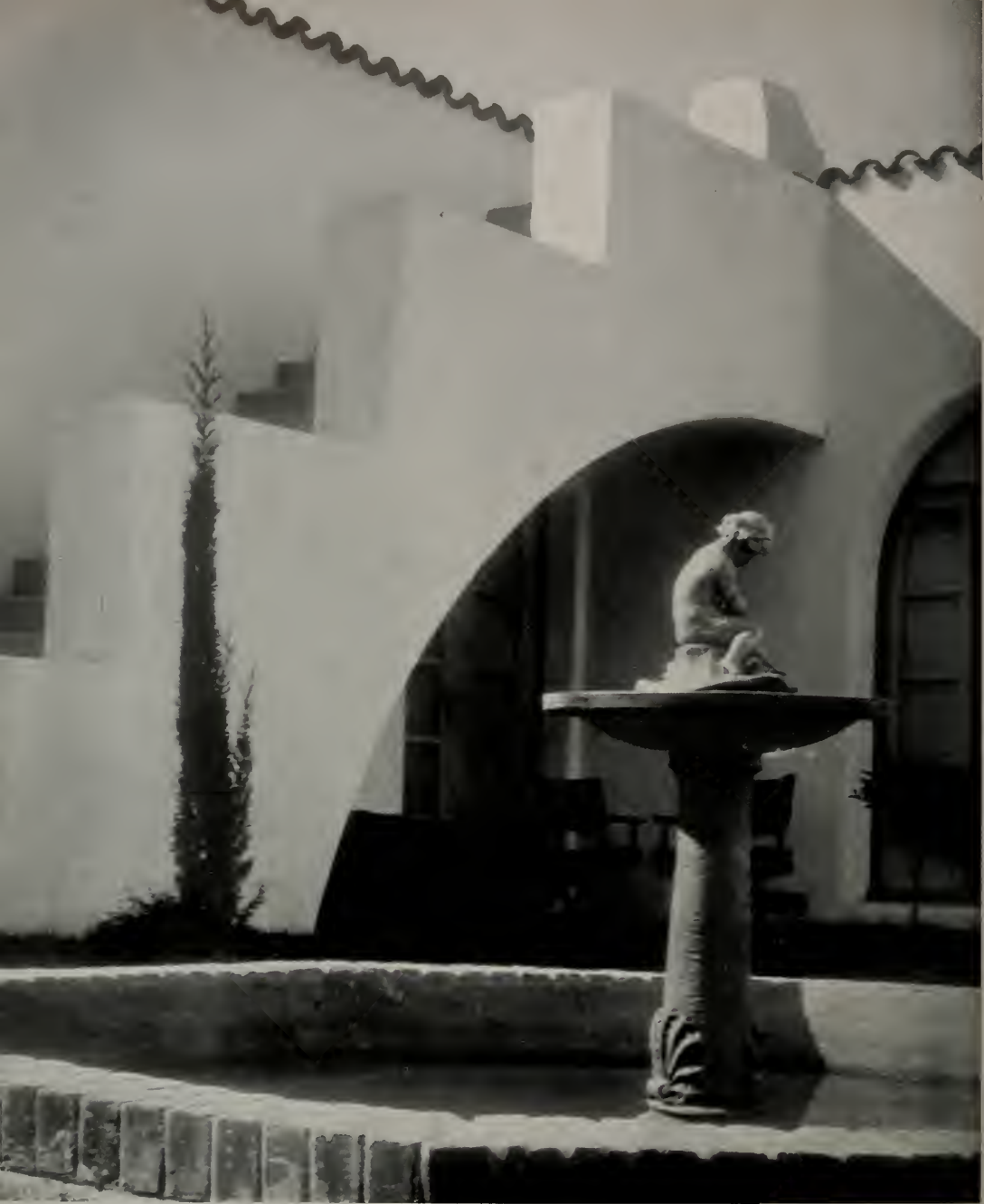
DETAIL OF PATIO, WINTER RESIDENCE OF A. W. STARKE, PALM SPRINGS, CALIFORNIA LELAND F. FULLER, ARCHITECT
