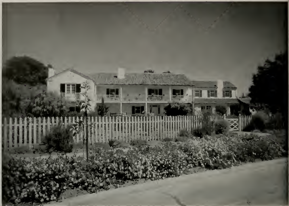
RESIDENCE OF E. M. MANNING, PALO ALTO, CALIFORNIA GARDNER A. DAILEY, ARCHITECT
