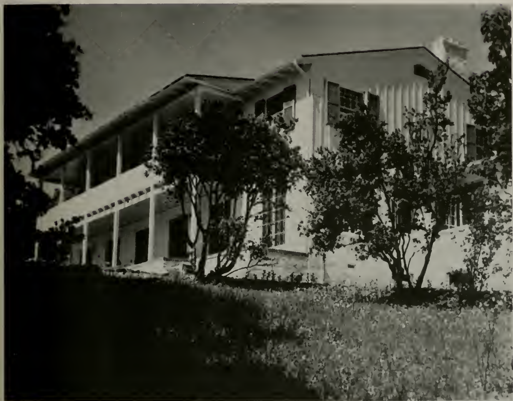
RESIDENCE OF MR. AND MRS. J. D. ADAMS, ROSS, CALIFORNIA ALBERT JOHN EVERS, ARCHITECT
