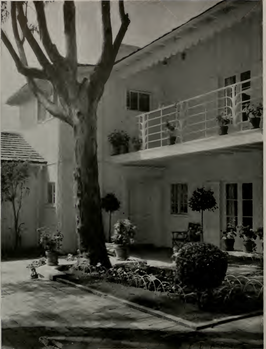
RESIDENCE OF DR. CARY SNODDY, VALLEJO, CALIFORNIA FREDERICK L. R. CONFER, ARCHITECT
