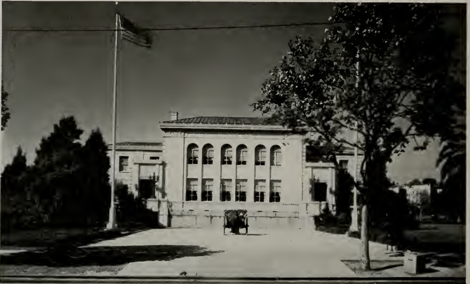
VETERANS MEMORIAL BUILDING, OAKLAND, CALIFORNIA Henry H. Meyers, Architect George R. Klinkhardt and Mildred S. Meyers, Associate Architects
