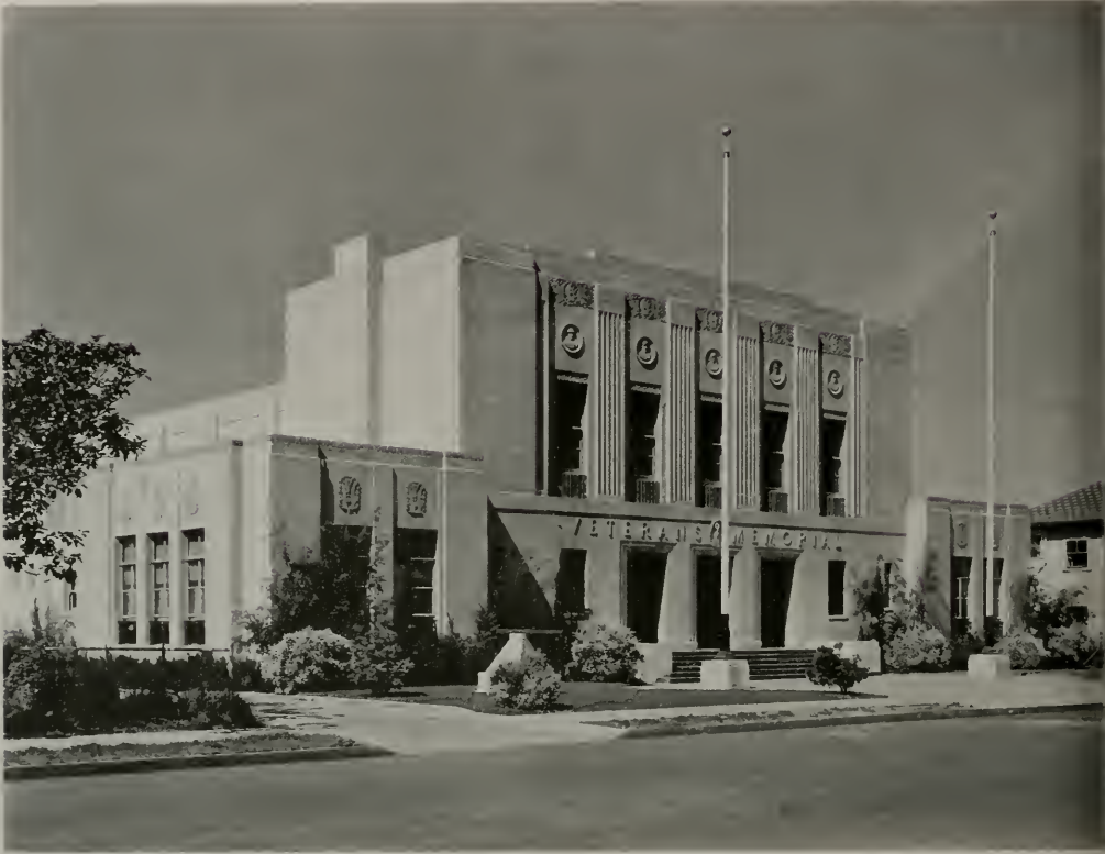
VETERANS MEMORIAL BUILDING, HAYWARD, CALIFORNIA HENRY H. MEYERS. ARCHITECT: GEO. R. KLINKHARDT AND MILDRED S. MEYERS. ASSOCIATES
