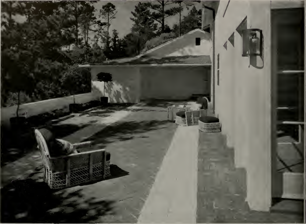
RESIDENCE OF MR. AND MRS. E. C. CONVERSE, CARMEL, CALIF. WILLIAM WILSON WURSTER, ARCHITECT
