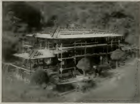
STEEL FRAME HOUSE—Tile shingles stacked on roof ready for laying.
