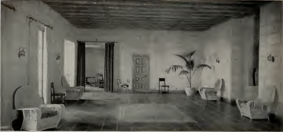
CAST-IN-PLACE CONCRETE FLOORS FOR APARTMENT BUILDINGS AND RESIDENCE. The integrally colored concrete floor finish in this building has been marked off in squares with a cutting tool. Highly polished with wax, this type of floor harmonizes with the quiet dignity of the interior decoration.
