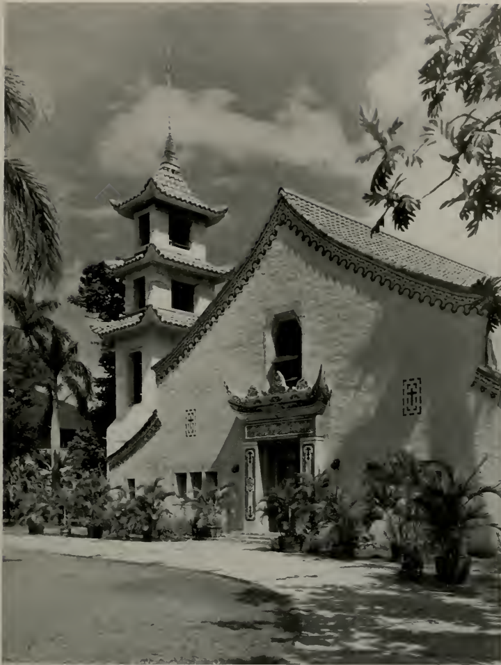
FIRST CHINESE CHURCH OF CHRIST, HONOLULU, T. H. Hart Wood, Architect
